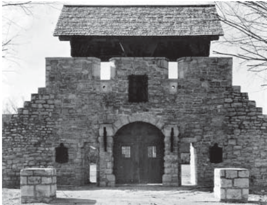
Front gate of Fort de Chartres. Courtesy Illinois Historic Preservation Agency.
