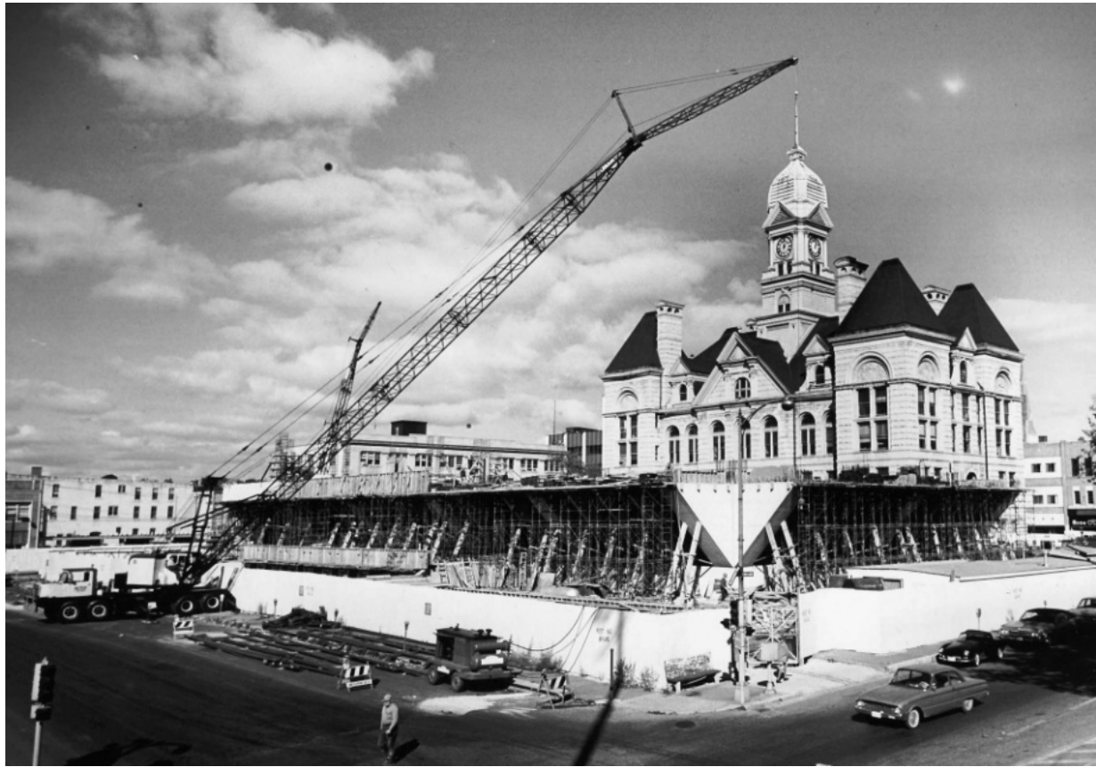
Figure 12: Will County Courthouse under construction, circa 1966 (Courtesy Courthouse Preservation Partnership)
