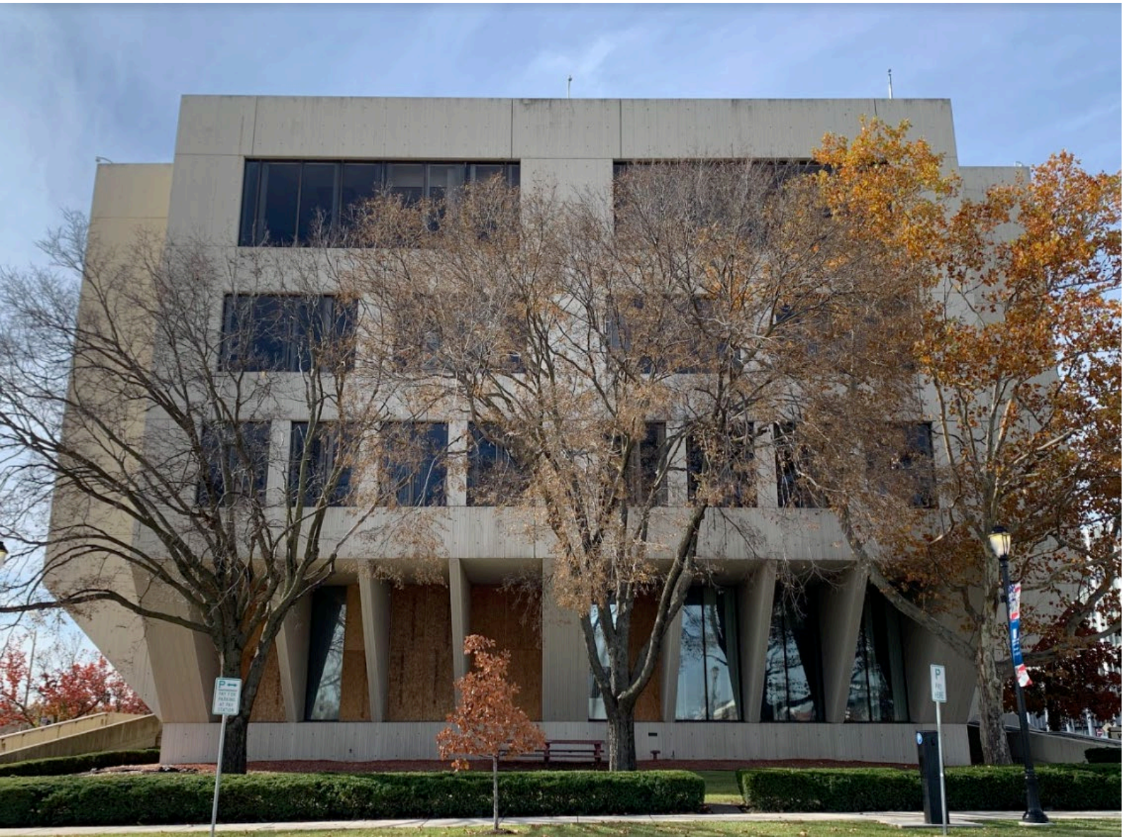
Photo 4: East facade, looking west (Jonathan Solomon)
