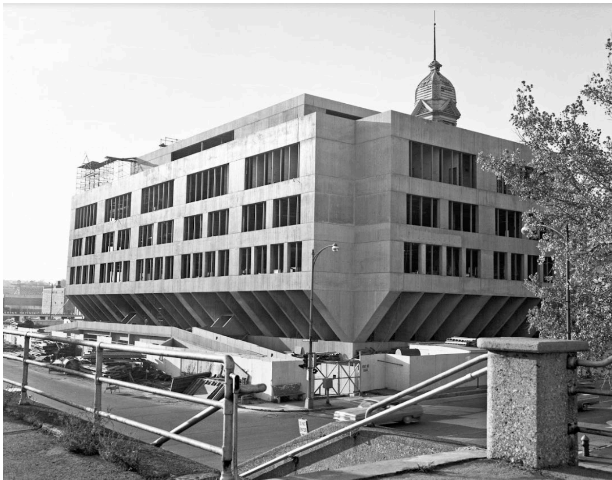
Figure 13: Will County Courthouse under construction, circa 1968 (Courtesy Courthouse Preservation Partnership)
