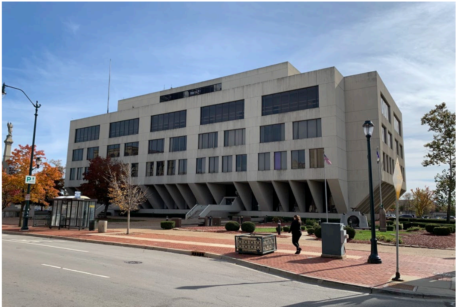
Photo 1: North facade, looking southeast (Elizabeth Blasius)
