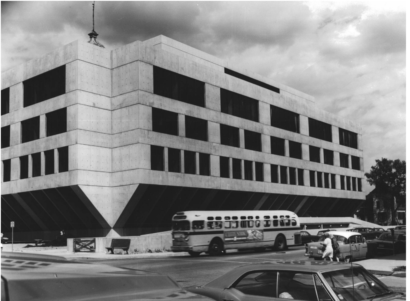
Figure 14: Will County Courthouse, circa 1969 (Courtesy Courthouse Preservation Partnership)
