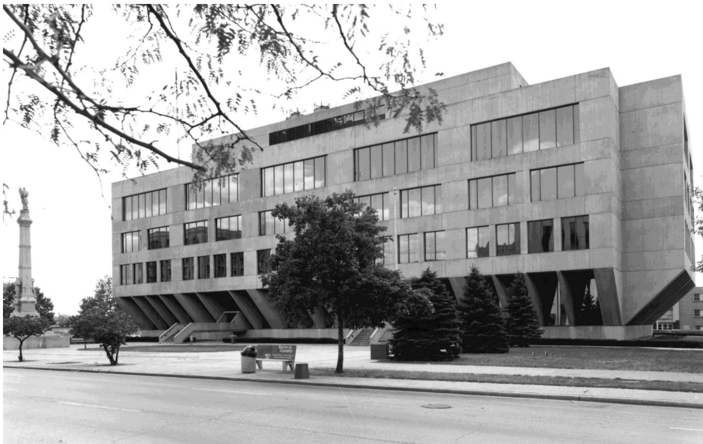
Figure 11: North facade, looking southeast, circa 1969 (Courtesy Courthouse Preservation Partnership)
