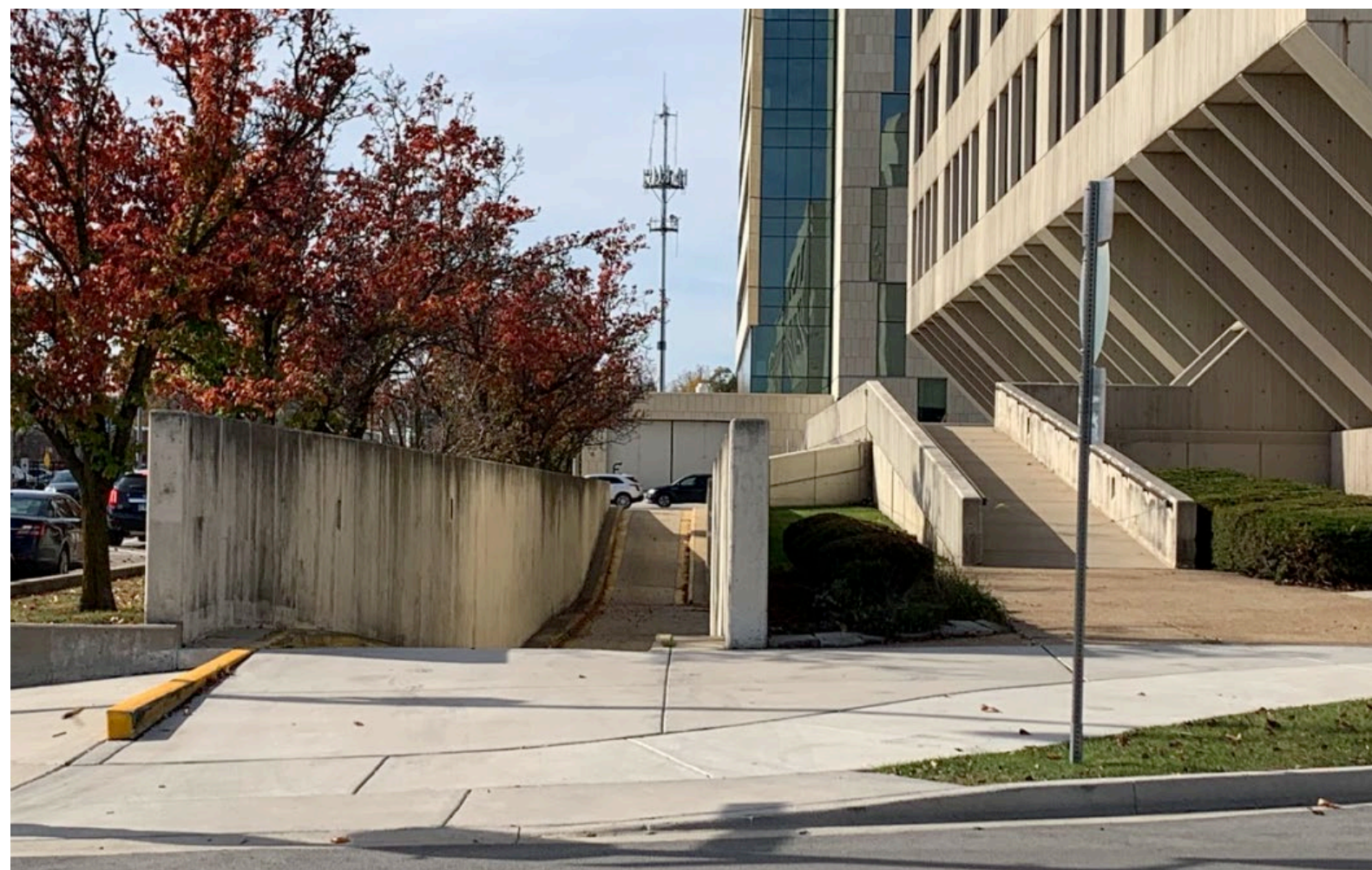
Photo 6: Entrance detail, south facade (Elizabeth Blasius)
