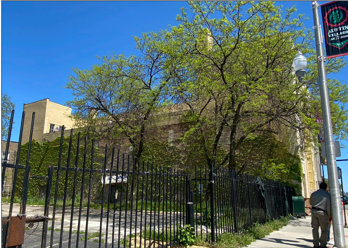
5. West elevation – looking northeast
