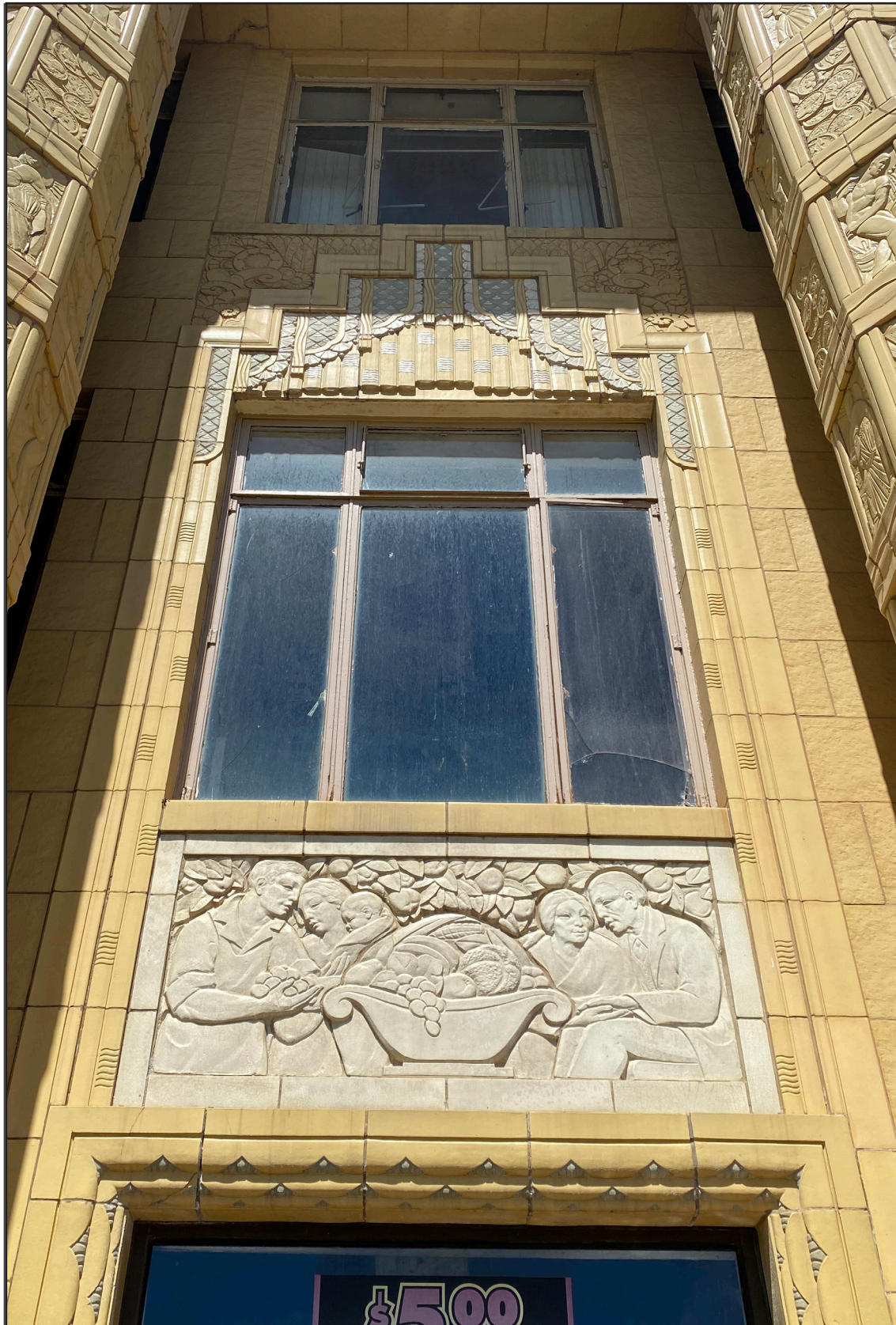
7. South elevation, detail of terra cotta above main entrance – looking north
