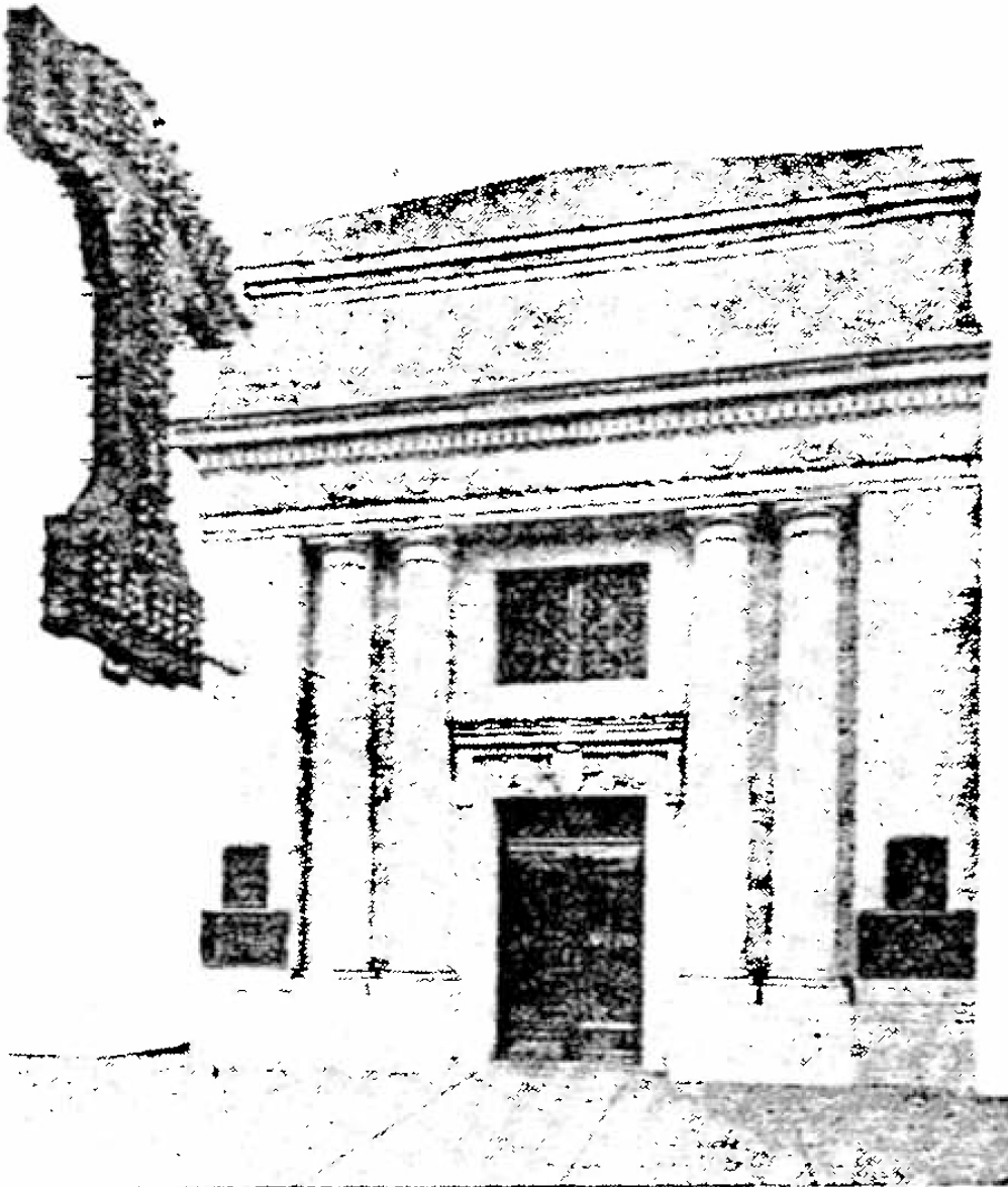
Figure 4. Historic image of Laramie State Bank Building before 1929 remodeling (Chicago Landmarks Commission Designation Report)
