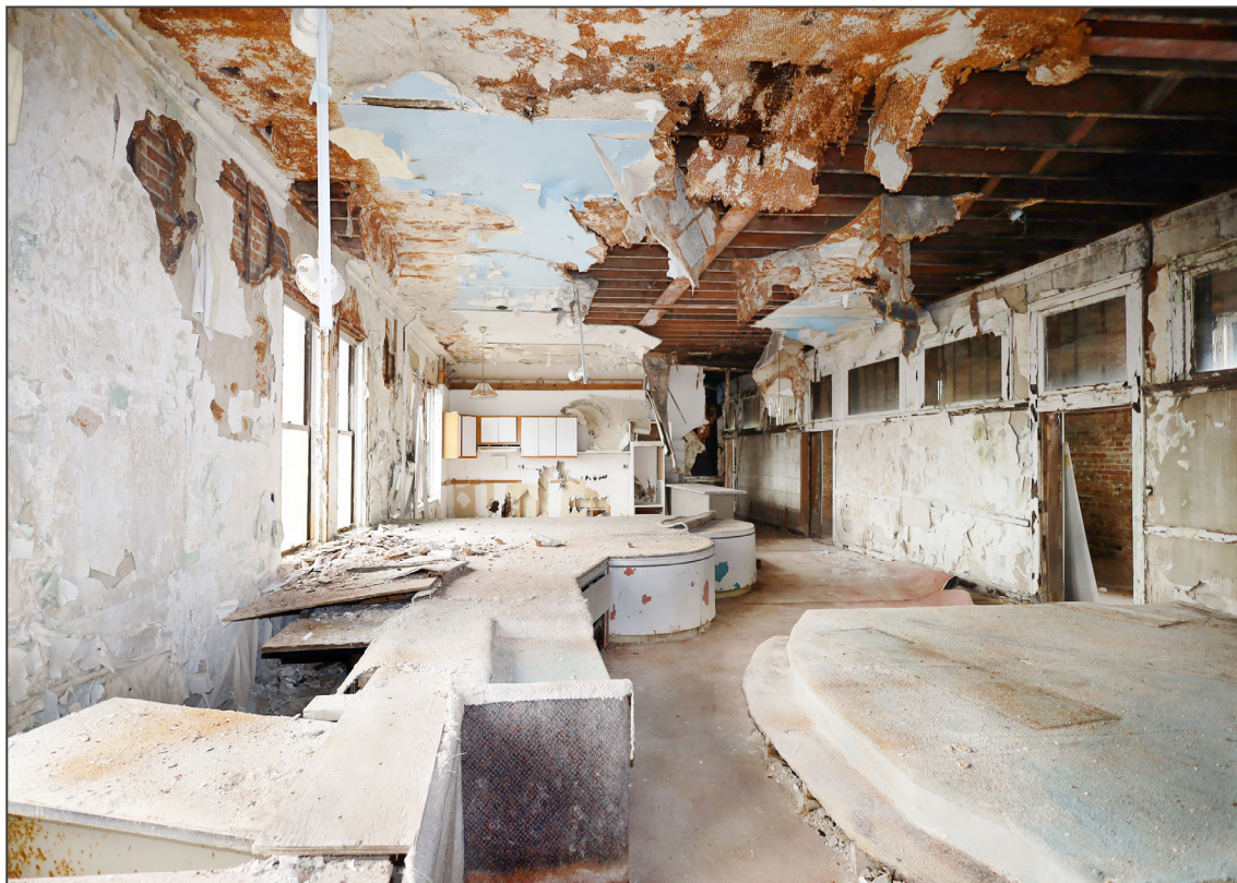
18. Third floor, typical office – looking southwest
