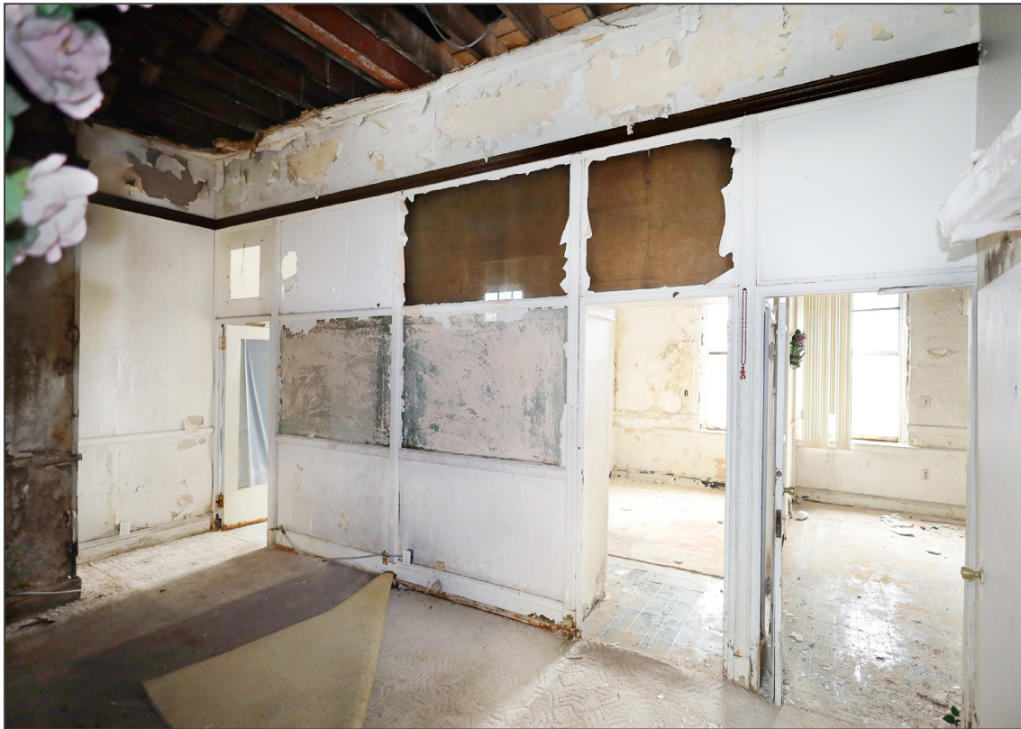
17. Third floor, typical office – looking northeast
