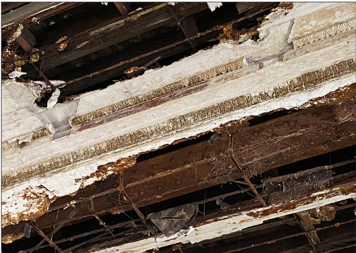
12. First floor, detail of plaster ceiling beam in the banking hall
