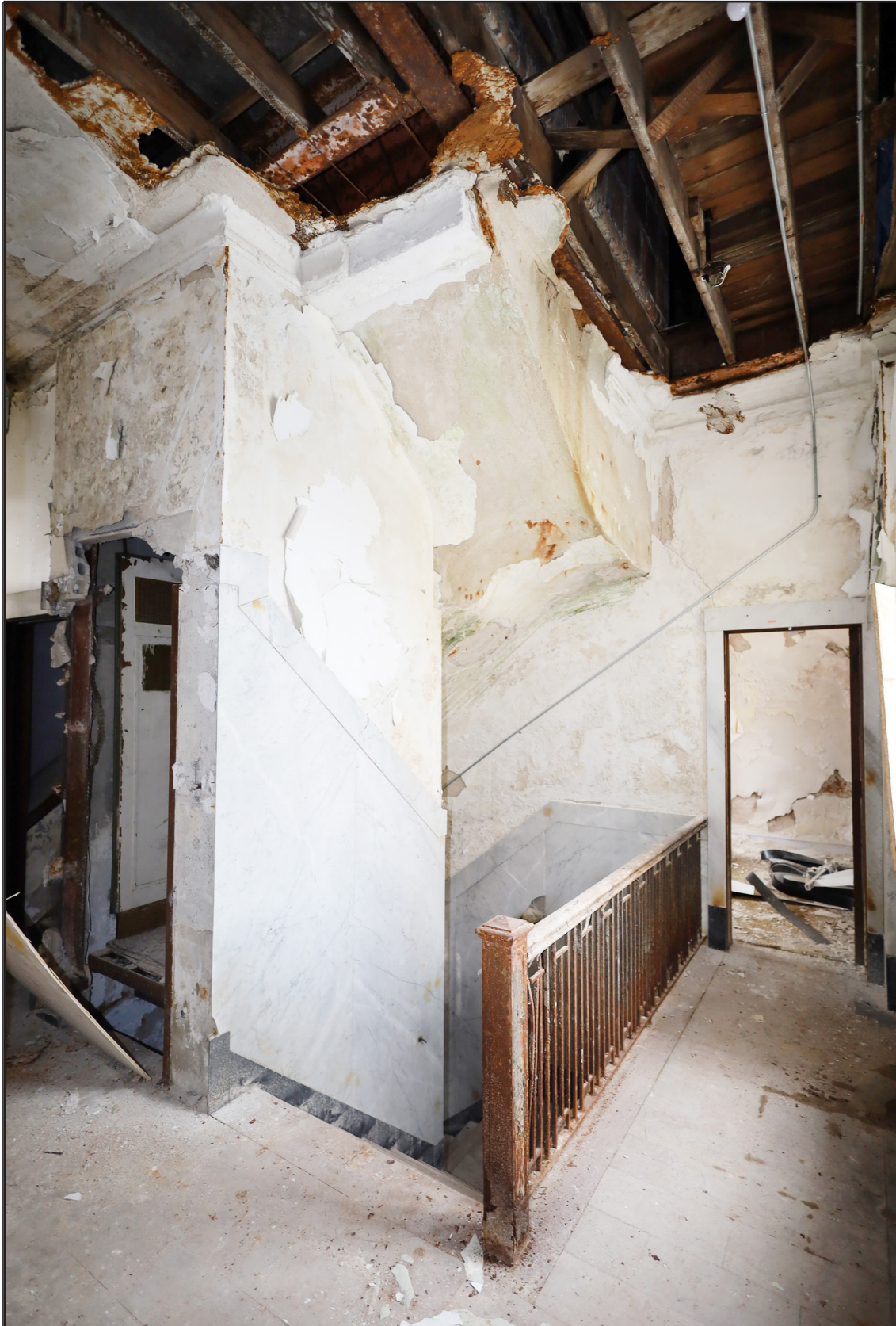
15. Third floor, main stair and elevator at the southwest corner of the building – looking southwest
