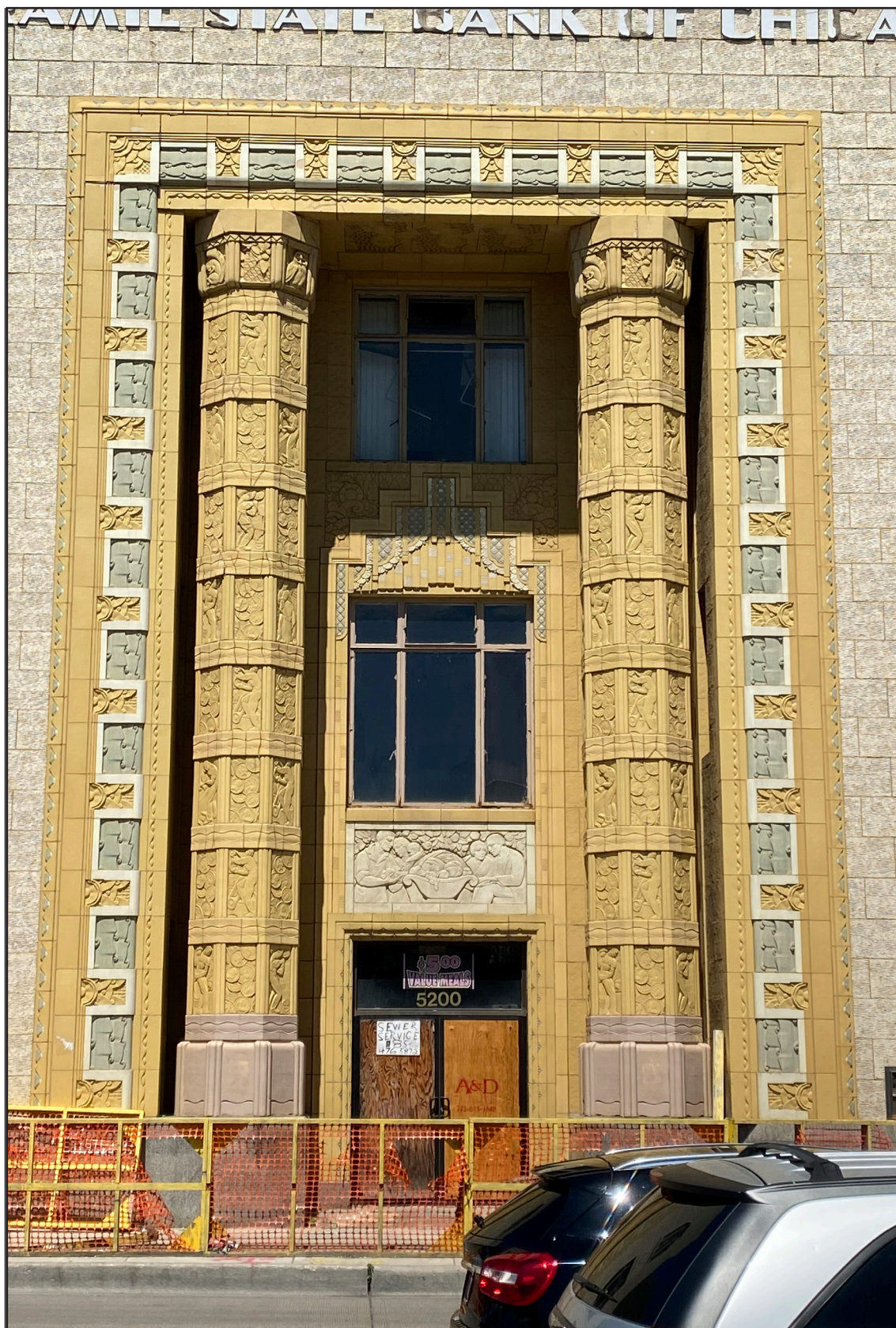
6. South elevation, main entrance – looking north
