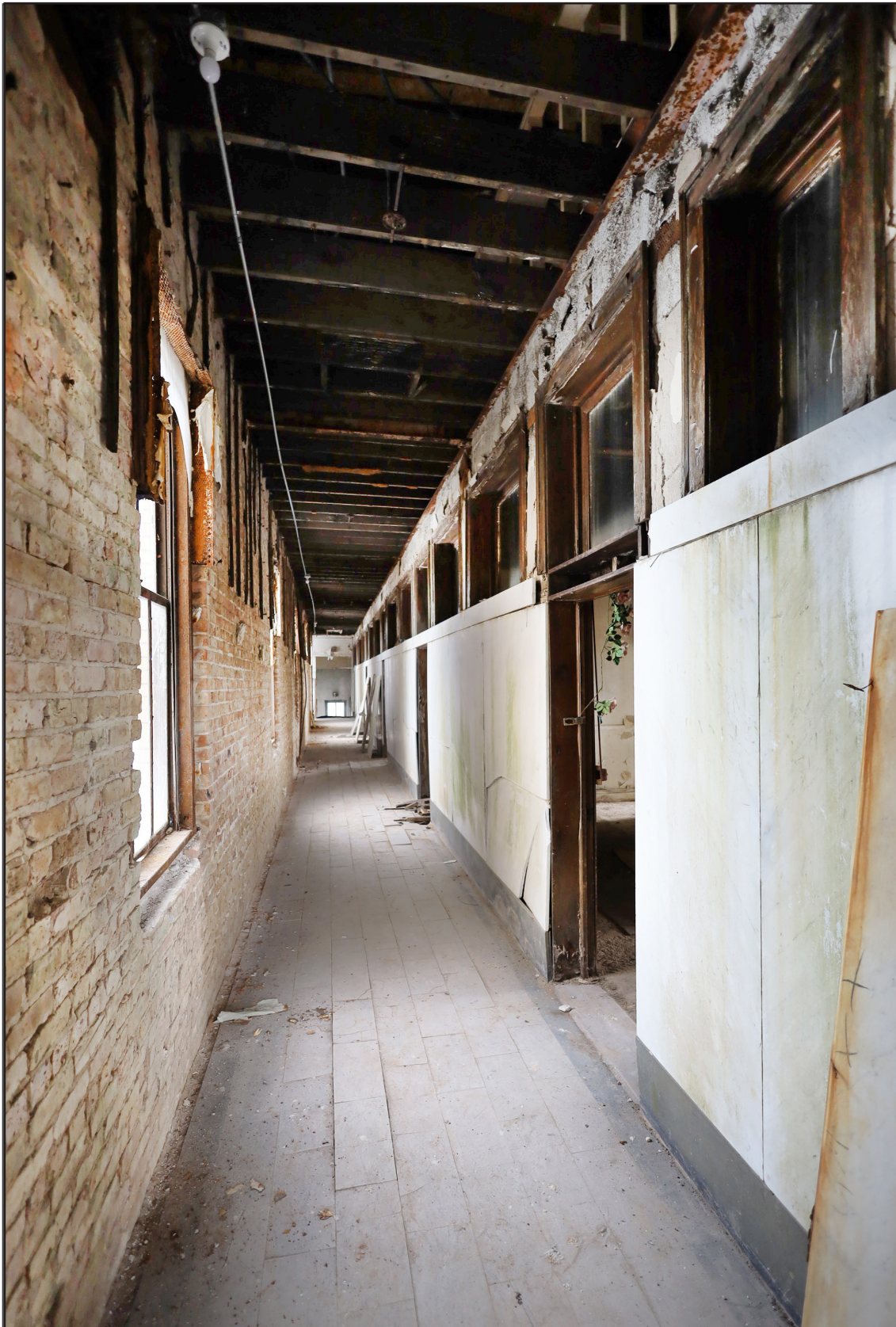
16. Third floor, corridor – looking north
