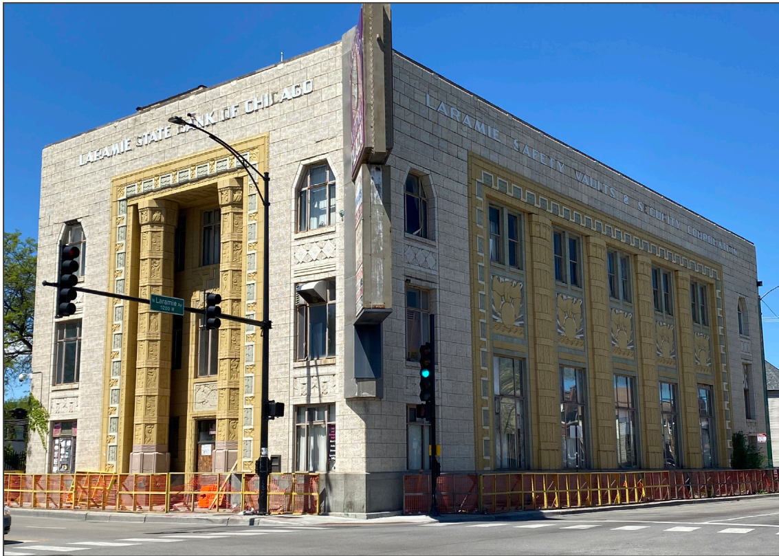
1. South and east elevations – looking northwest
