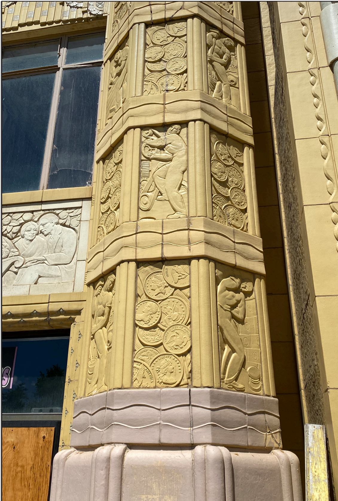
8. South elevation, detail of terra cotta column at main entrance – looking north
