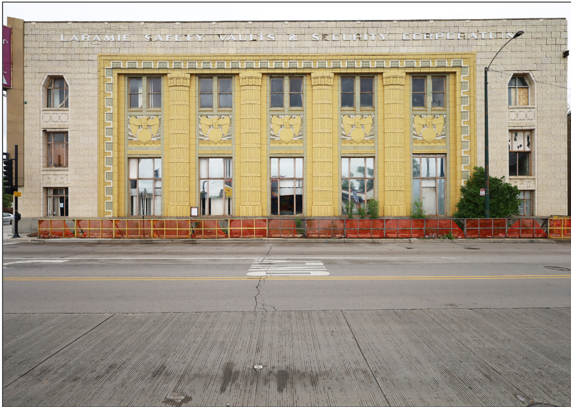
3. East elevation – looking west
