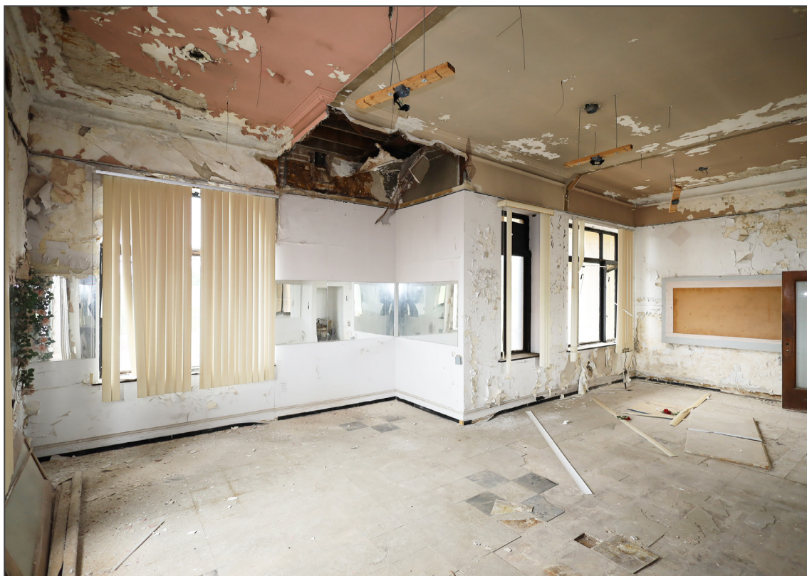
14. Second floor, room south of banking hall – looking southwest
