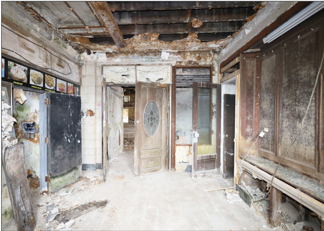
9. First floor, main entrance vestibule – looking north
