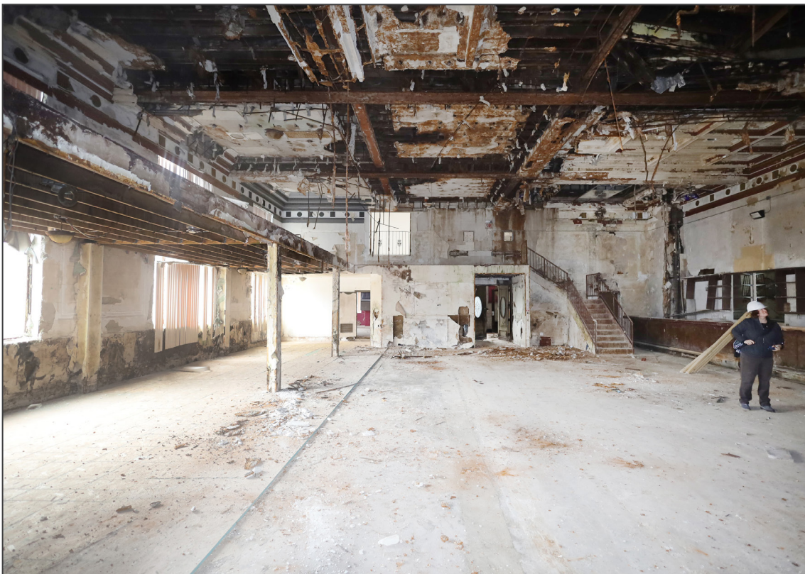
10. First floor, banking hall – looking south
