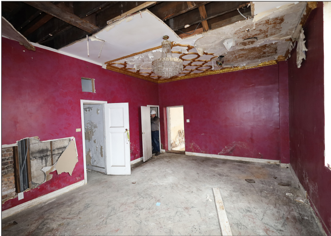
13. First floor, northeast corner office – looking north
