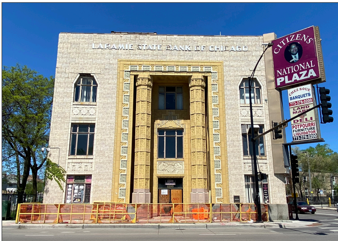
2. South elevation – looking north
