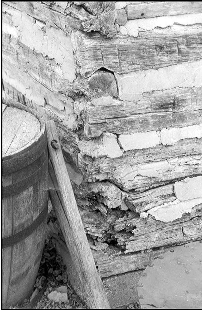
Figure 8. (Left) View of the northwest corner of the cabin, which is badly weathered. (Right) View down the west wall of the cabin (looking north), showing the deflection in the wall (FRR September 2001).
