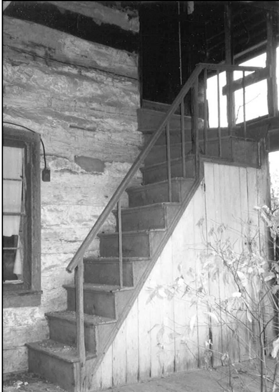
Figure 11. View of the front porch of the Hoerr House, showing the section of log wall that was not covered with siding. The logs have been coated with whitewash to provide a more finished appearance, as well as to protect them from infestation by insects. The exterior stairway shown provides the only access to the upper floor of the house (FRR October 1996).
