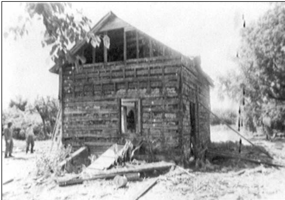
Figure 1. Two views of the Zeine Cabin during the course of its dismantlement in 1974. (Top) Oblique view, showing the present west and south elevations of the cabin. The demolition debris in the foreground is from a later frame addition. (Bottom) View of the cabin after the partial clean up of demolition debris. The gable-end wall shown is now the north elevation of the building. Note the bulkhead entrance to the cellar (WPSP August 1974).
