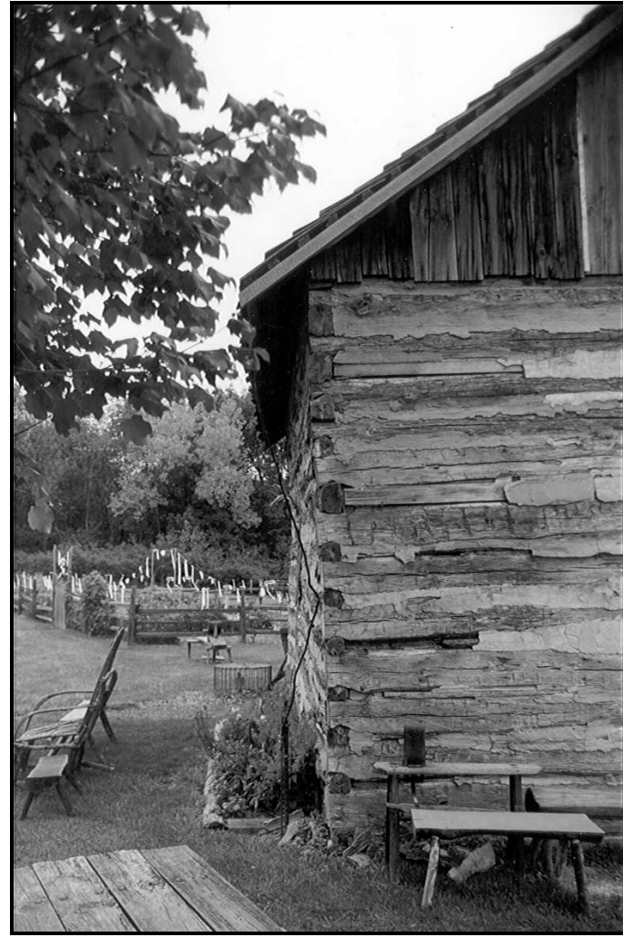
Figure 8. (Left) View of the northwest corner of the cabin, which is badly weathered. (Right) View down the west wall of the cabin (looking north), showing the deflection in the wall (FRR September 2001).
