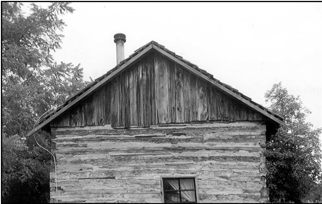
Figure 13. (Top) Detail of an 1974 photograph of the Zeine Cabin, showing the remnants of the horizontal siding originally used to enclose the north gable (WPSP August 1974). (Bottom) View of the vertical plank siding that currently encloses the north gable (FRR September 2001). It is recommended that the vertical planking be replaced with horizontal siding in event that the exterior of the cabin is sided.
