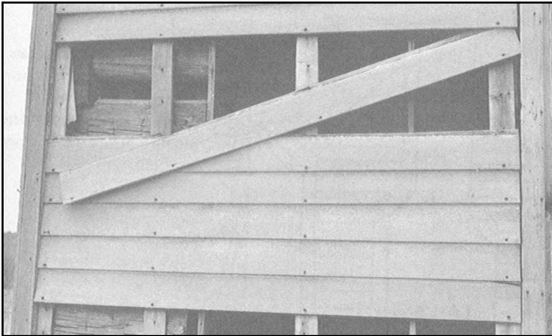
Figure 12. Two views illustrating the manner in which horizontal siding was attached to log buildings using vertical furring strips. A similar procedure should be used on the Zeine Cabin. (Top) The Barth House, in rural Carroll County, Illinois (Stratton and Mansberger 1998:39). (Bottom) A log house in southern Indiana (Roberts 1996:plate 14).
