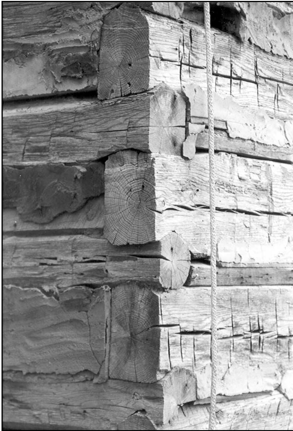
Figure 4. Detail of the northeast corner, showing the corner notching and hewing methods utilized in the construction of the cabin (FRR September 2001).
