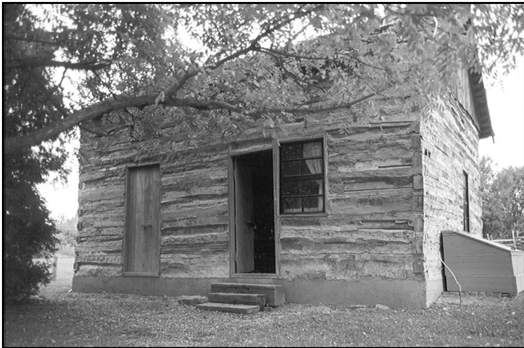
Figure 3. (Top) Oblique view, showing the west and north elevations of the cabin. (Bottom) View of the east elevation. The presence of two doorways here suggests that an addition may have once been present on this side of the dwelling, as was the case on the opposing elevation (FRR September 2001).
