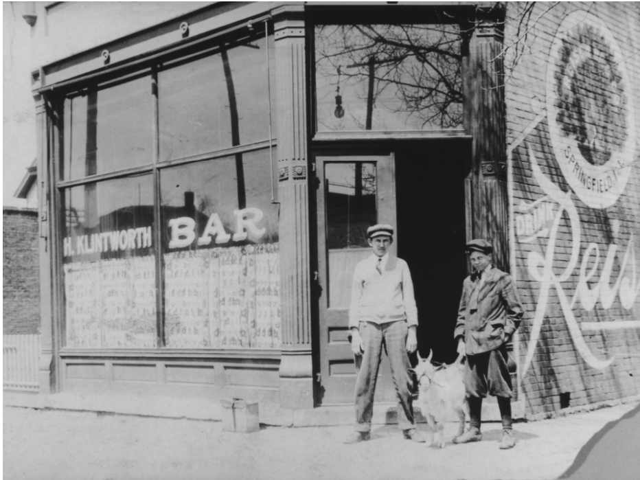
Figure 45. Henry Klintworth's tavern at 1231 East Cook Street, circa 1909. This commercial building was added onto the front of a pre-existing house by 1890. It originally was a meat market (Sangamon Valley Collection).
