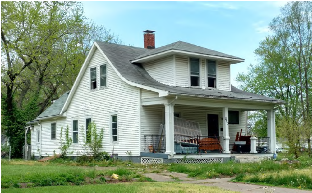
Figure 227. A side-gabled bungalow at 823 South Fifteenth Street. This home was built by Oscar Birdsong, an African-American building contractor, in 1911. He resided here until his death in 1958. This home is located within the survey area.
