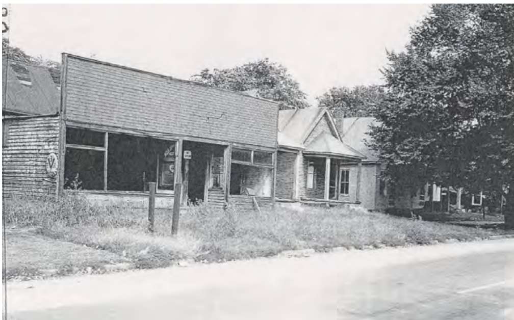
Figure 91. Photographs taken in September 1962, presumably for the Springfield Housing Authority, illustrating the character of the derelict buildings in the proposed urban renewal area along east Washington Street. These pictures depict a series of small frame cottages. Top: Looking northwest across Thirteenth and Washington Streets. Bottom: Looking northeast from Twelfth and Washington Streets (SVC).
