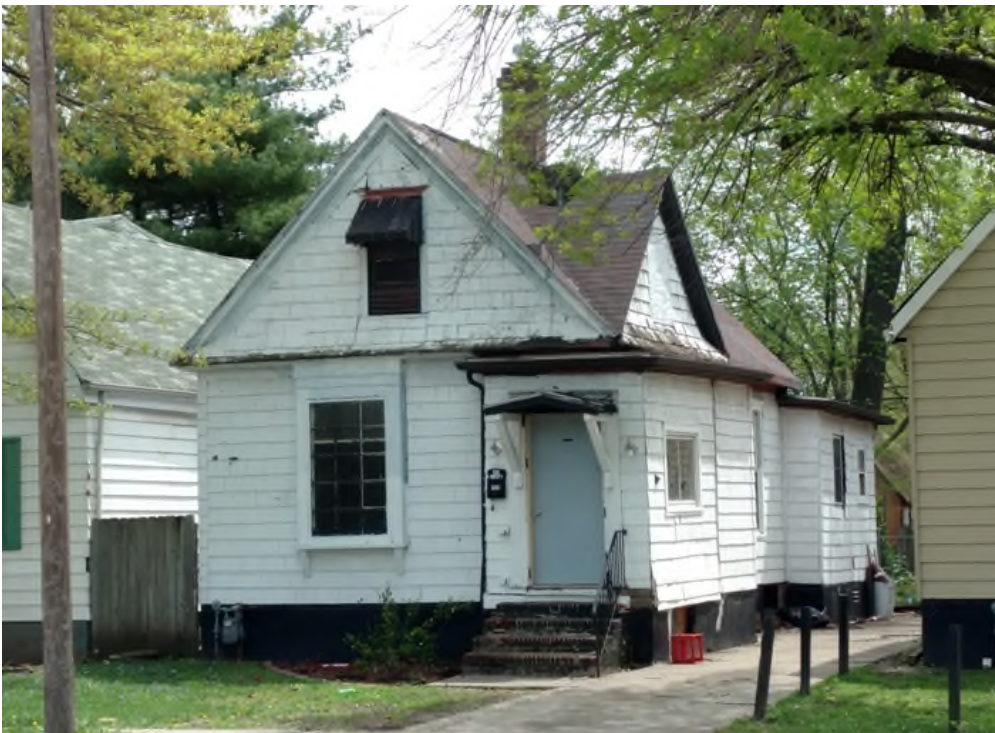
Figure 191. Side-Entrance, Front-Gable Cottage at 1610 East Cook Street. The side entrance porch has been enclosed.
