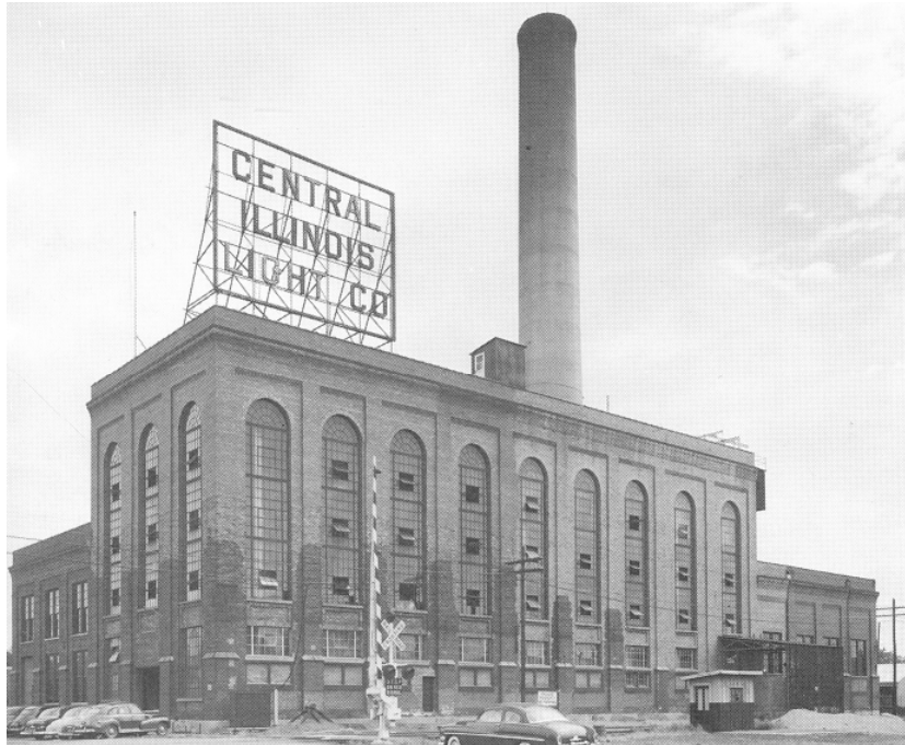
Figure 47. Central Illinois Light Company (CILCO) plant at Tenth Street and Capitol Avenue, as pictured in the 1950s (Russo et al. 1998:30). Built in 1906, this plant occupied a half-block area and replaced a row of single-family houses formerly located here. The plant underwent several major remodelings over the years, including the addition of two new boilers in late 1925.
