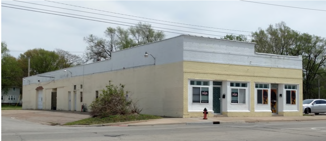
Figure 207. One-Part Commercial Block at 600-604 South Eleventh Street. This building was constructed in two episodes, with the section left being earlier.
