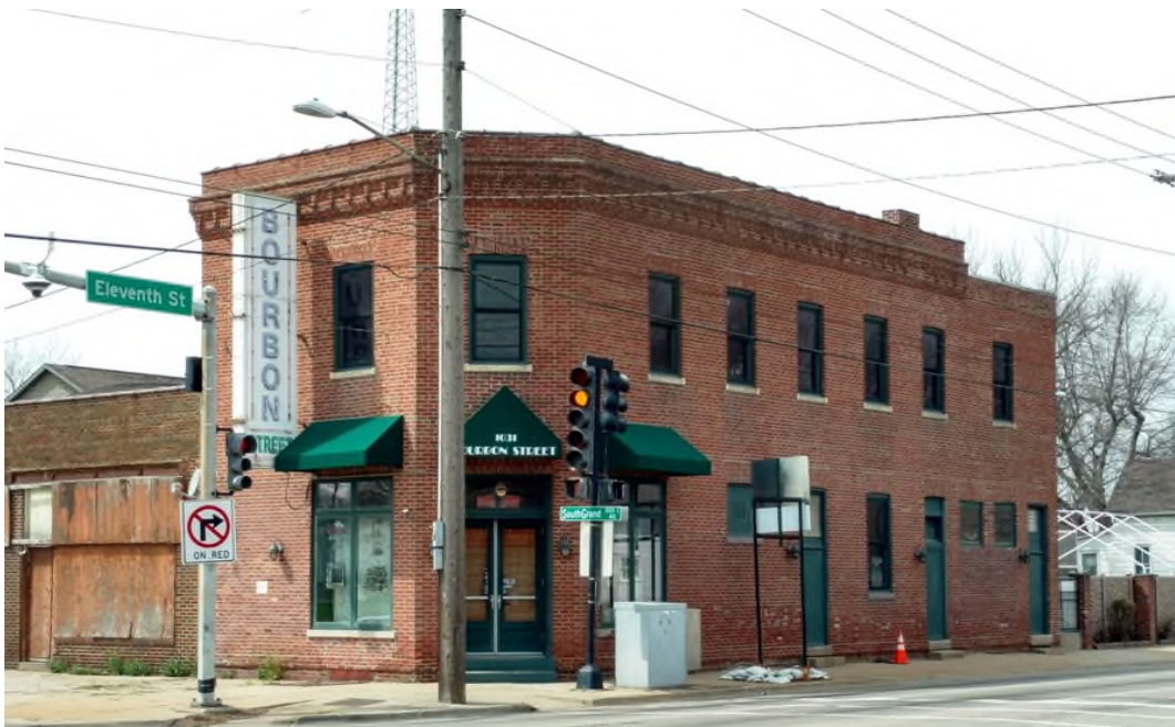
Figure 208. Two-Part Commercial Block at 1031 East South Grand Avenue. This building occupies the northwest corner of South Grand Avenue and Eleventh Streets.
