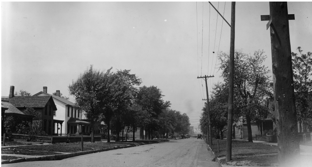
Figure 44. Washington Street at Thirteenth Street, looking west. The street is paved, and automobiles appear in the background. This block represented the eastern end of the commercial district along Washington Street. Several one-story, frame commercial buildings (looking a little worse for wear) appear in the distance at right.
