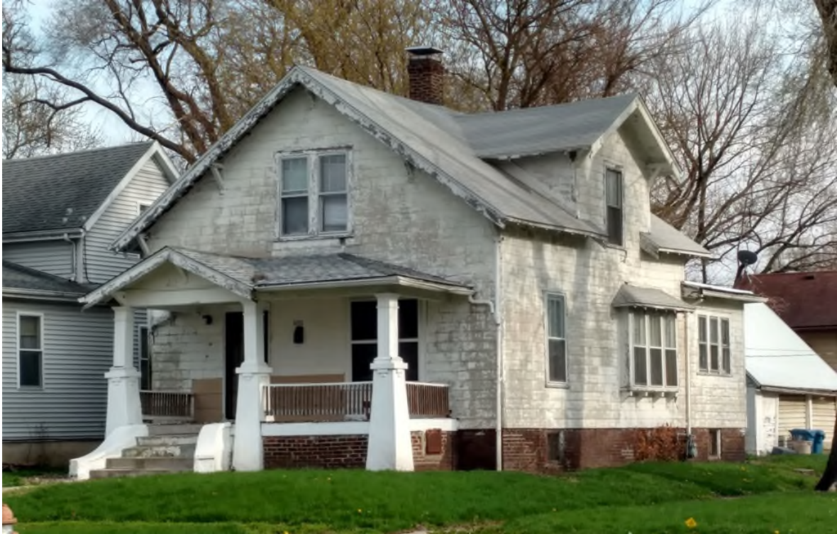
Figure 179. Craftsman-style Front-Gabled Cottage at 1400 East Edwards Street. Note eave brackets and battered porch piers.
