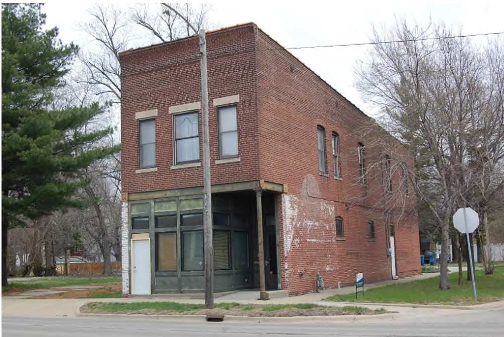
Figure 210. Two-Part Commercial Block at 930 South Eleventh Street, constructed in circa 1900-02 for Jacob Rosenweig. It provides commercial space on the first floor and residential space on the floor above. Originally upstairs may have been Rosenzweig Hall.
