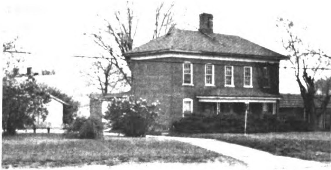
Figure 4. One of the few structures documented by earlier surveys within the Central East Neighborhood: The Burns House, located at 1625 West Jefferson Street. Constructed immediately after the Civil War, and later occupied by Michael H. Burns, a teamster in the Civil War who purchased the house in 1884 (IDOT 1980:I-72 and I-73; Barringer 1966).
