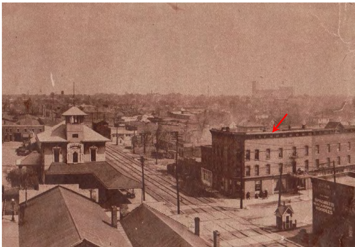
Figure 119. View of the Tenth Street corridor, looking north/northeast from a point between Washington and Adams Streets in 1931 (likely taken the roof of the Bunn Warehouse). The towered building seen in middle distance at left is the Wabash Railroad's passenger depot. The building directly opposite from the depot (marked with red arrow) is the Wabash Hotel. By 1950 The Wabash Hotel operated under the name "Hotel Ferguson," which catered to black clientele. The commercial block adjoining the hotel also rented rooms to black borders (SVC; ? 1931)
