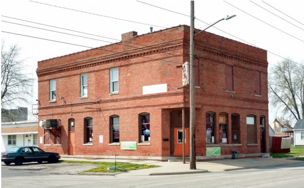
Figure 209. Two-Part Commercial Block at 1029-1031 South Eleventh Street. This building was constructed in two episodes, with left-hand section coming first (circa 1910), followed by right-hand third in circa 1930. Once expanded, it provided two storefronts. The upper floor serves as a meeting hall.
