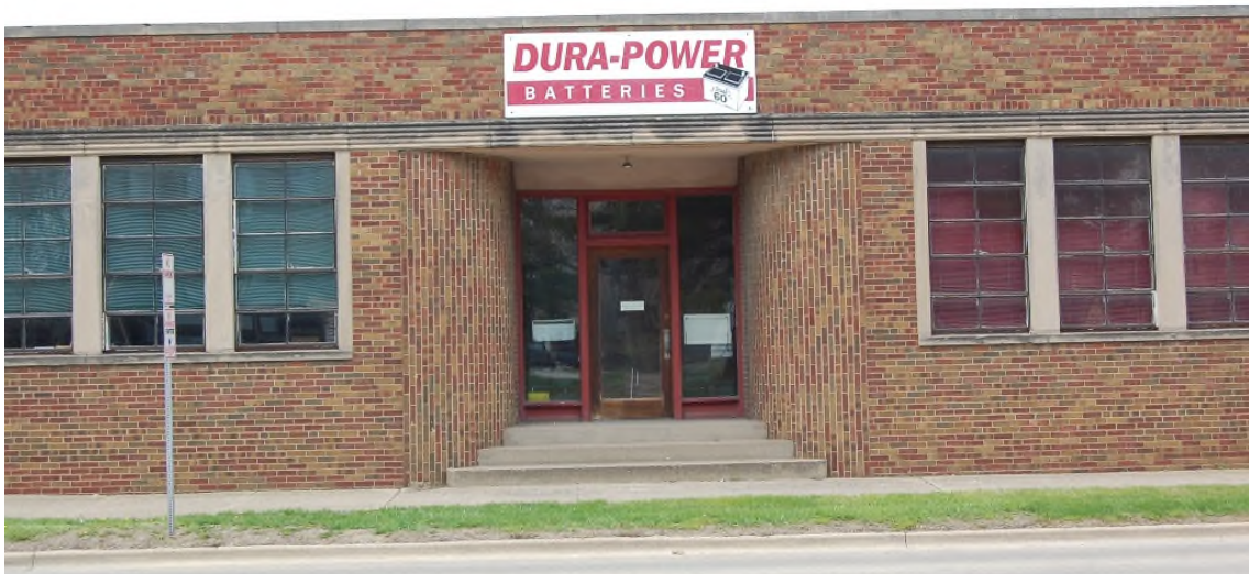
Figure 182. The battery factory at 931 South Eleventh Street has an Art Moderne-influenced front entrance, ribbon windows, and wall banding.
