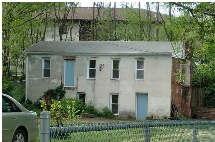
Figure 235. (Top) A 1917 Sanborn map illustrating the commercial laundry owned by W. H. Murrell at 1240 West Jefferson Street, on the west side of Springfield. Murrell resided on the same lot. (Bottom) Present-day view of the former laundry.
