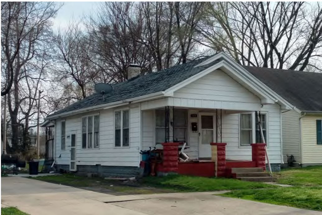
Figure 118. Although over 20 tourist homes were listed in the various Negro Green Books published over the years, only two have survived to the present. B. Eskridge Tourist House (1501 East Jackson Street) (top) and the H. Robbins Tourist House (1616 East Jackson Street).
