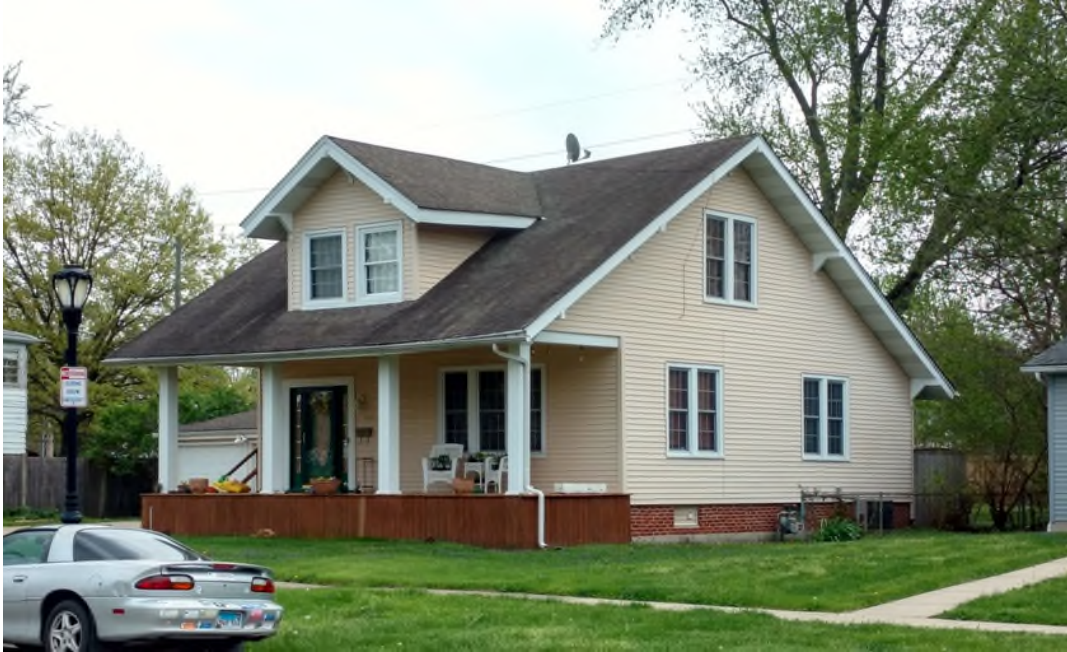
Figure 199. Side-gabled Bungalow at 1516 East Capitol Avenue.
