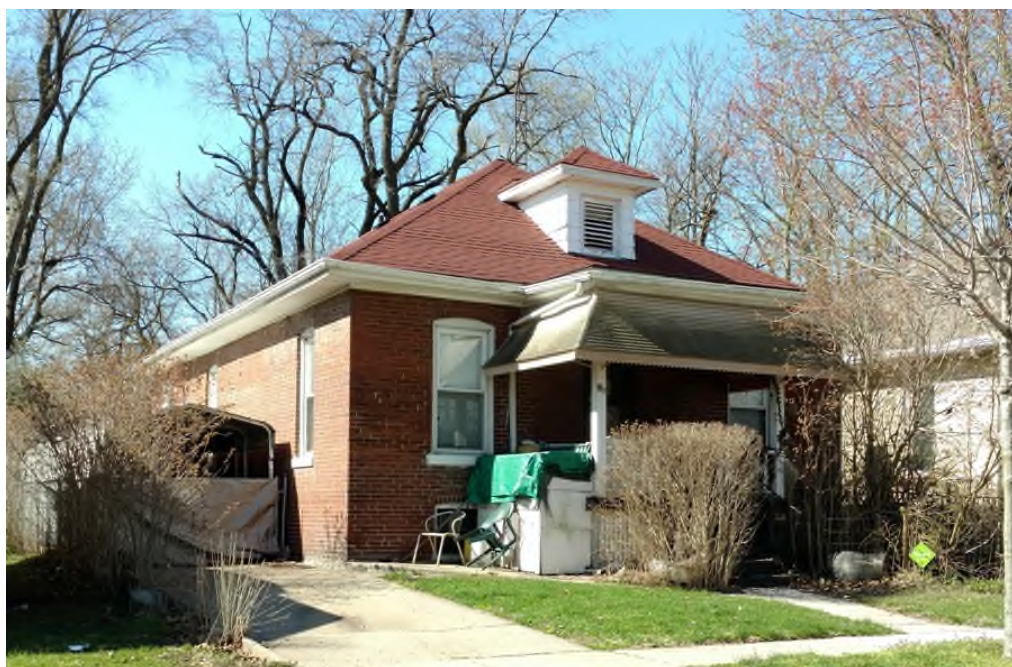
Figure 202. Hip-Roofed Cottage at 712 East Clay Street. This is one of two adjoining brick cottages of this form.
