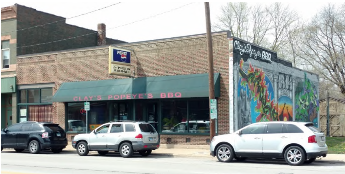
Figure 225. This building at 1121 South Grand Avenue served as the Lincoln Library's South Branch from January 1927 until September 1983. It is located just outside the survey area. The branch library would have served an important institutional role for the surrounding neighborhood during its 56 years of use as a library. Clay's Popeye's BBQ—a noted black-owned eatery presently occupies the building.
