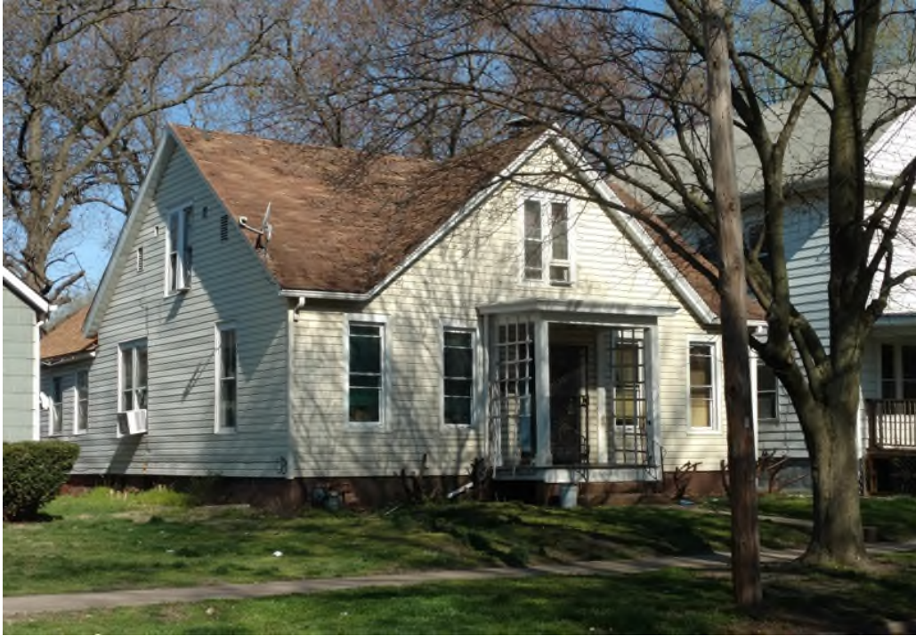
Figure 203. Side-Gable Cottage at 1203 South Twelfth Street.
