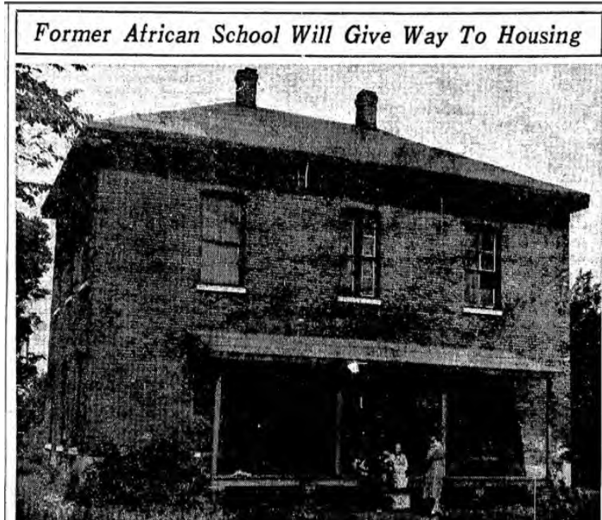
Figure 139. View of the former African School of Springfield, once located at 319 North Fifteenth Street. This picture was taken in June 1940 in anticipation of demolition for urban renewal. At the time, the building was being used as the home of Mrs. Edna Dorsey, who was being relocated due to the urban renewal project ( Illinois State Journal , 28 June 1940)
