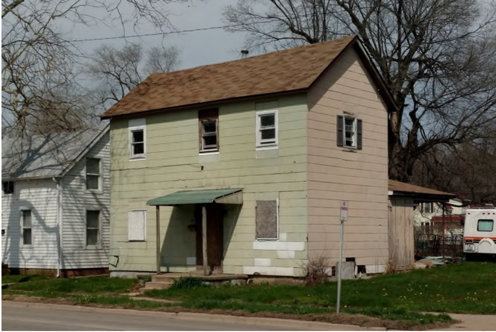
Figure 187. I-House at 1024 South Eleventh Street. This dwelling also pre-dates the Civil War.
