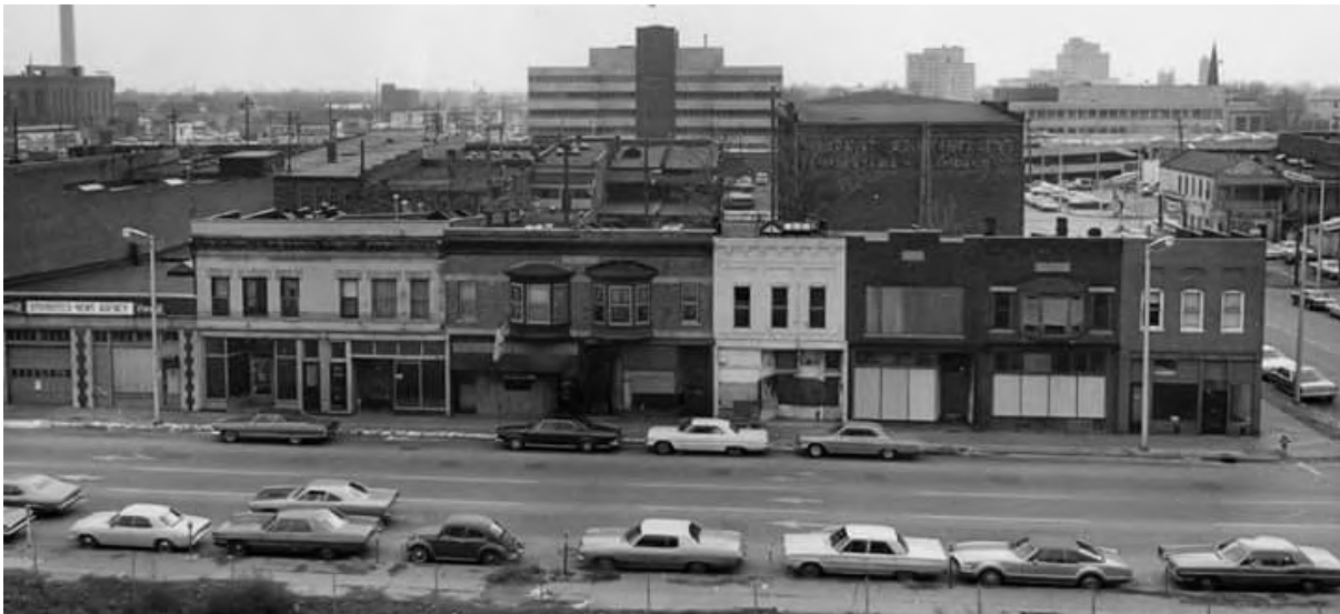
Figure 86. Two views of the south side of Washington Street, between Eighth and Ninth Streets. This area was once within the heart of the black commercial district known as the Levee. [SVC; 1960s images... Civic Center is under construction.]
