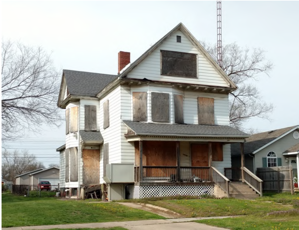
Figure 175. The Queen Anne residence at 1225 East Edwards Street. This home is one of the largest examples of Queen Anne architecture in the survey area and exhibits the “Free Classic” detailing typical of the style’s later period.
