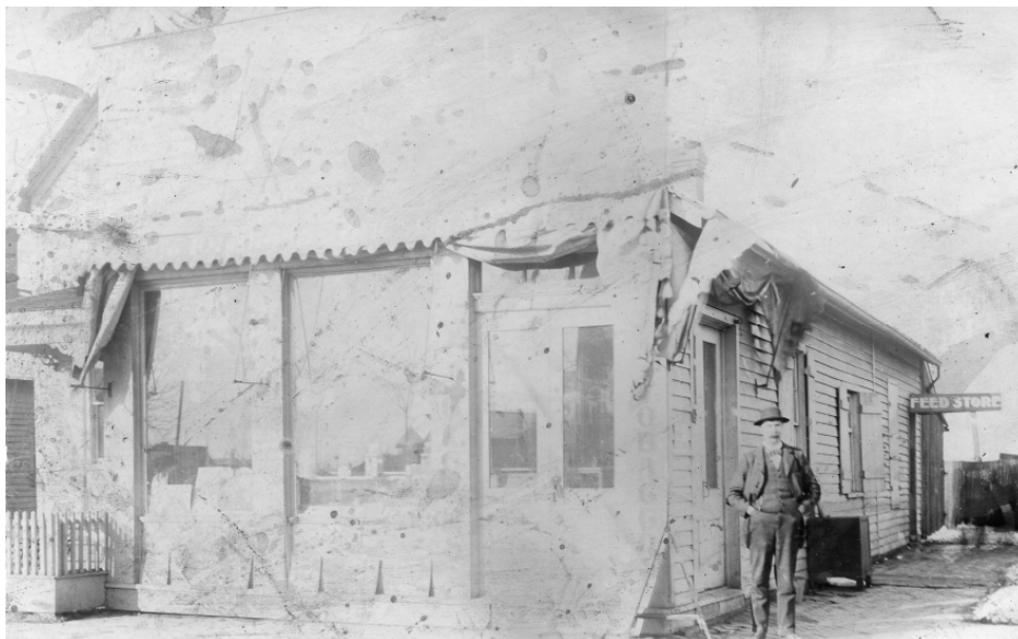
Figure 36. Charles Gallagher cigar and tobacco shop at 1031 East Capitol Avenue circa 1900. This one-story frame building, with raised false front, likely is typical of the early store buildings constructed with within the project (Sangamon valley Collection).
