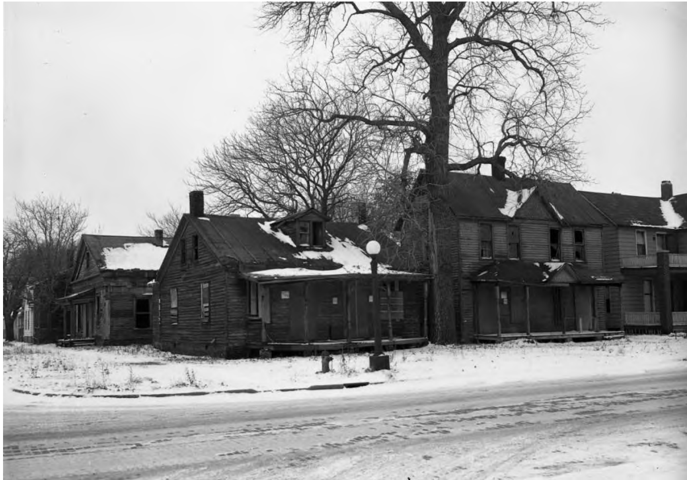
Figure 90. By the middle 1960s, many landowners in the Central East Neighborhood had allowed their properties to decline, and the older housing stock in the neighborhood had begun to show signs of neglect, soon followed by large scale demolitions. These dilapidated houses located at Thirteenth and Adams Street photographed in late January 1965, represent traditional house forms associated with the Central East Neighborhood (Mercury Studio Collections, Lincoln Library).
