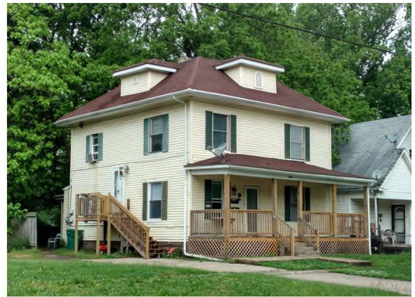
Figure 95. Residence of Frank Burns, located at 1213 S. Fourteenth Street ( Illinois State Journal , 21 July 1918).
