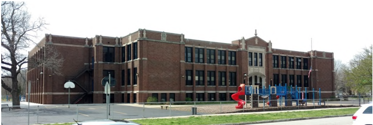
Figure 212. Feitshan School at 1101 South Fifteenth Street, built in 1922 in the Collegiate Gothic style. In 1929, it was converted to a high school (to supplement Springfield High)—a role it continued in until 1967. Much of its student body was African-American.
