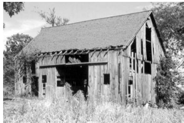
Figure 5-5: This barn, the Hallstein Barn, was constructed in the early twentieth century in Tazewell County, Illinois. An example of an English barn, it features a large entrance to the threshing floor on the eave ends (Stratton 2002).
