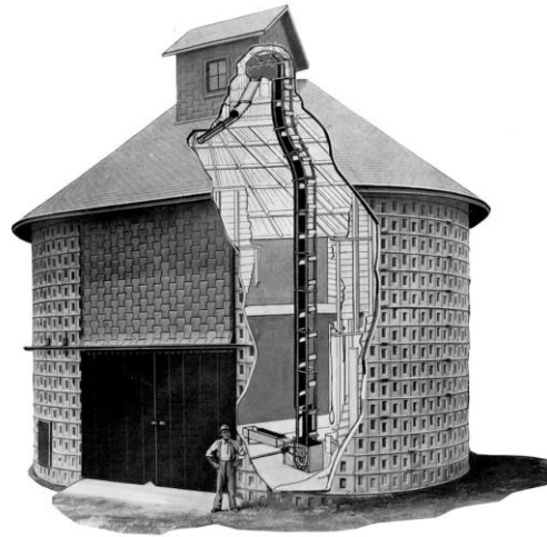
Figure 5-15: An interior elevator was used to deposit the ear corn, off loaded from trucks, which entered through the central door, into the grain bins (McLean County Museum of History 2025).
