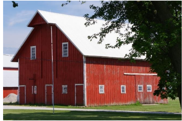
Figure 5-6: Resource JK52 is a transverse-frame barn constructed by French immigrant Michael Keiefer ca. 1890. In Illinois, this form was common from the mid-nineteenth century into the early twentieth century, evolving from earlier three-bay English barns but adapted for mixed farming needs, often with livestock in one or both side bays and mow space above. View looking southeast.
