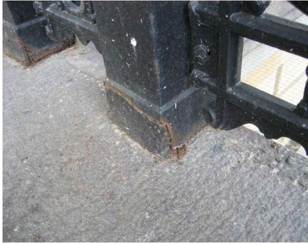
Figure C125. Cracked rail post.
