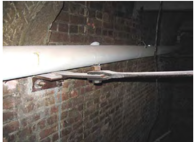
Figure C160. Added steel tie rods, tying drum of dome to load bearing masonry walls of the main structure.
