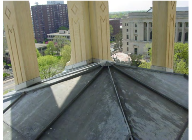
Figure C18. Uneven gray patina on the exposed surfaces of the lead coated copper.
