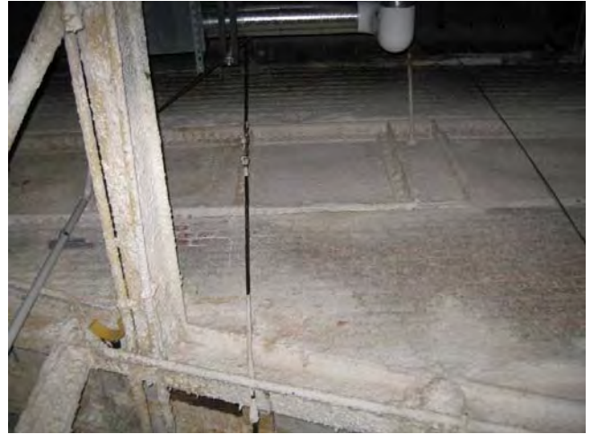
Figure C190. Transfer girder supporting the stone battered base of the dome.
