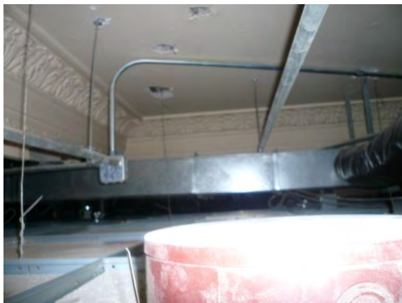
Figure B119. Original decorative plaster ceiling in place above acoustical tile ceiling in Room 216.
