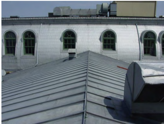
Figure B2. Overall view of a gable roof with a batten seam roofing. Note the flat lock shingles on the mansard in the background.
