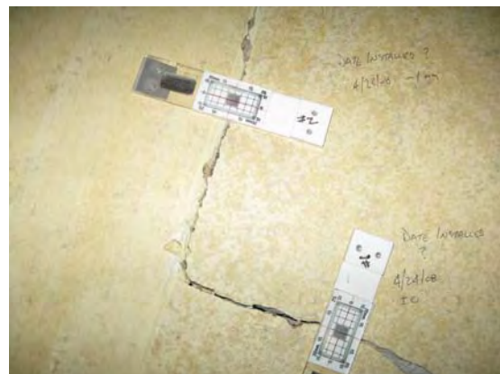
Figure C150. Cracking of the plaster clad masonry arch at the second floor north wing where tell tale monitors have been previously installed.
