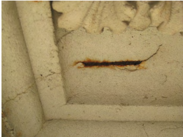
Figure C83. Corroding reinforcing steel at cornice.
