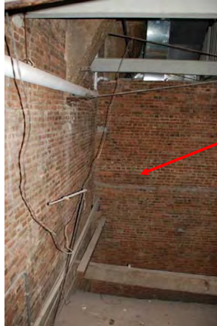
Figure C159. Cracking, indicated by the arrow of the radial wing walls surrounding the inner dome masonry walls.
