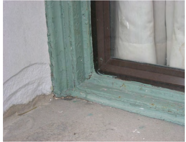
Figure C120. Peeling paint and minor surface corrosion on cast iron windows.
