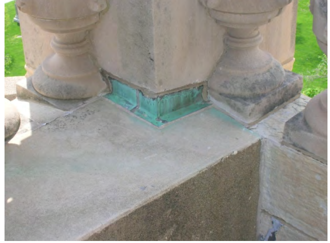
Figure C12. Run off from copper flashings have stained the balustrade.
