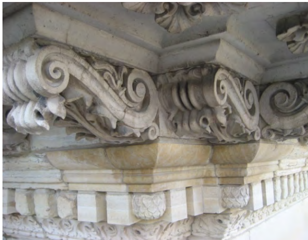
Figure C71. Replacement limestone.
