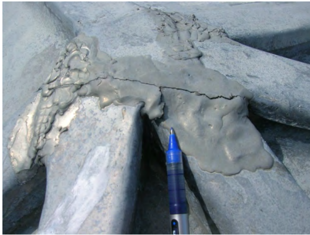
Figure C7. Cracked solder joint at the intersection of multiple battens.
