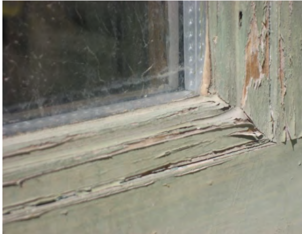
Figure C103. Deteriorated painted wood stop.
