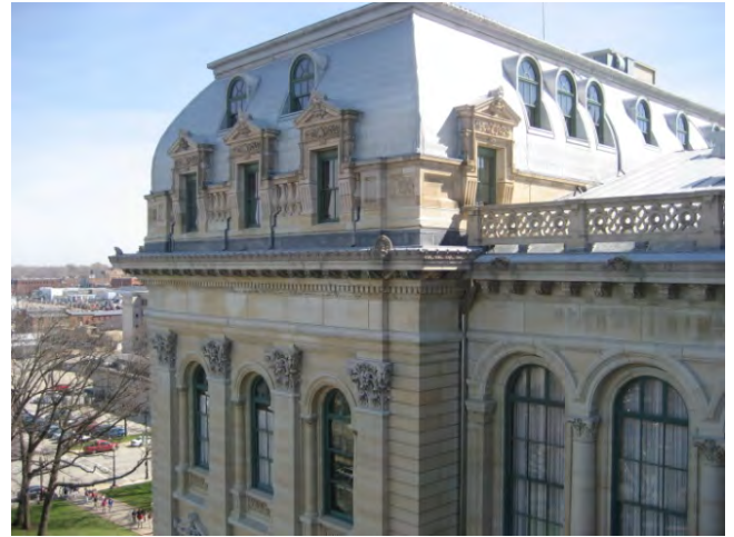
Figure C52. Surface erosion of limestone below cornice.
