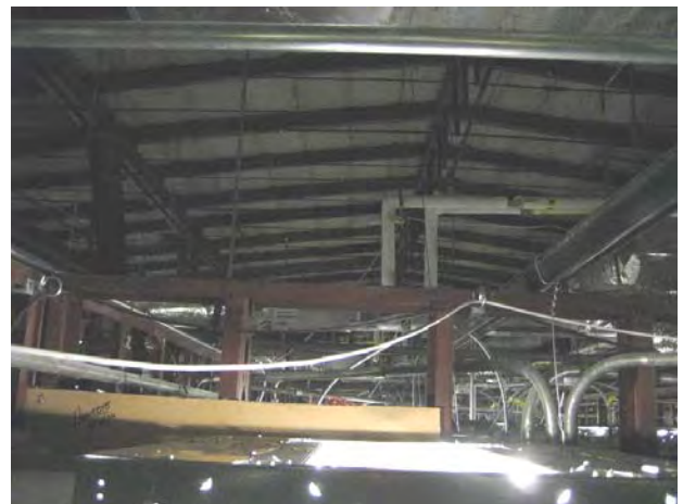
Figure C184. Overall view of mansard roof framing of south wing.
