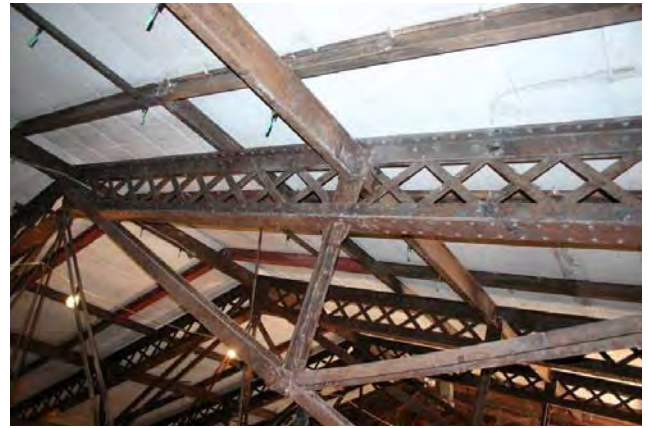
Figure C183. Close up view of wrought iron truss connections supporting roofing above House Chambers (south wing) during renovation.
