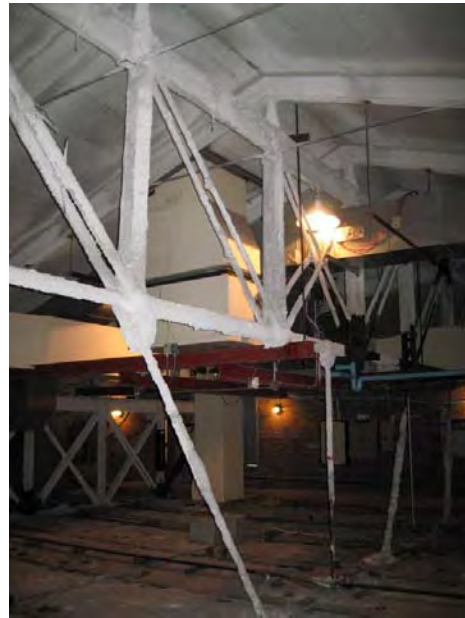
Figure C171. Main high truss supporting the ceiling of the west wing above room 309.
