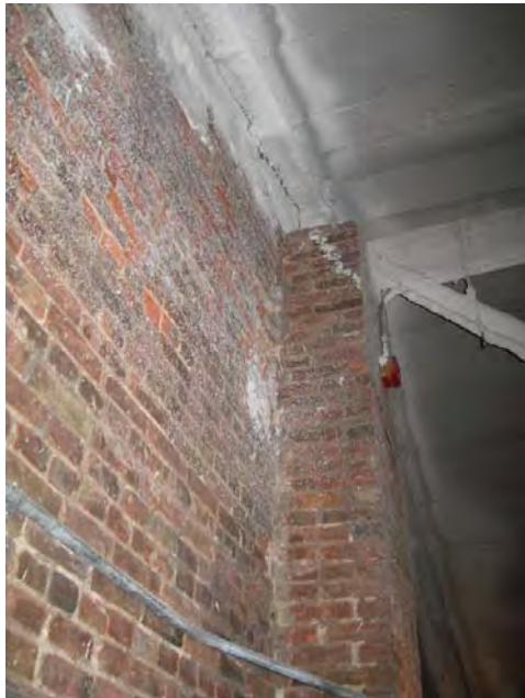
Figure C176. Cracking near roofline between backup masonry wall and roof framing to the south of main high truss.
