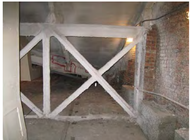
Figure C172. View of one of the main low trusses at west wall.
