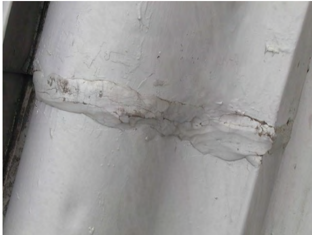
Figure C35. Open joint previously sealed at rib.
