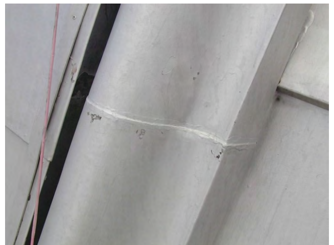
Figure C38. Lapped joint at rib.
