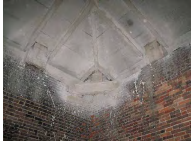
Figure C165. Roof framing of the tempietto structures, showing precast panels and wrought rafters.
