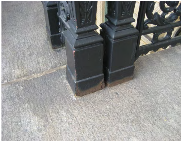
Figure C126. Corrosion of cast iron post.
