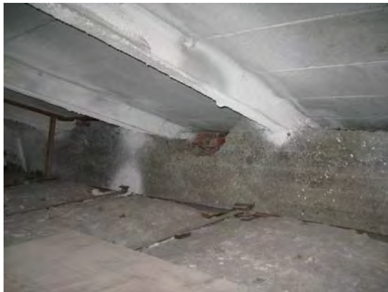
Figure C161. Concrete counterweights cast integrally with cast in place cornice on the exterior, as observed throughout attic spaces.
