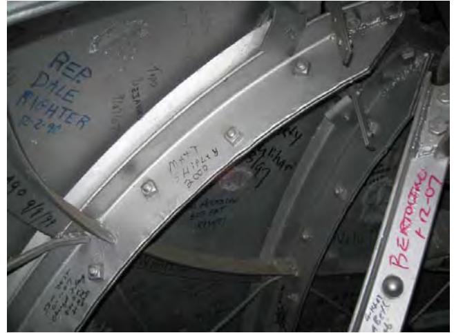
Figure C219. Structural framing of the roofing above the dome lantern consisting of semi-elliptical curved framing elements.
