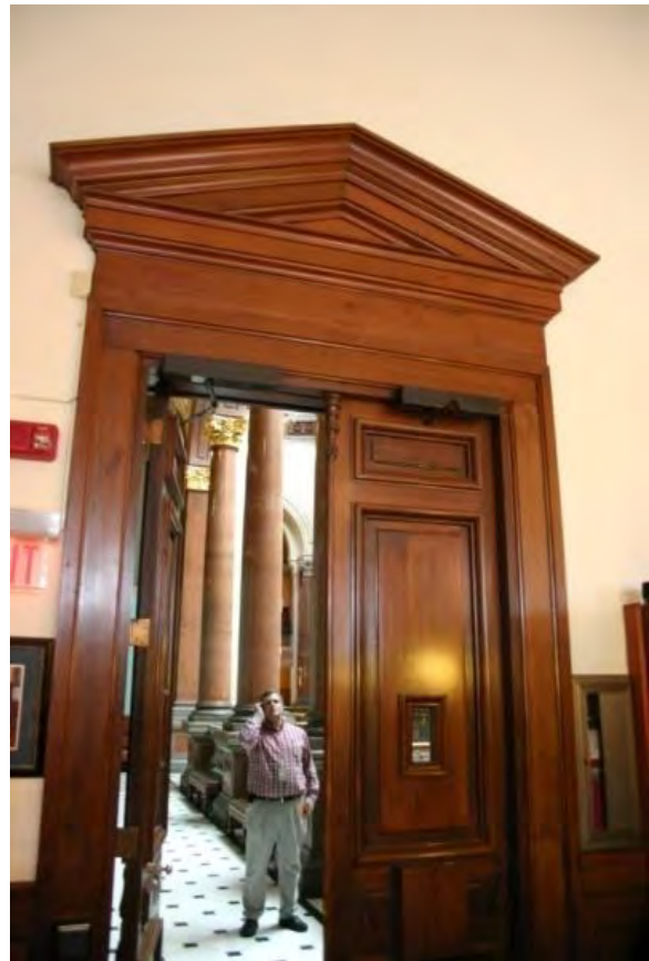
Figure B202. Original doors with their swing reversed.
