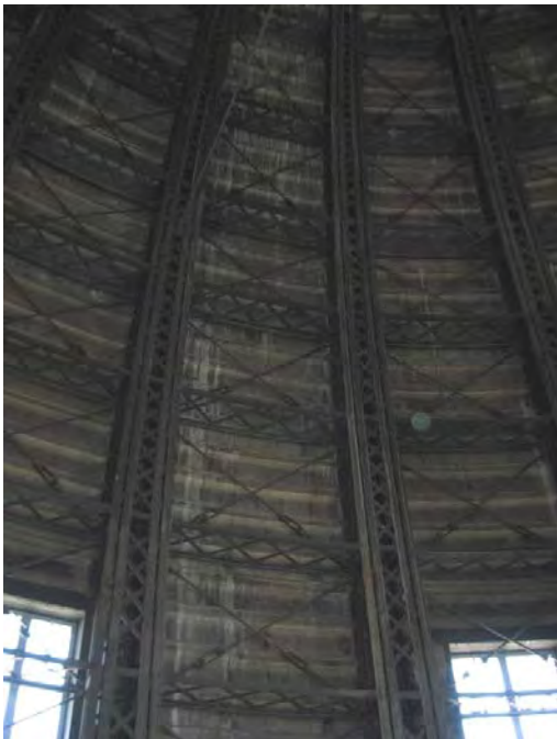
Figure C211. View of structural elements of outer dome, showing vertical trusses, circular trusses, cross bracing and window framing.
