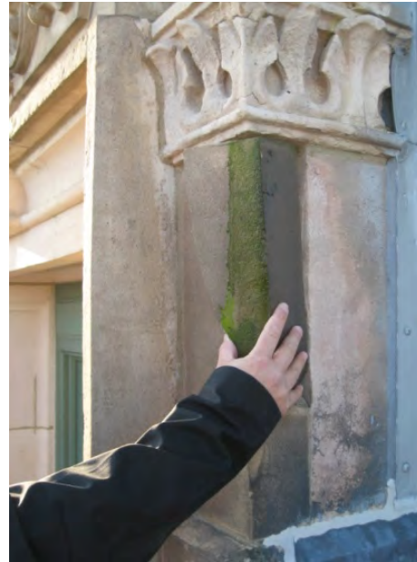
Figure C95. Spall of cracked terra cotta.
