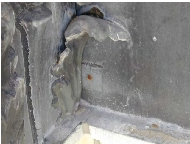
Figure C40. Corroded steel anchor. Lapped joint at rib.
