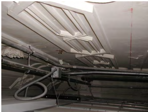
Figure B30. Decorative plaster above the suspended ceiling of the mezzanine.
