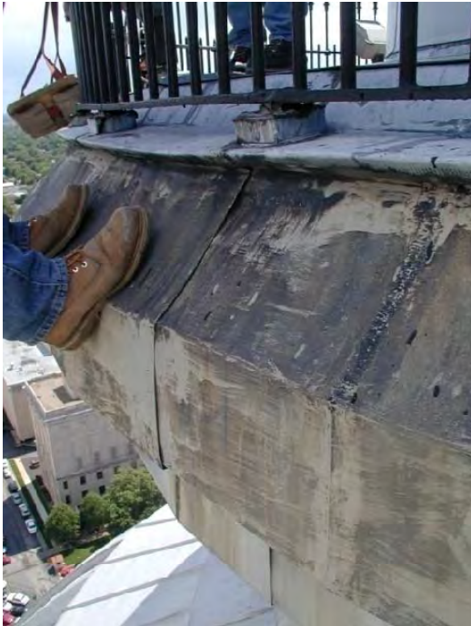
Figure C31. Black coating applied to zinc.
