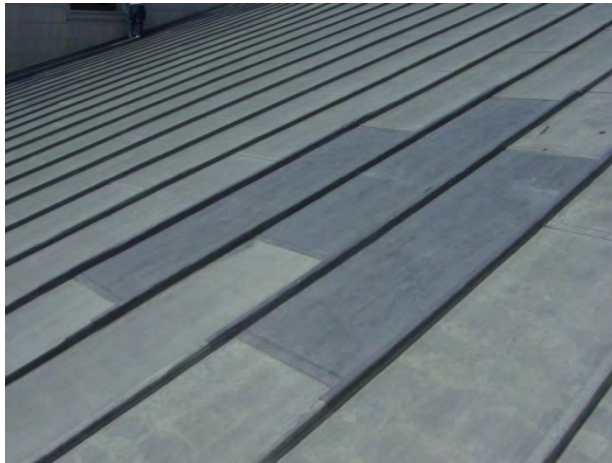
Figure C13. Replaced batten seam panels and batten caps.
