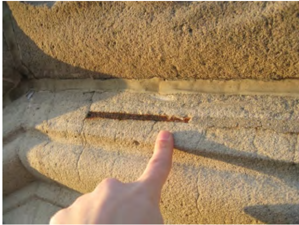
Figure C82. Corroding reinforcing steel at cornice.
