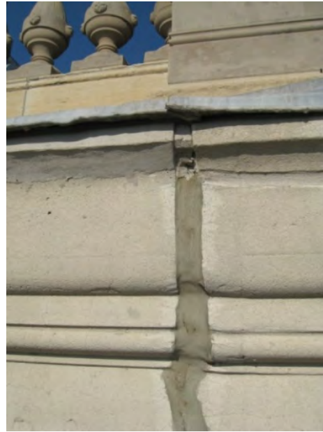
Figure C84. Patched concrete cornice.
