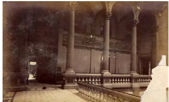
Figure C193. Historic photograph showing added cast iron column.
