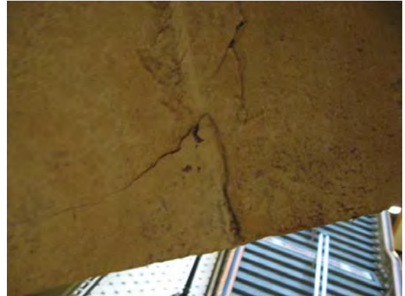
Figure C148. Cracking at the center of the masonry arches surrounding the rotunda on the second floor.
