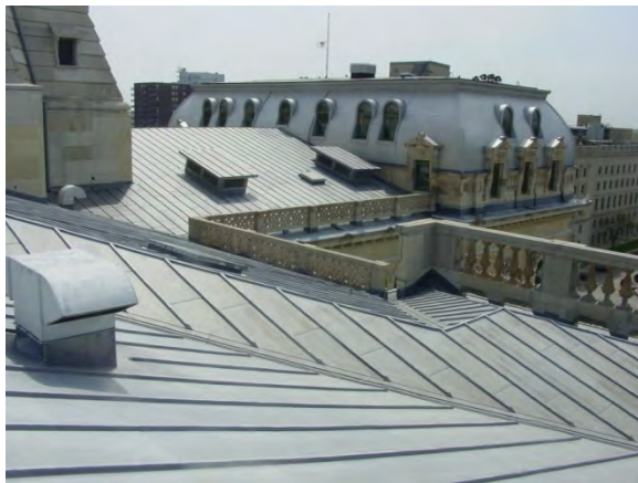
Figure B3. Overall view a series of intersection gables with a batten seam roofing system.
