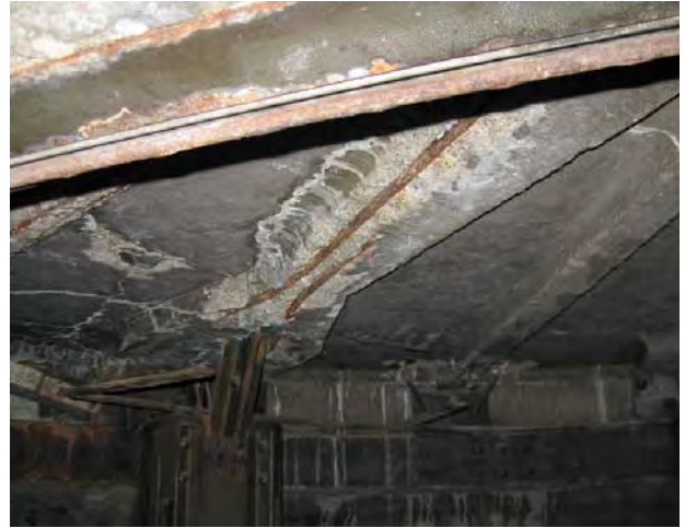
Figure C223. Underside of the attic floor, showing corroded reinforcing steel and spalled concrete.
