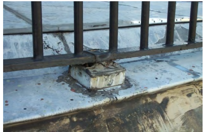
Figure D46. Cracked solder joint at embedment.
