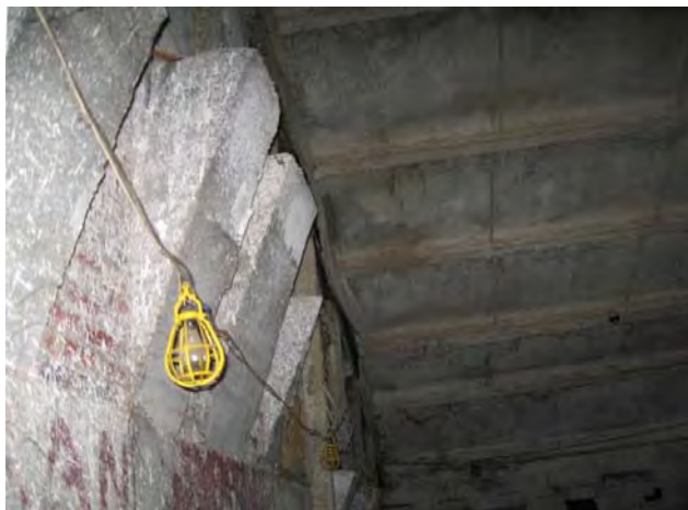
Figure C168. East portico roof framing also showing concrete counterweights of the cast in place concrete cornice.
