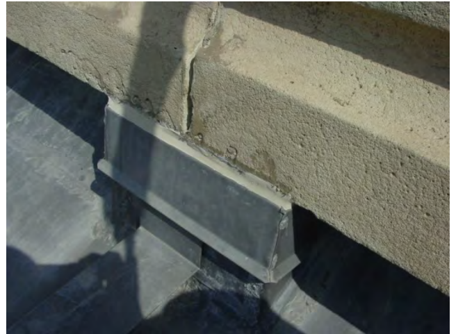
Figure C11. Open joints between sections of the balustrade.
