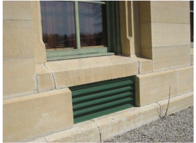
Figure C59. Cracked limestone lintel.
