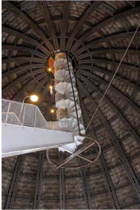
Figure C218. Interior view showing outer dome structure system and spiral staircase suspended from the compression ring and braced with metal tie rods.
