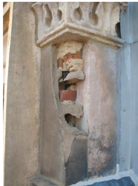
Figure C96. Removed terra cotta spall.
