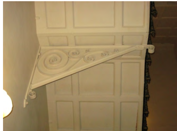
Figure B270. Added bracket at the north and south staircase.
