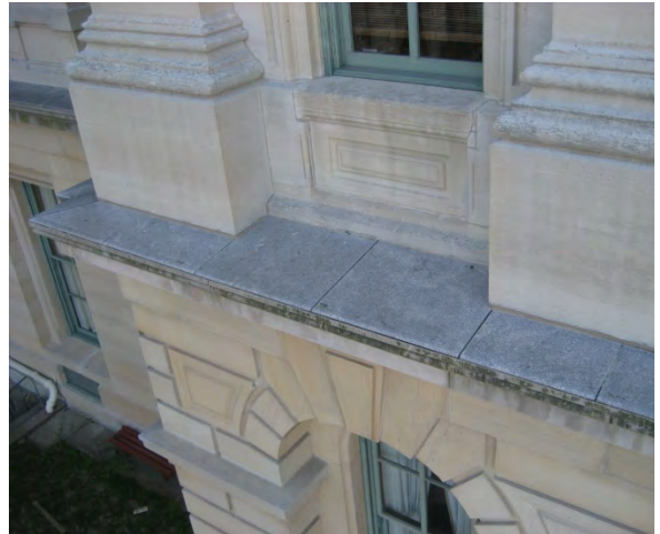
Figure C65. Granite wash above water table.
