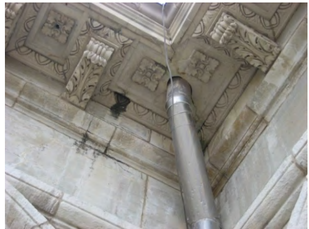
Figure C89. Overall view of black deposit.
