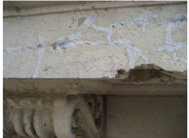
Figure C88. Slim coat of sealant.
