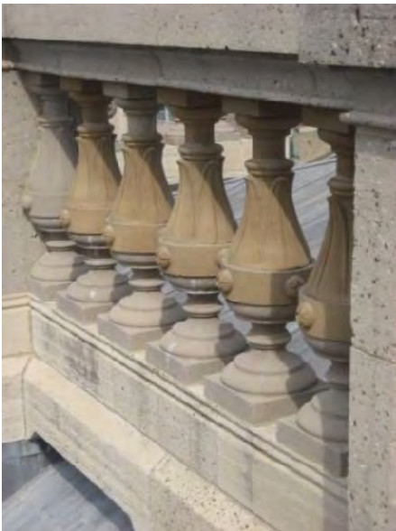
Figure C98. Replacement balustrades.
