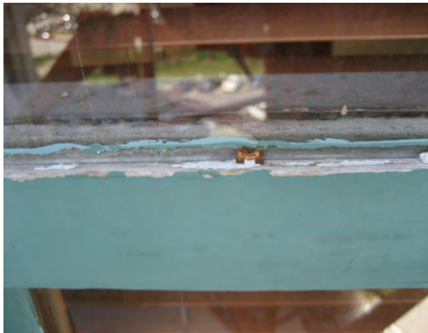
Figure C101. Exposed glazing points.
