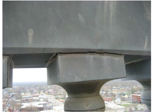
Figure C29. Open joint previously sealed with sealant.
