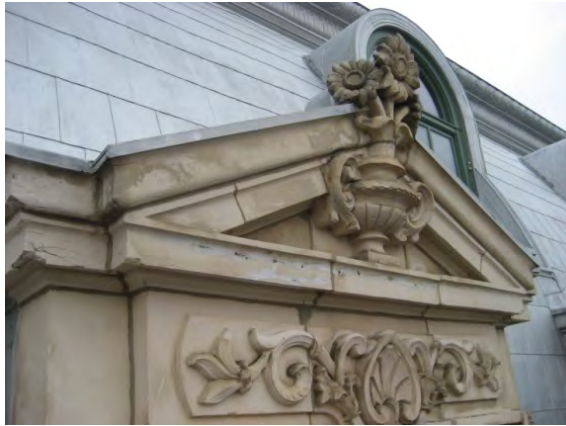
Figure C93. Epoxy injected on limestone.
