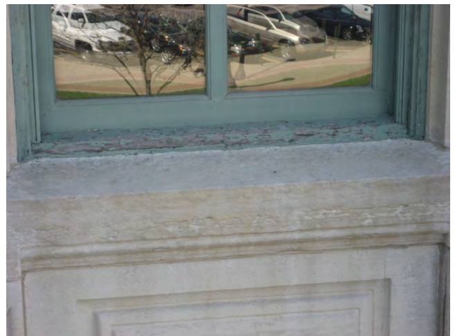
Figure C111. Paint failure and wood deterioration at sill.
