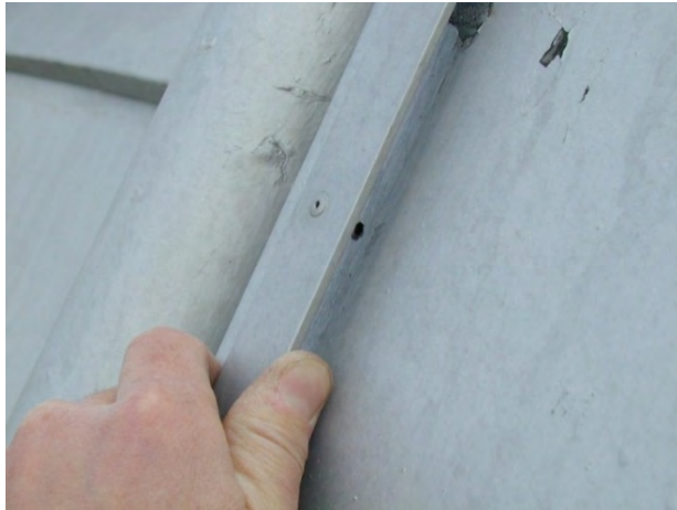
Figure C34. Open joint at rib.
