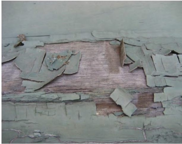
Figure C112. Detail of paint failure and wood deterioration at sill.
