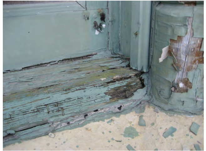
Figure C110. Deteriorated wood at sill and brick molding.
