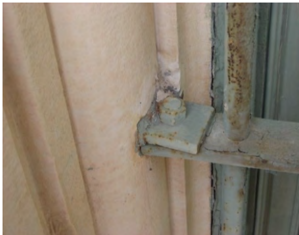
Figure C113. Security grill anchor.
