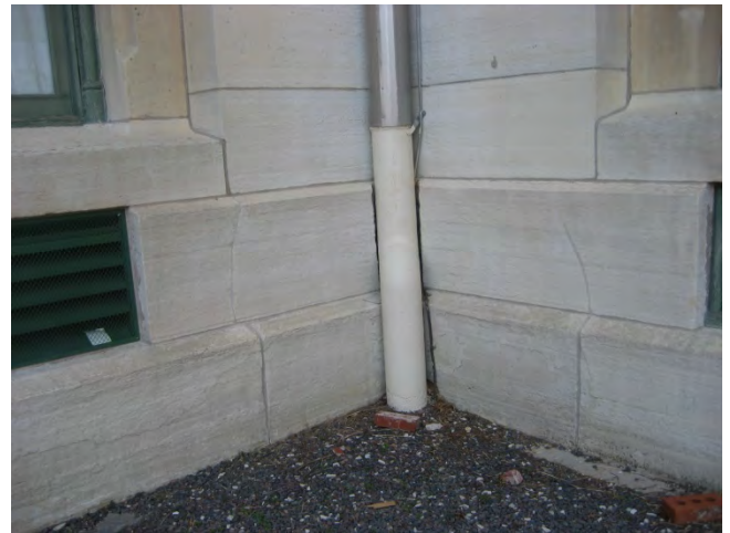
Figure D49. Cracked ashlar limestone unit.
