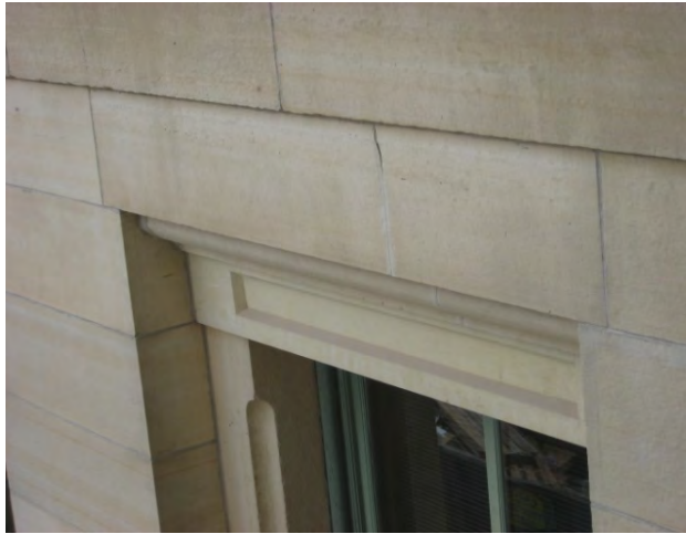
Figure C57. Cracked limestone at lintel.
