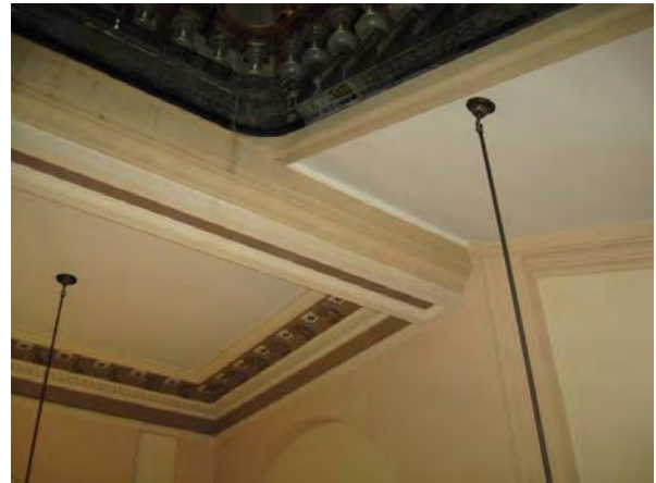
Figure C153. Close up view of large plaster clad wrought iron box beam, supporting the header of the grand staircase on the third floor.
