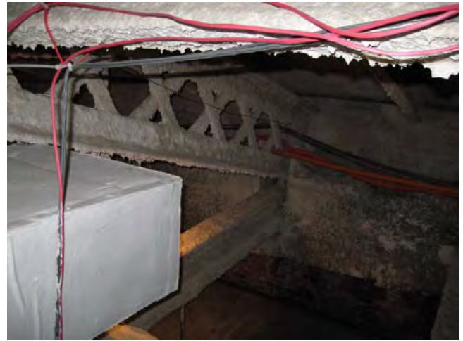
Figure C180. Close up view of wrought iron trusses above Senate Chambers in the north wing.
