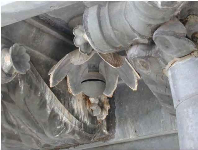
Figure D44. Cracked ornamental piece.
