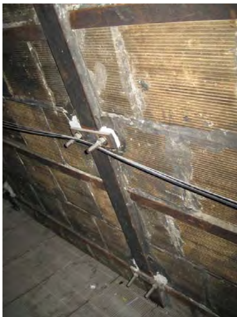
Figure C189. Retrofit anchorage at stone portion of the battered base of the dome, showing wrought iron framing and clay tile infill between framing.
