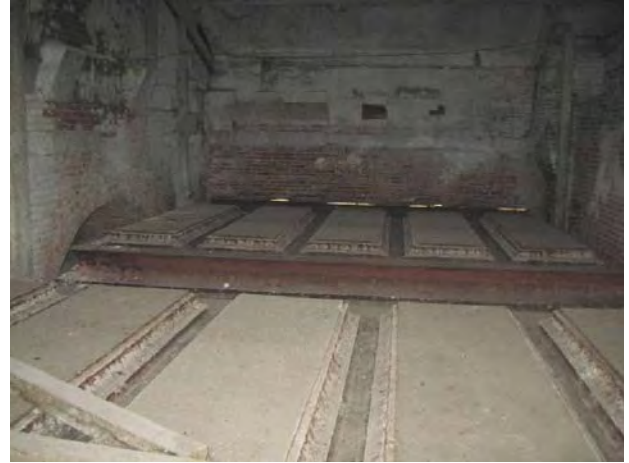
Figure C169. Topside of cast iron coffer ceiling of east portico, supported by wrought iron framing.
