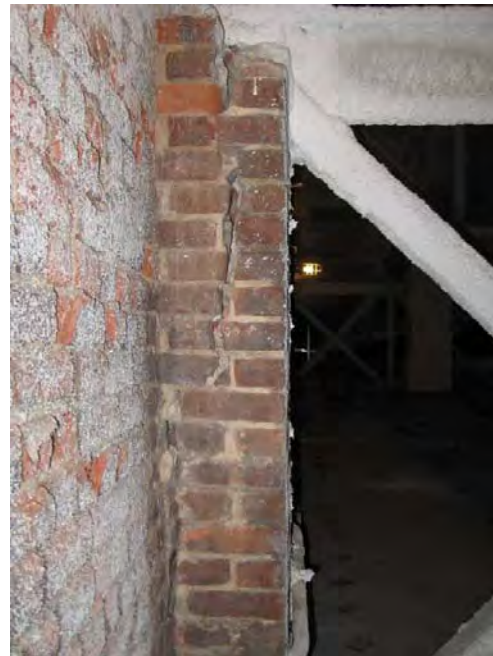
Figure C178. Significant cracking of integral masonry pier supporting main low truss. Also, note the spalling, flaking and efflorescence of the backup masonry wall.
