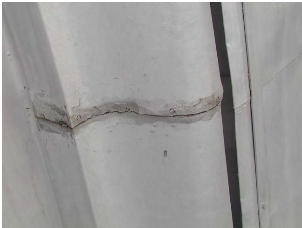
Figure C36. Open joint previously sealed at rib.
