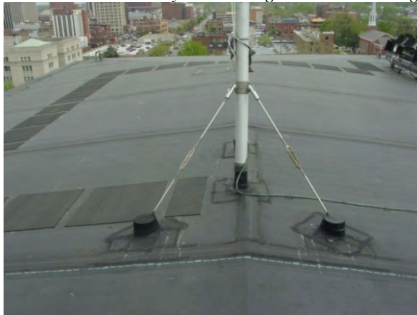
Figure C25. Penetrations flashed with pitch pans will require routine maintenance.
