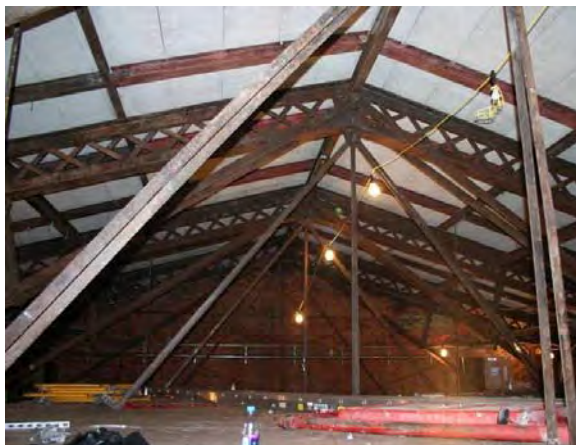
Figure C182. View of wrought iron trusses supporting roofing above House Chambers (south wing) during renovation.
