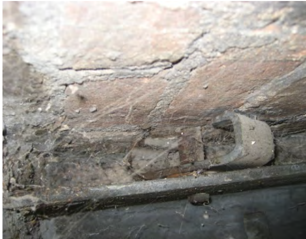
Figure C119. Window anchor with surface corrosion.
