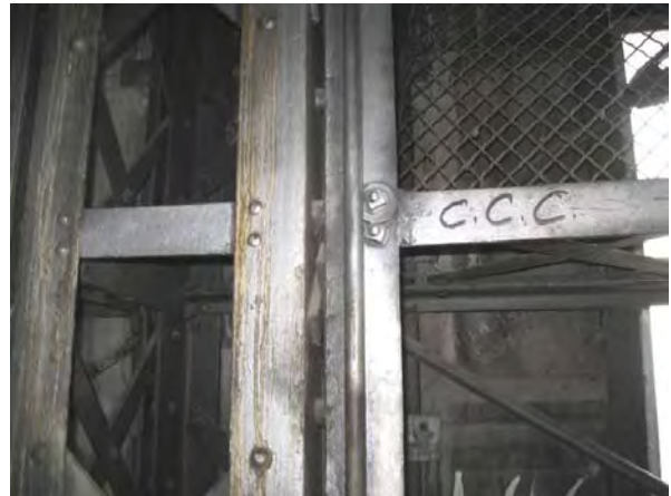
Figure C213. Close up view of connection between vertical and circular trusses.
