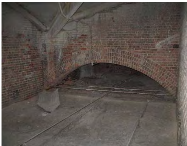
Figure C164. Load bearing masonry framing the tempietto structures.
