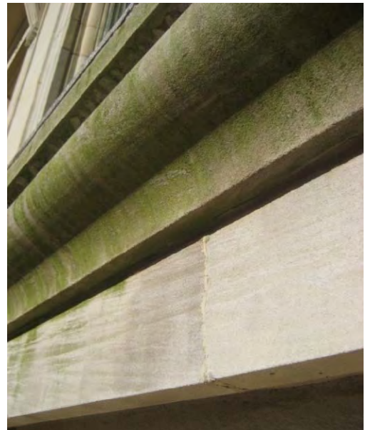
Figure C69. Biological growth on limestone.
