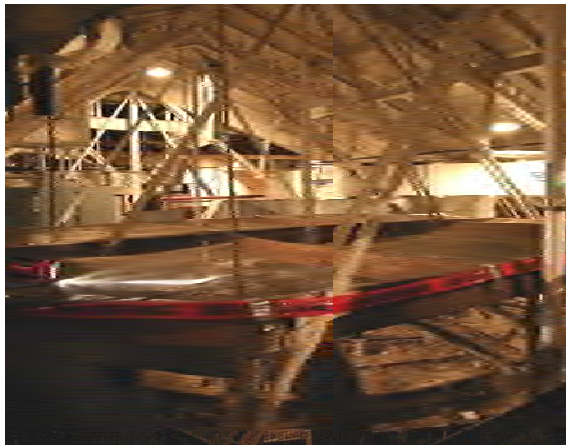
Figure C181. View of wrought iron trusses supporting roofing above House Chambers (south wing) prior to renovation.
