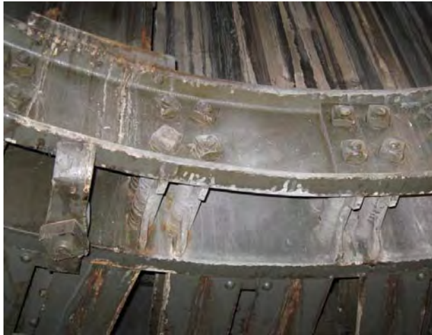
Figure C215. Close up view of the compression ring.
