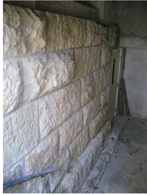
Figure C128. Rusticated Joliet limestone ashlar units forming the foundation walls, at north wing.
