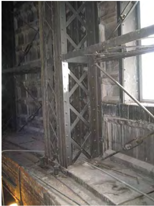
Figure C214. Overall view of connection between vertical and circular trusses.
