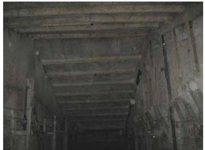
Figure C166. Roof framing of east portico, showing 8WI and sag rods between purlins.
