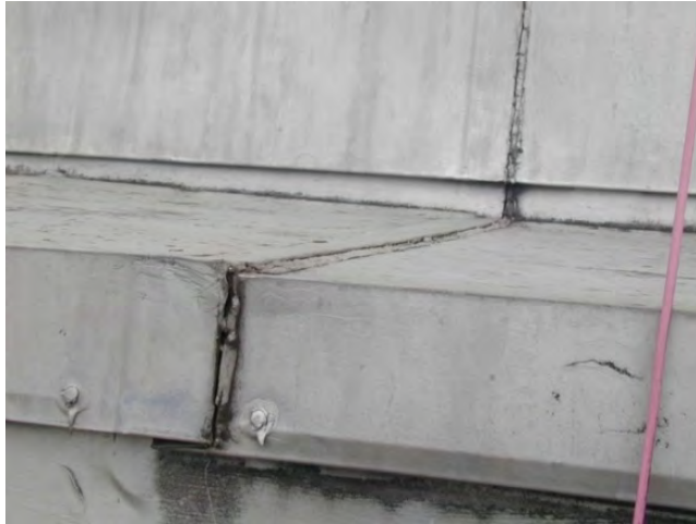
Figure C39. Deteriorated sealant joint at deteriorated solder joint.
