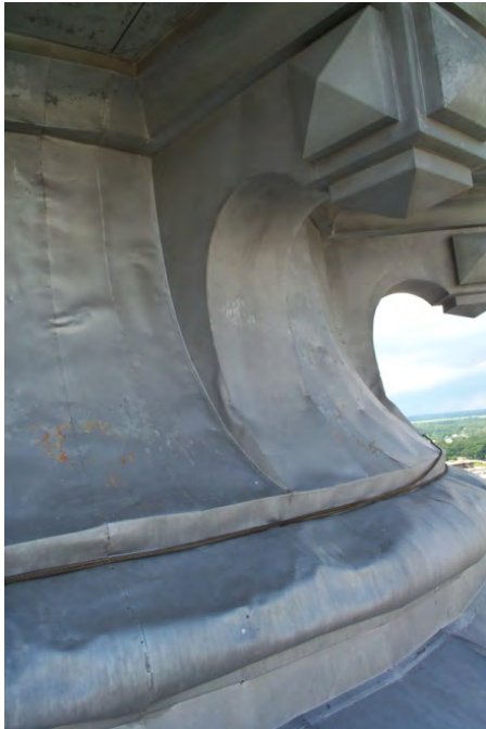
Figure D48. Typical dented portion of cladding.
