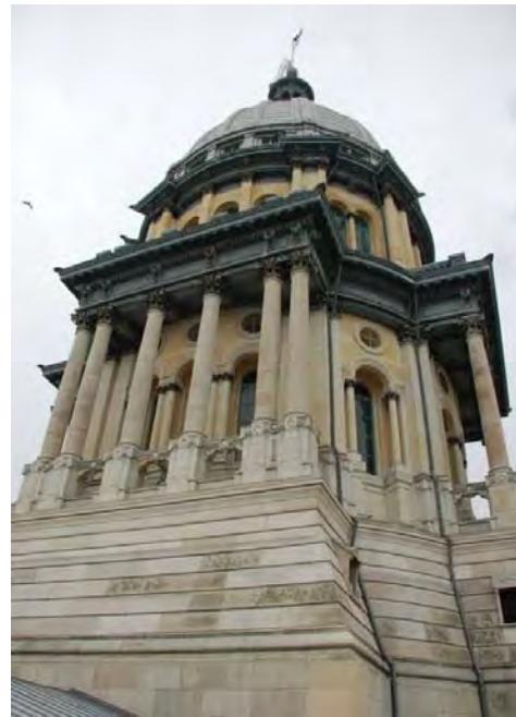
Figure C196. The exterior stone portion of the dome consists of 4 large porches at each of the principal elevations, each of these porches have six stone columns.
