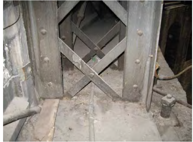
Figure C208. Close up view showing base of vertical truss framing outer dome.
