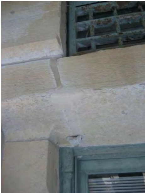
Figure C58. Detail of cracked limestone lintel.
