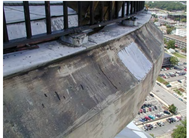
Figure C30. Sheet metal patches.
