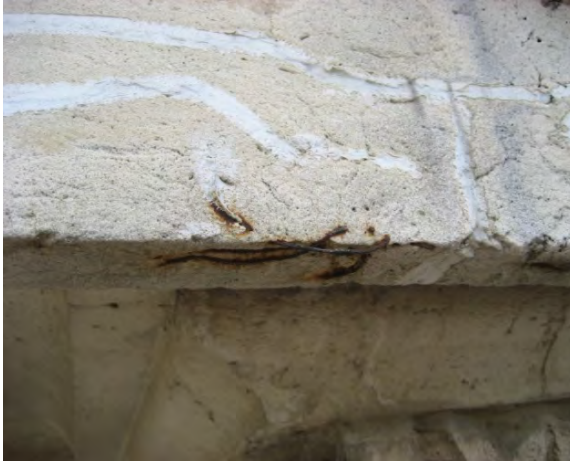
Figure C79. Fragment of wire in cast concrete.
