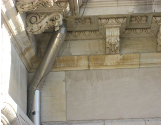
Figure C70. Replacement limestone.
