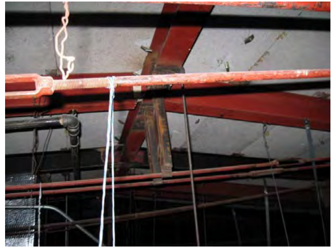
Figure C187. Close up view of deviator bracket between wrought iron framing and steel retrofits of south wing mansard roof framing.
