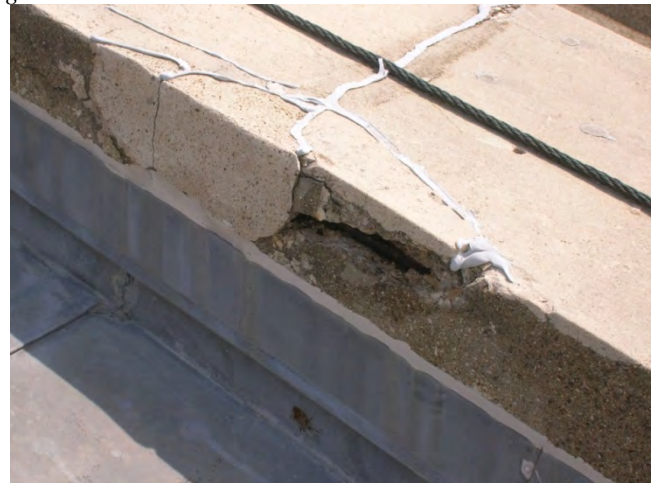
Figure C17. Deteriorated cast-in-place concrete at the east and west gables.
