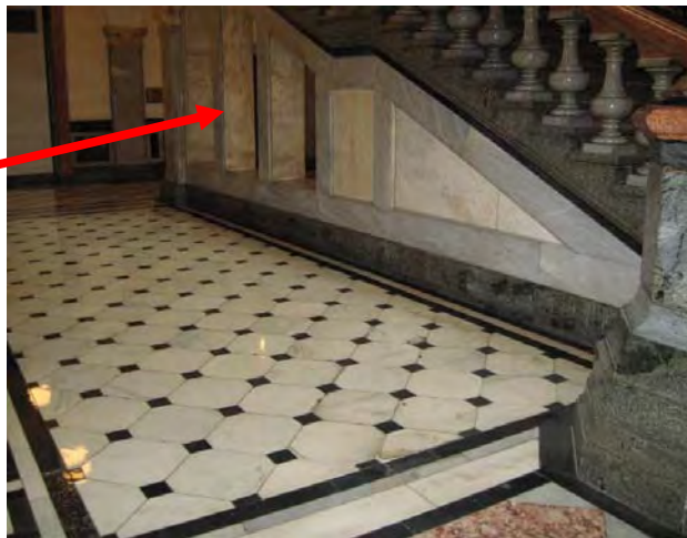
Figure C144. View of columns clad in marble supporting the grand staircase between second floor and second floor mezzanine.
