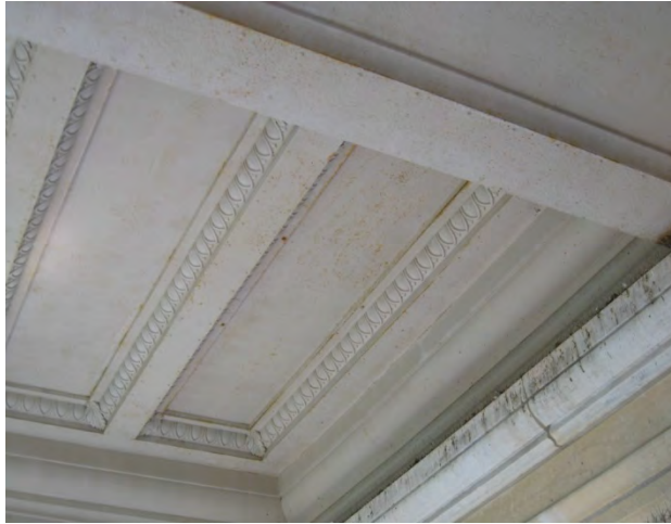
Figure C122. Minor peeling paint and corrosion of cast iron soffit.
