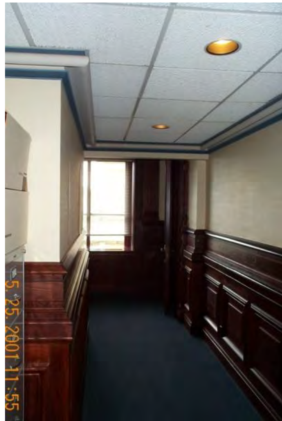
Figure B138. Original and replicated wainscoting in Room 205.
