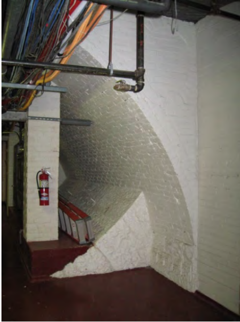
Figure C127. Large masonry groin vault beneath rotunda space, with limestone buttress.
