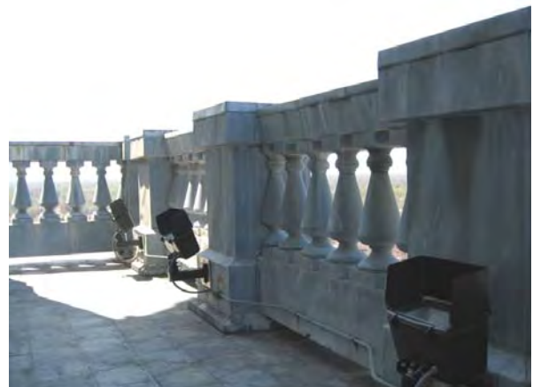
Figure C201. Exterior porches clad in sheet metal, framed into masonry drum of the outer dome structure.
