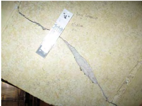
Figure C151. Cracking of the plaster clad masonry arch at the second floor south wing where tell tale monitors have been previously installed.
