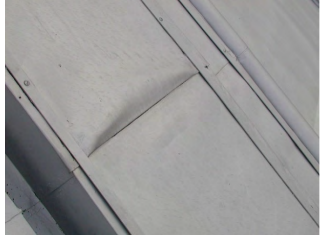
Figure C33. Buckled metal cladding at dome.
