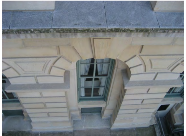
Figure C68. Biological growth on limestone.
