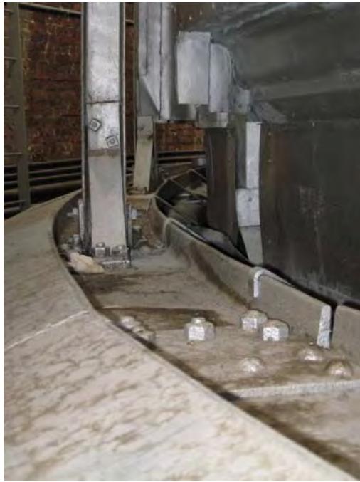
Figure C204. Interior dome structure connection to channel iron atop circular masonry wall supported by interior columns.
