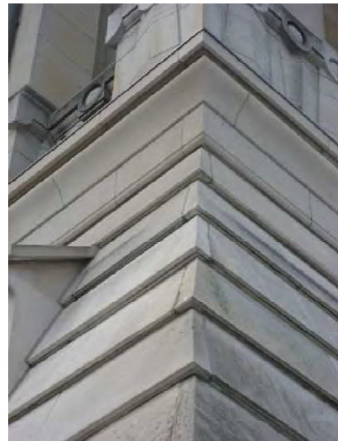
Figure C66. Battered walls at the base of the dome.
