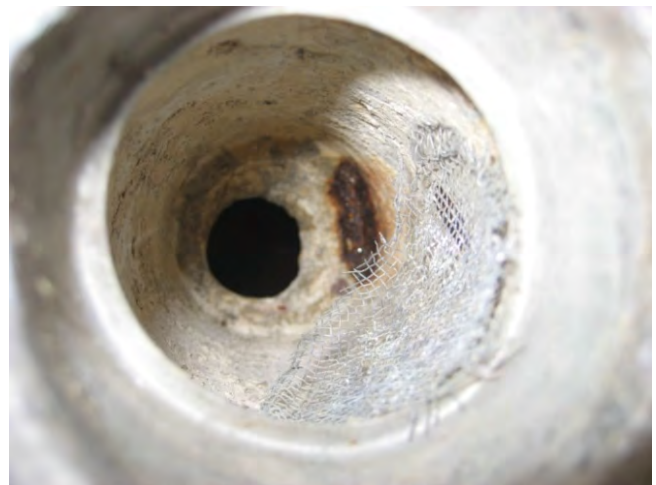
Figure C81. Detail of added vent.
