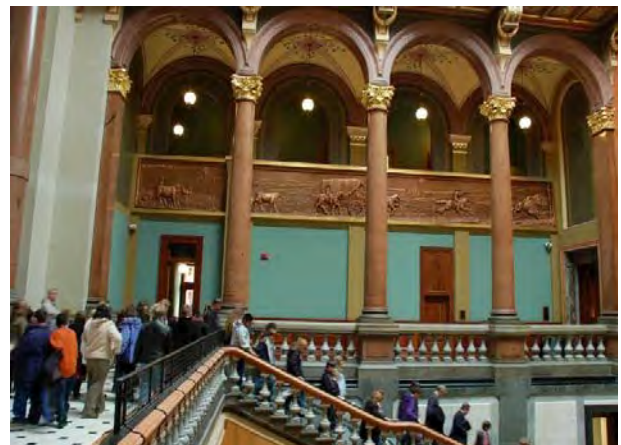
Figure C154. Plaster frieze concealing the trusses supporting the flooring of the fourth floor galleries.
