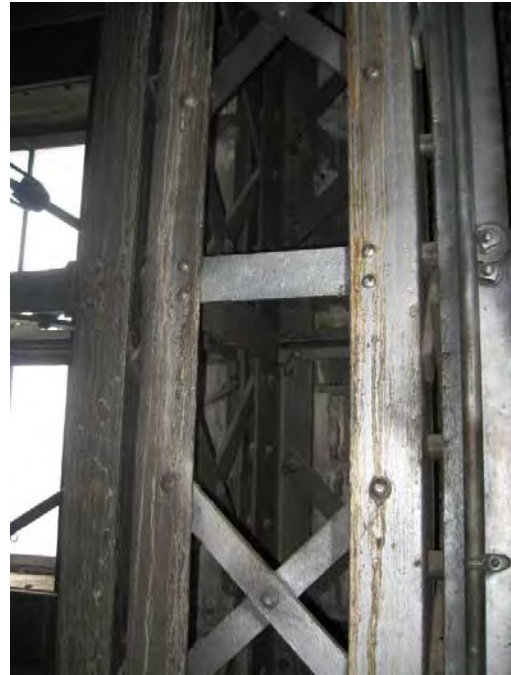
Figure C209. Close up view showing vertical truss elements framing outer dome.
