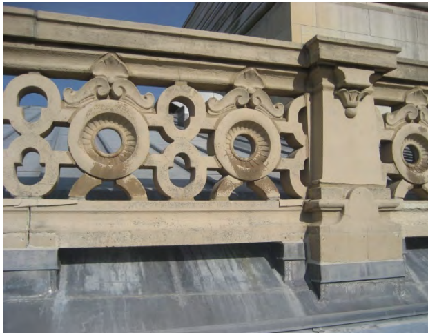
Figure C91. Deteriorated coating on cast stone.
