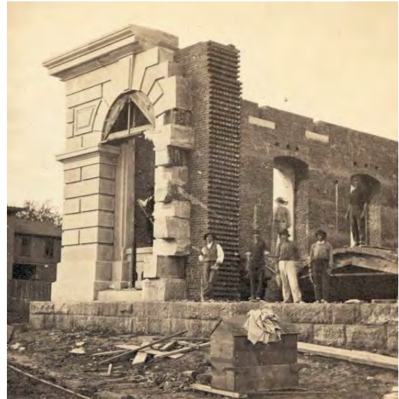
Figure C133. First floor construction photo, showing face limestone and backup brick masonry
