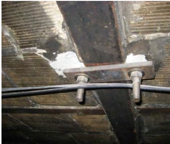
Figure C67. Detail of new anchor from backside.
