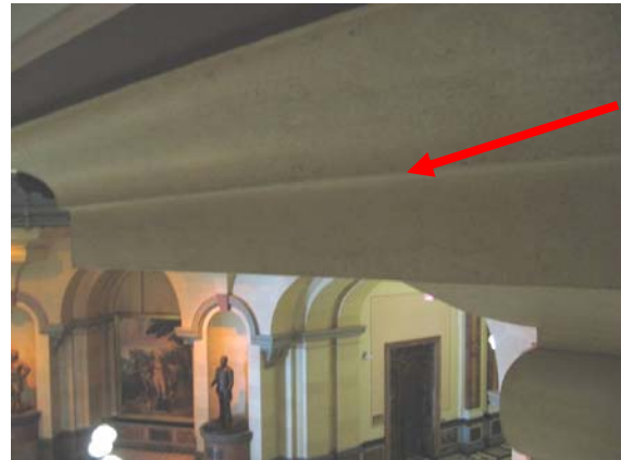
Figure C149. Hairline cracks running along the plaster clad wrought iron beams framing the drop pendant.
