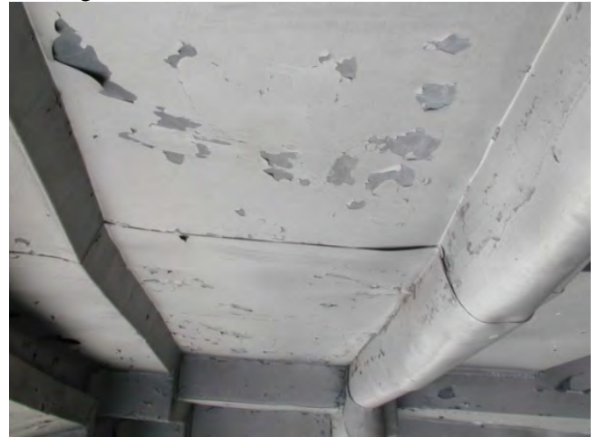
Figure C41. Peeling paint at dome cladding.
