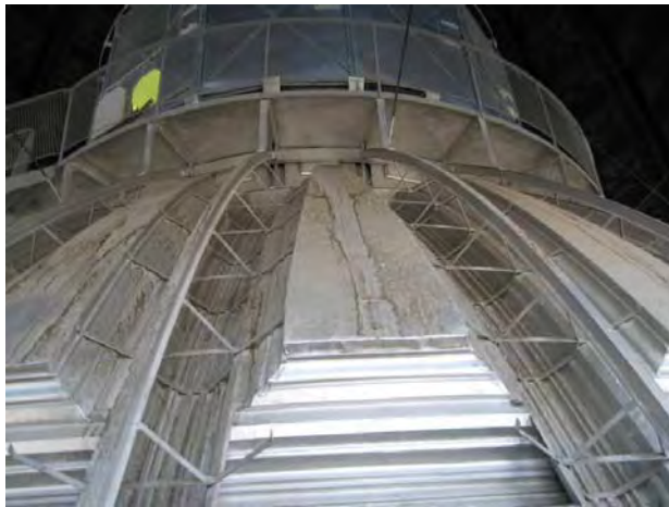
Figure C205. Interior dome space frame like structure, with main ribs consisting of 4" wrought iron I-beams.
