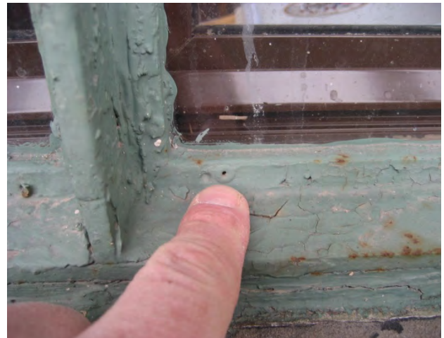
Figure C121. Detail of peeling paint and minor surface corrosion on cast iron windows.
