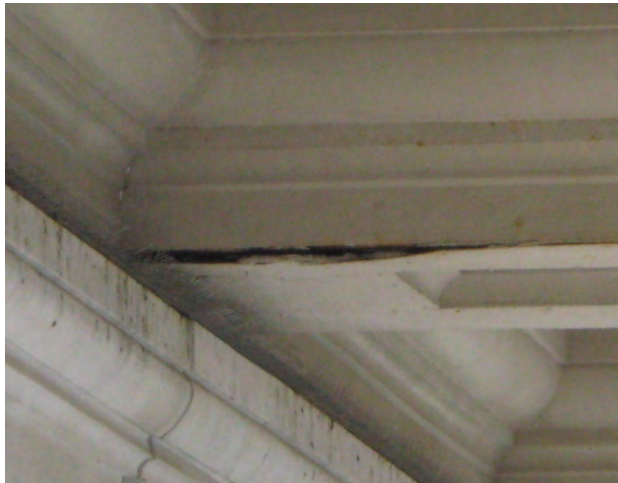
Figure C123. Corrosion scale at cast iron soffit panels.
