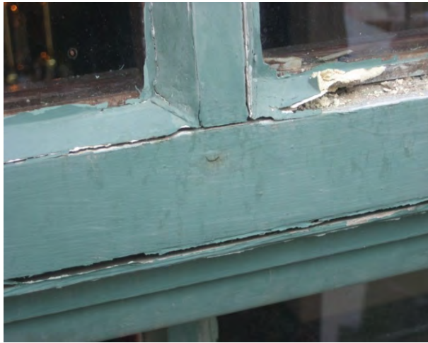
Figure C100. Cracked glazing compound.
