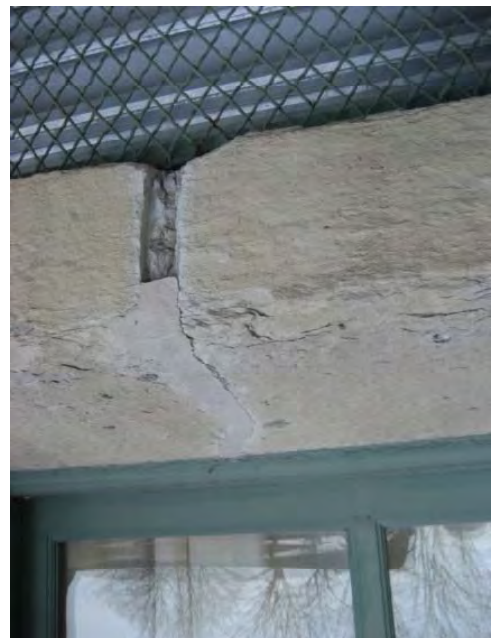
Figure C56. Cracked limestone at lintel.
