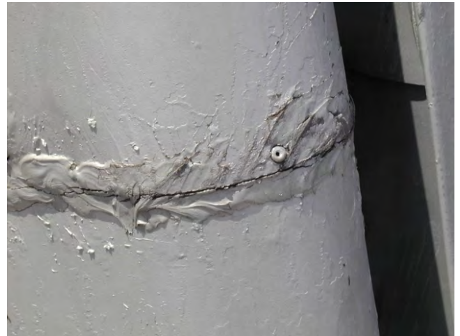
Figure C37. Joint repaired with sealant and pop rivet.
