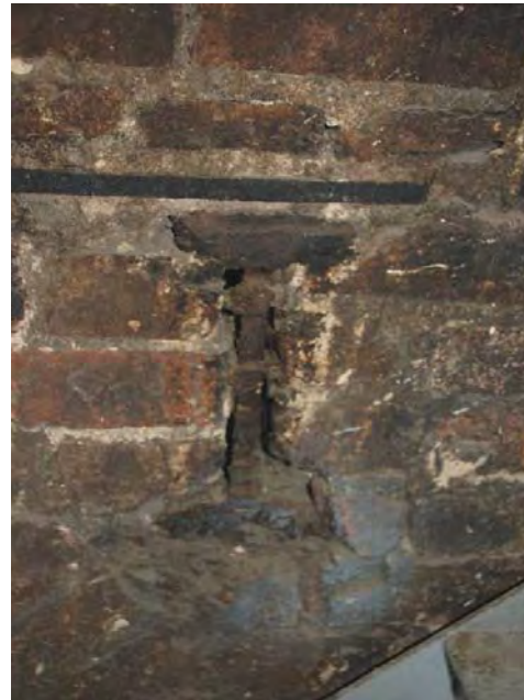
Figure C200. Slightly corroded remnants of cast and wrought iron framing elements of the porches and balustrades clad in sheet zinc.
