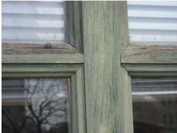
Figure C104. Deteriorated painted wood stop.
