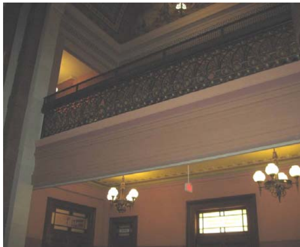
Figure C155. Large plaster beam concealing the wrought iron truss, supporting the fourth floor of the east wing.
