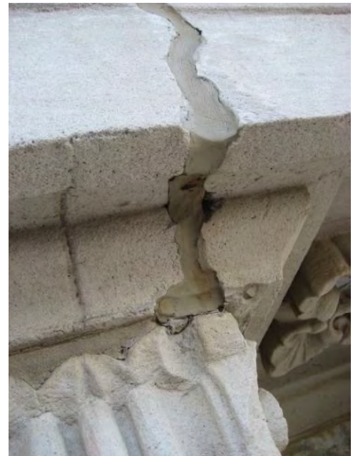
Figure C78. Detail of sealant installed in cracked concrete.
