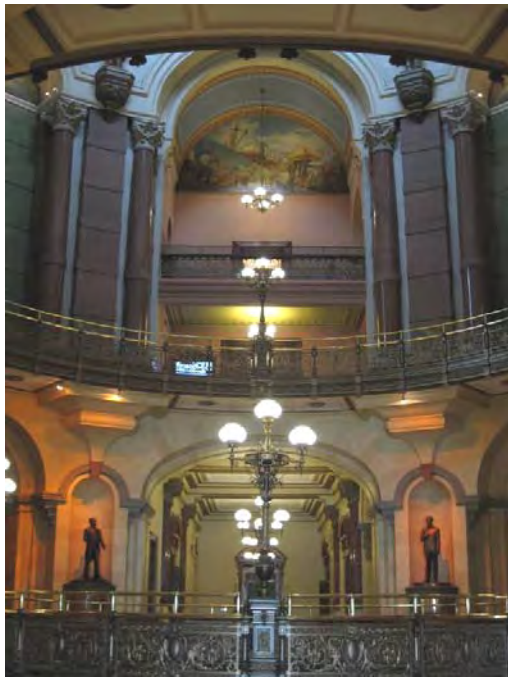
Figure C202. Large archways on fourth floor transferring loading from the dome to the four massive masonry piers (elevator coves).
