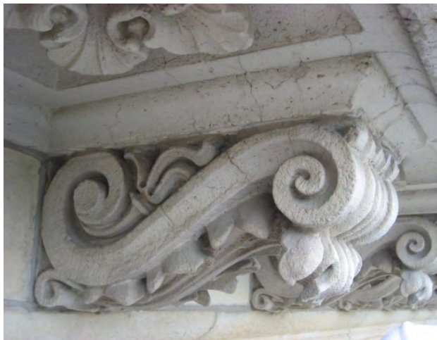
Figure C76. Regularly spaced shrinkage cracks in cast-in-concrete ornament.
