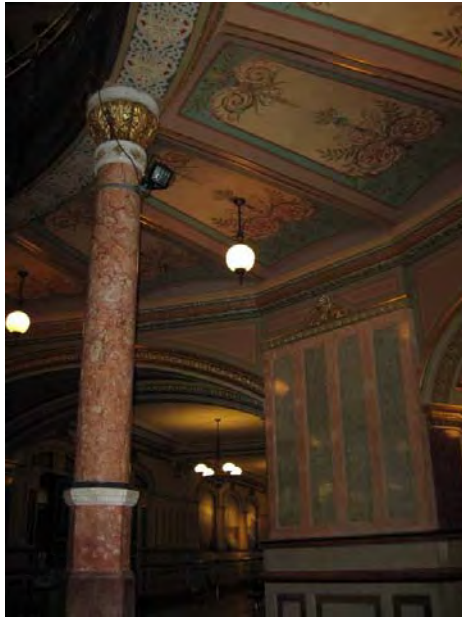
Figure C141. One of the four cast iron columns supporting the second floor of the rotunda.
