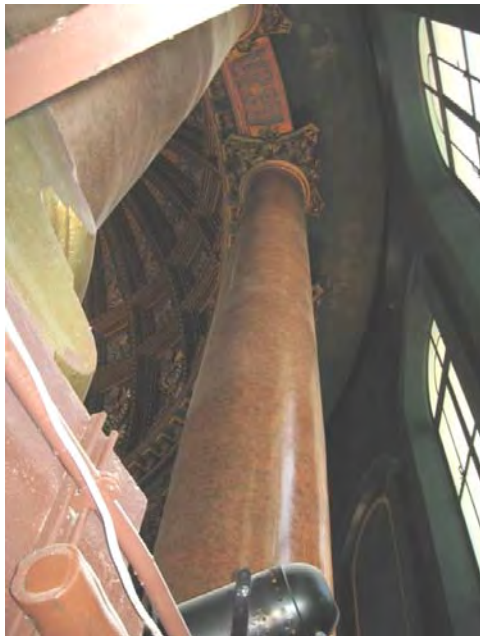
Figure C199. Interior brick columns at colonnade level of dome, supporting inner dome structure.
