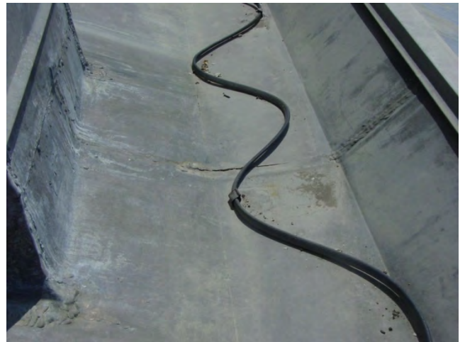
Figure C5. Cracked solder joints in the flat lock roofing in the built-in gutters.
