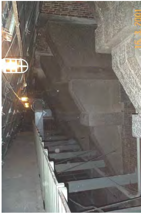
Figure C198. Large limestone corbels constructed integrally with the brick masonry of the dome drum, support the exterior limestone porches and columns and the colonnade level.
