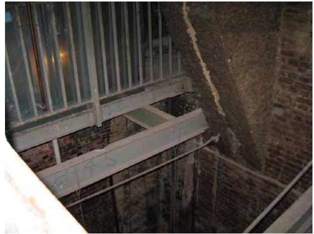
Figure C206. Steel framing of cat walk structure, showing limestone corbel in background.
