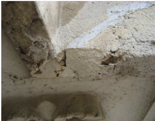
Figure C87. Skim coat of sealant applied to cracks.
