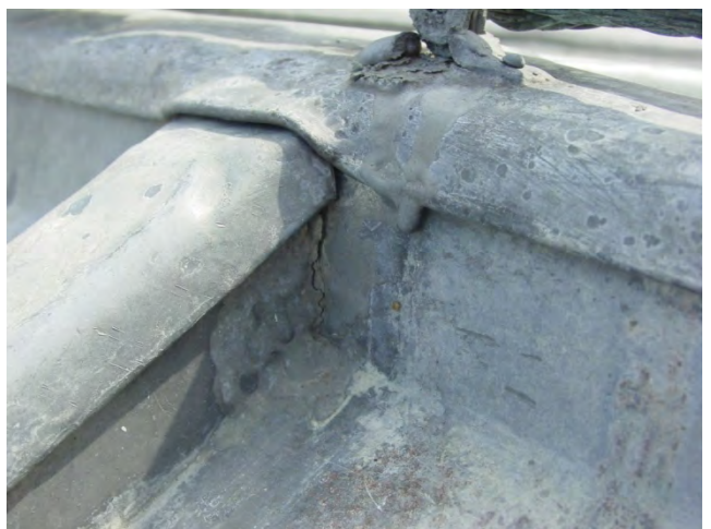
Figure C6. Cracked solder joints at the intersection of a typical batten and the ridge batten.
