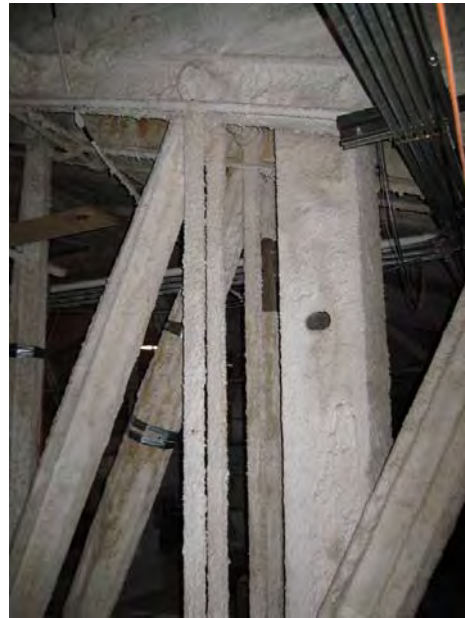
Figure C192. Square cast iron column, between double truss elements, added to support the transfer girder and loading of the battered base of the dome.
