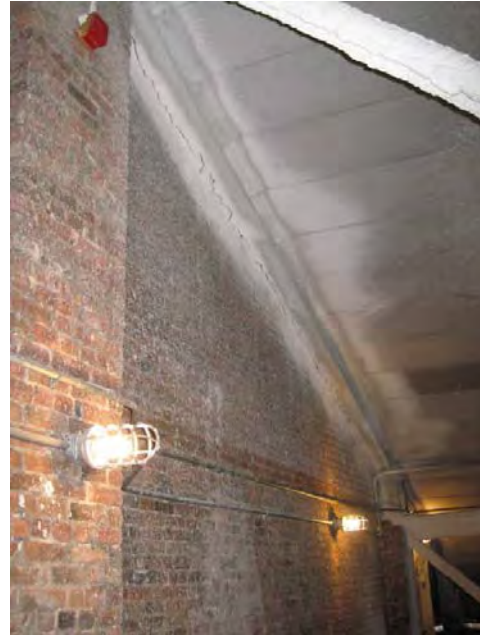
Figure C177. Cracking near roofline between backup masonry wall and roof framing to the north of main high truss.
