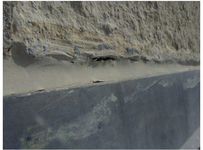
Figure C10. Failed sealant at the masonry bed joint above the counterflashing.
