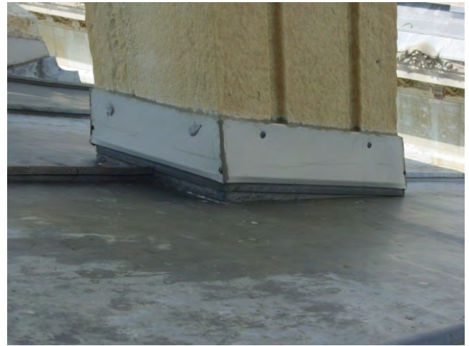
Figure C21. Previous repairs include the installation of membrane clad counterflashings at the base of the columns.
