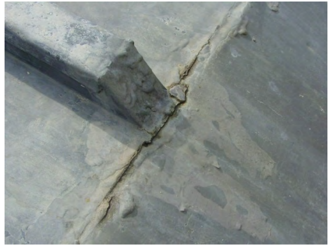
Figure C4. Cracked solder joints in the flat lock roofing around the balustrades.
