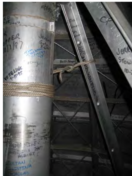
Figure C220. Structural framing of the roofing above the dome lantern, showing framing for the flagpole in the foreground.
