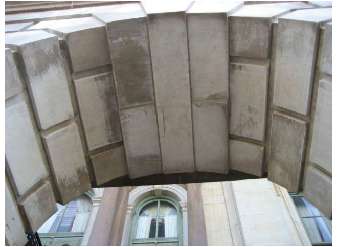
Figure C62. Detail of remnants of previous coating on arch.
