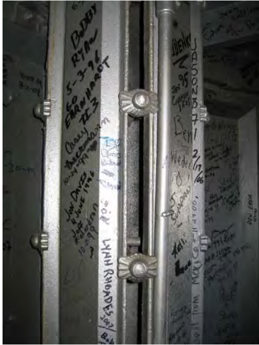
Figure C221. Close up view of built-up wrought iron column supporting the lantern.
