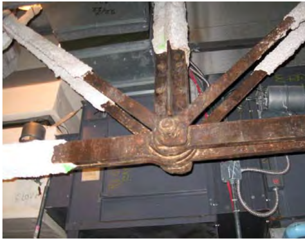
Figure C173. Close up view of connection of main high truss elements.
