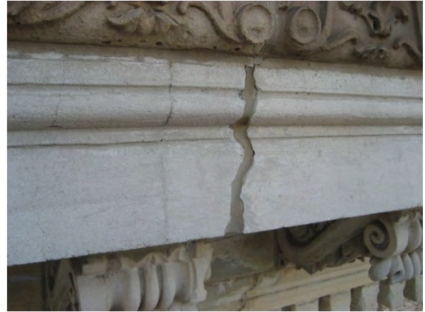
Figure C77. Crack in concrete repaired with sealant.
