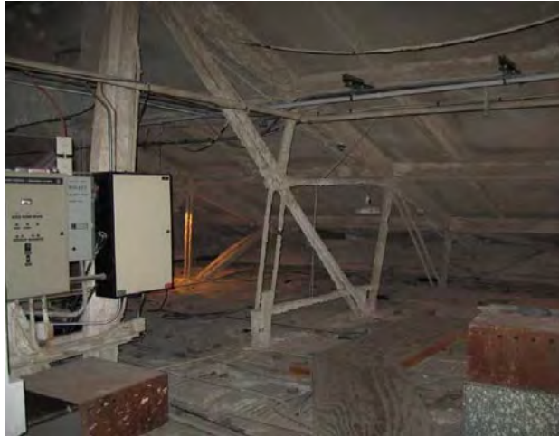
Figure C163. Roof framing truss at location of original skylight.
