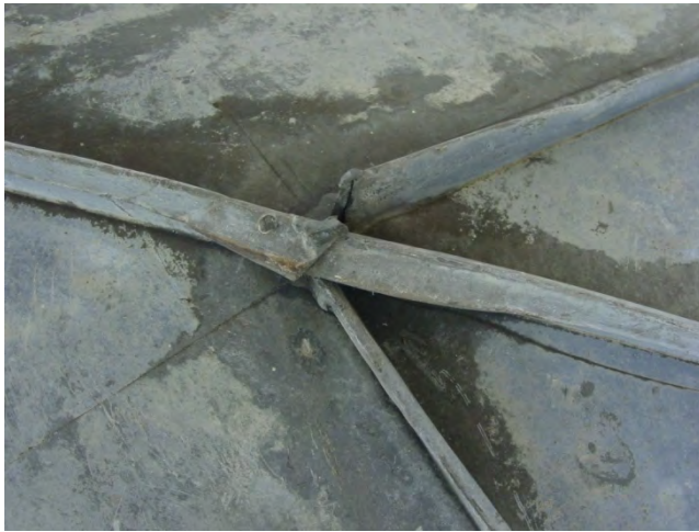
Figure C19. Open standing seams at the intersection of the typical seam and the ridge seam.
