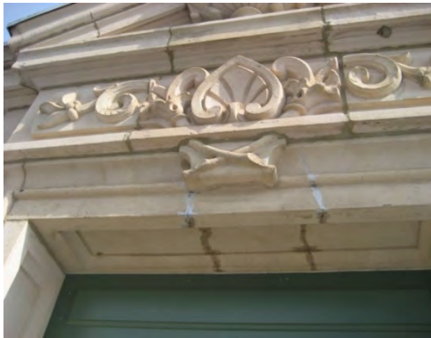
Figure C94. Epoxy injected repairs.
