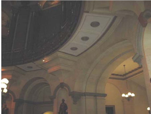
Figure C147. The ceiling of the second floor rotunda displays drop pendants and coffers.
