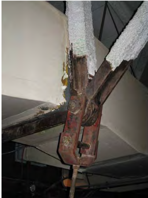
Figure C174. Close up view of connection of main high truss elements.
