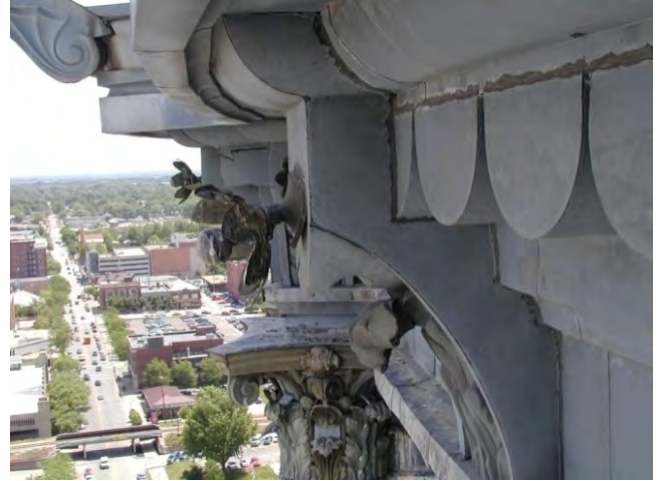
Figure D45. Corroded ornamental metal.
