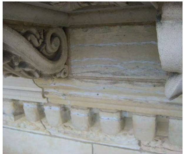
Figure C60. Epoxy injection repair of bedding plane.
