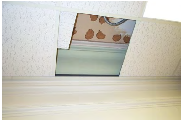
Figure B25. Simple plaster cornice molding above the suspending ceiling in Room 109B.
