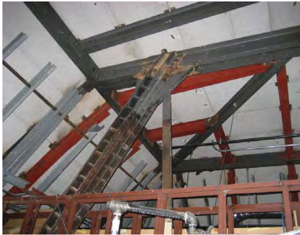
Figure C185. Close up view of wrought iron truss and steel retrofits of south wing mansard roof framing.
