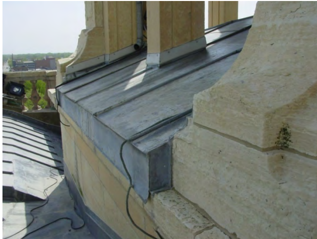
Figure C20. Deteriorated plastic washers and the loose apron flashing at the south side of the north tower.
