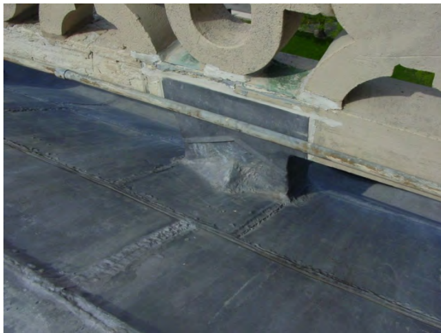
Figure C9. Failed sealant between the counterflashing and balustrade.
