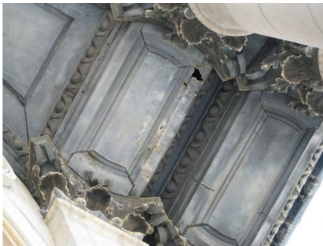
Figure C32. Area of corrosion on metal soffit panel.
