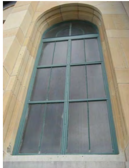
Figure C118. Replacement steel window.
