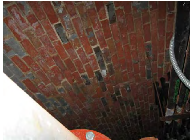
Figure C138. Spalling and flaking of brick arch on underside of vault beneath north portico.
