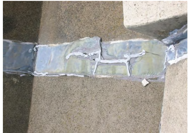
Figure C16. Failed previous repair at the east and west gables.
