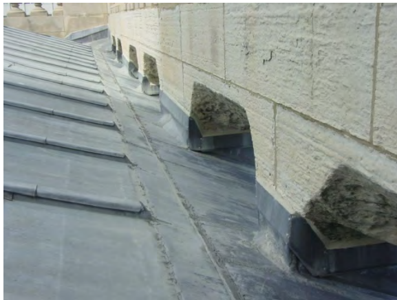
Figure B8. Batten seam roofing to flat panel roofing transition at the perimeter balustrade.
