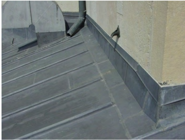
Figure C8. Batten seams that stop short of the dome and the wall flashings that do not include expansion provisions.
