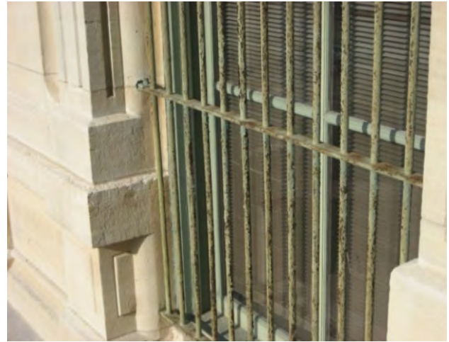
Figure C114. Peeling paint and corrosion of security grills.
