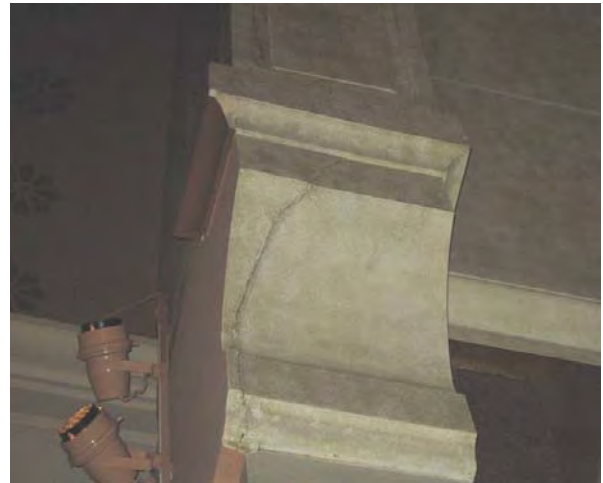
Figure C156. Cracking of the plaster of the spring point of the brick arch above the fourth floor.
