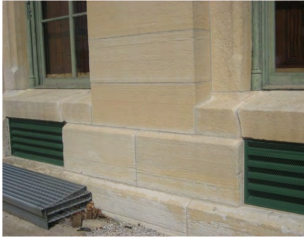
Figure C116. Replacement aluminum louvers.
