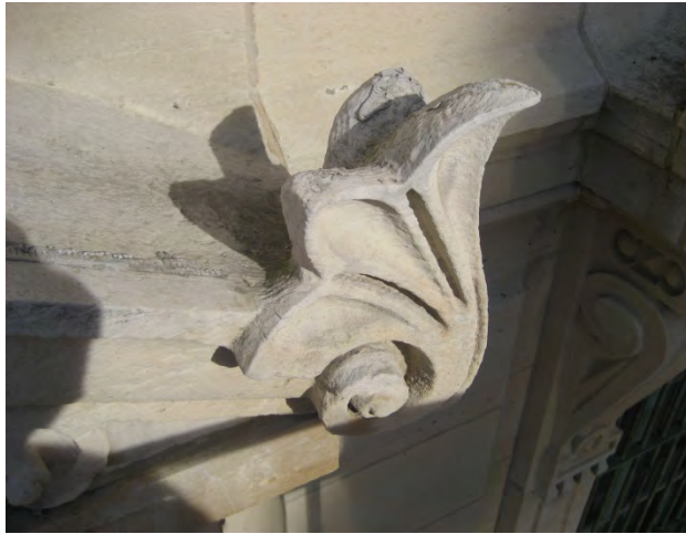
Figure C75. Eroded limestone unit.
