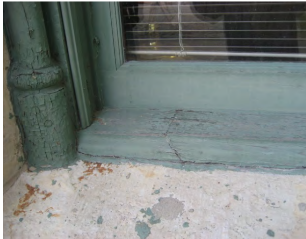
Figure C109. Dutchman installed on sill.
