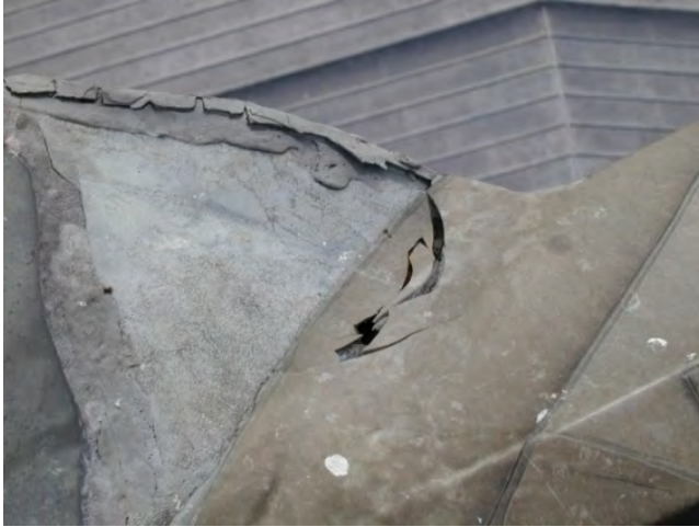
Figure D43. Open hole in projecting cap.
