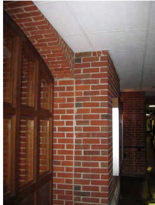
Figure C136. Brick infill between brick piers and vaults in basement.
