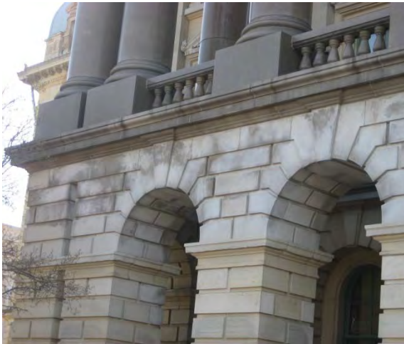
Figure C61. Remnants of previous coating of limestone arch.
