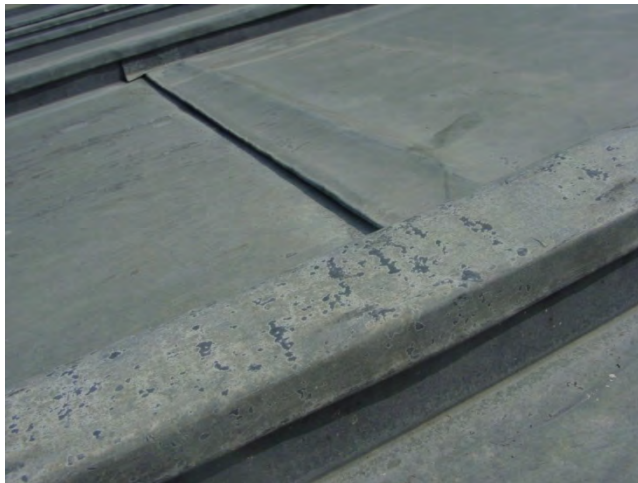
Figure C2. Minor pitting in the surface of the lead coated copper.
