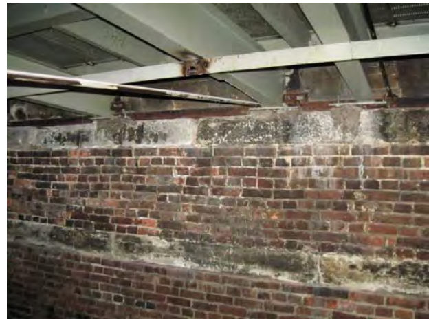
Figure C207. Underside of steel framing of the cat walk structure, bearing on back up masonry of outer dome.
