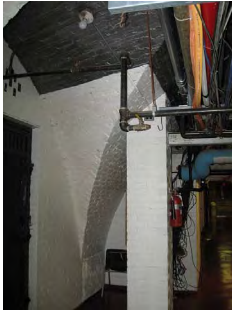
Figure C134. Large masonry groin vault beneath rotunda, with added brick pier.
