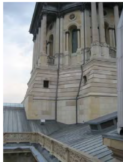
Figure C63. Replacement Indiana limestone units at drum of dome.
