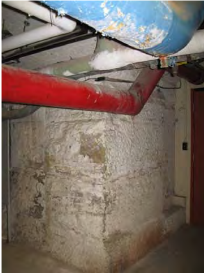
Figure C130. Interior Joliet limestone foundation wall beneath north portico.
