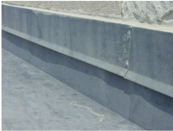
Figure B7. Batten seam roofing terminated behind a counterflashing mounted in a masonry bed joint.
