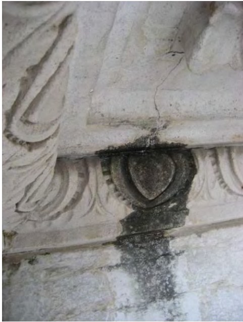
Figure C90. Detail of black deposit at cornice.
