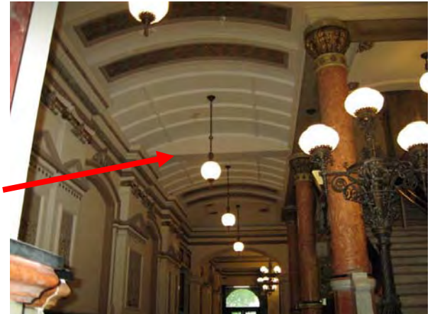
Figure C142. View showing wrought iron box beam clad in plaster supporting the foot of the grand staircase on the second floor.
