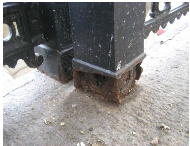
Figure C124. Cracked rail post.
