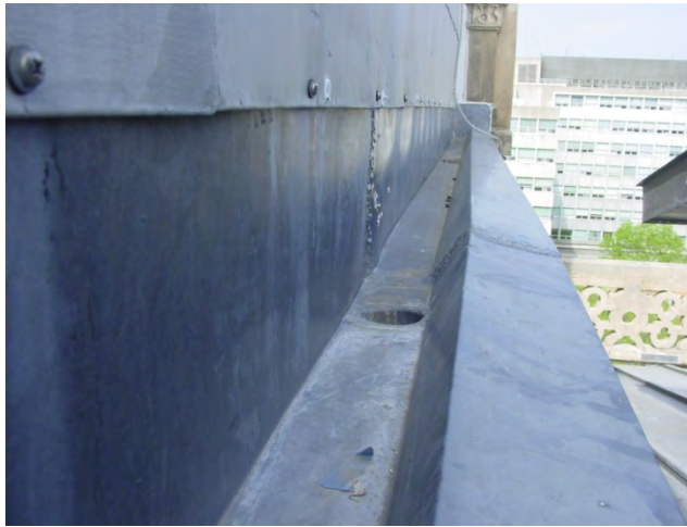
Figure C23. Screws with neoprene washers installed through the first course of shingles to resist wind uplift.
