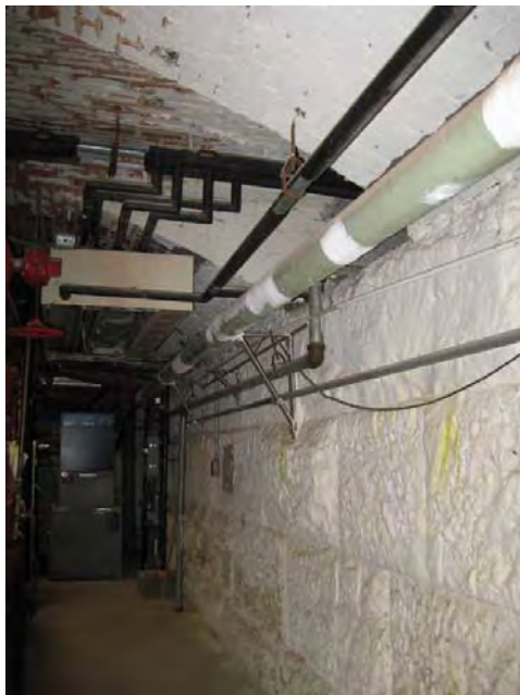
Figure C137. Interior face of Joliet limestone foundation walls supporting east portico.
