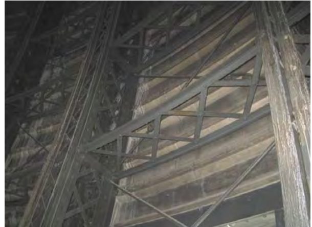
Figure C212. View of structural elements of outer dome, showing vertical trusses, circular trusses, cross bracing and precast concrete panel sheathing.
