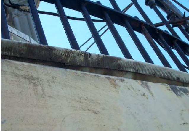
Figure D47. Front lip of cladding riveted to underside.
