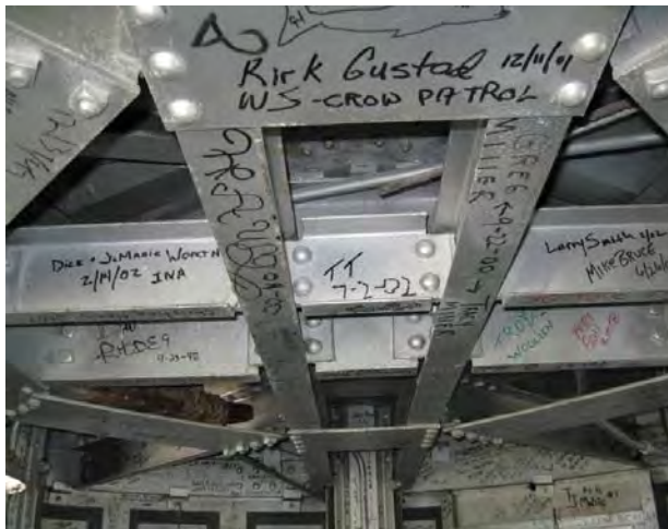
Figure C222. Steel framing of the lantern floor, surrounding wrought iron columns.
