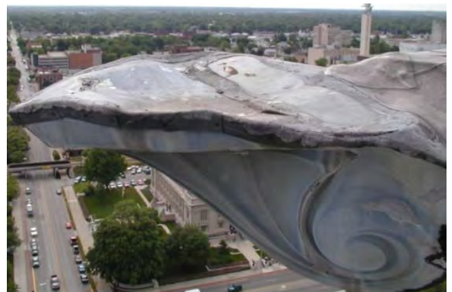
Figure D42. Dented projecting cap.
