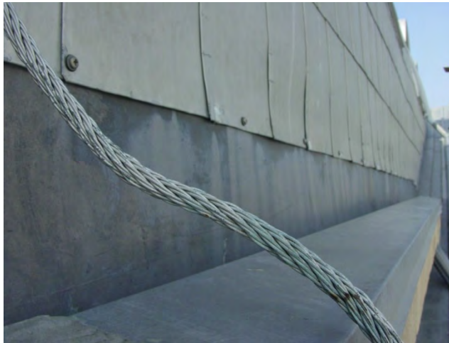
Figure C24. Water stains below the first course of shingles indicate that water may be able to get behind the shingles.
