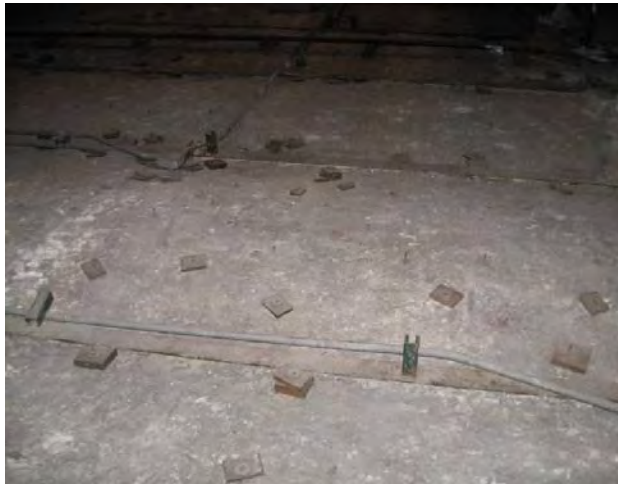
Figure C158. Anchors used to suspend the plaster ceilings from the corrugated metal arches.
