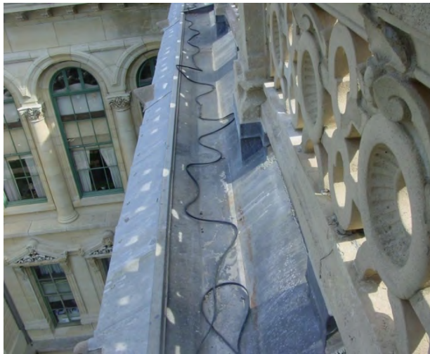
Figure C14. Heat trace cables added to the built-in gutters.
