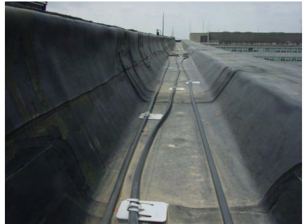
Figure C26. Heat trace cables installed in the built-in gutters.
