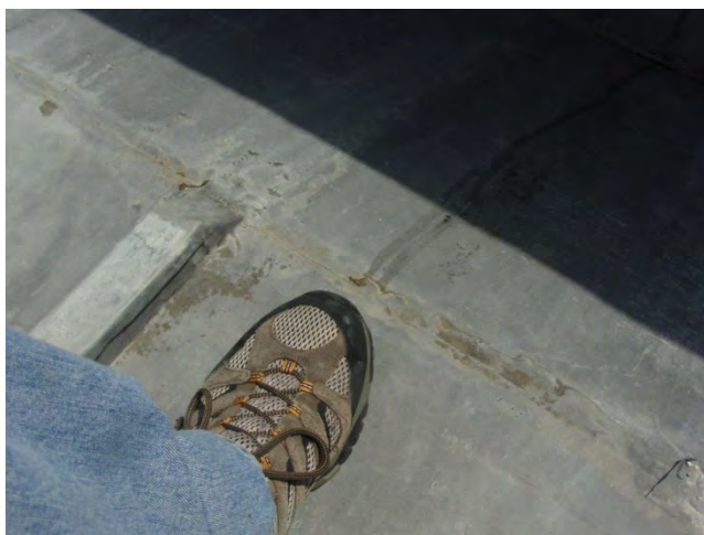
Figure C3. Water flowing out of the seam between the flat seam roofing and the batten seam roofing.
