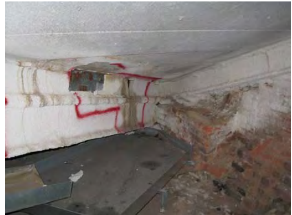
Figure C175. Typical 12WI valley beam at west wing.
