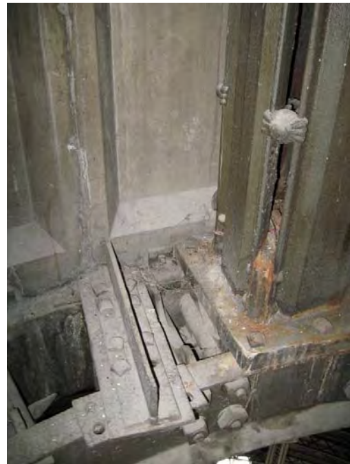
Figure C217. Built up wrought iron lantern columns fastened to the compression ring, aligning with the vertical trusses below.
