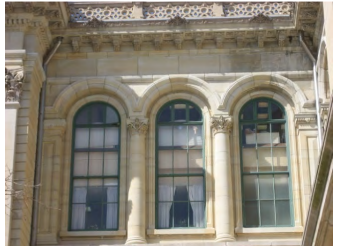
Figure C53. Surface erosion of limestone below cornice.
