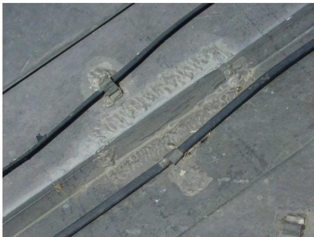
Figure C15. Previous repair that included soldering a patch to the existing lead coated copper.
