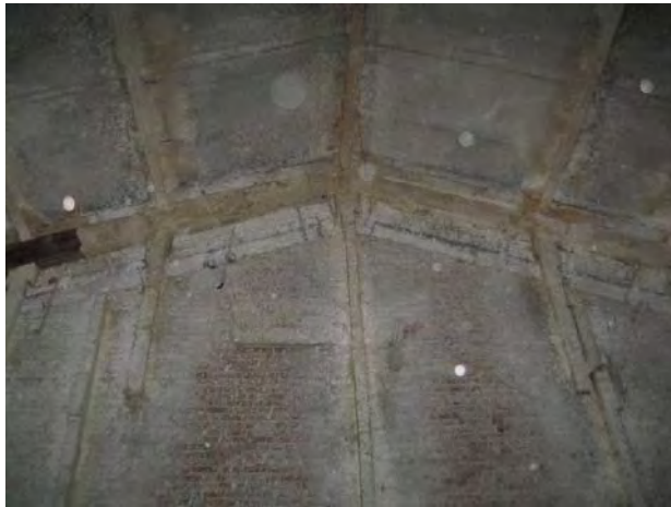
Figure C167. Close up view of ridge beam of east portico roof framing, showing remnants of wood framing, as well as precast concrete panels, which have replaced the wood sleepers and deck.
