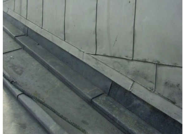
Figure B6. Batten seam roofing terminated behind the flat lock mansard shingles.
