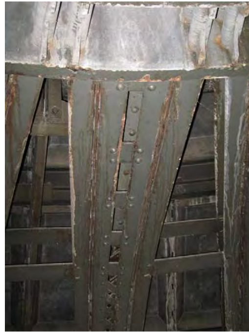
Figure C216. Built up wrought iron vertical trusses tying into the compression ring, aligning with the wrought iron columns above.
