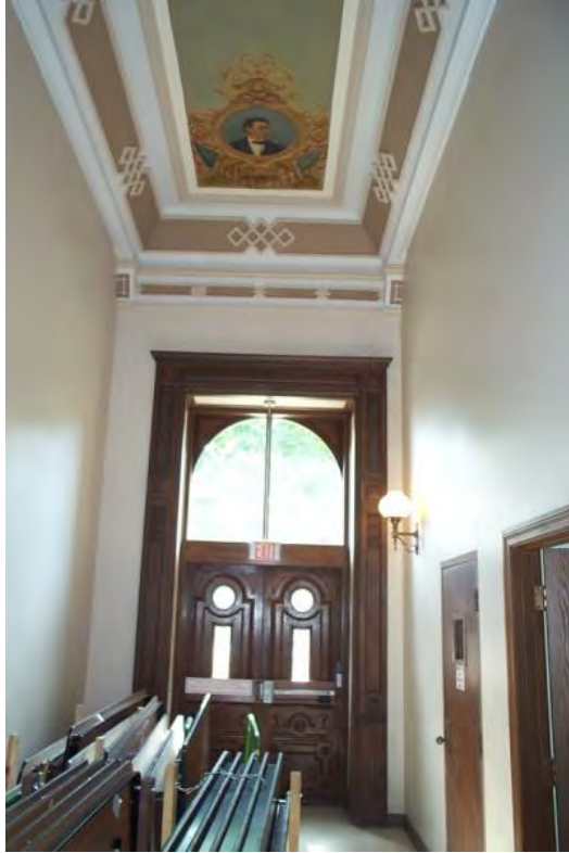
Figure B35. Original window trim in place around added exit door.
