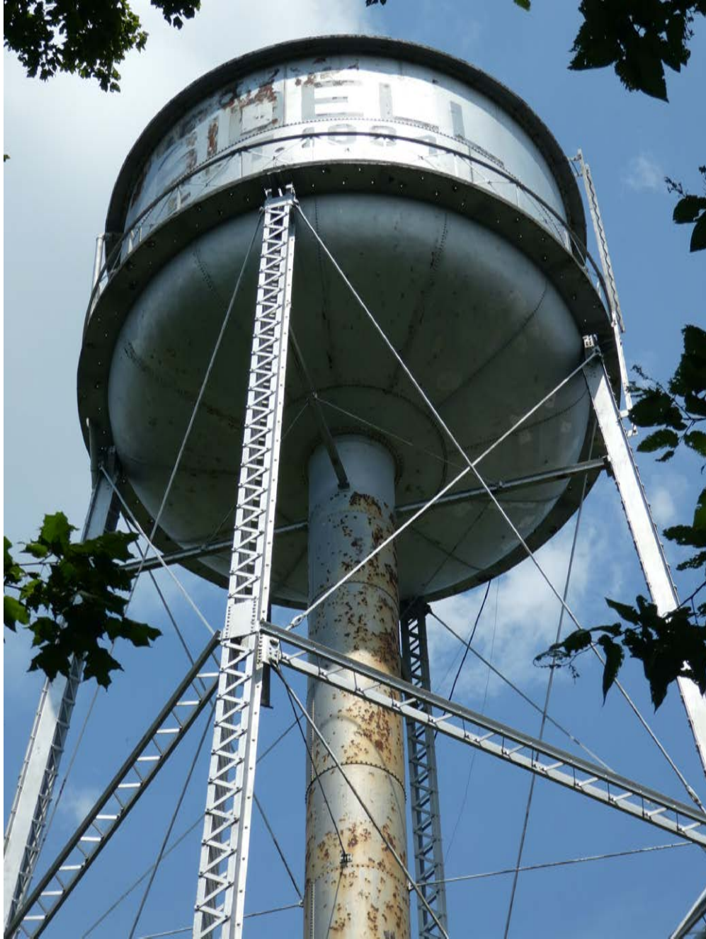
Figure 10. Detail view of storage tank underside, facing northeast.
