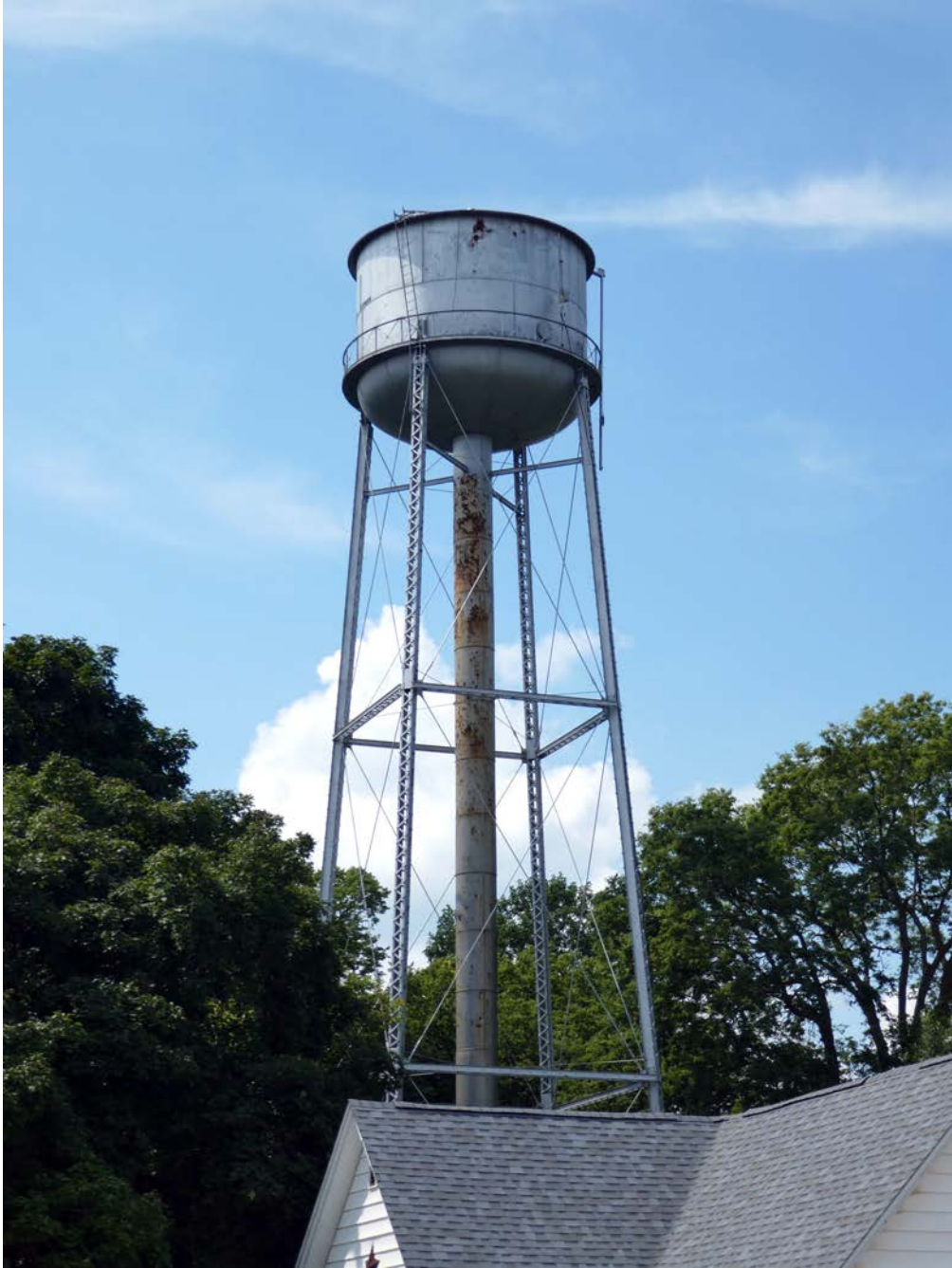
Figure 7. Sidell Elevated Water Storage Tank, facing northwest.
