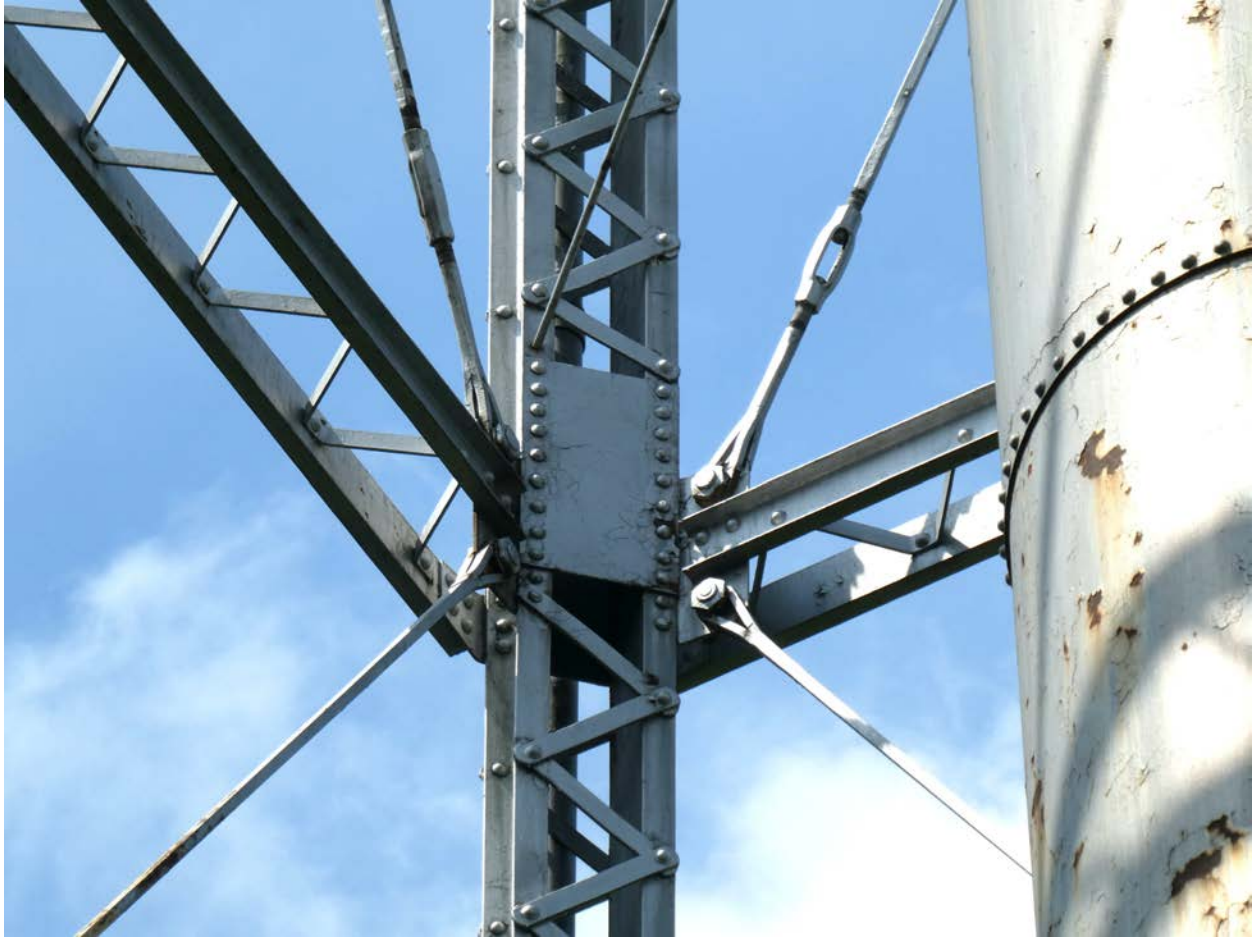
Figure 12. Detail view of interior leg and support, facing northwest.
