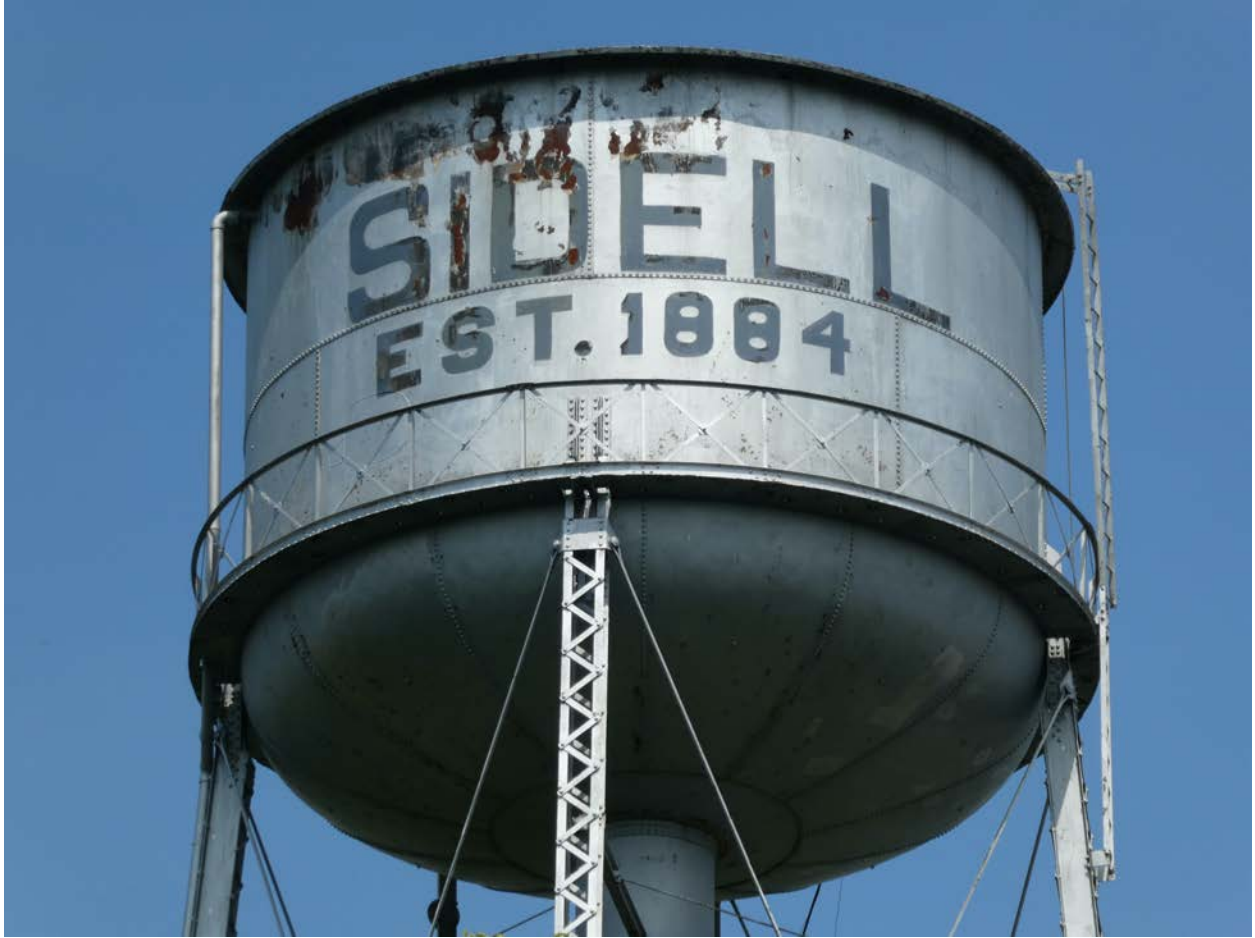
Figure 8. Detail view of storage tank, facing northeast.
