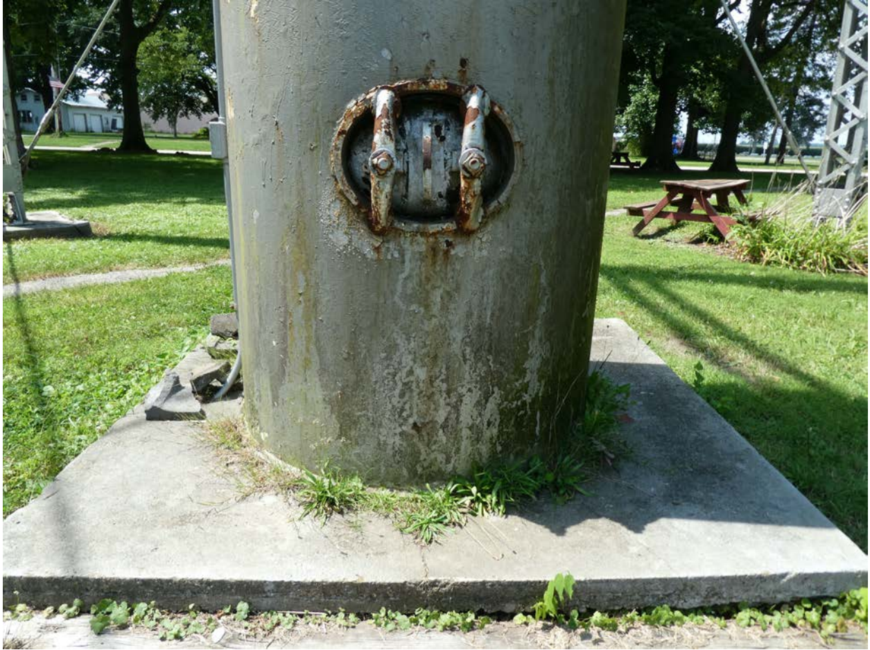
Figure 15. Detail view of riser access hatch, facing west.
