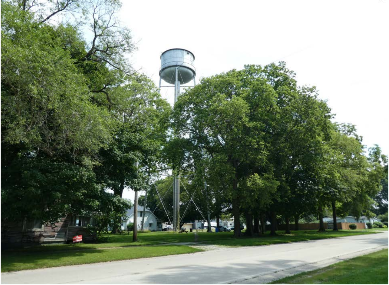
Figure 4. Sidell Elevated Water Storage Tank contextual view, to southeast.
