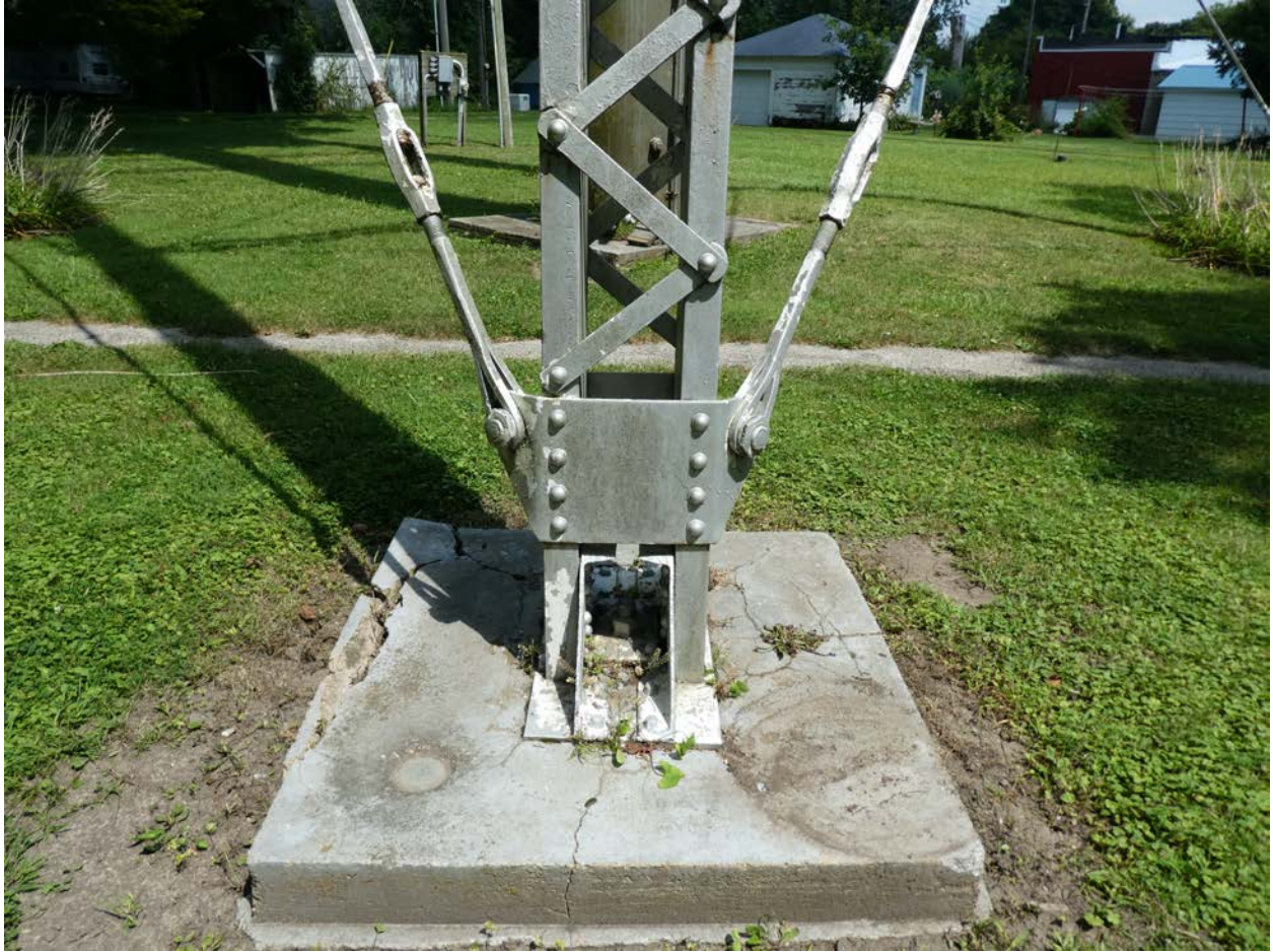
Figure 13. Detail view of tower leg support structure, facing northeast.
