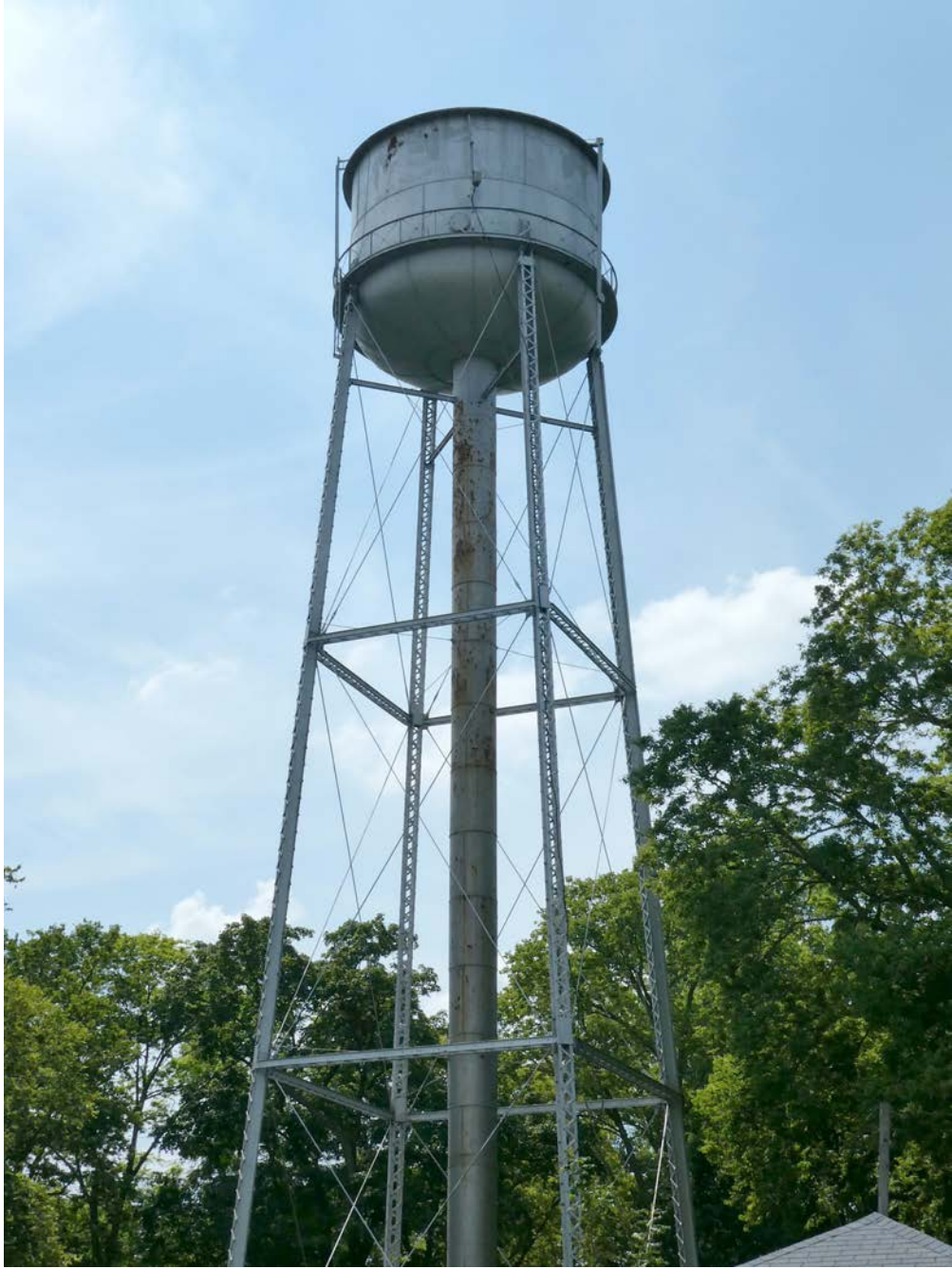
Figure 6. Sidell Elevated Water Storage Tank, facing southwest.
