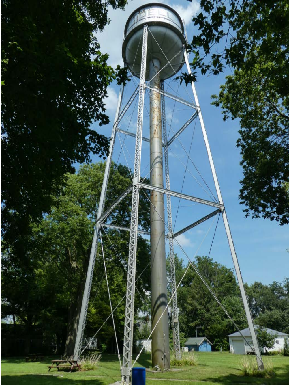
Figure 5. Sidell Elevated Water Storage Tank and Well House, facing northeast.
