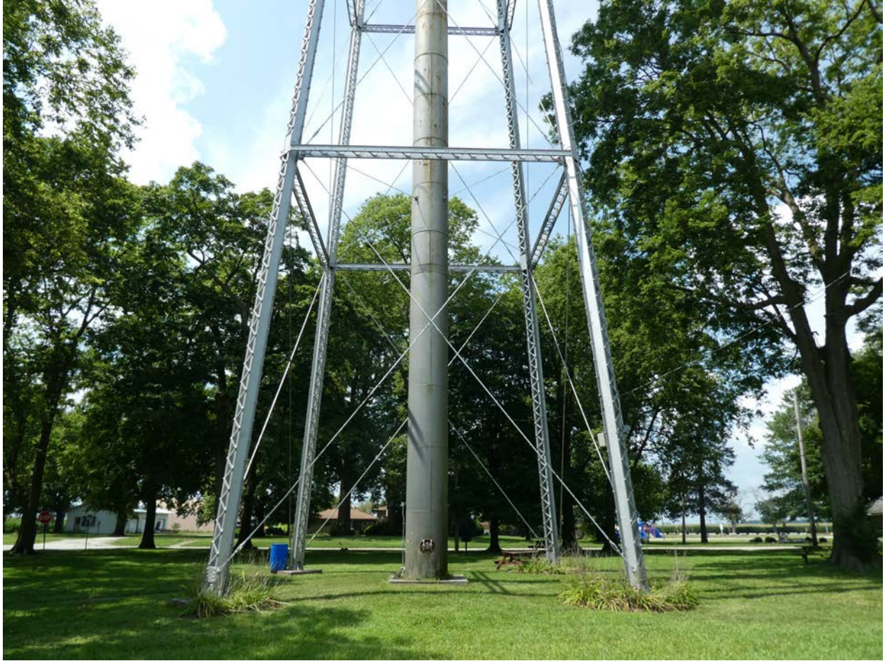
Figure 11. Detail view of support structure, facing west.
