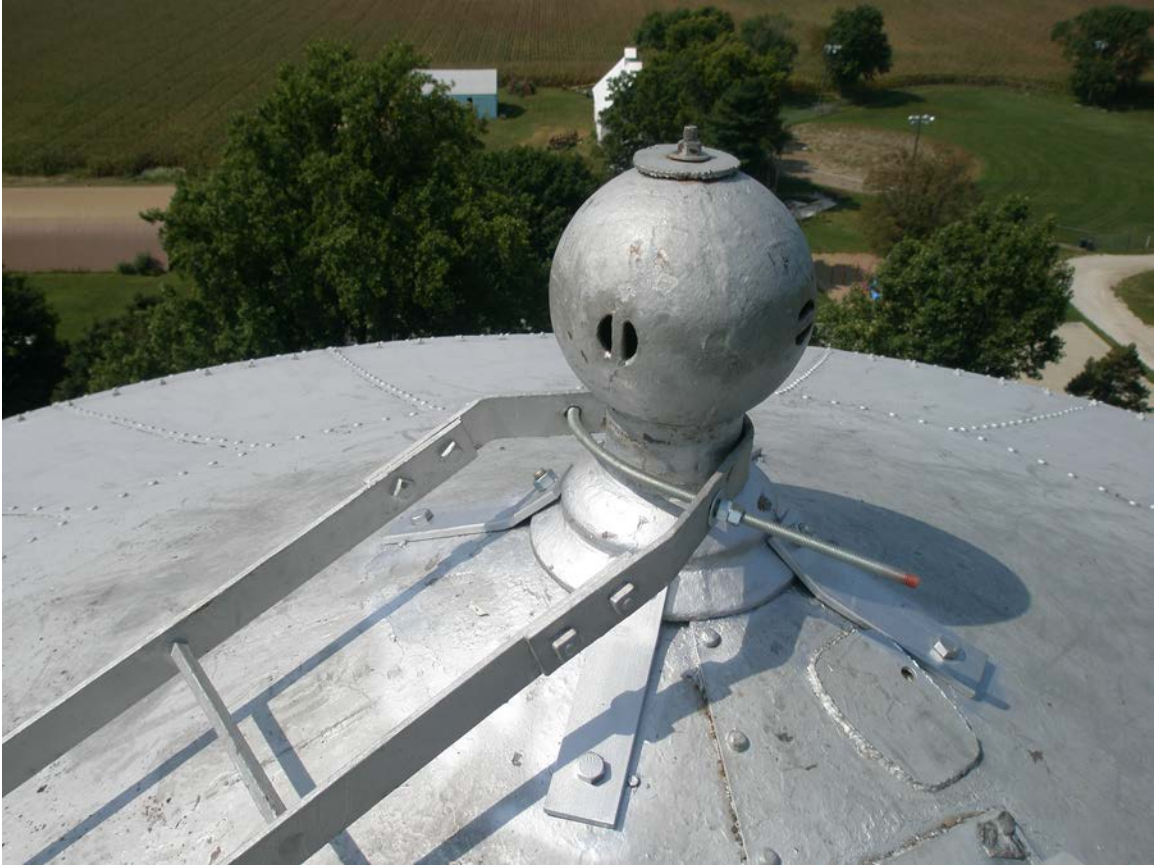
Figure 16. Photo of storage tank finial (courtesy of Lorin Kinney).
