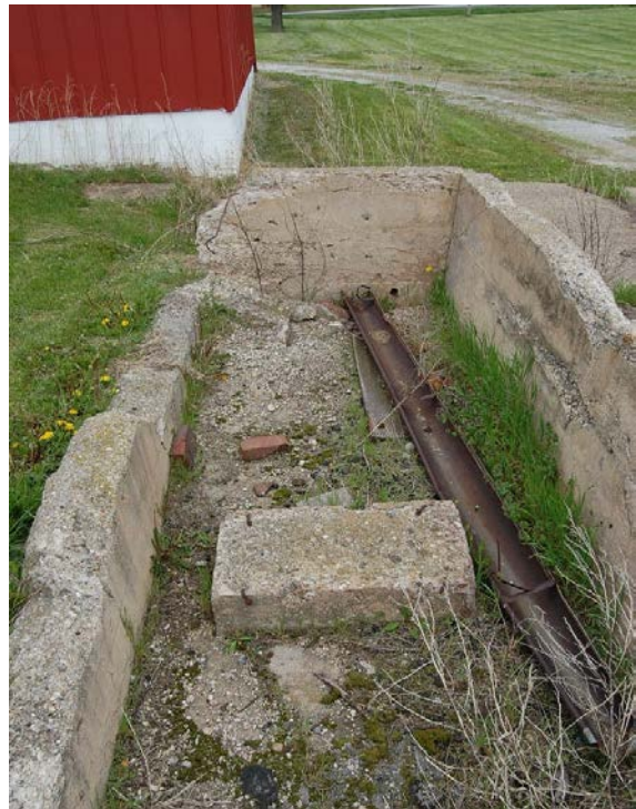
Figure 124. Details of the concrete water trough, or tank located west of the garage and milk house. Overflow water from the milk house passed via an iron pipe to this trough. Similarly, overflow water from this trough flowed out the east end of the trough and utilized a natural drainage way that headed off to the southwest. The raised “platform” in the center of the tank, with its iron anchor bolts, probably held a water tank heater that prevented the water tank from freezing over during the winter.
