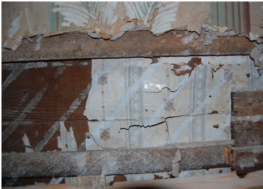
Figure 75. Two views of the interior wall finishes intact within the existing stair hall closet. This interior wall surface helped determine the sequence of events associated with the interior of this dwelling. Based on this remnant wall section, the original dwelling walls (and probably ceiling) within the main room of the house were covered with horizontal tongue and groove planks and applied over a black oiled paper. The plank wall surfaces were then covered with wallpaper, whereas the ceilings may have been painted. Over this surface, sometime during the later nineteenth century, lath were applied on a diagonal (using machine cut nails), and subsequently surfaced with plaster (and presumably wallpaper). Later, during the early twentieth century, this original lath was removed, and a second episode of lath was applied on the horizontal (using wire drawn nails). Remnants of the plaster and wallpaper of this latest episode are intact within the closet.
