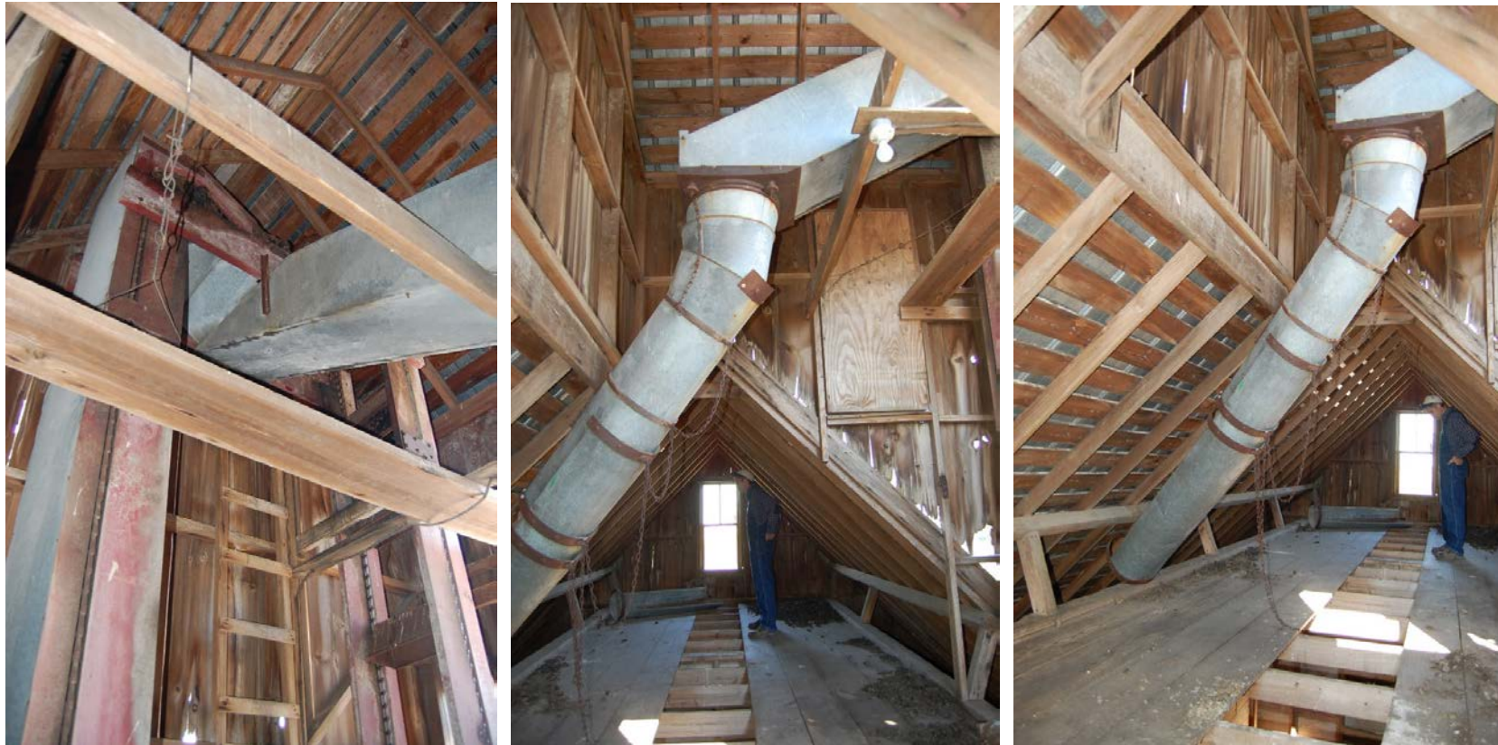
Figure 143. Three views of the headhouse and the cup elevator.
