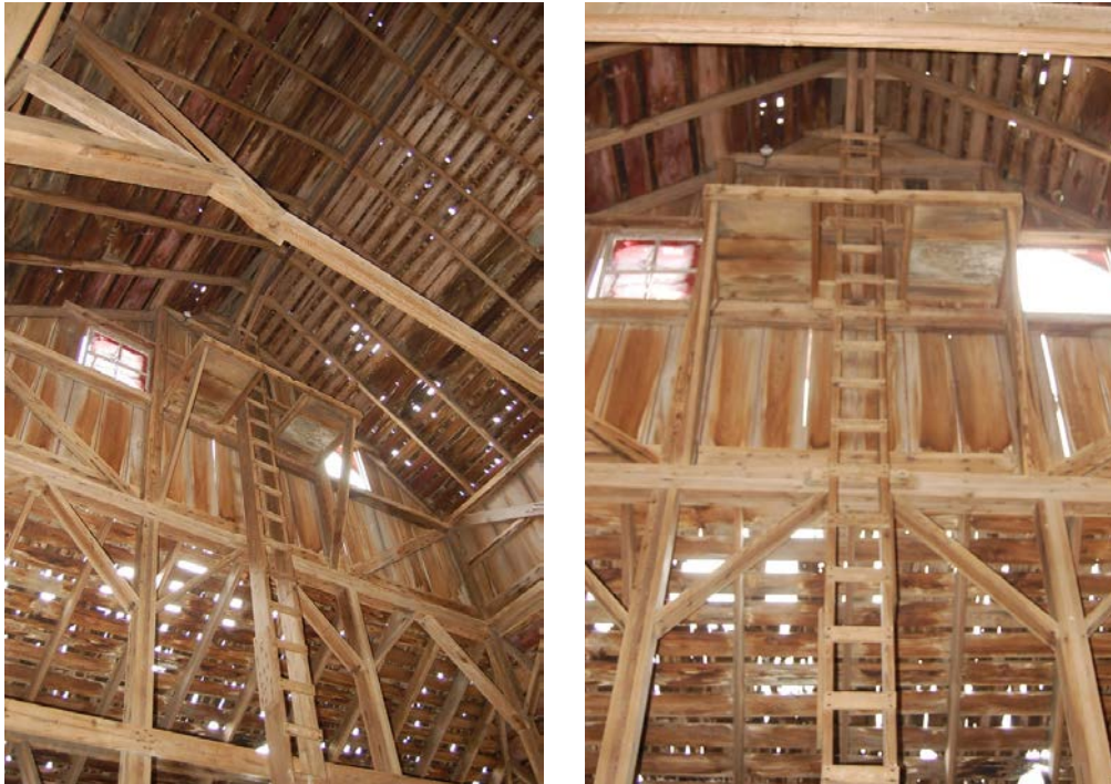
Figure 104. Two views of the ladder and raised platform located along the south end of the hay loft. This raised platform was used by workers operating the hay carrier. A rope “chute” for operation of the hay carrier (or “unloader”) was built into the back side of the ladder.
