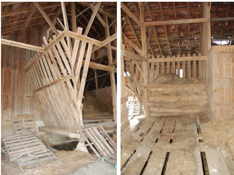
Figure 100. The majority of the original feed bunks and hay racks within the loafing shed area had been removed within the recent past. Nonetheless, the west end of the combination feed bunks and hay racks remained intact (left). The view at right is taken from within the hay loft area that extends into the loafing shed.
