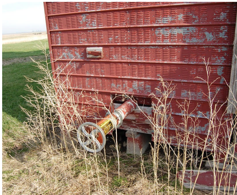
Figure 135. Miscellaneous details illustrating changes associated with the conversion of the corn crib to shelled corn (from ear corn). Top: detail of overhead grain shoot, and reinforced floor joists to handle the movement of the grain and the increased overhead weight, respectively. Bottom: detail of exterior slotted metal sheathing and central conveyor for removal of shelled corn.
