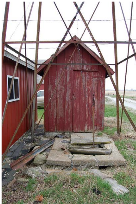
Figure 123. Three views of the frame milk house, with it's interior concrete water trough, or tank (for temporary storage of milk stored in large metal milk cans). This tank would have been filled with water pumped from the adjacent well by the overhead windmill. Overflow water from this tank would have passed via iron pipe to the nearby animal water trough (which was located slightly downhill from the milk house).
