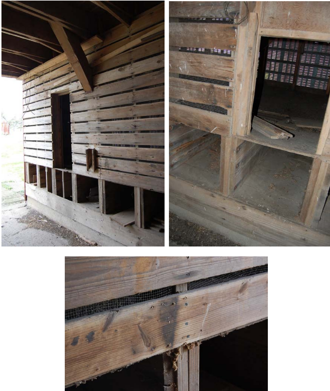
Figure 134. Two views of the corn cribs located each side of the central aisle. As originally constructed, the bins were designed with a flat floor, wood slatted “skin”, and long narrow hinged doors along the aisle for unloading the ear corn. Sometime during the middle twentieth century, the crib was retrofitted for handling shelled corn. At that time, a raised and sloped floor (with under-floor conveyor system) was installed, the structural system was strengthened, the exterior wood slats were replaced with slotted metal panels, and the interior surface of the wood slats was covered with wire mesh. Top left: note removal of original doors and presence of new grain shoot. Top right: note raised, sloped floor. Bottom: note “ghost” of original hinge for removed door.
