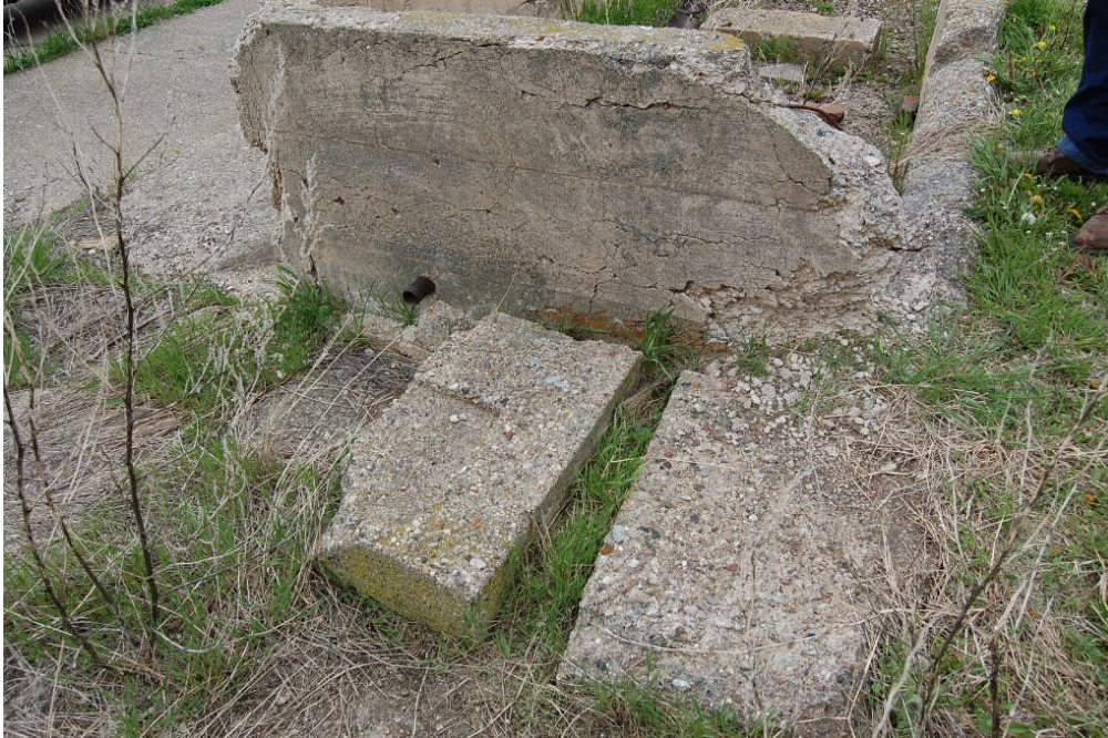
Figure 126. View of the east end of the water trough. Note the iron pipe overflow near the base of the tank. The function of the two concrete pads is unknown.
