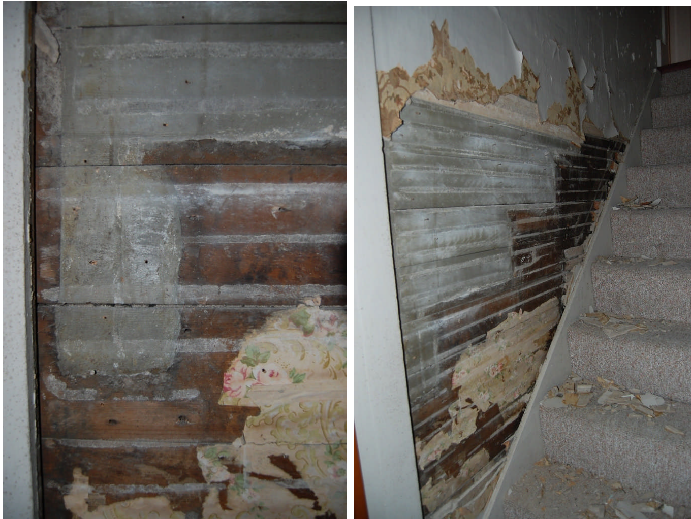
Figure 80. Two views of the walls located in the existing stairway documenting the location of the original stairs, and the character of the wall finishes above and below the original steps.
