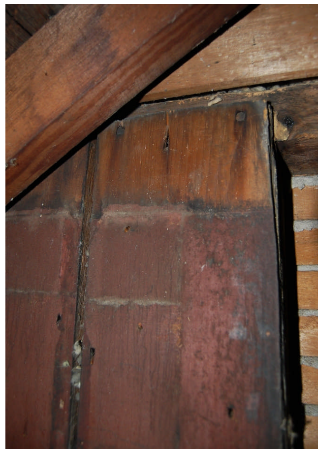
Figure 72. Detail of the original exterior surface of the one-room, 1 ½-story dwelling illustrating the character of the board and batten siding, as well as the location of an original window opening (left). The image at right also indicates that a relatively wide molding or trim board was located at the eave. This picture also indicates horizontal paint/dirt lines and nail holes (associated with machine cut nails) once associated with horizontal siding that had been applied over the original board-and-batten siding. This siding appears to have been applied prior to the expansion of the house—and the raising of it to a full two stories in height. The original board-and-batten siding appears to have been painted with a red paint.
