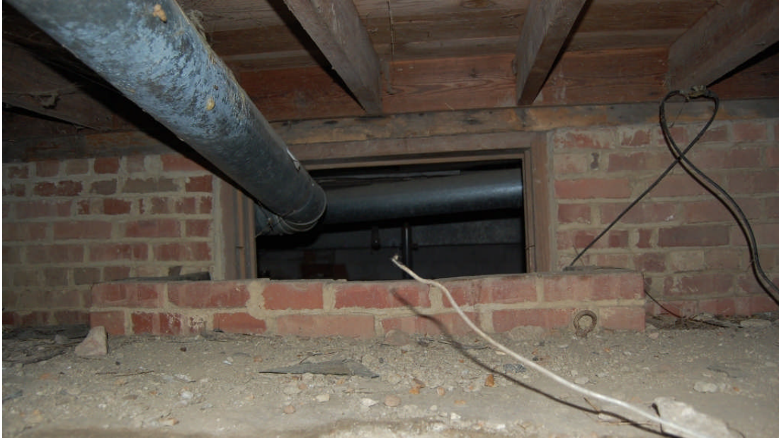
Figure 70. Detail of original brick foundations under original one-room dwelling illustrating the encapsulated window and window well associated with this early structure.
