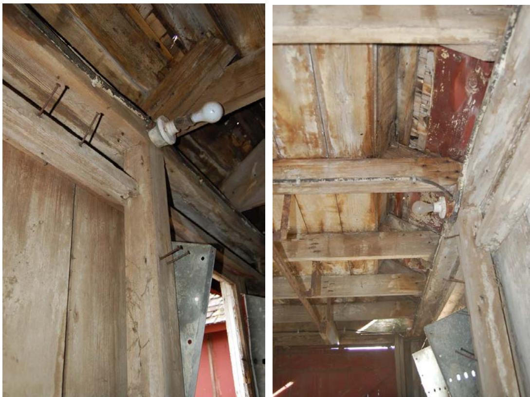
Figure 111. View of framing details within the side wings. Note the boxed-in character of the eave (right) which would have prevented hay from accumulating within the inaccessible location overhead.
