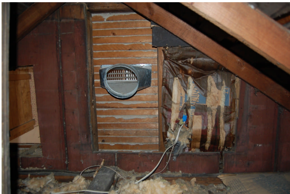
Figure 72. Detail of the original exterior surface of the one-room, 1 ½-story dwelling illustrating the character of the board and batten siding, as well as the location of an original window opening (left). The image at right also indicates that a relatively wide molding or trim board was located at the eave. This picture also indicates horizontal paint/dirt lines and nail holes (associated with machine cut nails) once associated with horizontal siding that had been applied over the original board-and-batten siding. This siding appears to have been applied prior to the expansion of the house—and the raising of it to a full two stories in height. The original board-and-batten siding appears to have been painted with a red paint.
