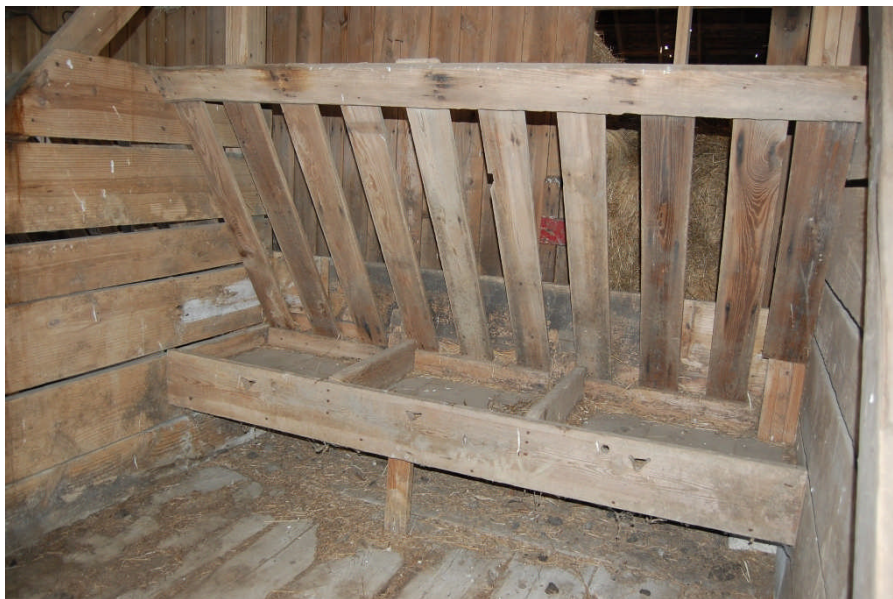
Figure 87. Of the three stalls present within the west section of the barn, one had a deep box manger without a hay rack (top; designed to accommodate a single animal) and three had shallow box mangers with overhead hay racks (bottom; with each stall designed to accommodate three smaller animals). The deep box manger represents the original style manger, with the other three representing replacement mangers. Although the original deep mangers were designed for use with draft horses, it is unclear as to the function of the later replacement managers.
