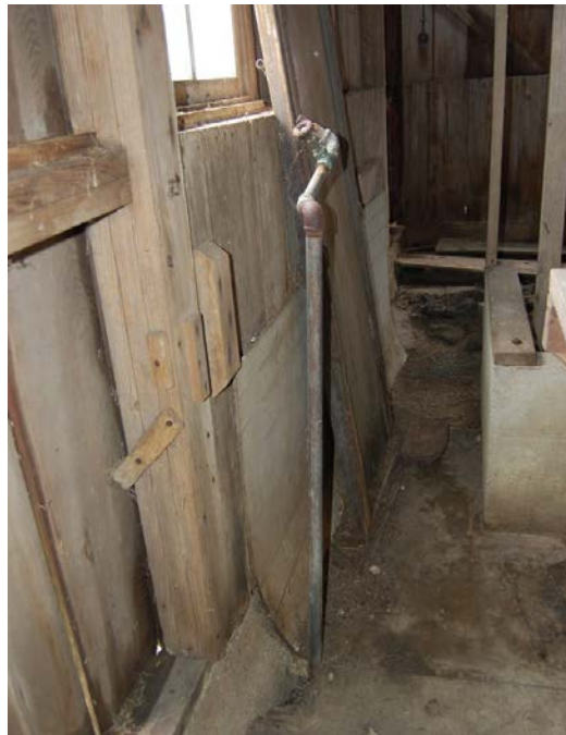
Figure 120. Running water delivered by underground pipe to the barn was a later modification to this structure. The original source of water for the animals in the barn was a nearby well and associated water trough east of the barn. A shut off valve was located immediately outside the barn opposite this standpipe. The date of this modification is not known. Additionally, there is no evidence of a cistern or well dedicated solely to barn use.
