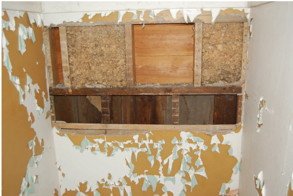
Figure 71. Second story framing detail illustrating the original rafter plate of the one-room, 1 ½-story dwelling. During the early years of the twentieth century, this small structure was expanded greatly, in both floor plan space and height. This photograph illustrates the expansion of the original short knee walls to full-height walls at this time.
