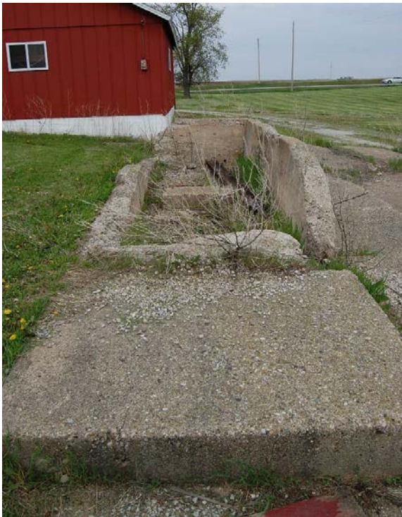
Figure 124. Details of the concrete water trough, or tank located west of the garage and milk house. Overflow water from the milk house passed via an iron pipe to this trough. Similarly, overflow water from this trough flowed out the east end of the trough and utilized a natural drainage way that headed off to the southwest. The raised “platform” in the center of the tank, with its iron anchor bolts, probably held a water tank heater that prevented the water tank from freezing over during the winter.
