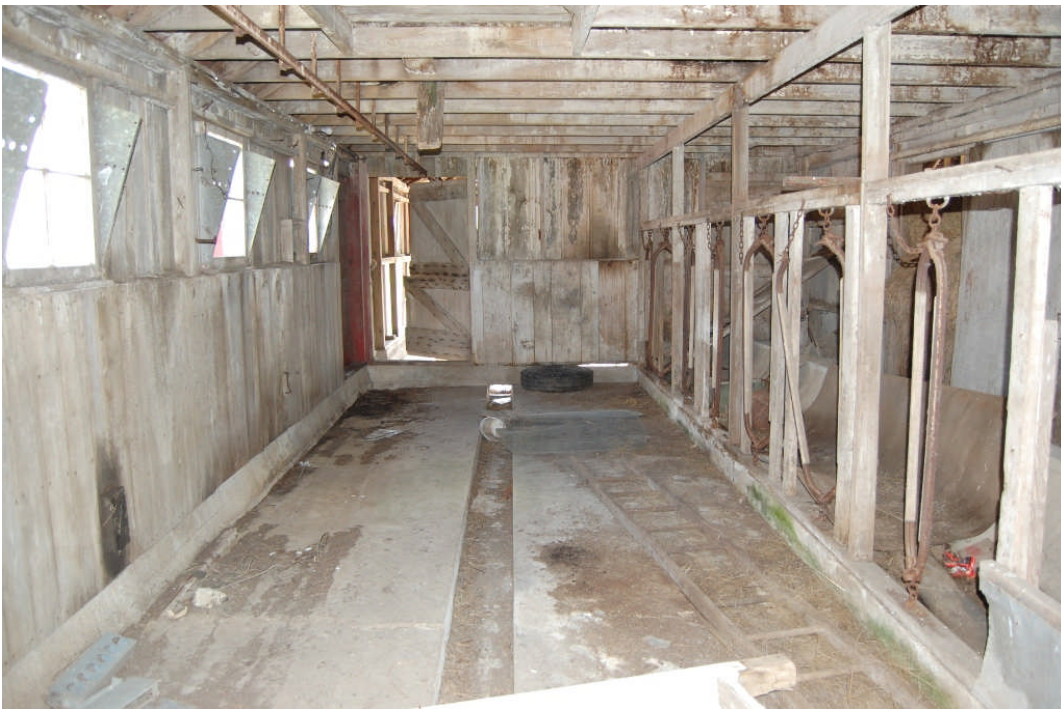
Figure 91. Two views of the milking parlor, taken from within the litter alley. Top: Looking north. Bottom: Looking south. Note the presence of the tubular steel stanchions within a wooden framework, an overhead track for removal of litter, and the overall white character of the room (as it had been painted white).
