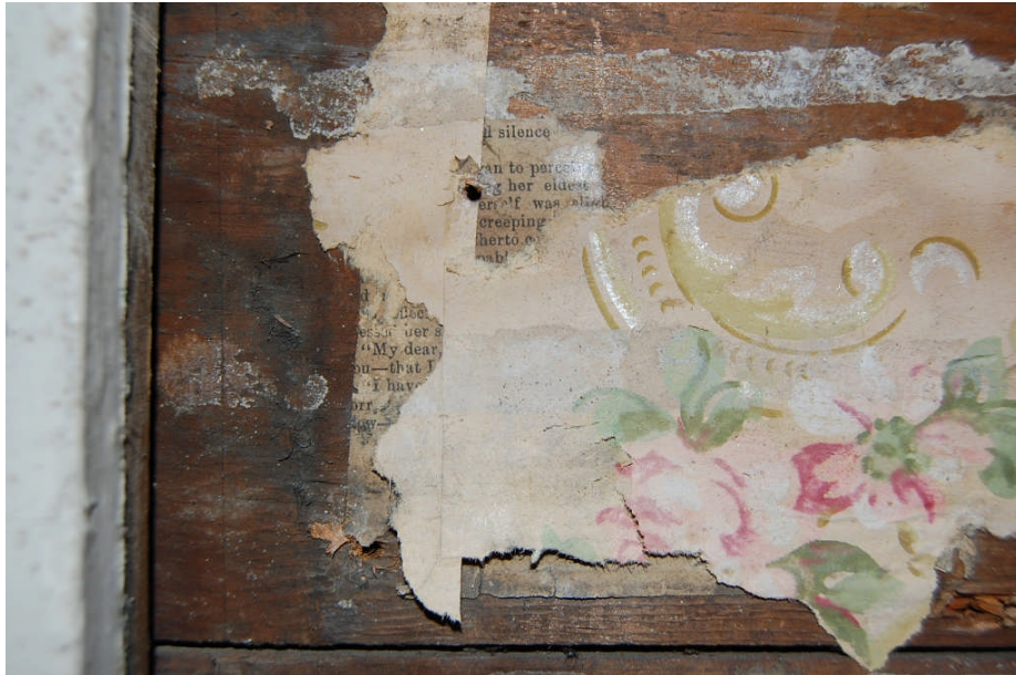
Figure 78. Detail of the newsprint applied directly over the unpainted plank wall surface. In turn, the wallpaper was applied over the newsprint, and finally the plaster (with horizontal lath; represented by the horizontal white line) was applied over the wallpaper.
