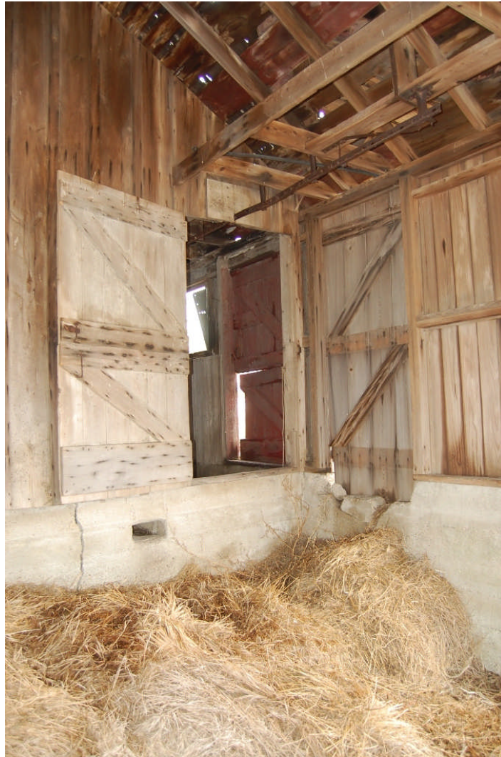
Figure 103. View of the northeast corner of the loafing shed area, illustrating doors leading into the milking parlor (left), and into the adjacent silo connector (right). Based on the character of the concrete threshold (which appears to have been broken through the original concrete foundations), it appears that the doorway that leads into the small room that accessed the silo was not original to this structure. As such, the original barn may not have been designed to feed silage to the dairy cattle. Also note the presence of the floor drain, and overhead litter carrier track—both of which dumped the cattle waste into this loafing shed area. Not illustrated in this photograph is a “catwalk” (with railing) that connected the silo door and the doorway located on the south end of the milking parlor’s feed aisle. This walkway and door were not original to the barn—probably constructed when the silo was added. This modification to the barn—consisting of the construction of the silo and the introduction of ensilage as feed—marks one of the most significant changes that affected the functional use of this barn.
