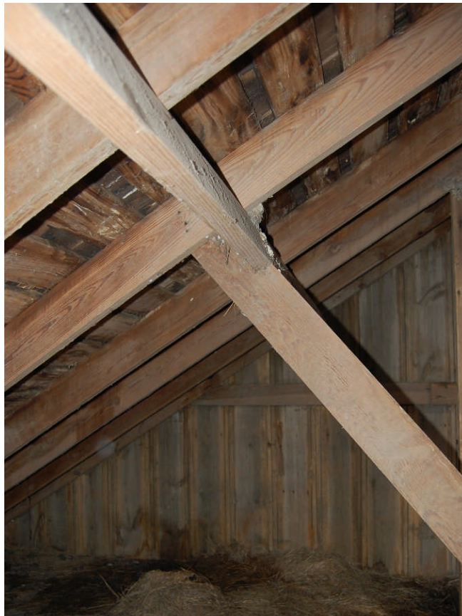
Figure 110. Detail of the queen post truss supporting the rafters within each of the side wings of the barn.
