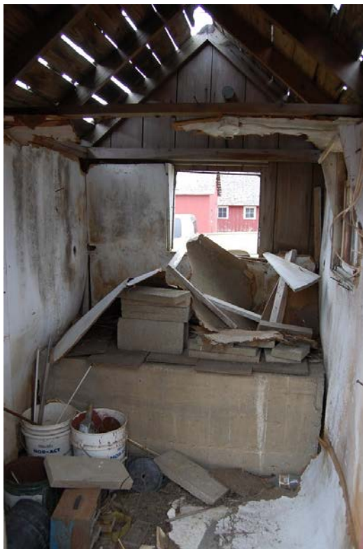
Figure 123. Three views of the frame milk house, with it's interior concrete water trough, or tank (for temporary storage of milk stored in large metal milk cans). This tank would have been filled with water pumped from the adjacent well by the overhead windmill. Overflow water from this tank would have passed via iron pipe to the nearby animal water trough (which was located slightly downhill from the milk house).
