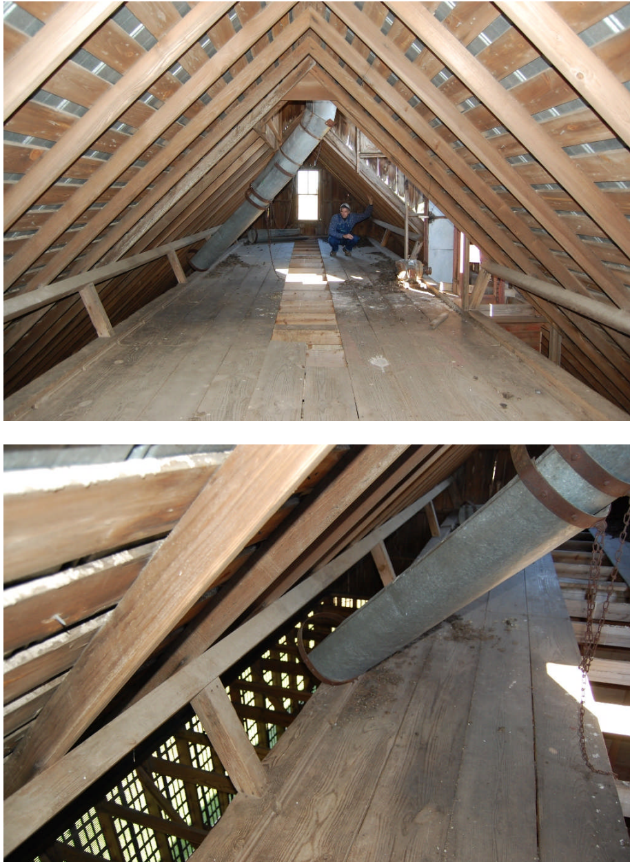
Figure 142. View from within the loft of the corncrib. The bins to each side, originally designed for ear corn, are accessed by the openings below the rafter plate. The grain bins over the central aisle are accessed by the openings running the length of the building in the center of the plank floor.
