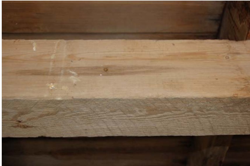
Figure 113. Lumber used within the construction of the barn was a hard yellow (or Southern) pine. The lumber had been cut from the tree with a circular saw. Much of the lumber used in the construction of the barn was in the form of planks which had been surfaced four sides (S4S). The above timber, representing one of the larger non-plank timbers used in the construction of this structure, was surfaced only on two sides (S2S).
