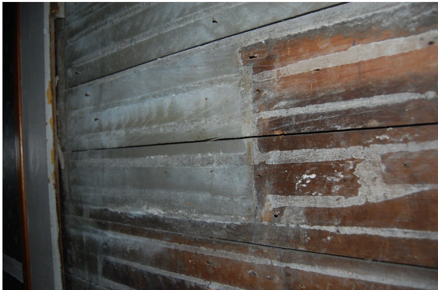
Figure 79. The “ghost” of the original stairs leading to the second story was preserved beneath the lath and plaster within the existing stairway. This evidence indicated that the original stairs were of the “winder” variety, with the doorway located along the south wall of the stair hall—opening into the small downstairs room of the original dwelling. As this photograph illustrates, the exposed plank walls leading to the upstairs were washed or lightly painted.
