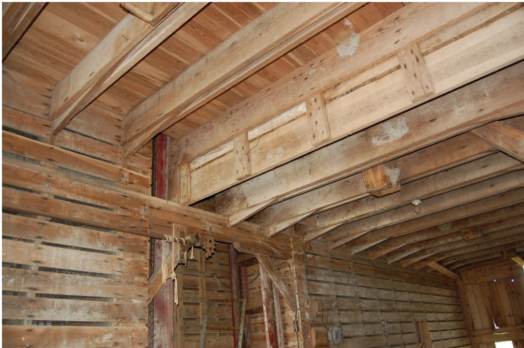
Figure 141. Overhead detail from within center aisle of corn crib illustrating the manner in which the original ceiling joists had been strengthened. This was done at the time the overhead storage area was converted from ear corn to shelled corn and/or grain—which would have increased dramatically the overhead load.
