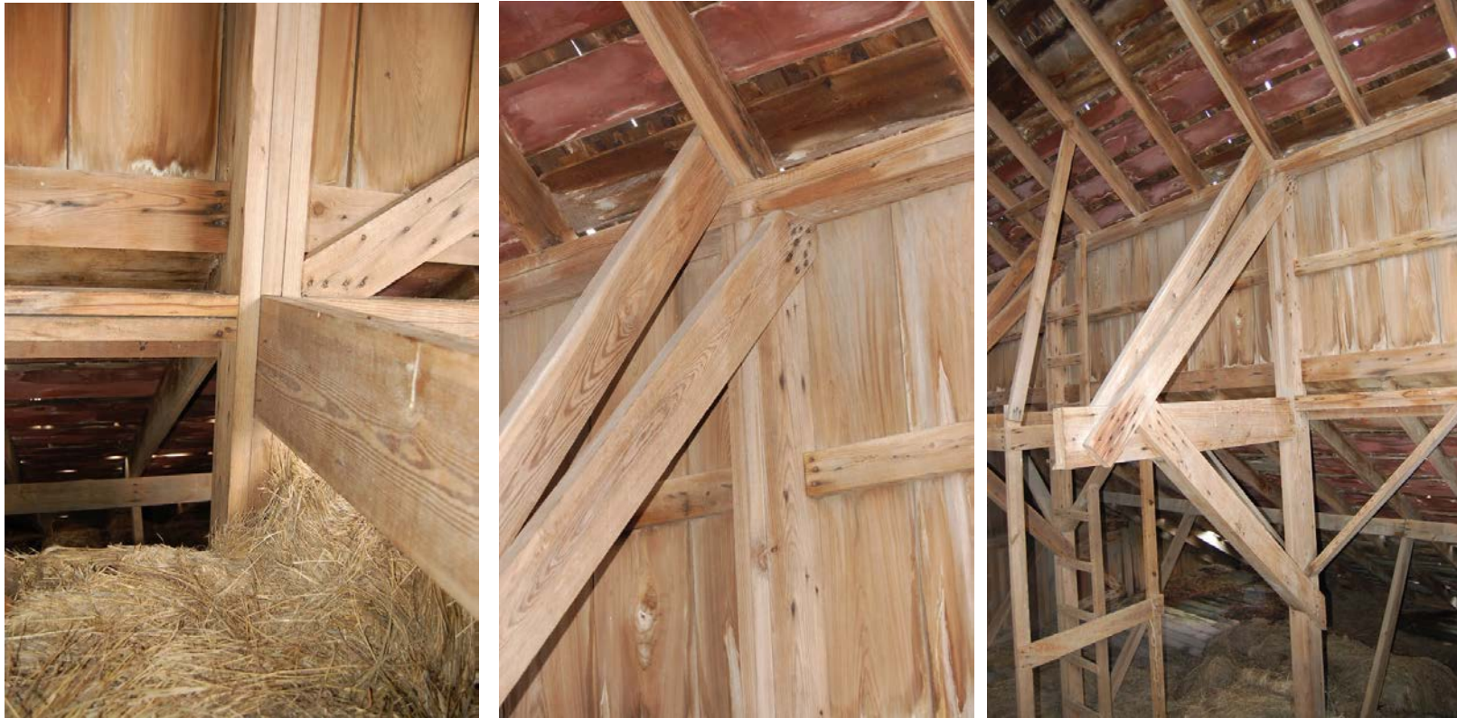
Figure 109. Three views of the barn’s framing system, taken from within the loft. This barn was constructed using “plank” construction methods. The materials used in the barn were predominately southern pine/fir that had been surfaced-four-sides (S4S). Wire-drawn framing nails were used extensively throughout the building. Note the use of wind bracing tied into the overhead rafters (center and right photograph). This may be an effort to give the barn’s roof some protection from severe wind damage—as tornados were feared by many a farmer. [A tornado may have just missed this farm in late summer 1927, as one struck the southwest side of Sibley doing extensive damage to that community at that time.]
