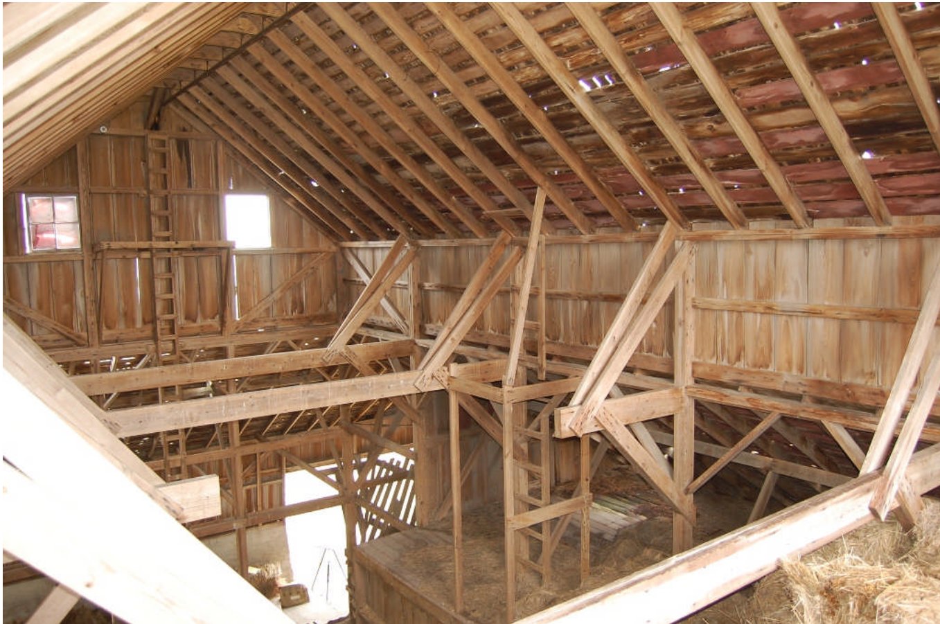
Figure 107. View of the upper framing system of the hay loft (looking southwest). The one large girt has been removed, probably to facilitate the loading of hay into the lower section of the loft.
