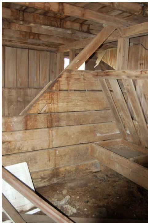
Figure 88. Four box stalls were located within the west section of the barn, which was originally designed for the care of draft horses. These stalls had plank side walls, with the upper two planks cut off in line with the diagonal brace forming the sidewall support for each stall. The stalls had thick plank floors set over a concrete surface. A floor drain drained the end of each stall. A wide litter aisle was located at the west end of each stall, separated by swinging gates that corresponded to each box stall. A single, sliding sash window was associated with each of the stalls along the exterior (west) wall.
