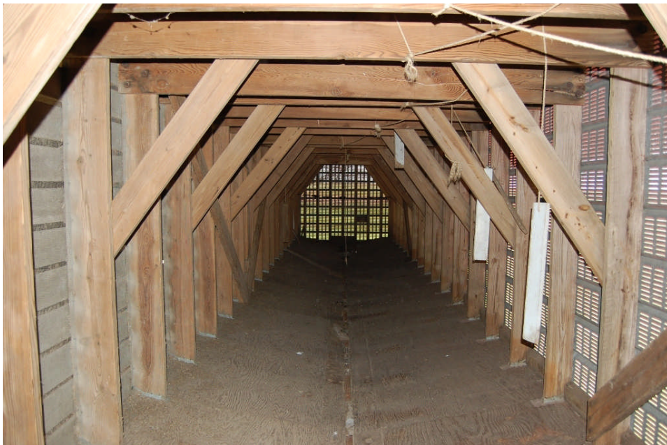
Figure 133. View looking south, down the center of the west bin of the corn crib. As originally constructed, this structure was designed to store ear corn and had a wood slat exterior skin. The current slotted metal siding and the sloped floor with recessed conveyor system is a later modification adapting the structure to storage of shelled corn.
