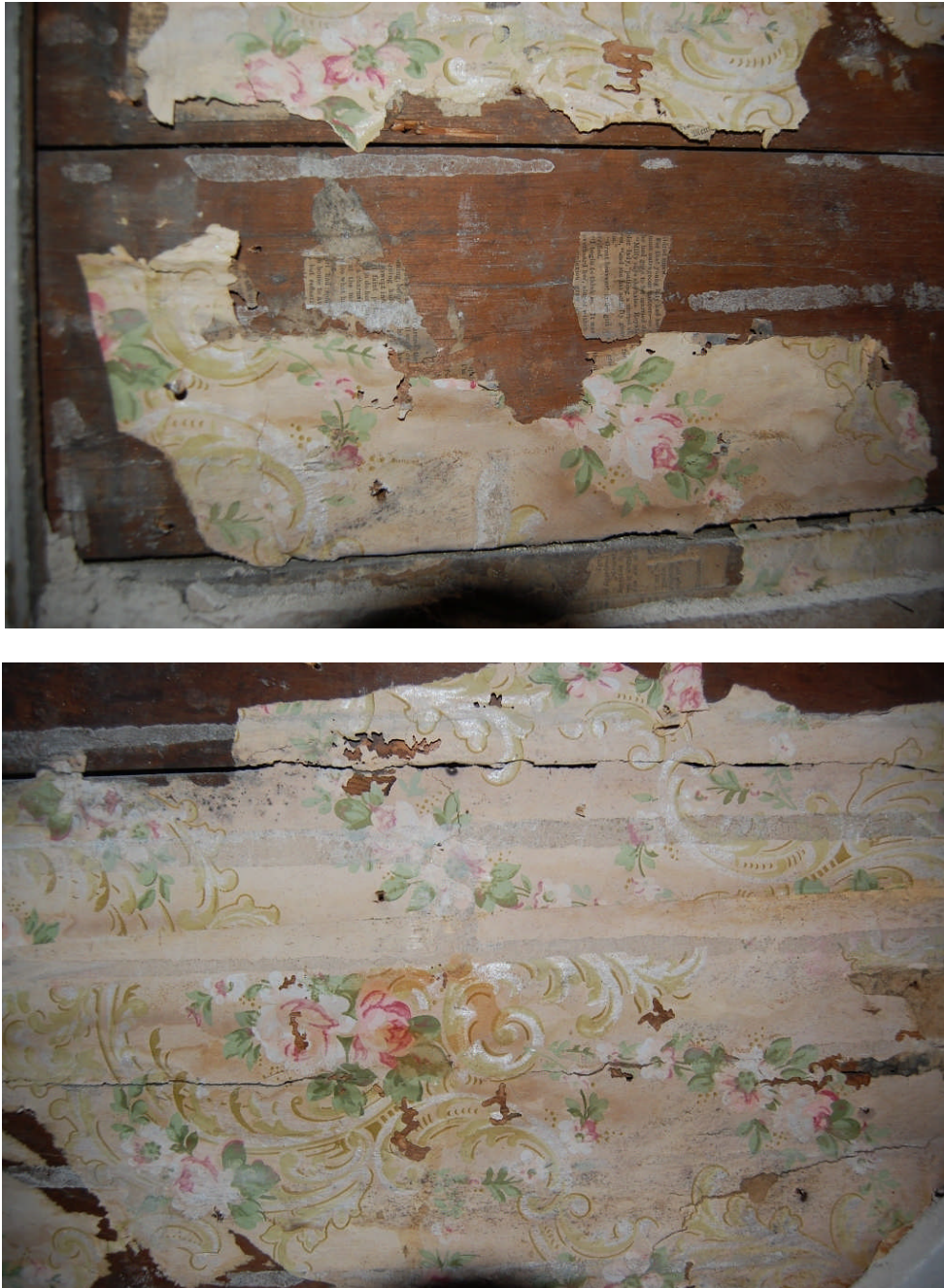
Figure 77. In contrast, the area within the original “under-the-stairs” closet had been covered with newsprint in lieu of wallpaper. At a later date, this newsprint was covered with a late nineteenth century wallpaper. Subsequently, with the re-configuring of the stairs, and the enlarging of the closet, the wall surface was covered with horizontal lath (attached with wire-drawn nails). The area within this early closet—unlike the room outside the closet—was never covered with the earlier episode of diagonal lath (and plaster). Both the newsprint and wallpaper surface had deteriorated substantially by the time the lath had been applied.
