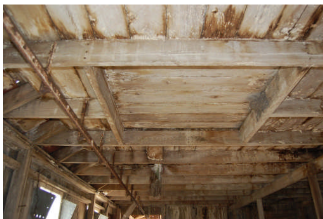
Figure 96. Centrally located within the ceiling over both the east wing (dairy parlor) and the west wing (horse stalls) was a large door accessing the hay loft overhead. This door allowed for hay and/or straw to be dropped down into the stall areas. Note also the metal track for use with a litter carrier.
