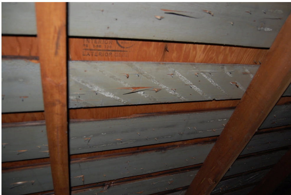
Figure 73. Details of existing house roof framing. The existing roof over the front portion of the house was constructed in a single episode using re-used materials (sheathing), as well as apparently newly purchased materials typical of an early twentieth century construction episode (southern pines, surfaced on four sides). The re-used sheathing included what appears to have been pieces of vertical board siding (not illustrated), as well as tongue-and-groove planking (exhibiting evidence of a lath and plaster finish having been applied over the original painted surface) (bottom photograph). This tongue-and-groove planking appears to represent the original interior wall and/or ceiling finishes of the circa 1870s house.
