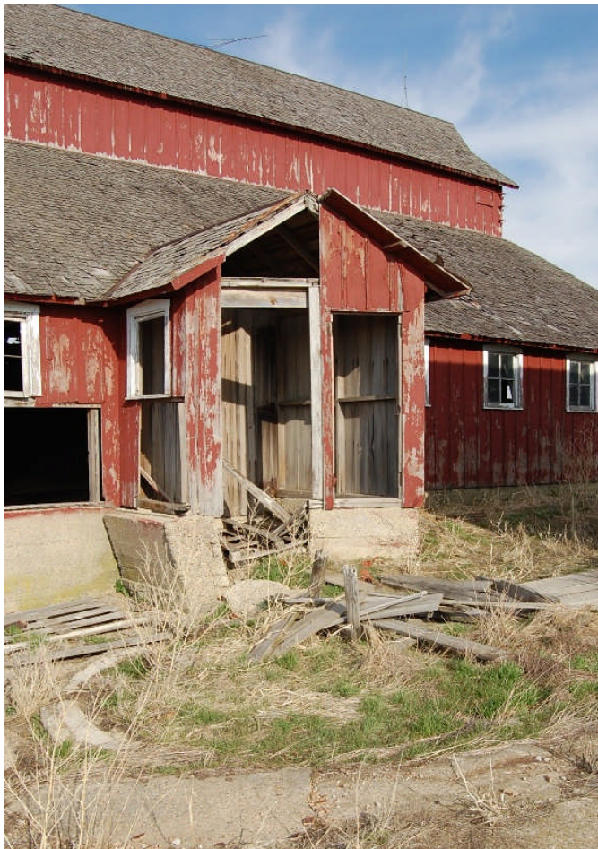
Figure 85. Located off the southeastern corner of the milking parlor was a small frame wing that connected the barn with a silo (which is no longer present). The silo was constructed of ceramic tile manufactured by the NATCO Company ( Country Gentleman , December 9, 1916; page 2132). This small frame wing (and presumably silo) was not original to the barn, but represents a later improvement to this structure.
