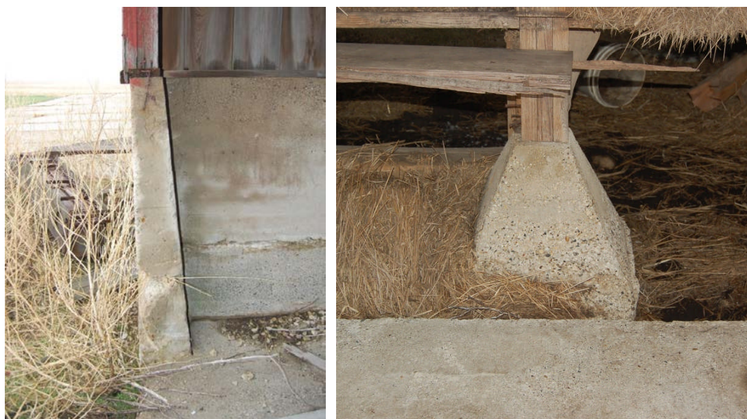
Figure 112. View of barn's poured concrete perimeter foundations (left) and piers (right).
