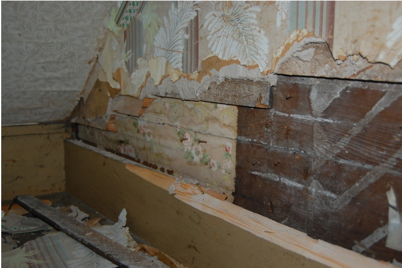
Figure 74. The current closet beneath the existing stairs is considerably larger than the original closet once present. As such, remnants of the outer room and interior closet finishes from the original circa 1870s dwelling were preserved in place. This picture depicts the transition from the inside of the closet (left) to inside of the main room (right).
