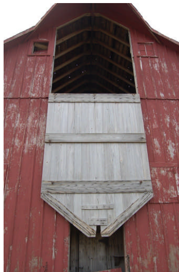
Figure 84. Each side of the large mow door (located on the north elevation of the barn) was located two windows and two small hinged doors. One window was located each side of the mow near the gable and furnished light and ventilation to those working in the mow. A second window was located low on this elevation and allowed light to enter the service aisle for each side of the barn and serviced the milking parlor on the east and the horse stalls on the west. The two small doors located above each of the lower windows had very different functions. The outer-most door on each side allowed access to the hay in the loft located above both the milking parlor and the horse stalls. The smaller and/or inner door accessed a frame chute that lead to the interior granary located immediately off the service aisle in the center of the barn.
