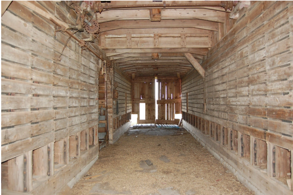
Figure 132. View looking south, down the central aisle of the corn crib. Note the elevator “niche” on the left center of the aisle, and the overhead truck or wagon lift for dumping corn (and other grains) into the elevator.
