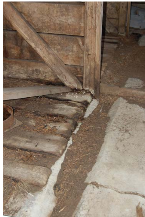
Figure 88. Four box stalls were located within the west section of the barn, which was originally designed for the care of draft horses. These stalls had plank side walls, with the upper two planks cut off in line with the diagonal brace forming the sidewall support for each stall. The stalls had thick plank floors set over a concrete surface. A floor drain drained the end of each stall. A wide litter aisle was located at the west end of each stall, separated by swinging gates that corresponded to each box stall. A single, sliding sash window was associated with each of the stalls along the exterior (west) wall.
