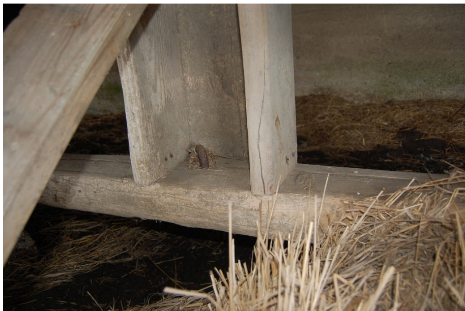
Figure 101. Located beneath the raised floor of the south end of the hay loft—and accessed from within the loafing shed area—was a lack bolt anchored to a heavy beam counterbalanced against the concrete foundations of the barn. This lack bolt probably held a pulley which was part of the operating system for the overhead hay carrier. The rope from the hay carrier traveled down a chute (seen here) and would have been accessible to workers within the center of the loafing shed area. As there is no room for operating a horse at this location, it would appear that a stationary engine and mechanical hoist system was probably used to operate this hay carrier. The chute was integrated into the personnel ladder that accessed the overhead carrier and raised platform located at the south end of the loft.
