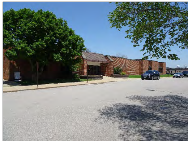
Figure 30. Facility 1948, facing northeast.
