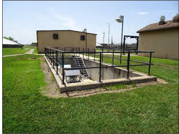
Figure 35. Facility 3295, facing southeast.
