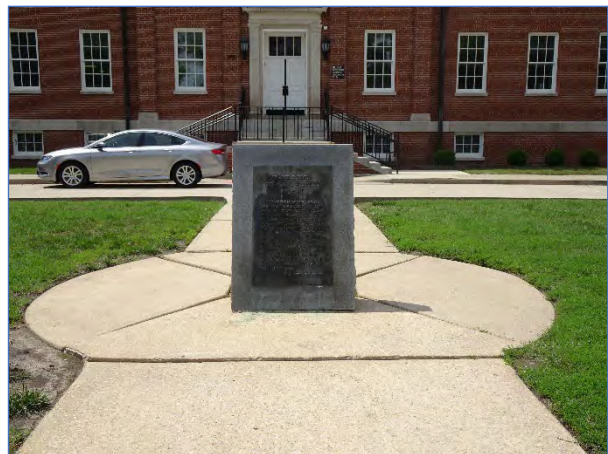
Figure 41. Facility 6005, facing south.
