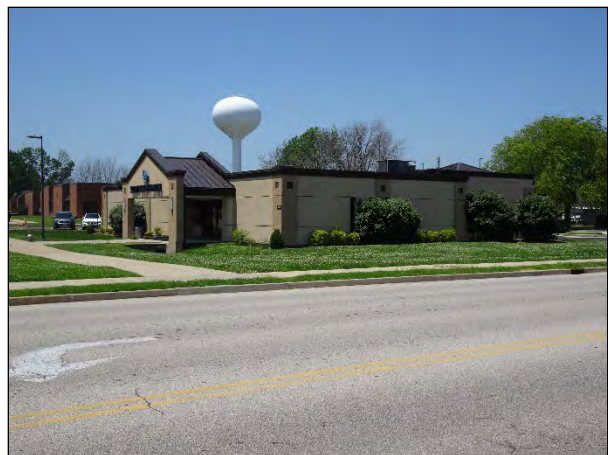
Figure 31. Facility 1950, facing northwest.
