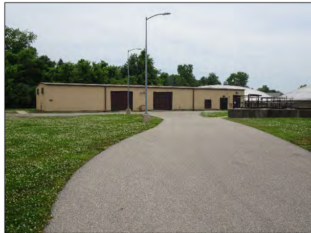
Figure 34. Facility 3292, facing east.
