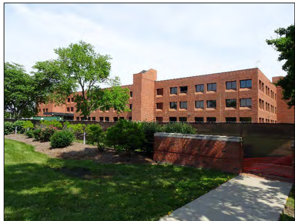
Figure 27. Facility 1600, facing southwest.
