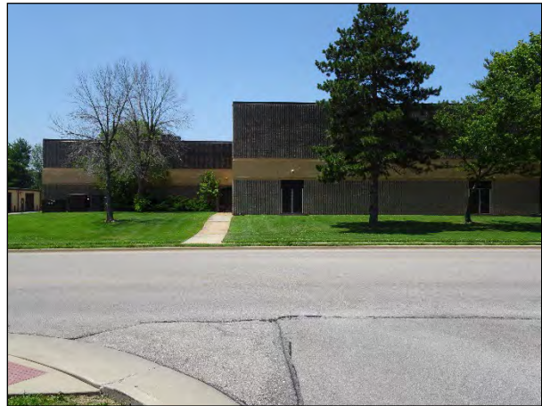
Figure 32. Facility 1987, facing west.
