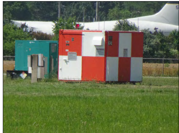
Figure 50. Facility 6742, facing south.
