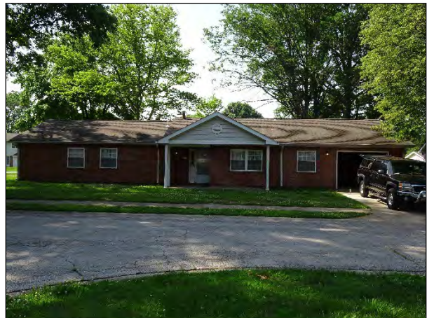
Figure 22. Facility 1481, facing northeast.
