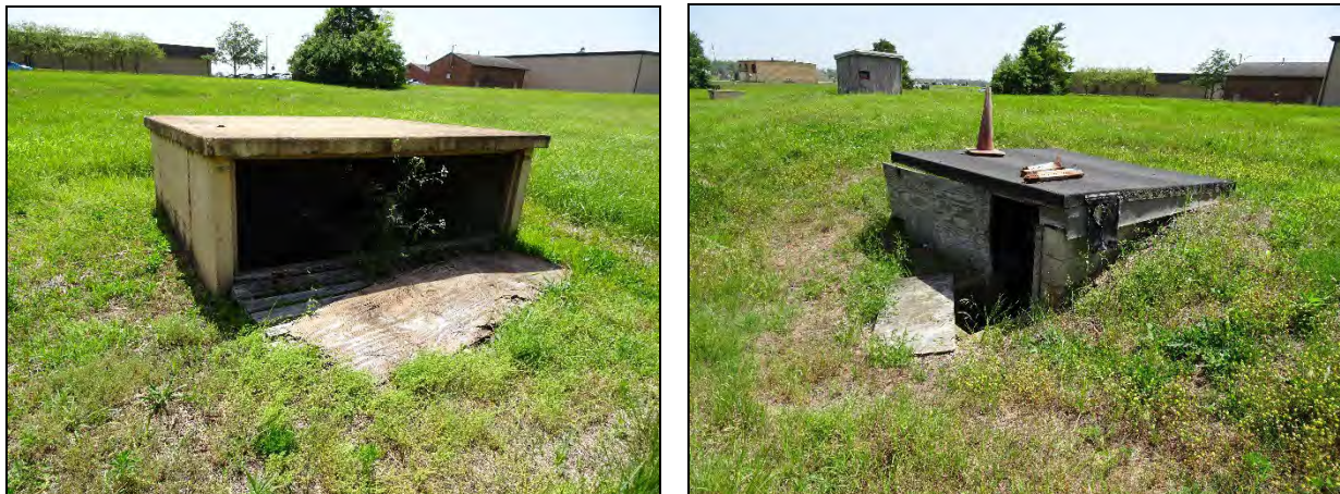
Figure 46. Facility 6160 concrete bunker, facing south (left); concrete bunker, facing southeast (right).
