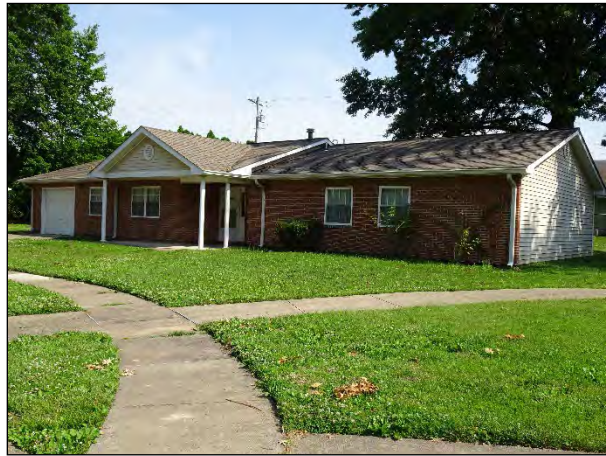
Figure 19. Facility 1475, facing west.
