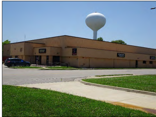
Figure 29. Facility 1934, facing southwest.
