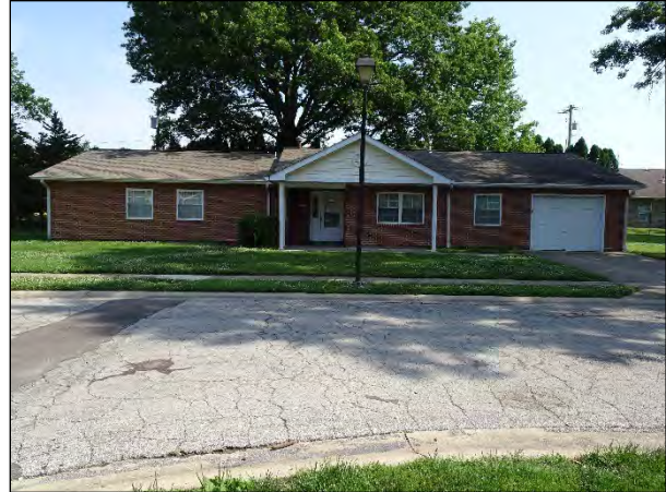
Figure 18. Facility 1473, facing west.
