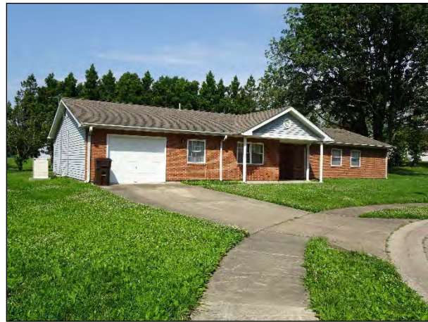
Figure 23. Facility 1483, facing southeast.
