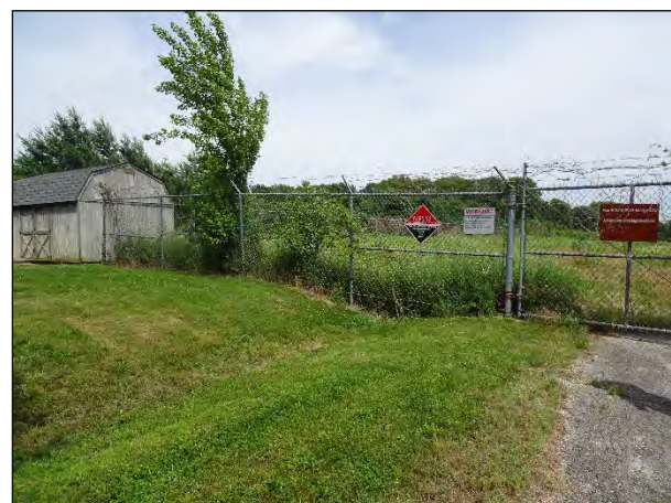
Figure 16. Facility 550, facing northeast.
