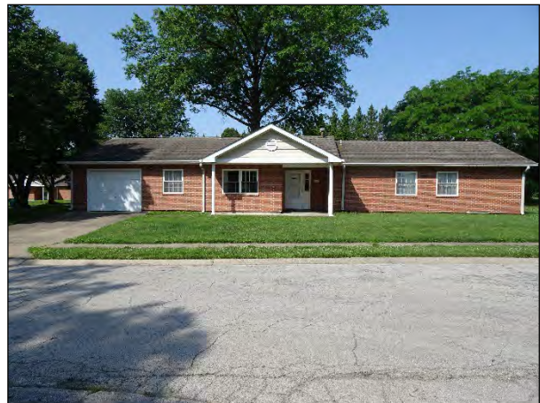
Figure 17. Facility 1471, facing southwest.
