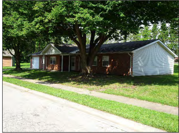
Figure 25. Facility 1487, facing southeast.
