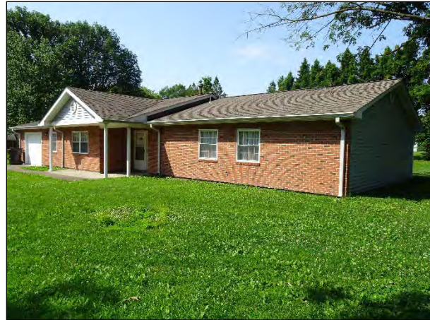
Figure 24. Facility 1485, facing south.
