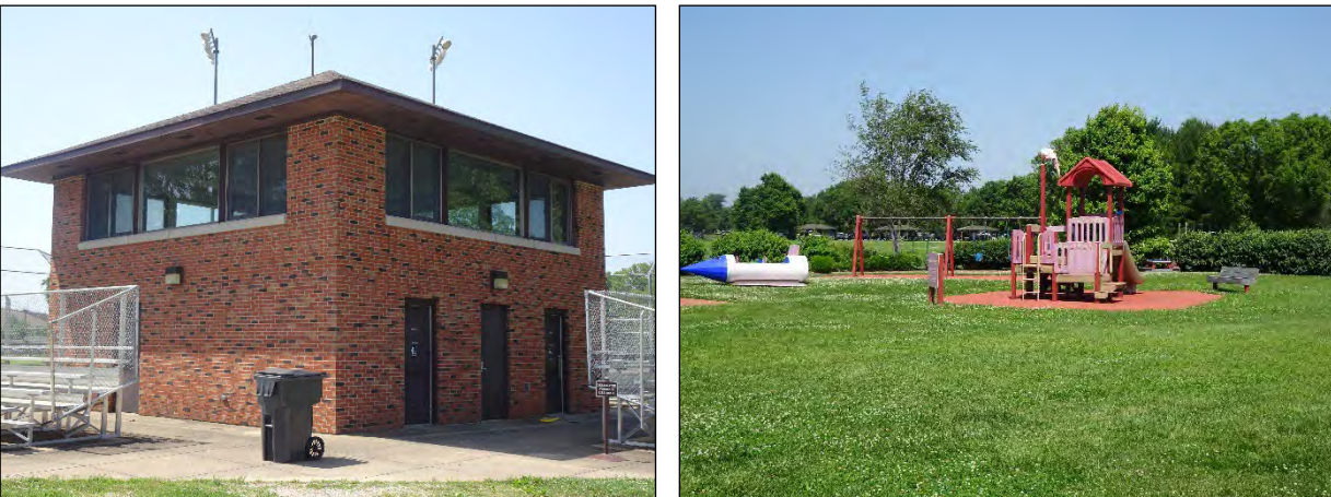
Figure 49. Facility 197 centrally located within Facility 6600, ca. 1980 observation building, facing south (left); Replacement playground equipment determined not of historic age, facing southwest (right).
