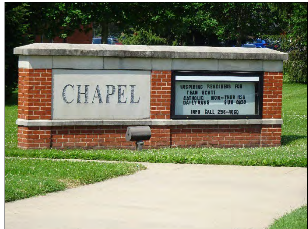
Figure 38. Facility 6002, facing west.
