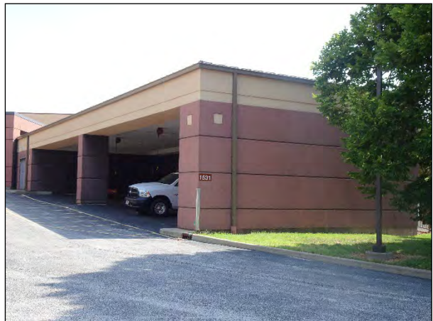
Figure 26. Facility 1531, facing northeast.
