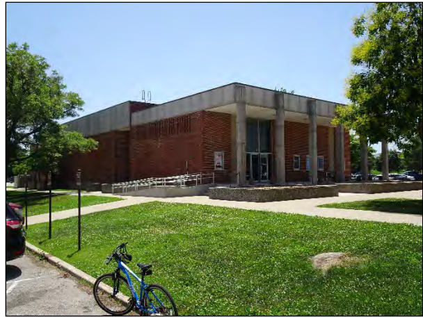
Figure 28. Facility 1670, facing southwest.
