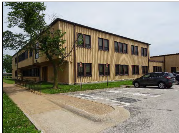
Figure 36. Facility 4001, facing southeast.
