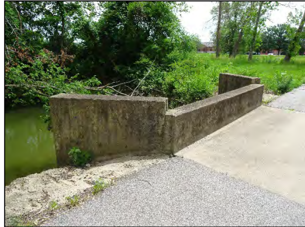
Figure 43. Facility 6009, facing southeast.
