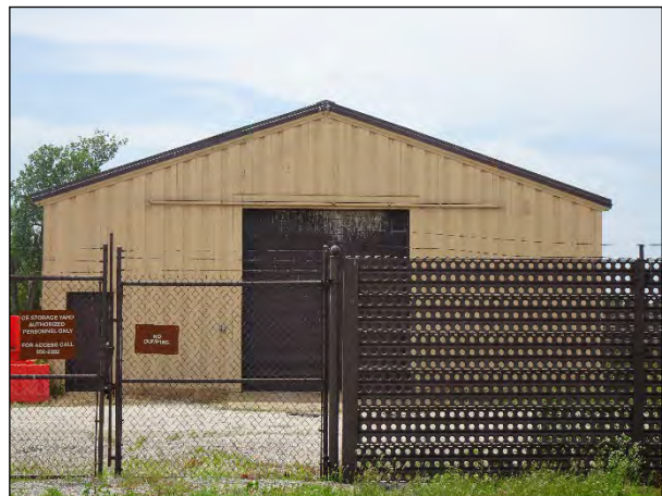
Figure 37. Facility 4130, facing south.
