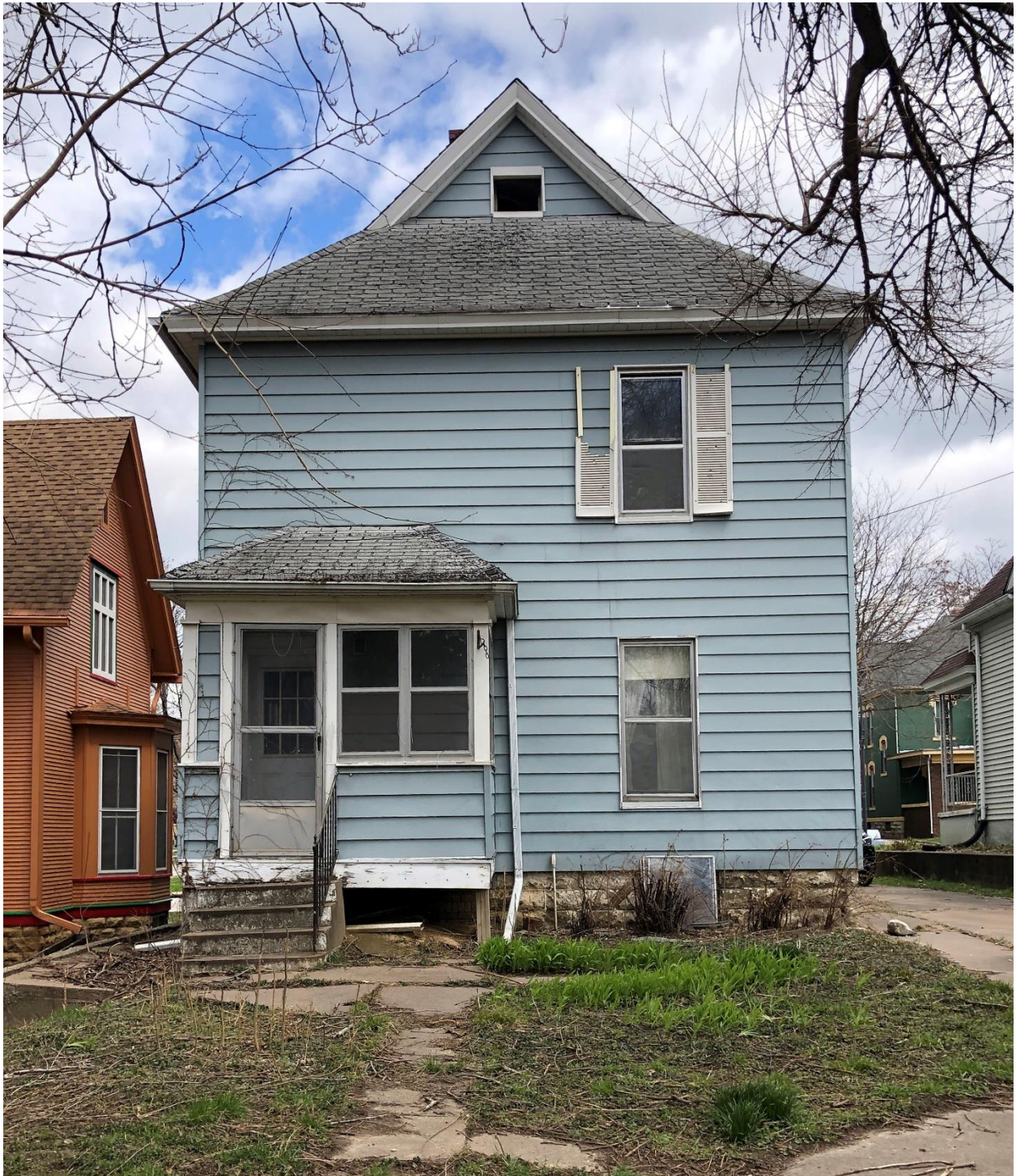
Photograph No. 4: View of the rear (west) façade of 1206 17 th Street looking east.
