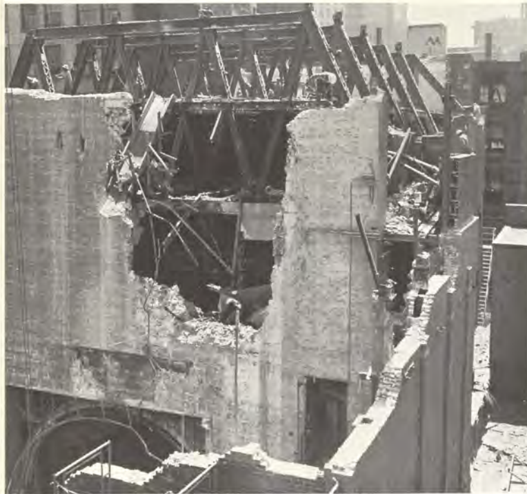
The "great trusses" as well as the sixth smaller truss can be clearly seen in this photo taken during the demolition of the Schiller.
