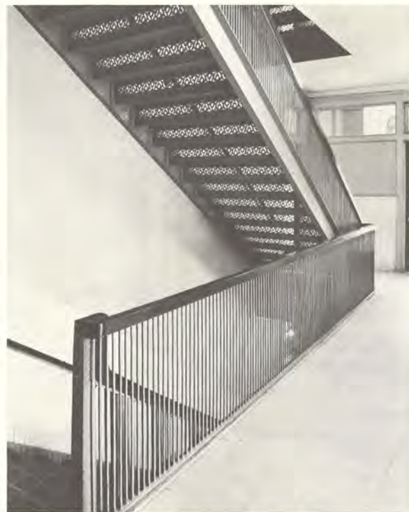
This stair and hallway in its simplicity and precision could be mistaken for the work of an architect of today. Frank Lloyd Wright's hand may be seen in the stair railing. Note the lightness and elegance achieved by the perforated ornamental insteps. The clerestory windows, above walls as well as doors, gave the interiors a natural illumination.
