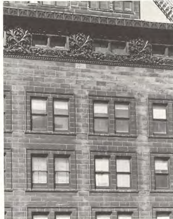
This is the east side of the Schiller showing the fourteenth floor frieze and straightforward expression of the use of the structure: an office building. Each pair of windows, with Wright's detailing, serves one office space. The surface of the side of the building was flat while the front and tower were deeply recessed. This differentiation is important for the former emphasized the setback and was expressive of the building's function while the latter made the loftiness effective.
