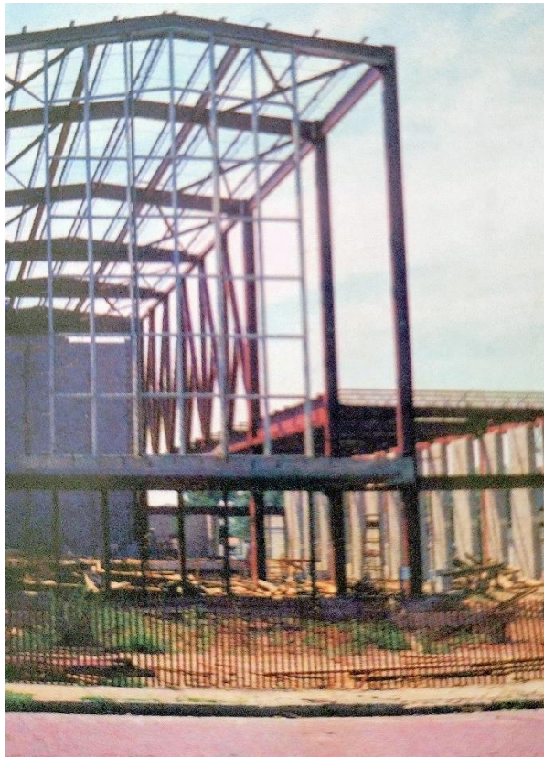
A view from Seventh Street looking through the front doors.
