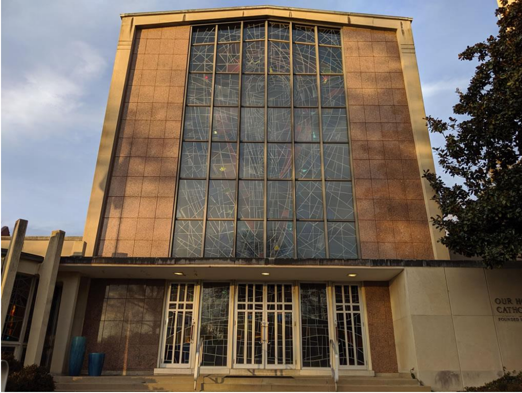
Holy Redeemer Church main entrance is nearly identical to St. Joseph Church.
