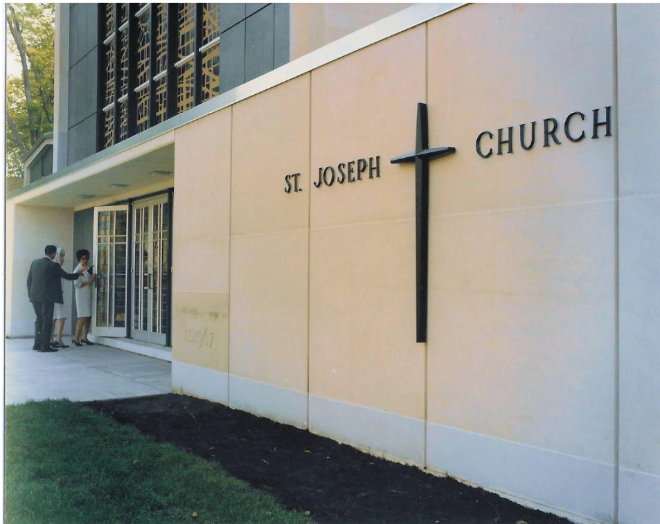
The new church and rectory were completed in 1968 with a contractual cost of $716,735. An additional $100,000 was spent on furnishings and fixtures.
