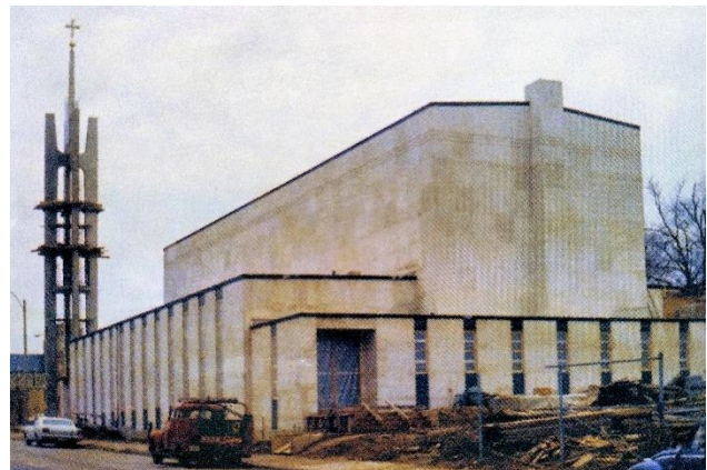
Looking southeast from Broadway Street.
