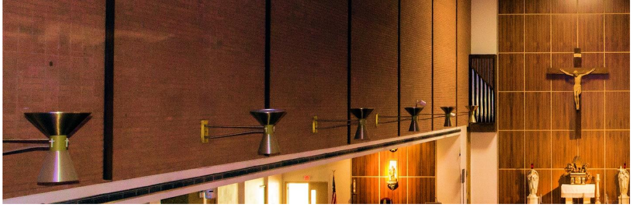
The hourglass shaped sconces on the upper brick walls of the nave are both lights (upper) and loudspeakers (lower).
