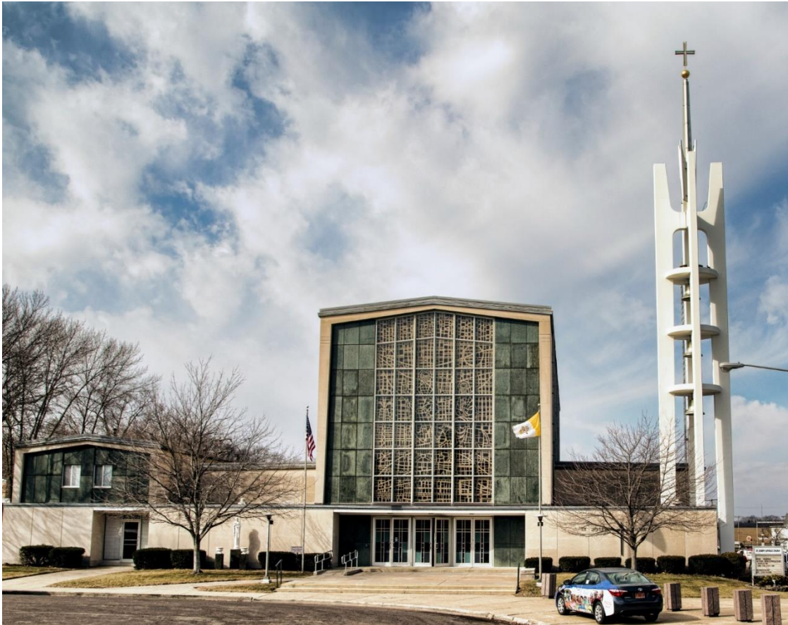
Bedford stone, brick, and concrete were blended into an imposing structure. The exterior is white Bedford stone (limestone from Southern Indiana, also known as Indiana Limestone or Salem Limestone) with polished greenstone trim from Virginia.
