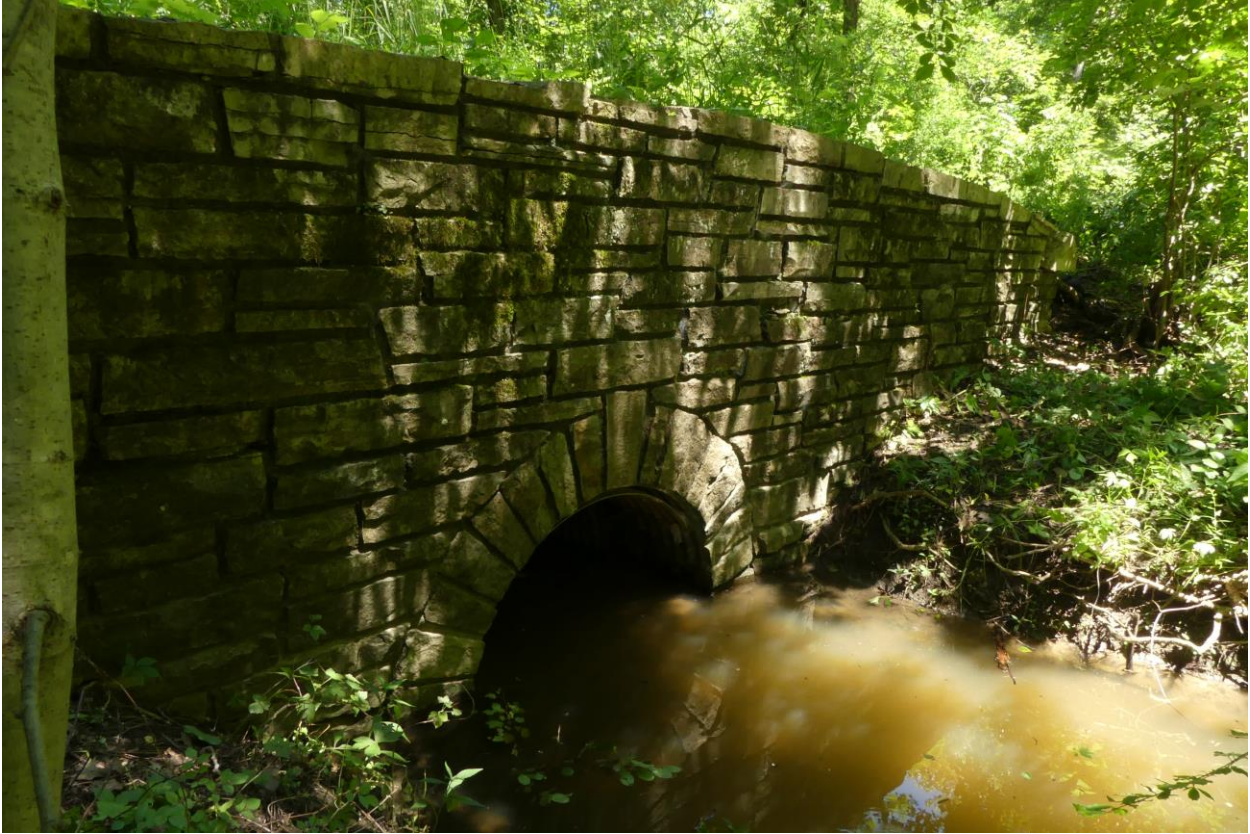
Figure 13. Coping on South elevation facing E.
