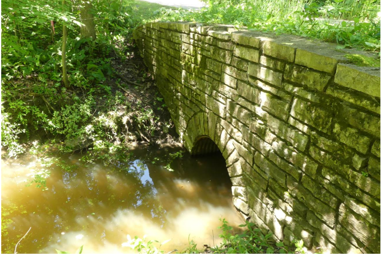
Figure 3. South elevation West half facing NW.
