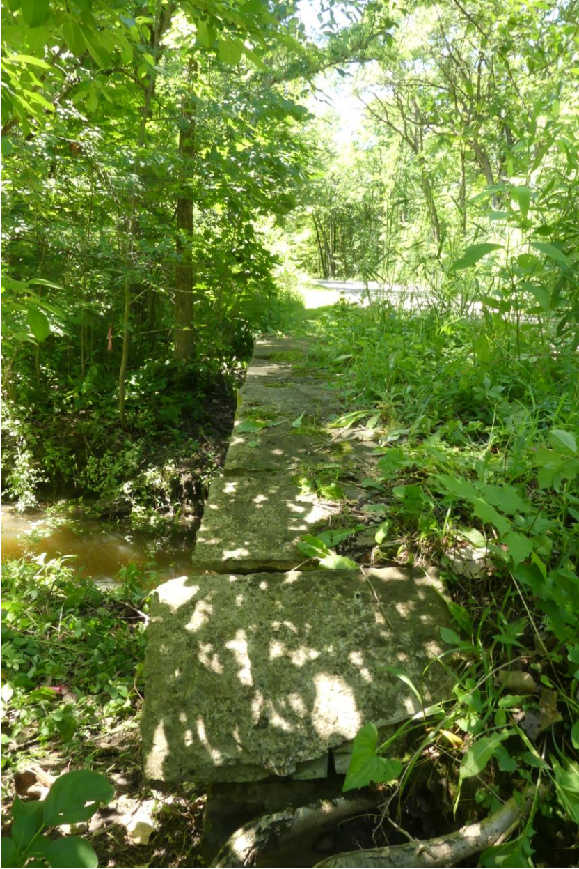
Figure 6. Coping on South elevation facing W.
