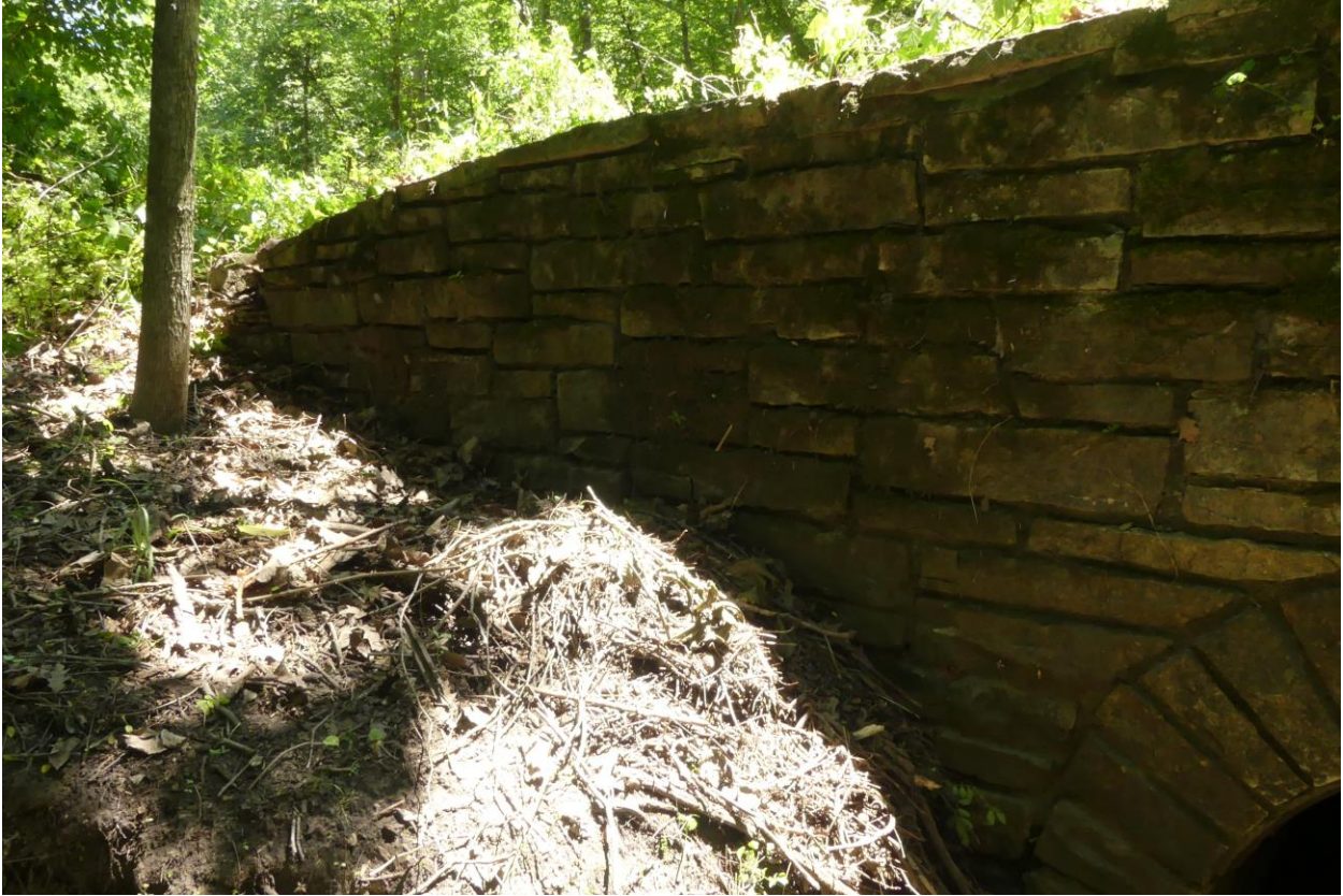
Figure 16. North elevation East half facing SE.
