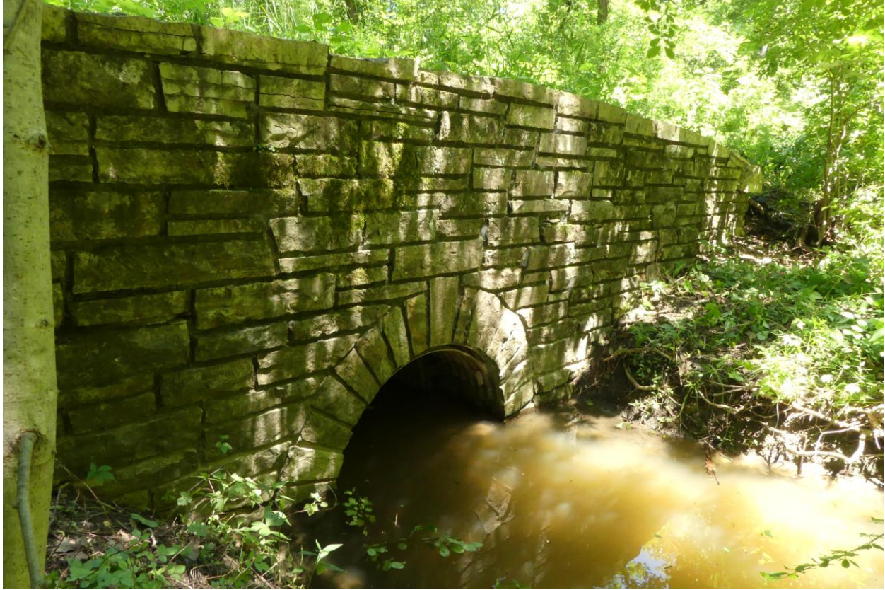
Figure 12. South elevation East half facing NE.
