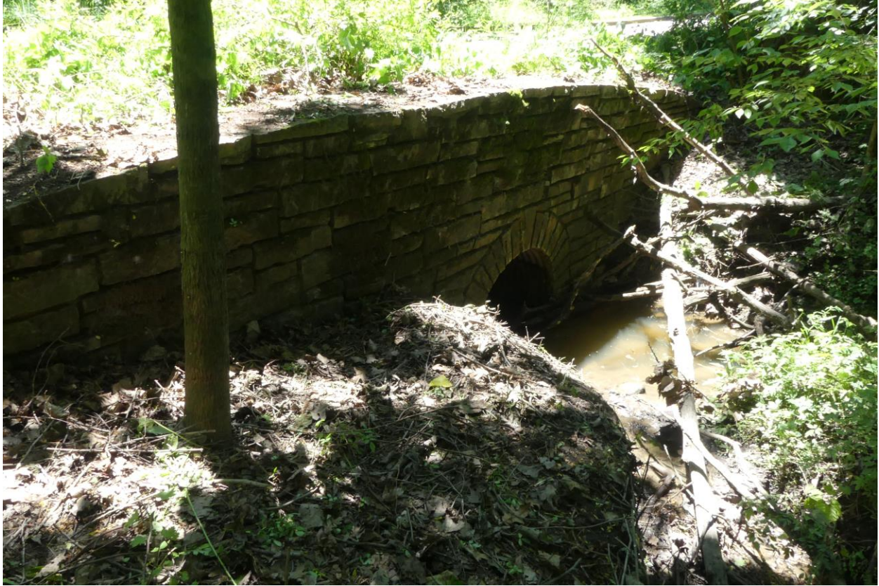
Figure 23. North elevation overview facing SW.
