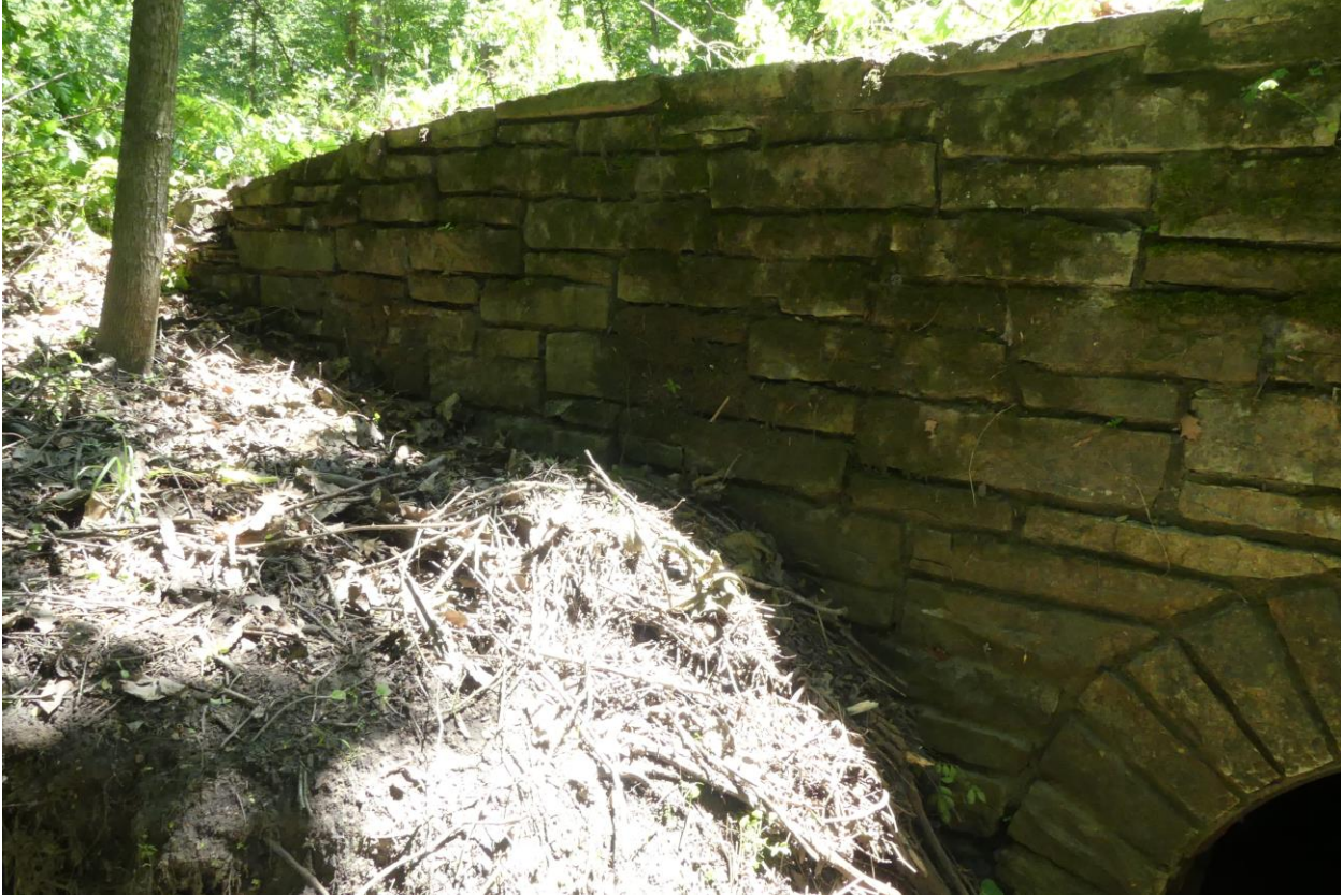
Figure 17. North elevation East half facing SE.
