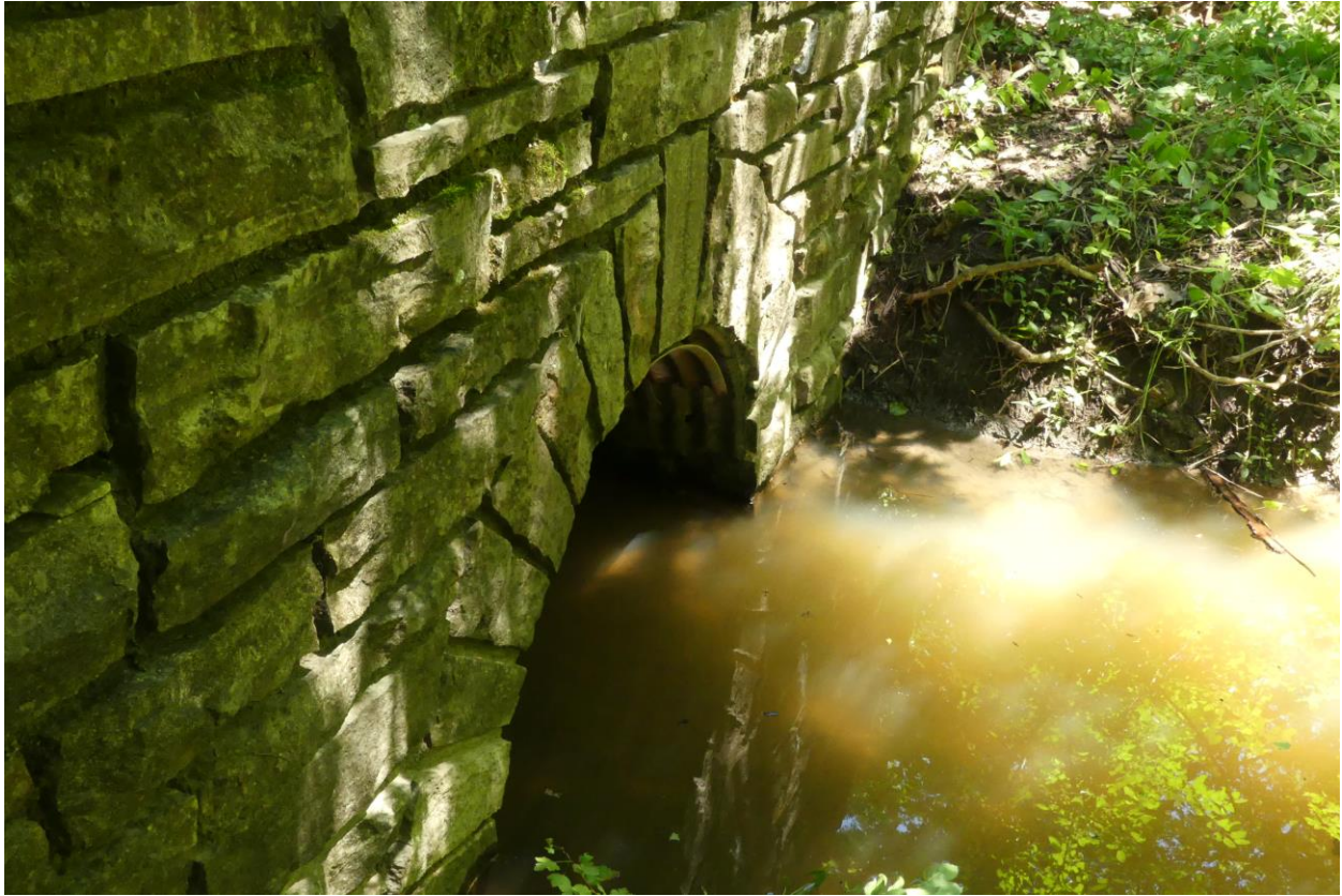
Figure 11. South culvert detail facing NE.
