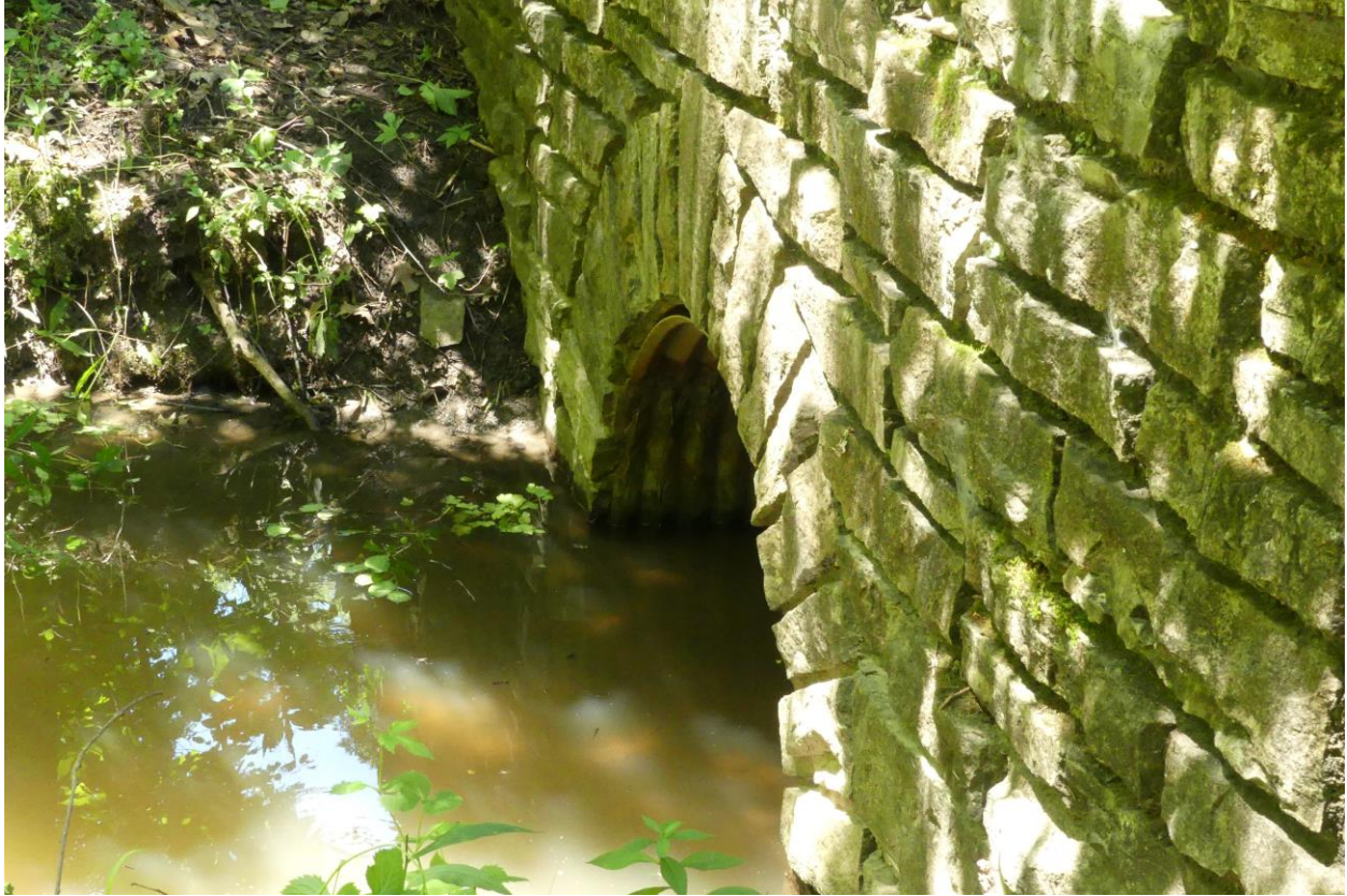
Figure 5. South culvert detail facing NW.
