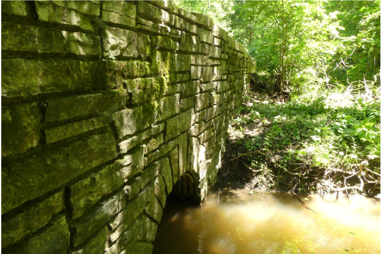
Figure 10. South elevation detail facing NE.
