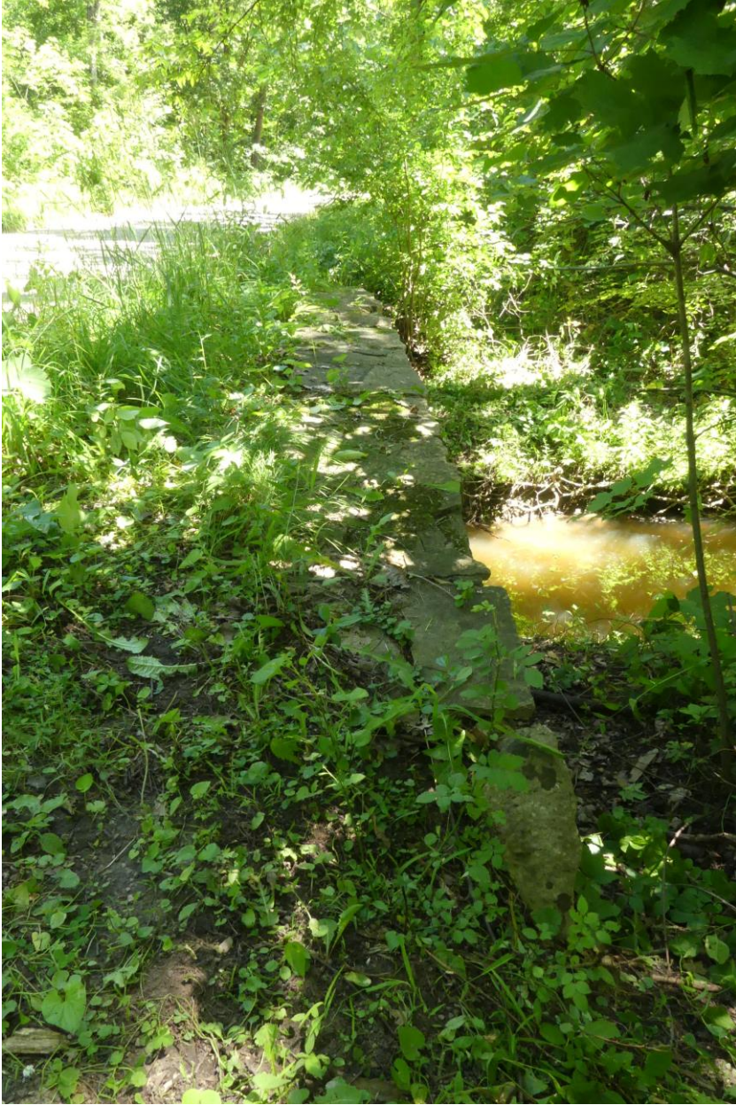
Figure 9. Coping on South elevation facing E.
