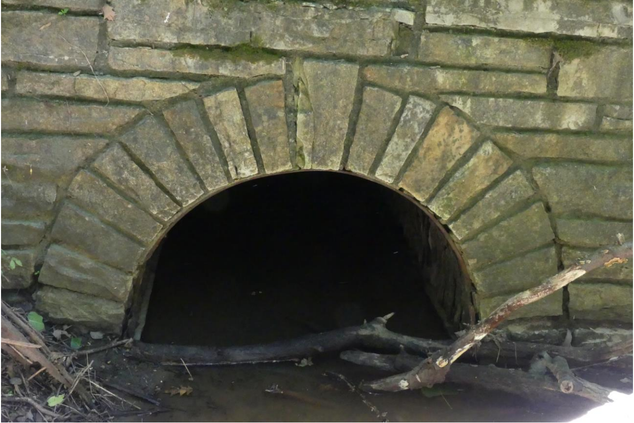
Figure 20. North culvert detail facing S.
