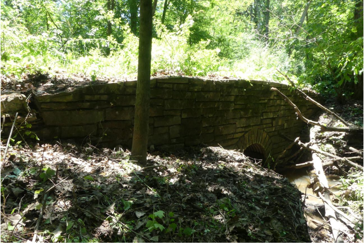
Figure 26. North elevation overview with tree facing SW.
