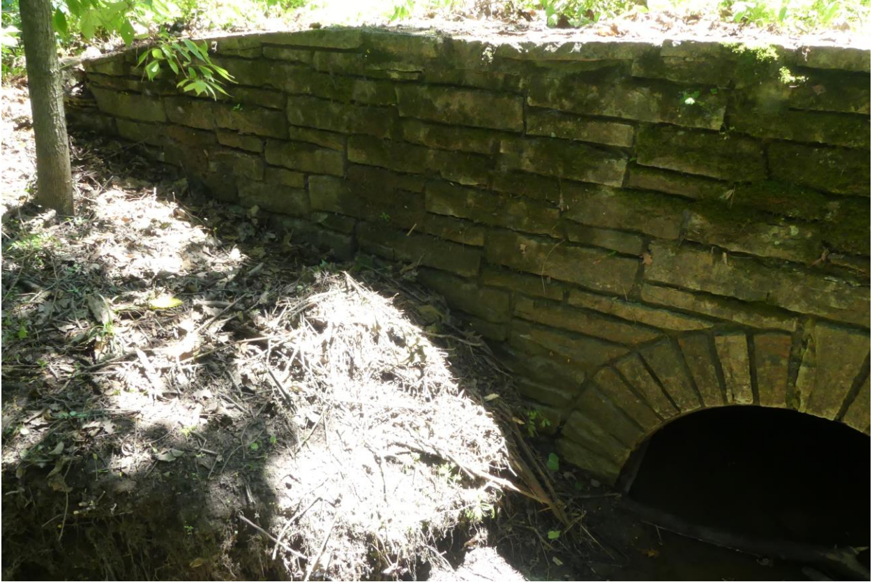
Figure 22. North elevation East half facing SE.
