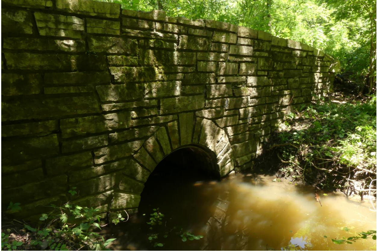
Figure 14. South elevation East half facing NE.
