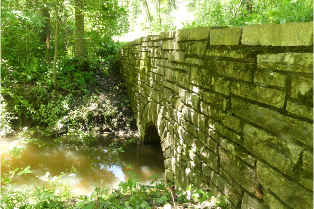
Figure 2. South elevation West half facing NNW.
