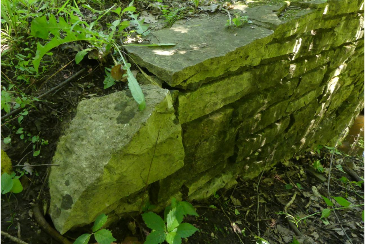
Figure 15. South elevation with coping detail facing NNE.
