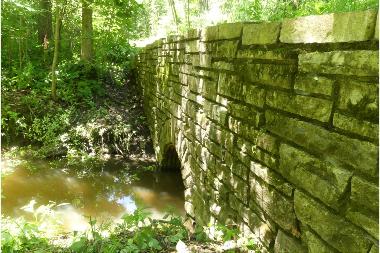
Figure 4. South elevation West half facing NNW.
