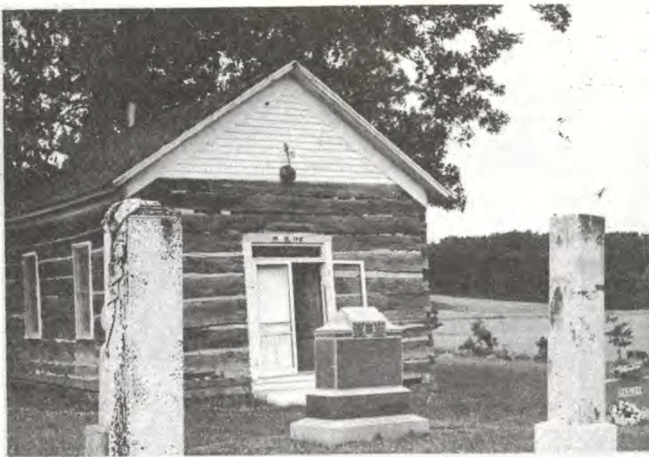
MT. OLIVE CHURCH in southeastern Webber Township is said to be the oldest existing church building in Jefferson County, having been built in 1840.
