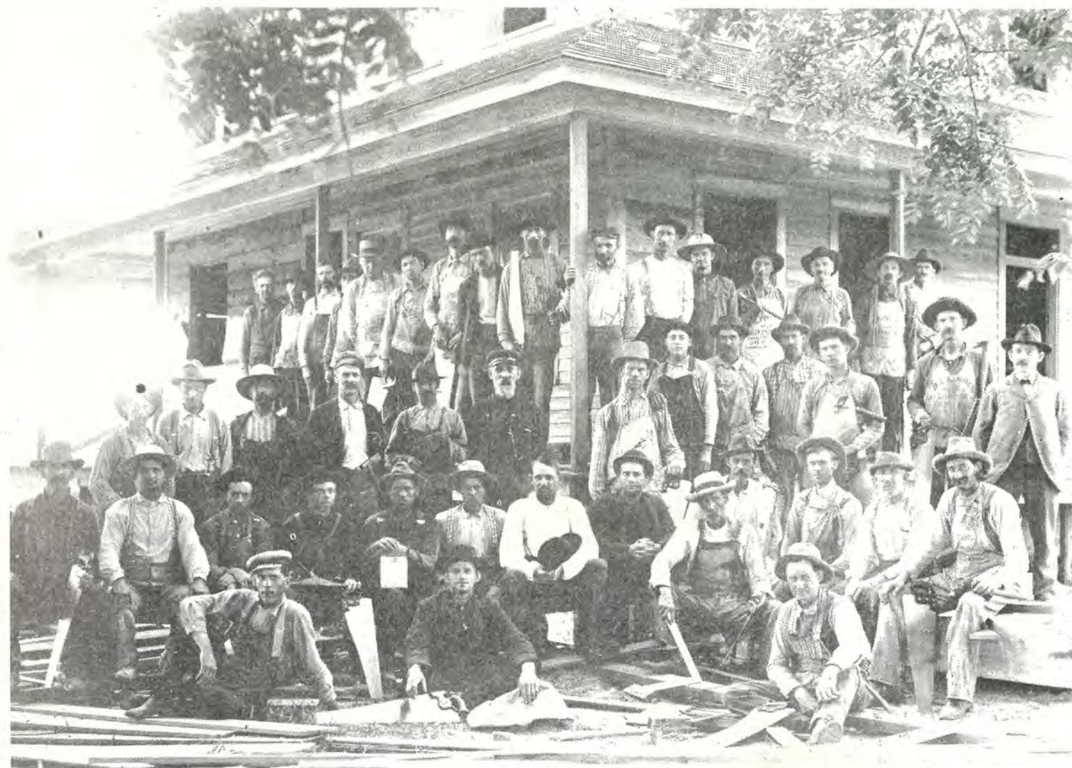
WORKMEN PAUSE for the photographer while building a "hotel", or boarding house, for men who were to work at the Little Muddy Coal Company's mine at the north edge of Tamaroa, early in this century. Photo courtesy Logan Taylor, Tamaroa.
