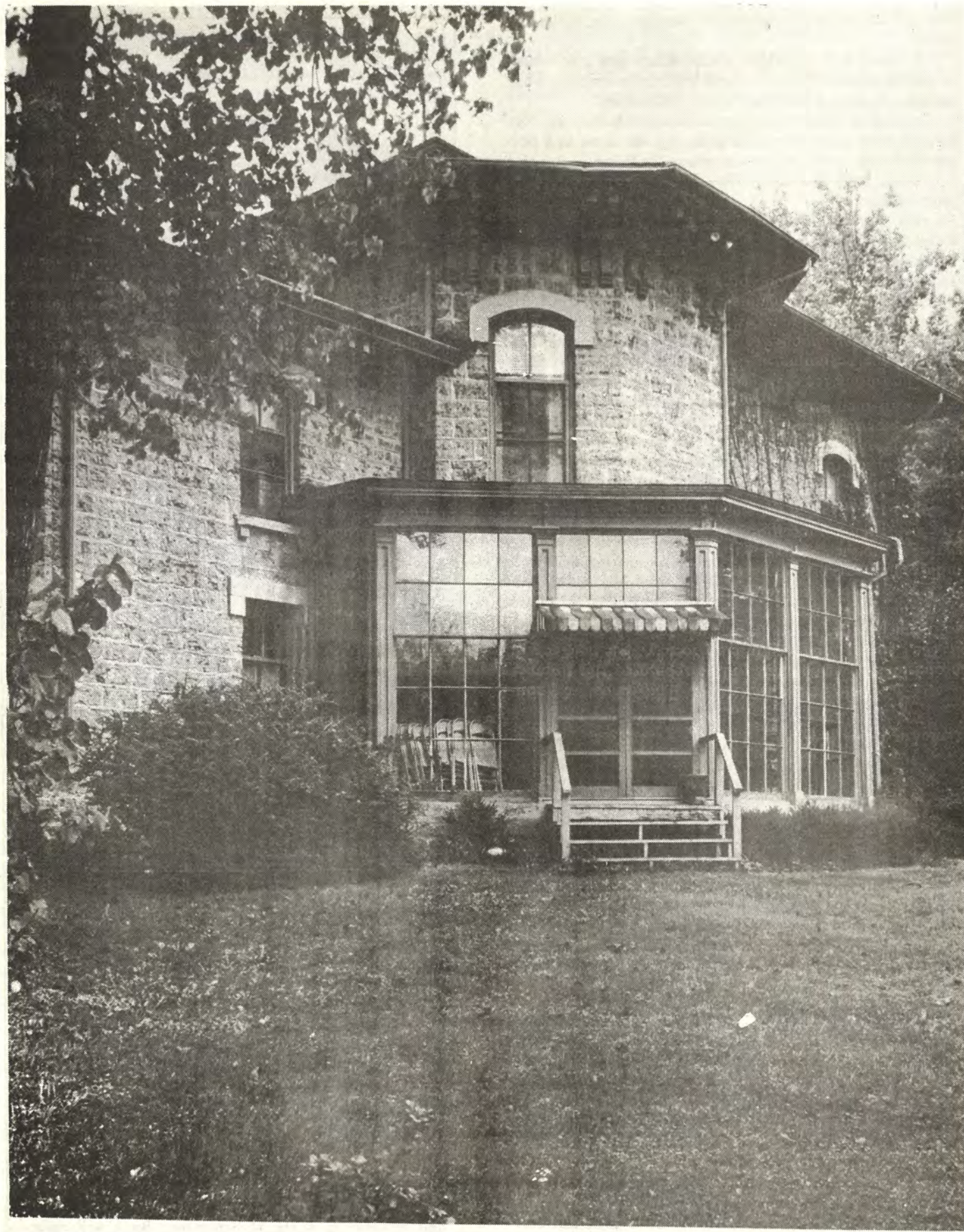
POLYGONAL BAY WITH projecting sun porch on south side of Taylor Mansion has door awning obviously out of place with the original design, as are plain steps leading to back yard.
