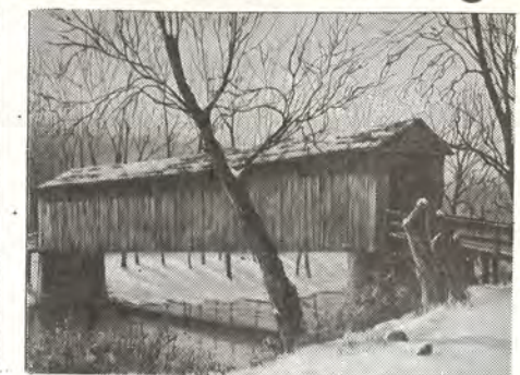
Thompson Covered Bridge
