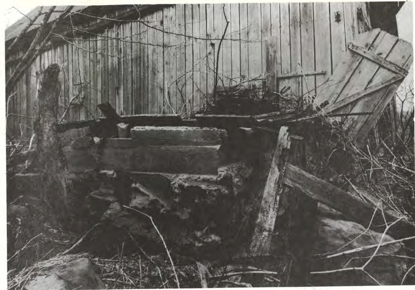
REMAINS OF a concrete fermentation vat located a few miles southwest of Herod in Pope County. At one time the barn extended over it. Inside measurement: 10' by 6½' by 3½'. This curiosity is on private land.
