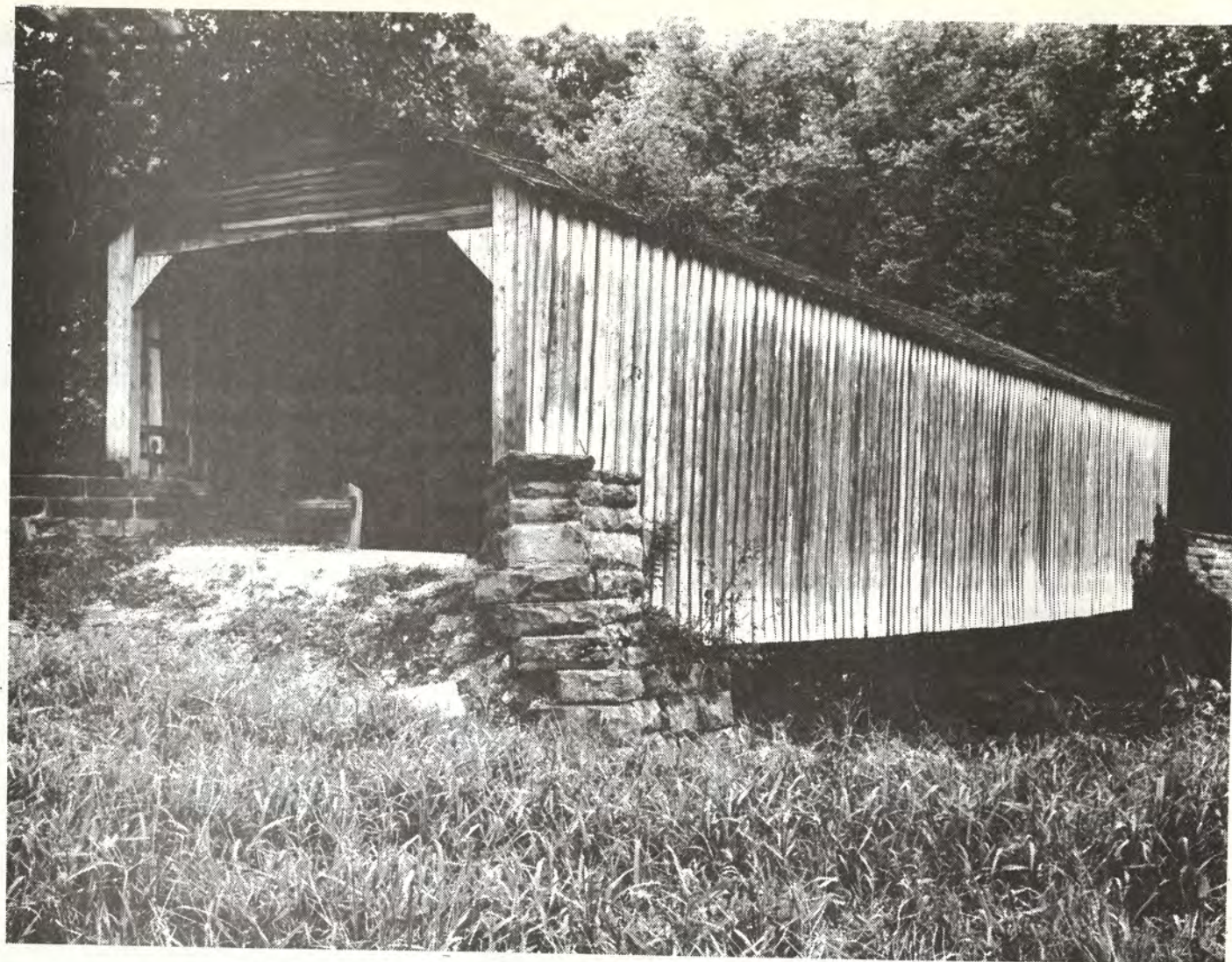
COVERED BRIDGE over the Little Mary's branch of the Mary's River, about five miles northeast of Chester on State 150, is possibly the oldest covered bridge in the state. It dates from 1854. View is looking south toward parking lot.
