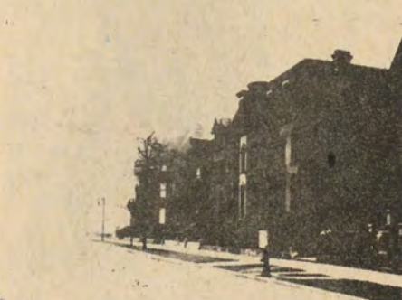
PRAIRIE AVENUE HISTORIC DISTRICT — Chicago—Cook County. This District comprises what remains of the once famous south Prairie Avenue Mansions. The photo, ca. 1900, gives a glimpse of the street's lost grandeur. (Photo—Illinois Historic Sites Survey)
