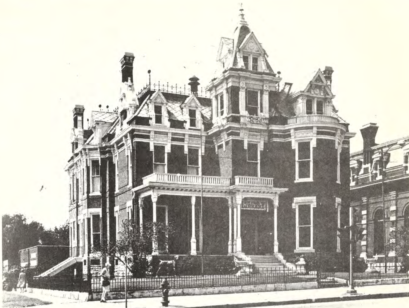
THE CLOUD MANSION, now the McCoy Memorial Library, is one of two distinctive 19th Century structures on the courthouse square in Hamilton County seat McLeansboro. View is of east front, looking northwest.
