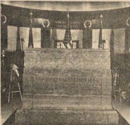
LINCOLN TOMB — Springfield — Sangamon County. The tomb's exterior design consists of a shaft 117 feet high which rests on a simple square building. It was dedicated in 1874. (Photo — Department of Conservation)
