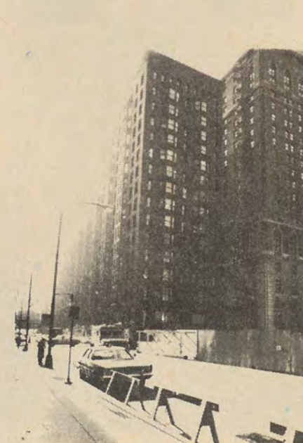
MONADNOCK BUILDING — Chicago — Cook County. This massive brick structure is the highest wall-bearing building in Chicago. It was designed in 1891 by the architects Burnham and Root. (Photo—Tom Yanul)
