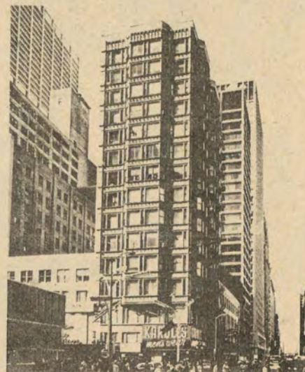
RELIANCE BUILDING — Chicago — Cook County. This building, designed by Charles Atwood, survived the disastrous Chicago fire of 1871. It is a refined and perfected version of the Tacoma Building, which was demolished in 1929. (Photo — Richard Nickel)
