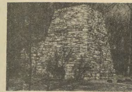
ILLINOIS IRON FURNACE — Near Rosiclare — Hardin County was added to the Register on March 7, 1973. The Furnace was originally built in 1837 and reconstructed in 1967 by the Golconda Job Corps. Iron was mined in the area and processed into "pigs" which were then hauled by wagon to the nearby Ohio River for shipment to market. The Furnace ceased operation for good in 1883. (Photo—Tom Yahraes)
