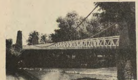
GENERAL DEAN SUSPENSION BRIDGE — Carlyle — Clinton County was added to the National Register on April 6, 1973. The bridge was built in 1859 and is believed to be the oldest and only bridge of its kind in Illinois. This unique bridge spans the Kaskaskia River and is located just below the Carlyle Dam. (Photo—Outdoor Illinois Magazine)
