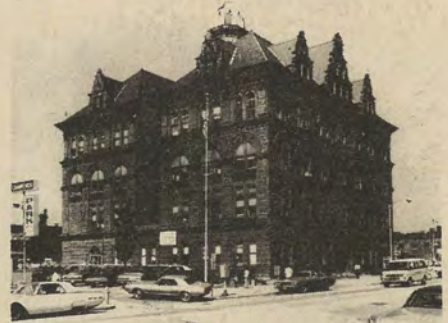
PEORIA CITY HALL — Peoria — Peoria County was accorded Register status on February 6, 1973. The City Hall was designed by Reeves and Baille and was built in 1892. Many of the fine features used in this building were later refined and used in the McLean County Courthouse. The building is Flemish Renaissance in style and is one of the last of Peoria's downtown Victorian era structures. (Photo—Leslie Kenyon)
