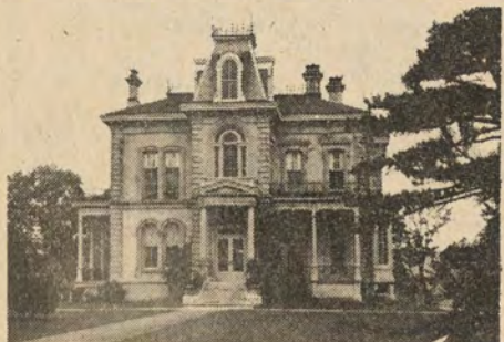
DAVID DAVIS MANSION — Bloomington — McLean County. Alfred H. Piquenard designed this house in 1872 for Supreme Court Justice David Davis. (Photo — Bill Farrar)
