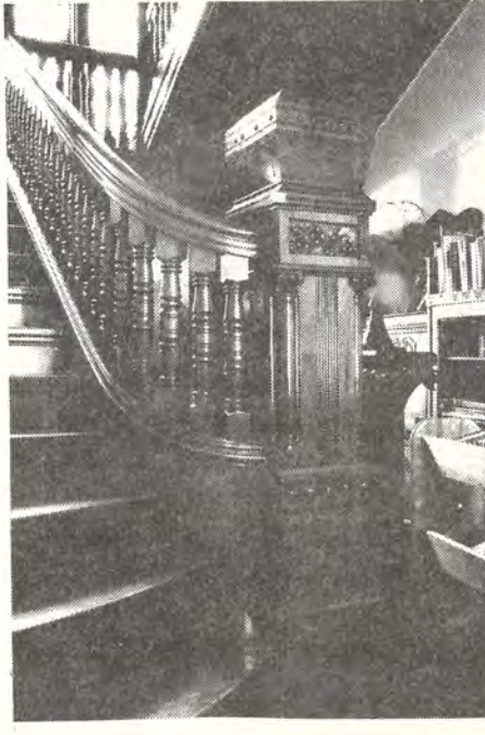
DETAIL OF newel post in hall, and balusters, shows exceptional detailing.
