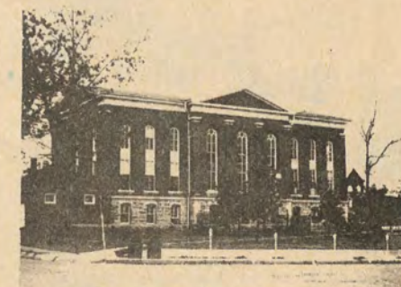
CARROLL COUNTY COURTHOUSE — Mt. Carroll — Carroll County was added to the National Register on November 26, 1973. The courthouse was built in 1858. Its cathedral style windows are one of its finest points. (Photo—Ted Hild)
