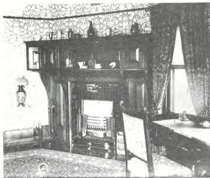
GUEST BEDROOM in northeast corner of house, looking northwest. Morris fabrics and wallpaper are clearly visible. About 1890.
