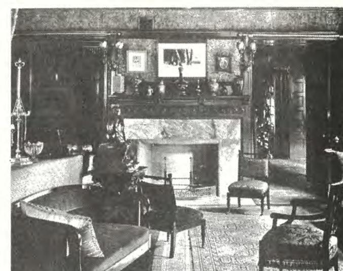
PARLOR , looking east about 1920. Marble fireplace is surmounted by beautifully-carved woodwork.
