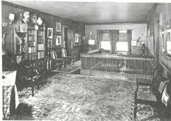
SECOND FLOOR hall, looking north. Bookcase on left was made by Isaac Scott in 1876. Photo about 1920.
