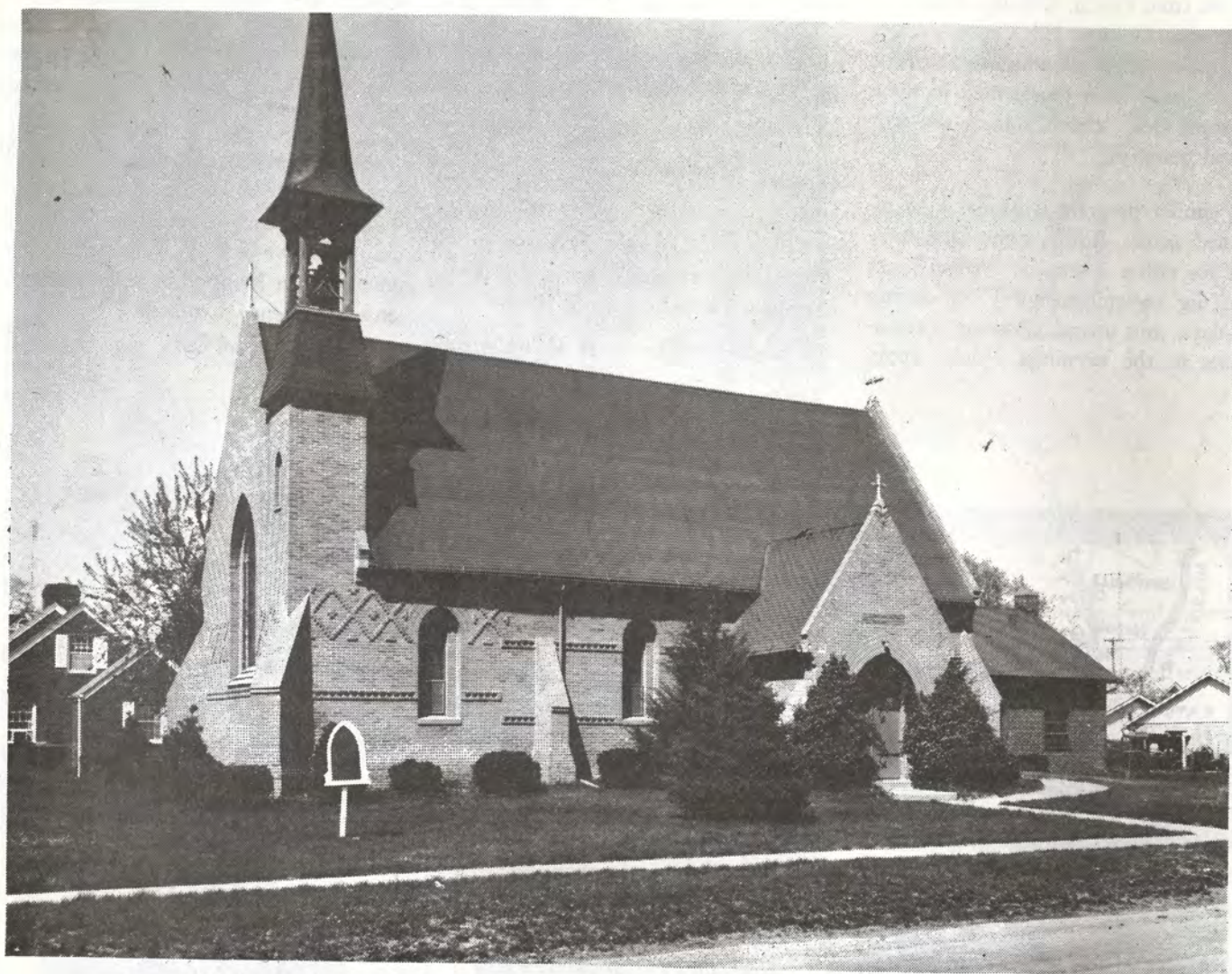
THE FLYING BUTTRESSES and open belfry are but two of the features on the classic Gothic church constructed in Lewistown a century ago. It was patterned after English country parish churches used by the Anglican faith.
