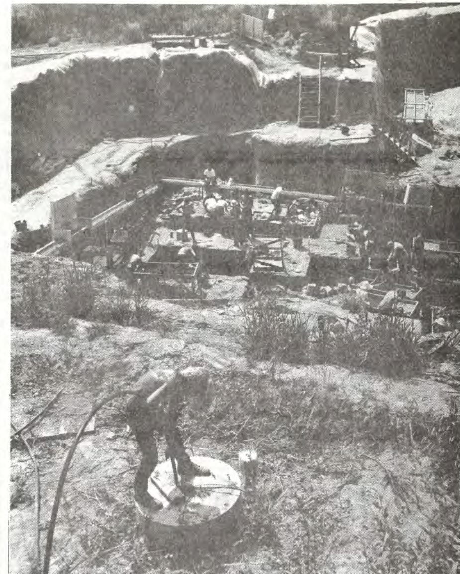
ONE OF SIX wells dug around perimeter of the Koster site (foreground) helps lower the water table below lower horizons. Worker adjusts well line as excavators work in the background. D. R. Baston photo.
