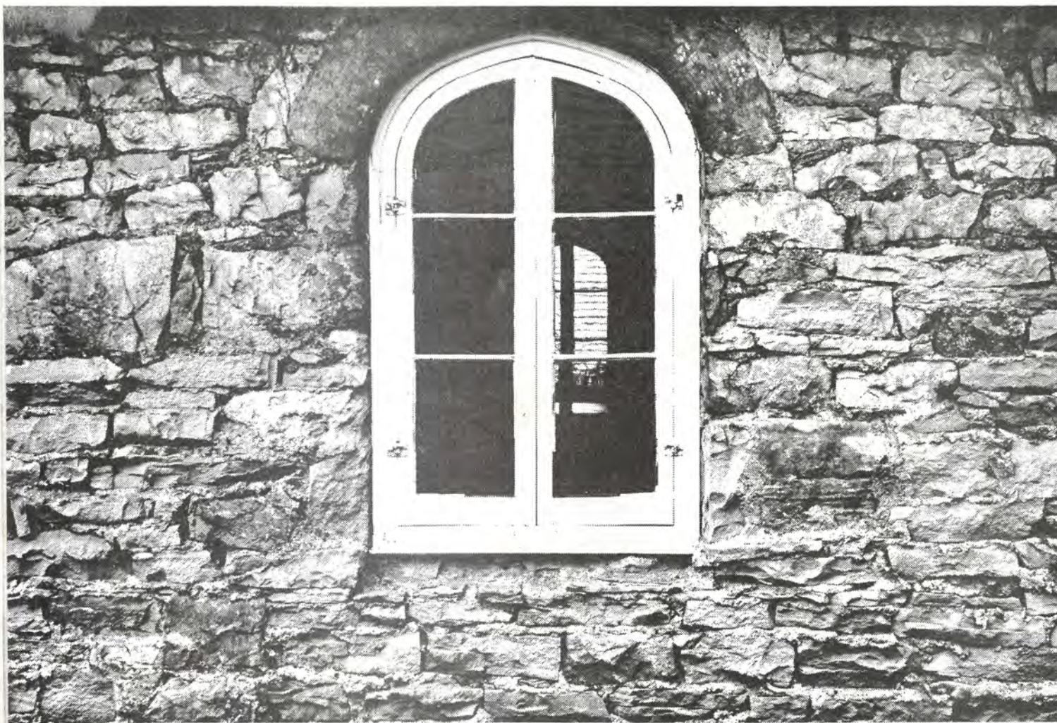
NORTH WALL shows detail of fieldstone construction. Anna, in Union County, has long been noted for quarries and early pottery works.
