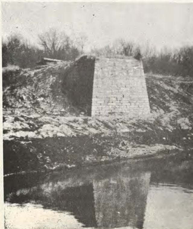
A TOLL BRIDGE across the Saline River near Equality, built early in the Nineteenth Century by William Hicks, used this stone abutment built by stone masons imported from Philadelphia.
