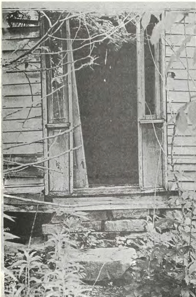
DOORWAY OF long-abandoned Burns House, on the Goshen Road in northwestern Hamilton County near site of the Riddle Tavern. Note sandstone foundation and steps.
