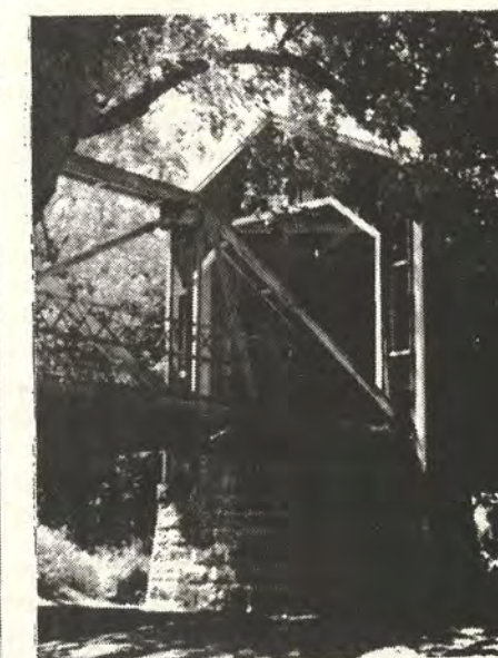
WOLF COVERED BRIDGE
