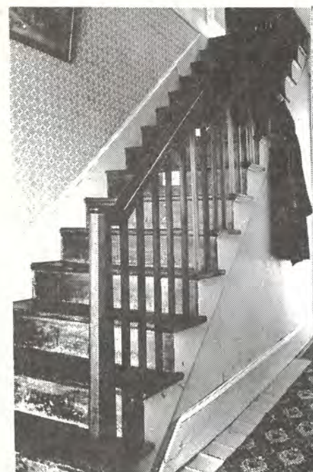
STAIRWAY TO second floor of the Mack House faces the front entrance. Stair hall leads to dining room.
