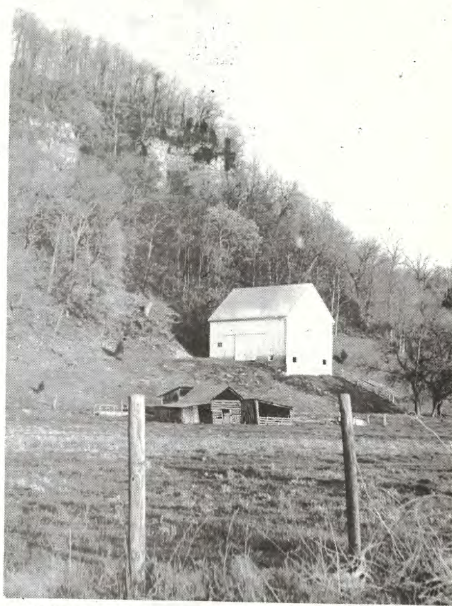
THE NEW supersedes the old on the east side of the ridge of hills that run the length of Calhoun County. Note the log barn in front of newer barn.
