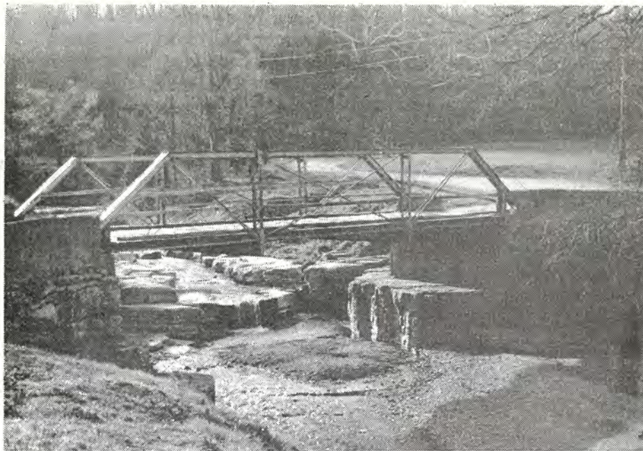
AN OLD IRON bridge at the south edge of Hamburg crosses a rock-bound stream common to the Calhoun ridge country. The bridge will be replaced soon.
