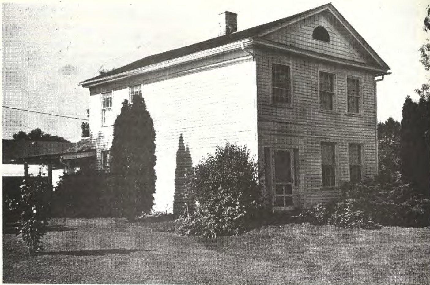
STEPHEN MACK'S HOUSE, built in 1839 overlooking the Rock River in the now-vanished community of Macktown, reflects the Greek Revival style which was prevalent in his native Vermont.
