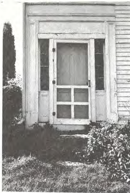
FRONT DOOR of the Mack House and the manner of framing the entrance indicate the structure's Greek Revival antecedents.
