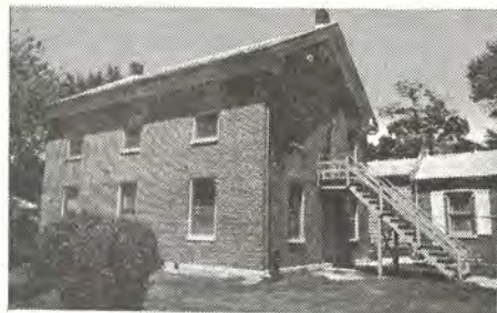
CALHOUN COUNTY Court House at Hardin was erected in 1848 at a cost of $1199. Photo courtesy Ralph J. Moses.
