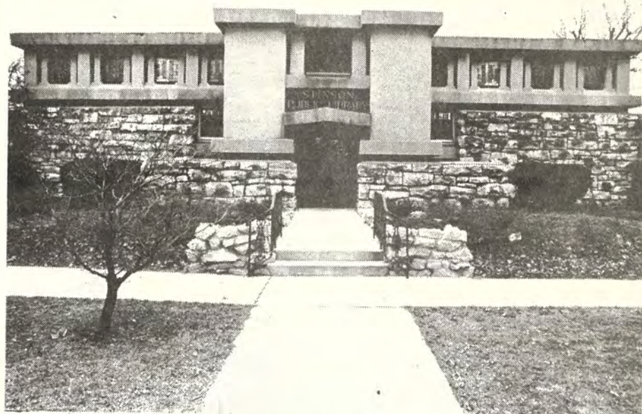
STINSON PUBLIC LIBRARY, designed by world-famous architect Walter Burley Griffin in a style which was far ahead of its time 60 years ago.
