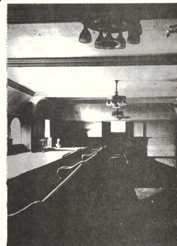
GALLERY of court room, looking east. Benches are original, partition is not.
