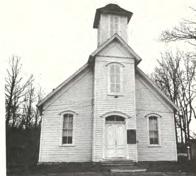
ST. JOHN'S Church, established in 1816 between Dongola and Mill Creek, was the first Lutheran Church established in Illinois.
