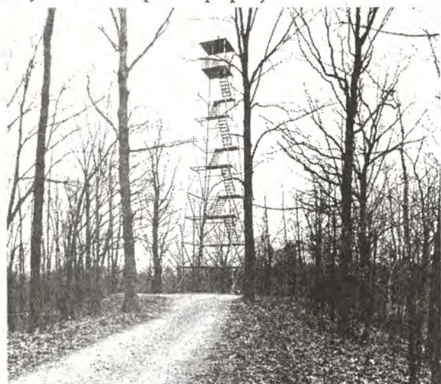
FIRE LOOKOUT TOWER, one of few remaining from era forest fires were spotted in this manner, stands in Trail of Tears State Forest.
