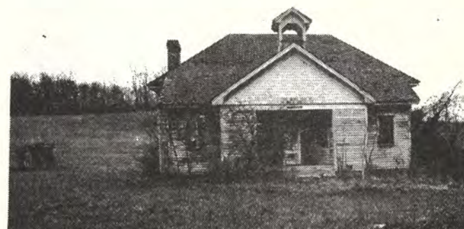
AS IN MANY other Illinois counties, abandoned schools mark the passing of a simpler though not necessarily inferior school system.
