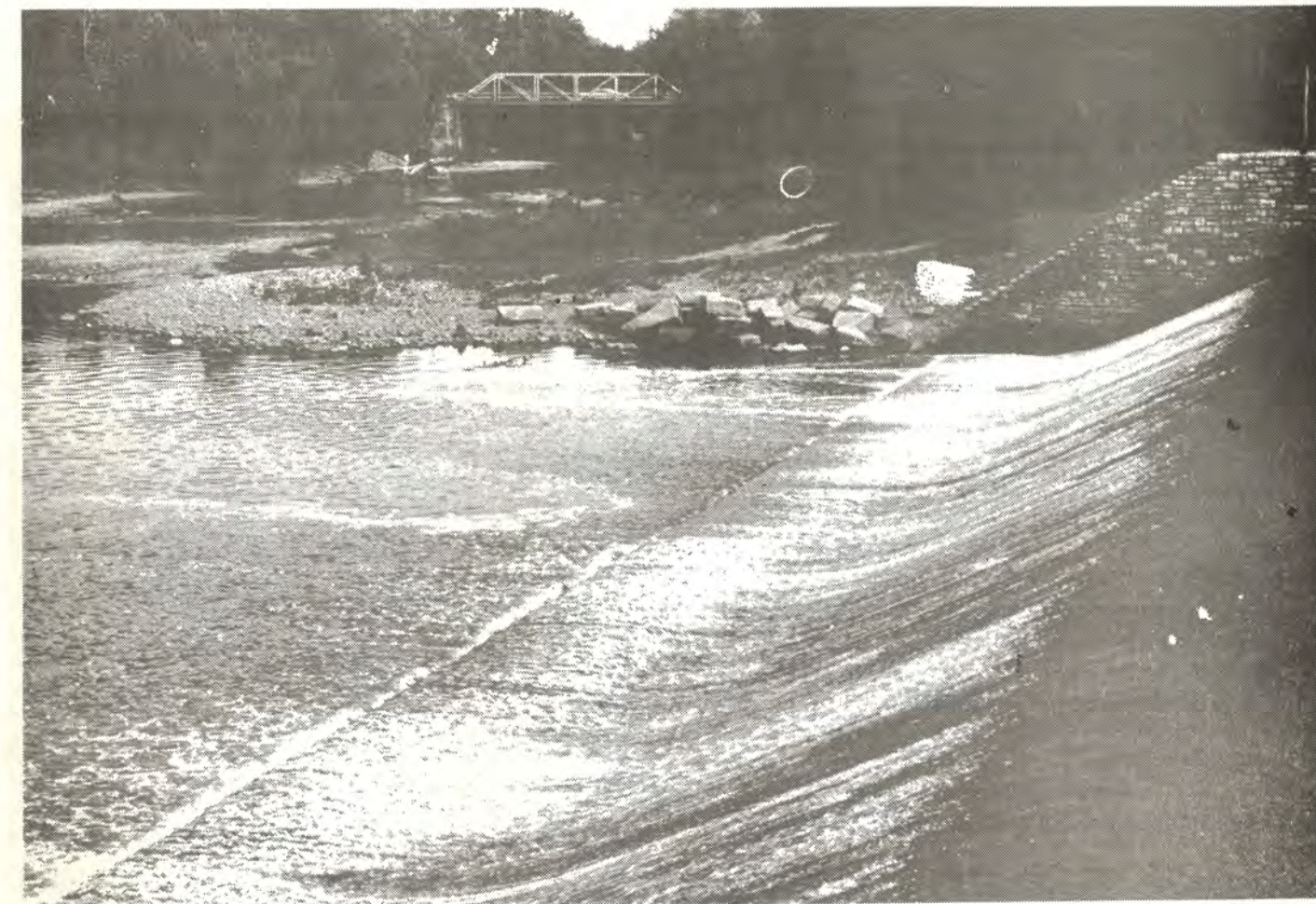
SPILLWAY AND DAM on DuPage River in Channahon Parkway, with bridge in the background.
