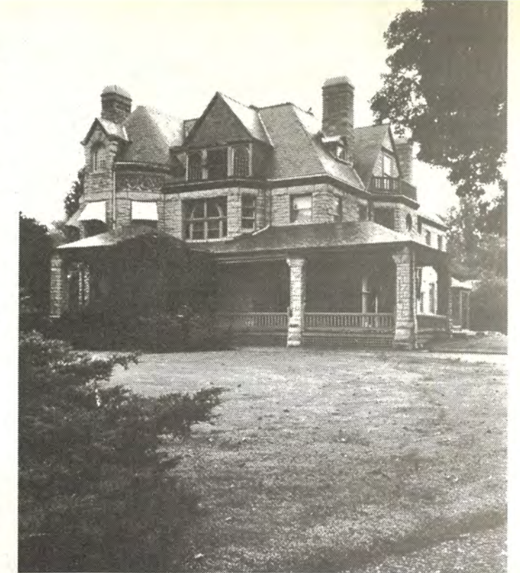
WEST FRONT, looking east, with porte cochere at left.
