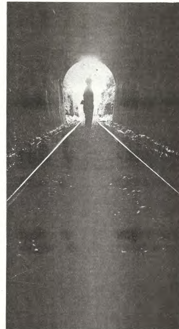
INTERIOR OF Penn Central tunnel at Tunnel Hill.
