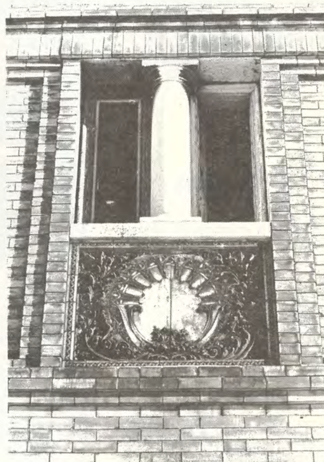
ORNAMENT DETAIL from Francisco Street front derives from Adler and Sullivan's Guaranty Building at Buffalo.
