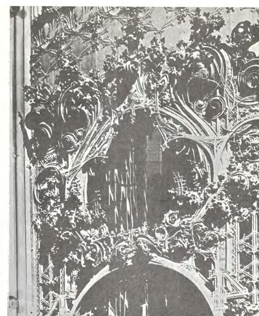
DETAIL OF ornate Sullivan metalwork in the Carson, Pirie Scott building, still standing on State Street. Photo by the late Richard Nickel, courtesy Illinois Historic Sites Survey.
