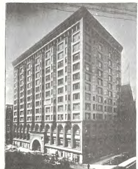
CHICAGO STOCK EXCHANGE building was demolished in 1972.
