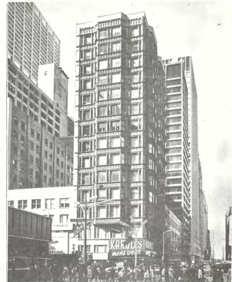
RELIANCE BUILDING, photographed by Richard Nickel for Commission on Chicago Historical and Architectural Landmarks.
