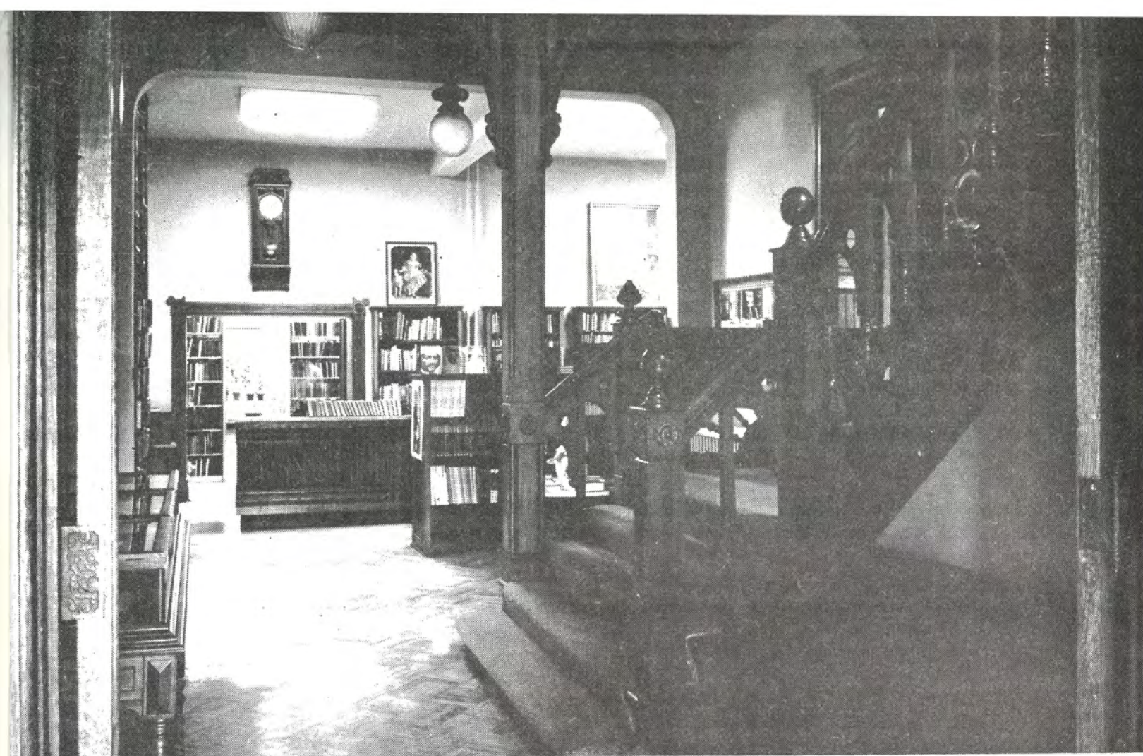
HALL, looking toward later addition from front door. Original polygonic termination ended near arch in back-ground.
