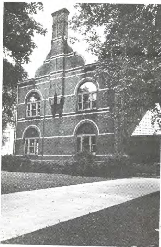
NORTHWEST SIDE , showing addition at rear, looking east toward Washington Avenue.
