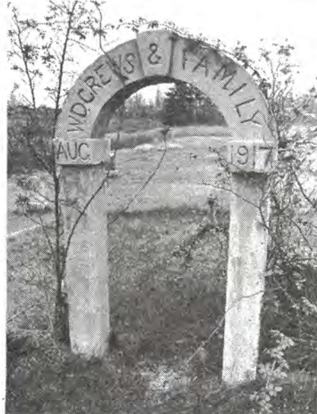
STONE ARCH leads into family cemetery plot of W. D. Crews. Erected in 1917.
