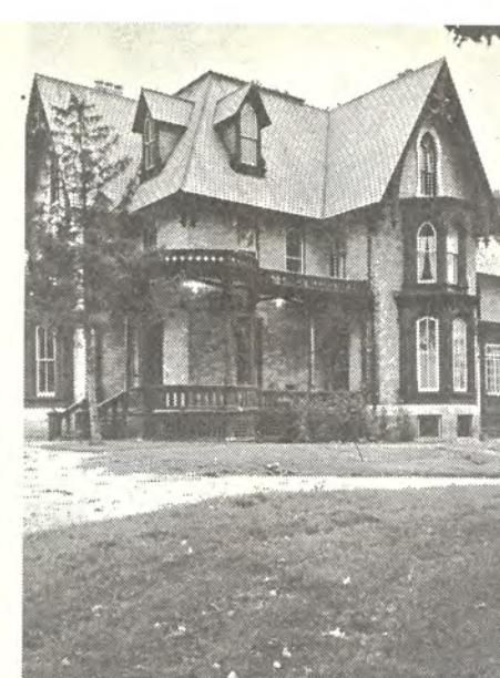
SIDE, looking east
