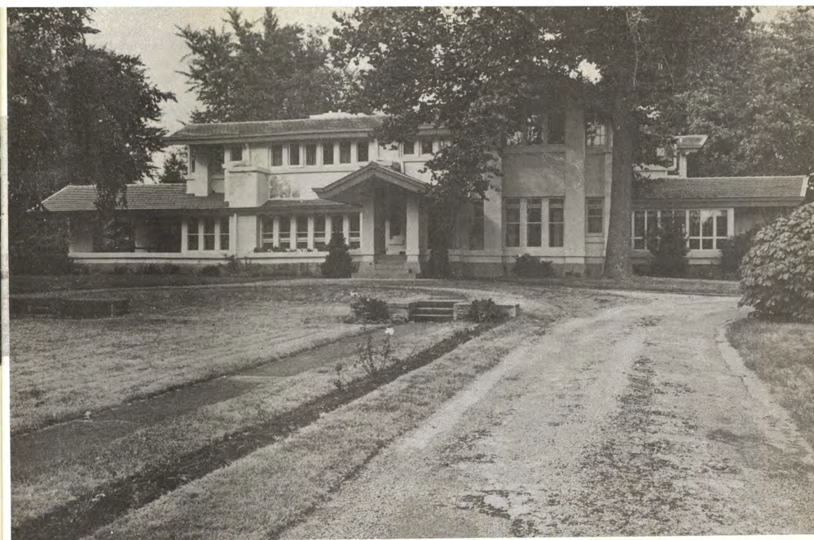
ADOLPH MUELLER HOUSE, on Millikin Place in Decatur, is one of three classic prairie-style residences influenced by the master architect of his time, Frank Lloyd Wright. View is from the front, looking north.
