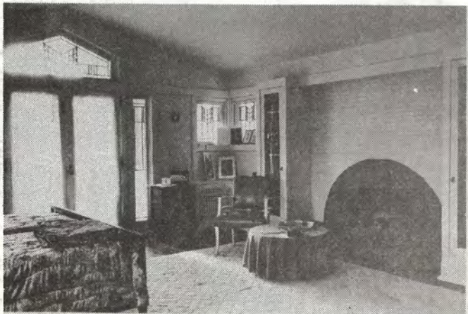
MASTER BEDROOM, above living room, looking northwest. Sleeping porch is through doors on left.
