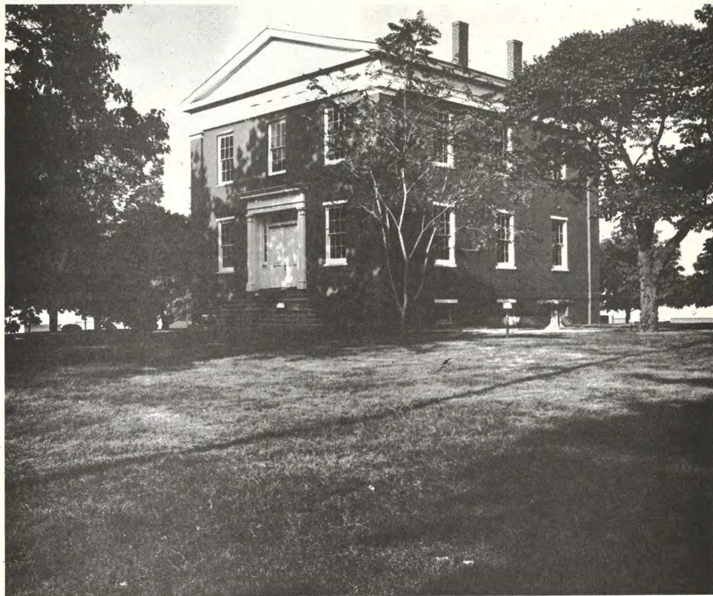
ERECTED IN 1848 as the Logan County Court House in Mt. Pulaski, this small Grecian temple shows the adaptability of its elegance and grace to a small government building.
