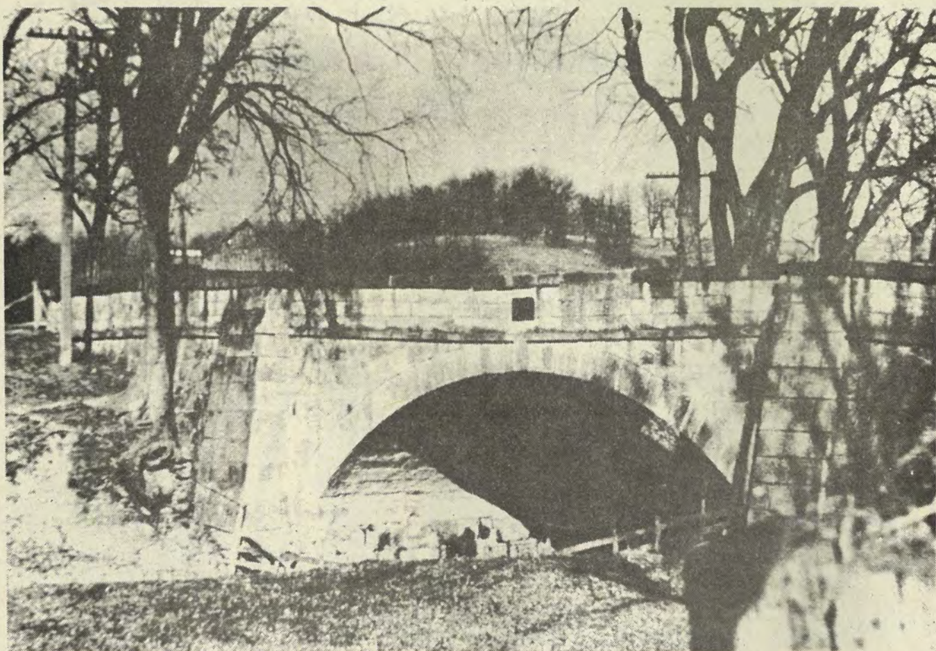
AN "S" BRIDGE in Ohio, located about five miles west of Old Washington, was erected in 1828. It is one of four remaining in that state. It is located in a small roadside park just off U.S. 40.
