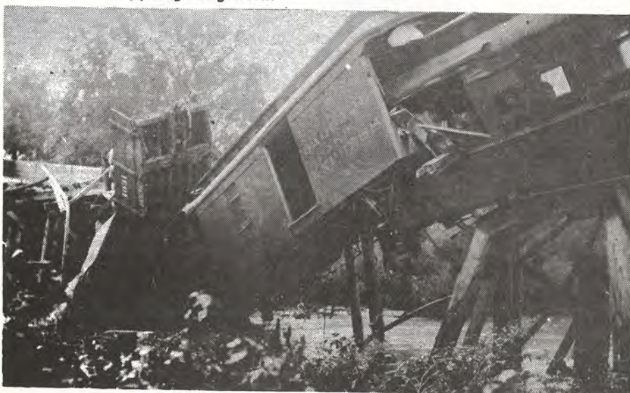
WRECK ON the W. C. & W (Wait, Charlie and Walk) near Pinckneyville on September 7, 1911, was apparently the result of faulty bridgework.
