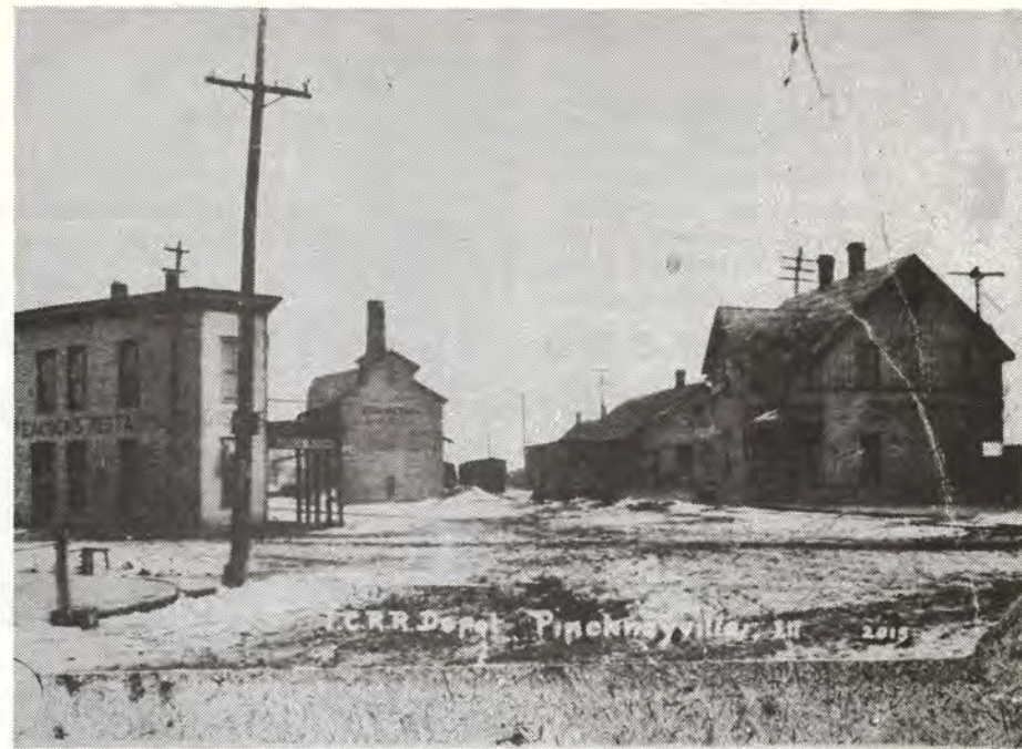
DEPOT OF the Illinois Central R.R. in Pinckneyville (right), is shown with flat-iron shaped Peacock's Restaurant (left) and grain elevator (center).
