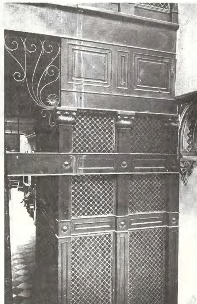
PASSENGER ELEVATOR appears to have been installed at the time of construction of the building.
