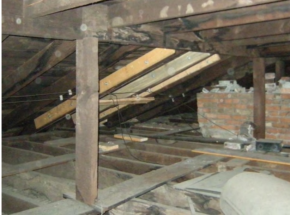
PHOTOGRAPH 17 Reddick Mansion Structural Evaluation 100 W. Lafayette St., Ottawa, Illinois
