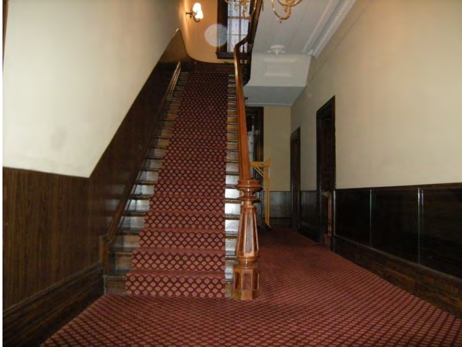
PHOTOGRAPH 13 Reddick Mansion Structural Evaluation 100 W. Lafayette St., Ottawa, Illinois
