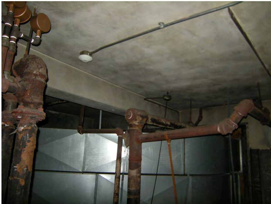
PHOTOGRAPH 14 Reddick Mansion Structural Evaluation 100 W. Lafayette St., Ottawa, Illinois
