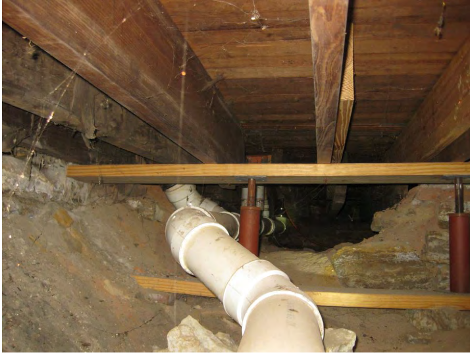
PHOTOGRAPH 7 Reddick Mansion Structural Evaluation 100 W. Lafayette St., Ottawa, Illinois
