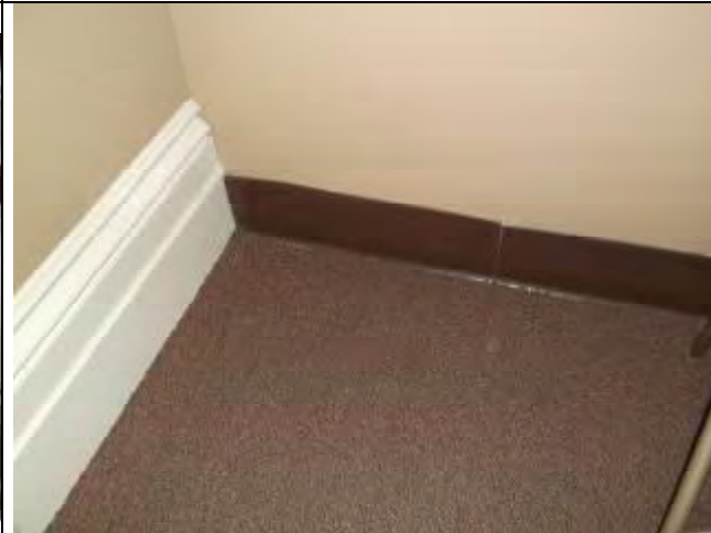
12. View of PACM 6'' maroon vinyl baseboard located on the second floor.
