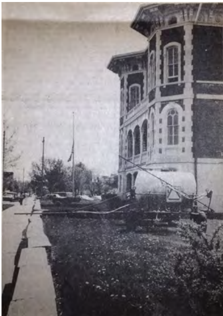
Photo Site – 28: Newspaper clipping (no date) showing the dilapidated state of the retaining wall in the mid-1970s. (RMA collection)
