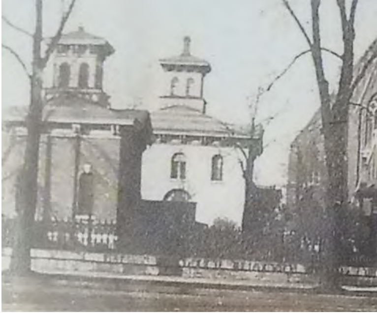
Photo Site – 11: Early view of the Caretaker’s House (note there is no entry porch) before the second story windows were installed. The Carriage house is beyond (From a larger panoramic photograph, RMA collection).
