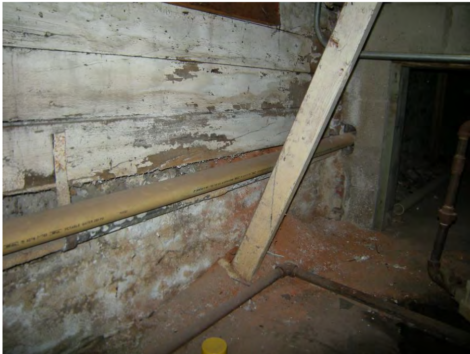
PHOTOGRAPH 12 Reddick Mansion Structural Evaluation 100 W. Lafayette St., Ottawa, Illinois
