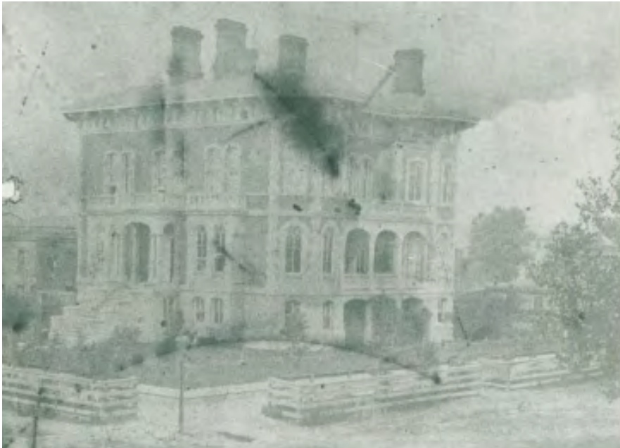
Photo Site – 25: Undated historic view of the Mansion and immediate site. (Reddick Library collection)
