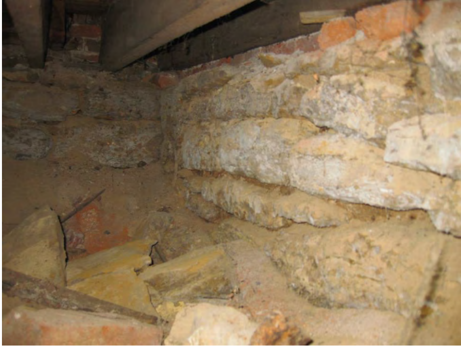
PHOTOGRAPH 9 Reddick Mansion Structural Evaluation 100 W. Lafayette St., Ottawa, Illinois
