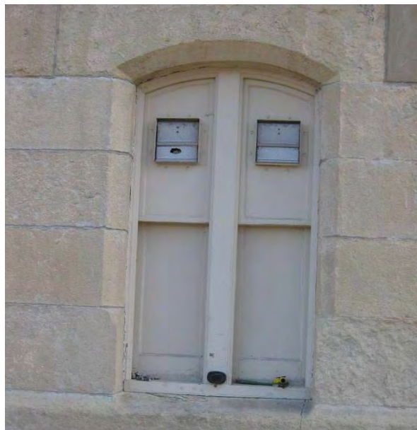
Exhaust Fan Discharge from First Floor Toilet Rooms
