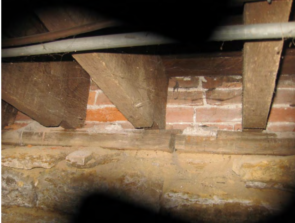
PHOTOGRAPH 1 Reddick Mansion Structural Evaluation 100 W. Lafayette St., Ottawa, Illinois
