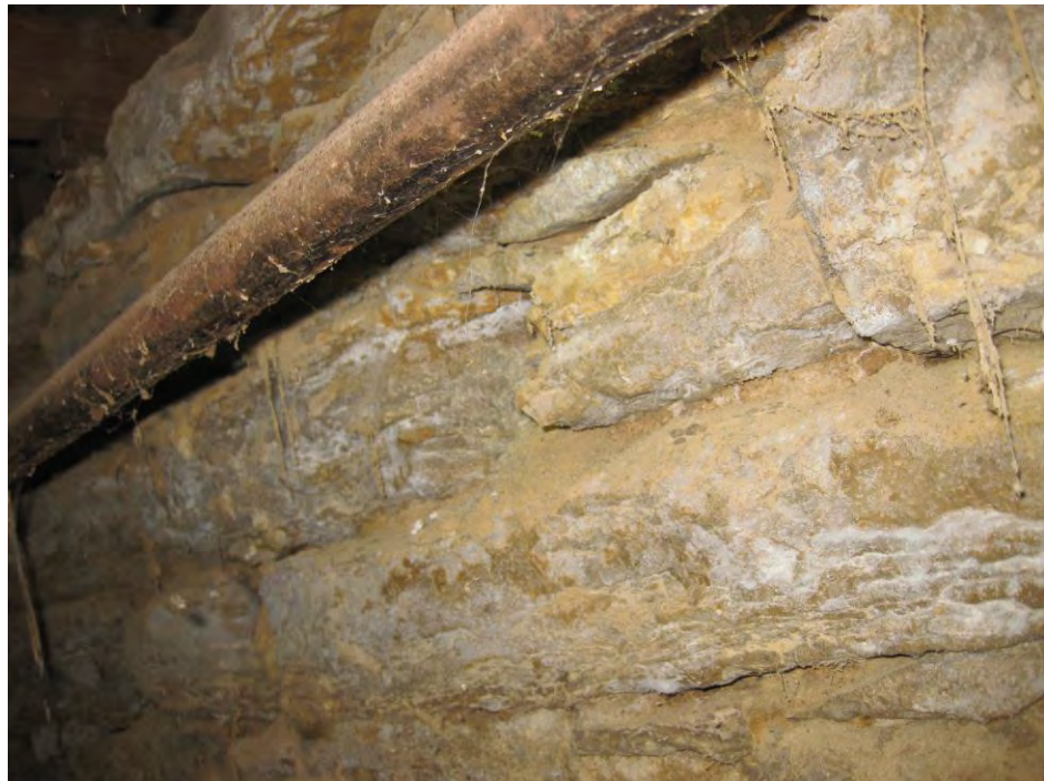
PHOTOGRAPH 10 Reddick Mansion Structural Evaluation 100 W. Lafayette St., Ottawa, Illinois
