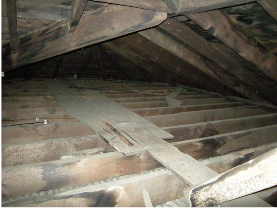
PHOTOGRAPH 15 Reddick Mansion Structural Evaluation 100 W. Lafayette St., Ottawa, Illinois
