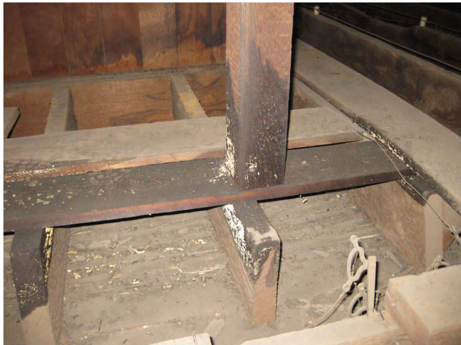
PHOTOGRAPH 16 Reddick Mansion Structural Evaluation 100 W. Lafayette St., Ottawa, Illinois
