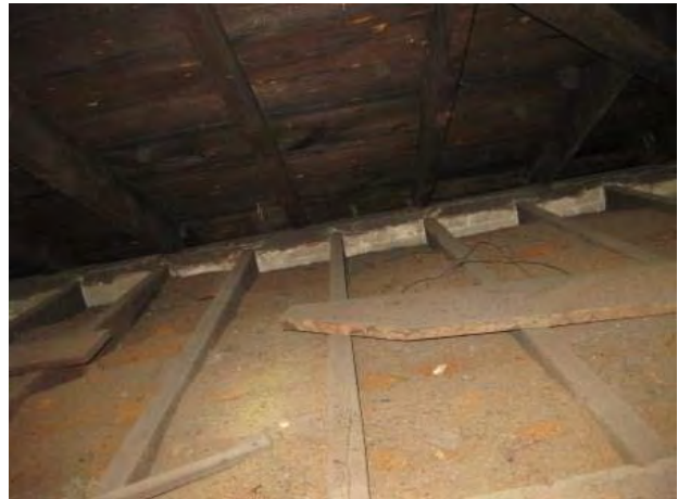
Insulation in Floor Joists Over Water Tank Room - Attic
