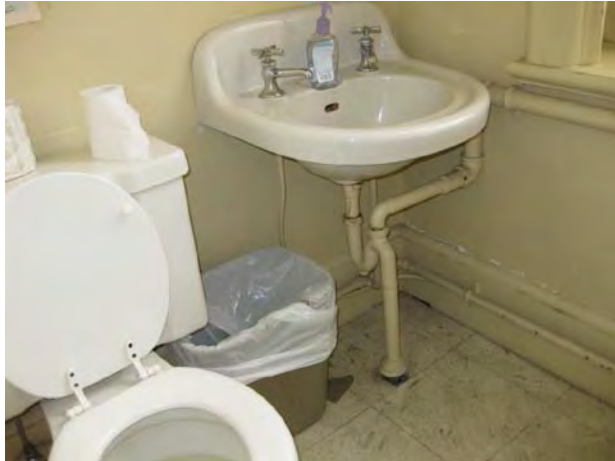
Third Floor Toilet Room
