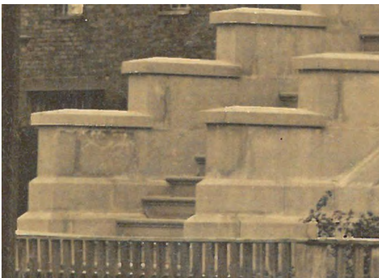
Photo E-20: Detail view from an early photograph shows how the treads once had a "lip" that overhung the risers.
