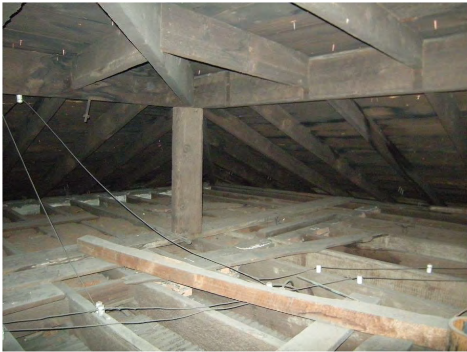
PHOTOGRAPH 6 Reddick Mansion Structural Evaluation 100 W. Lafayette St., Ottawa, Illinois
