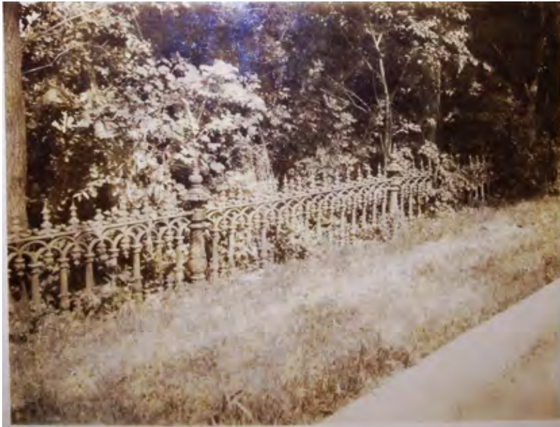
Photo Site - 26: View of the cast iron fence when it was installed at the Jewish Cemetery. (RMA collection)
