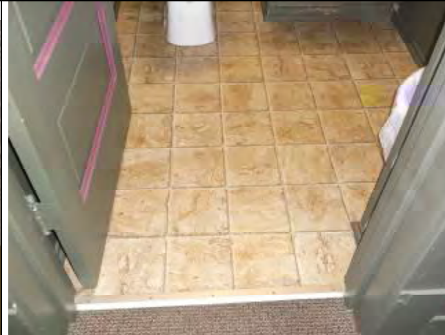
10. View of PACM vinyl sheet flooring located on the ground floor.
