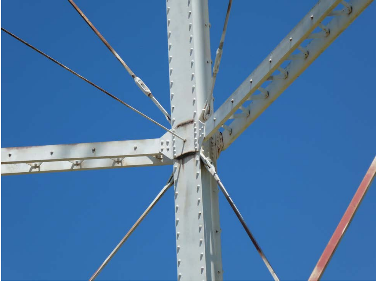
Figure 10. Detail view of interior leg and support, facing north.
