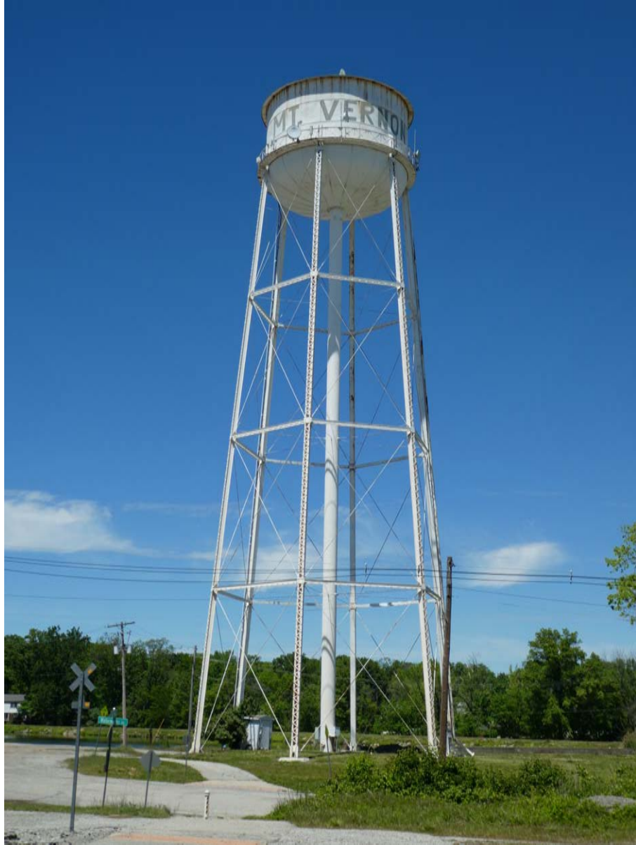
Figure 4. Mt. Vernon L&N Elevated Water Storage Tank, facing north.
