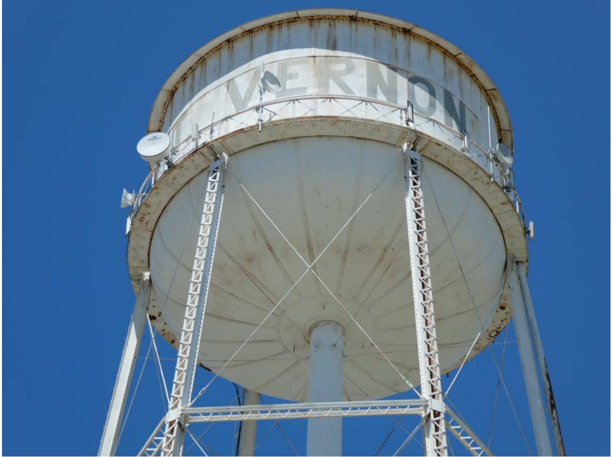
Photo 6 - Detail view of water tank, facing northwest.
