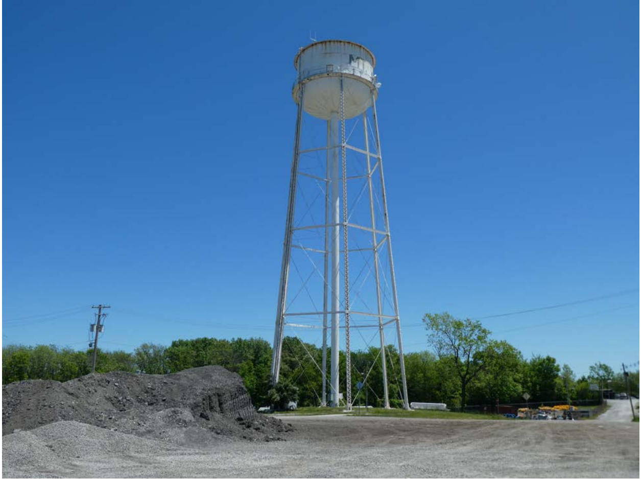
Figure 5. Mt. Vernon L&N Elevated Water Storage Tank, facing east.
