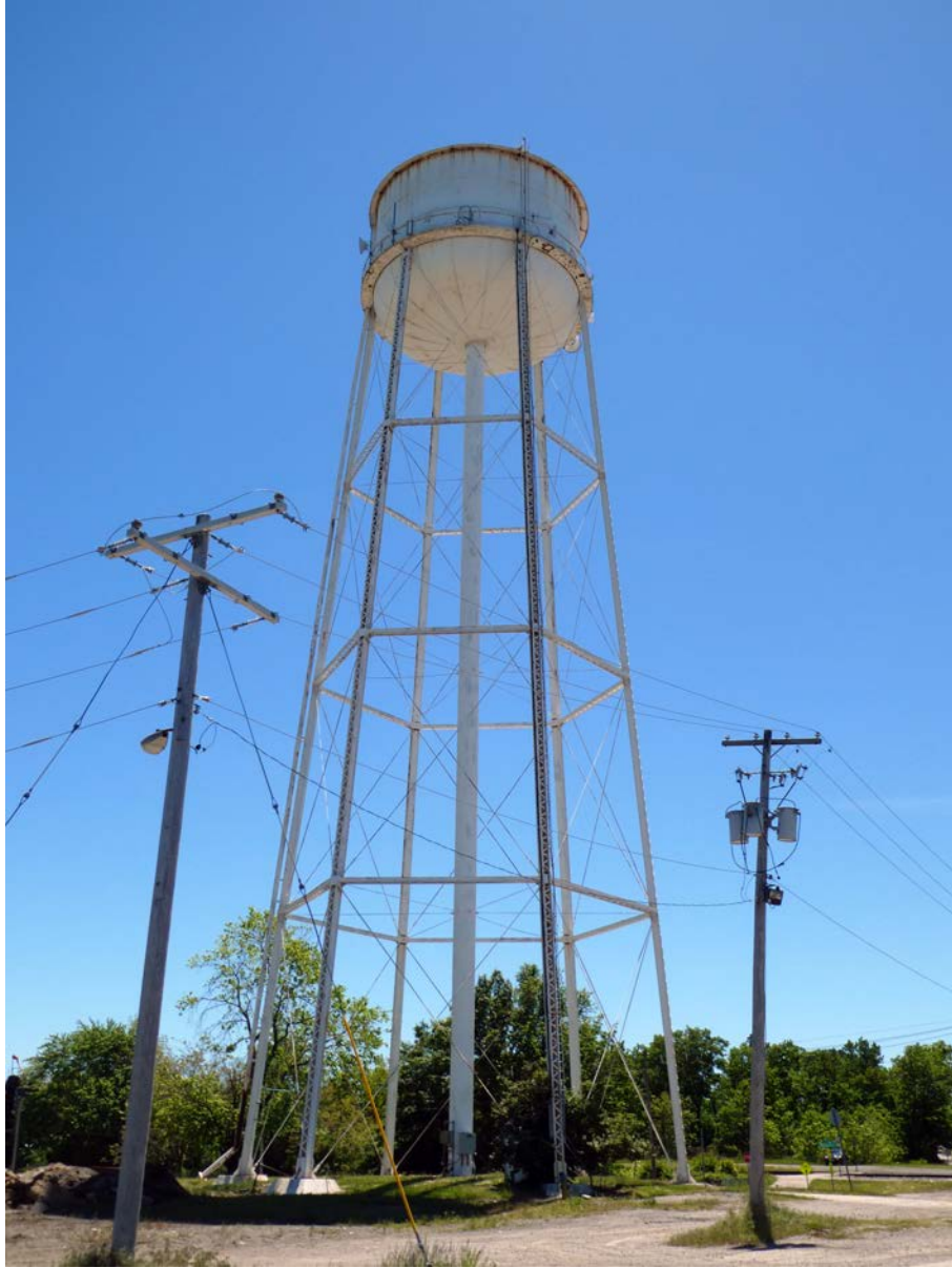
Figure 6. Mt. Vernon L&N Elevated Water Storage Tank, facing south.
