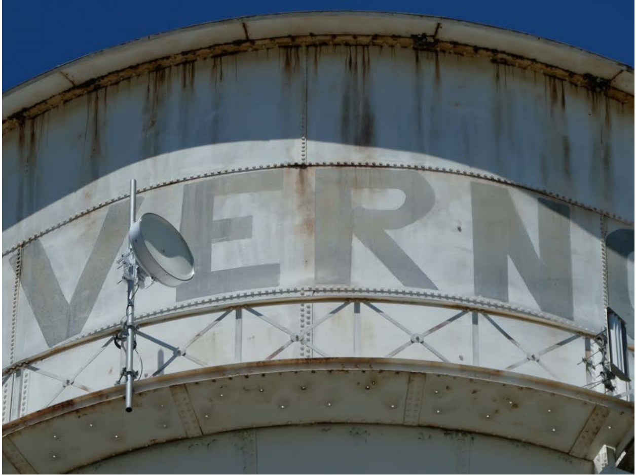
Photo 7 - Detail view of riveted tank construction, facing northwest.
