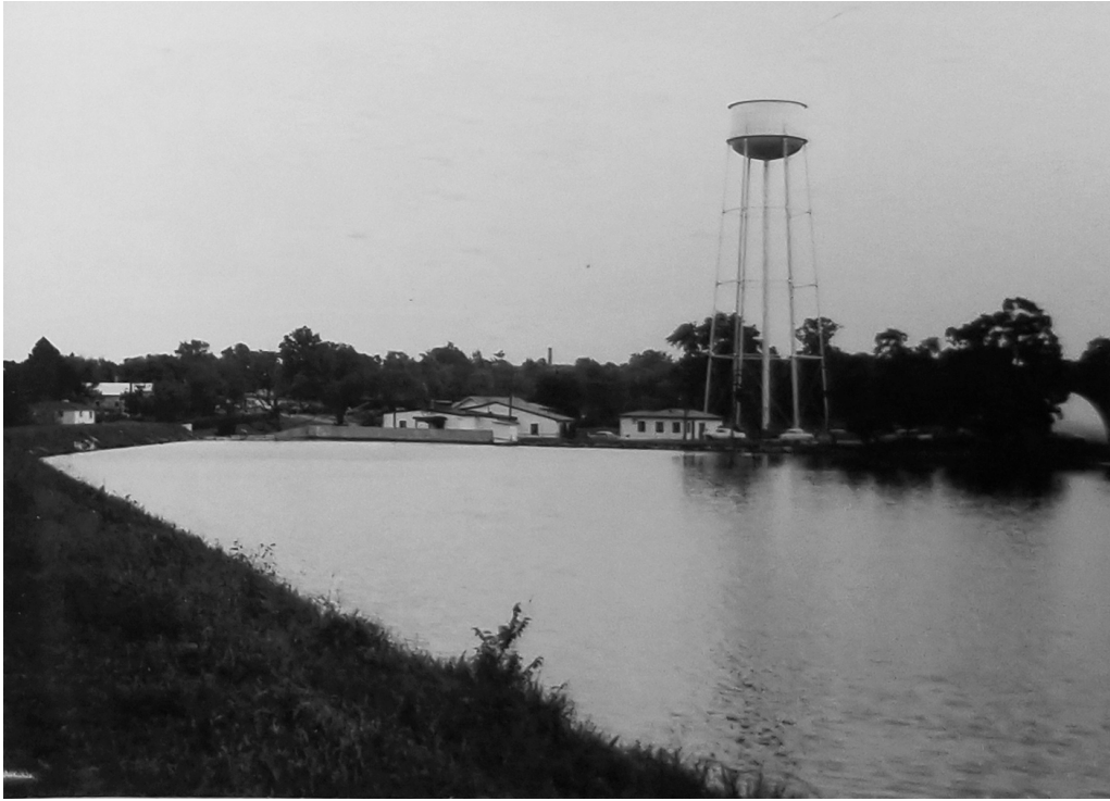
1959 Photograph of water tower (Courtesy of the Jefferson County Historical Society).
