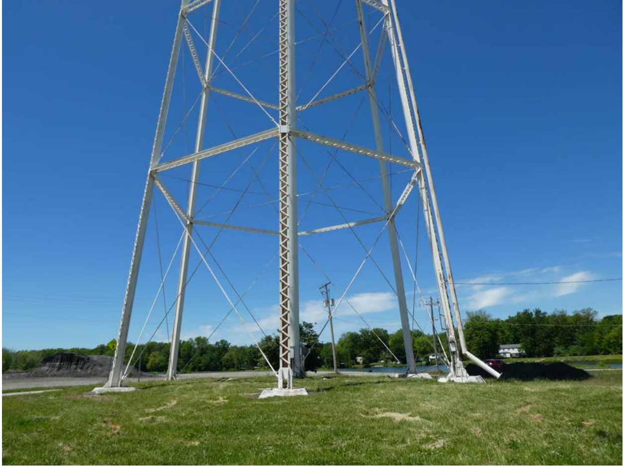
Figure 9. Detail view of support structure, facing northwest.
