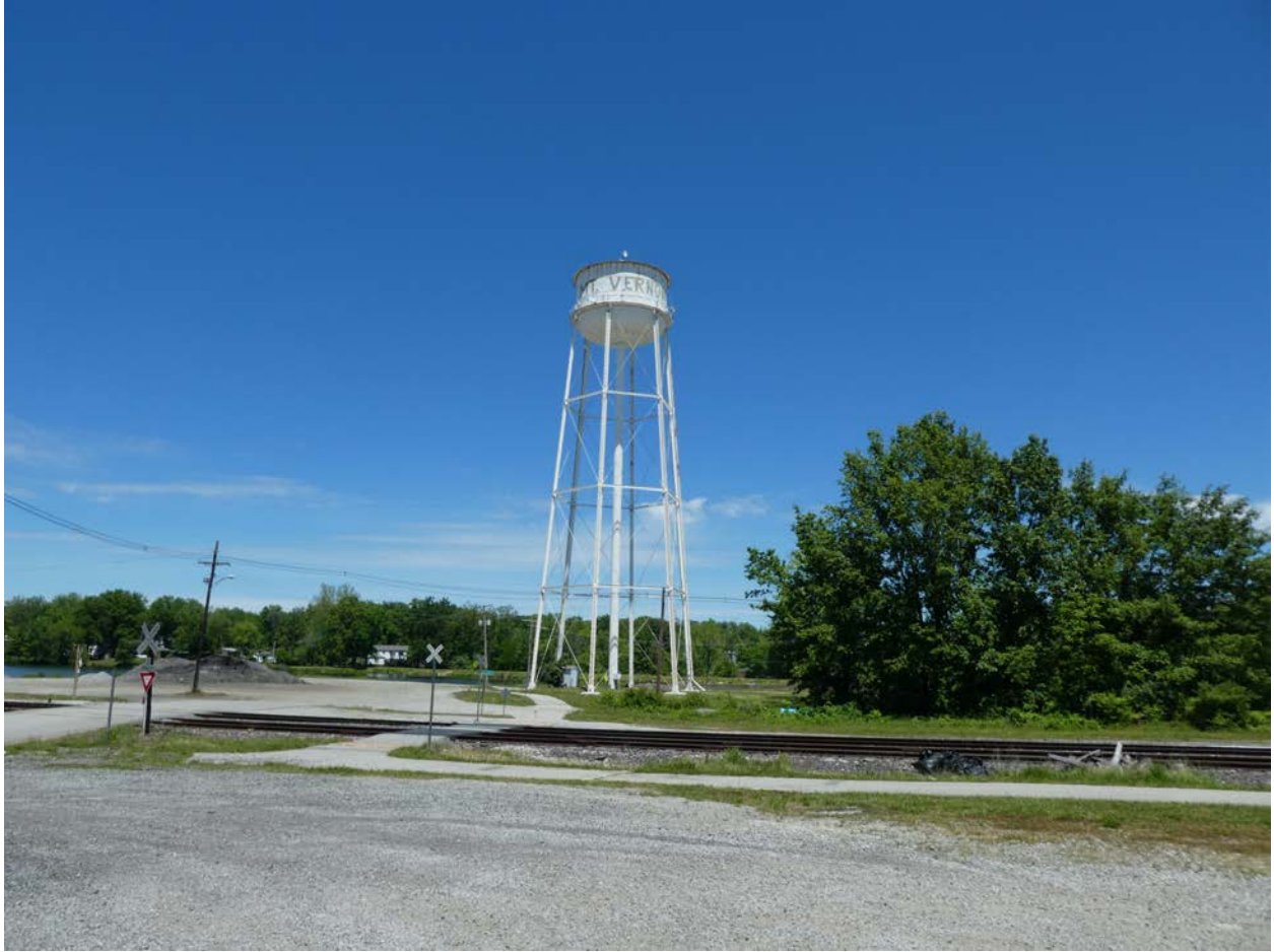
Photo 20 - Water tower area, approach to tower from 20th Street, facing north.
