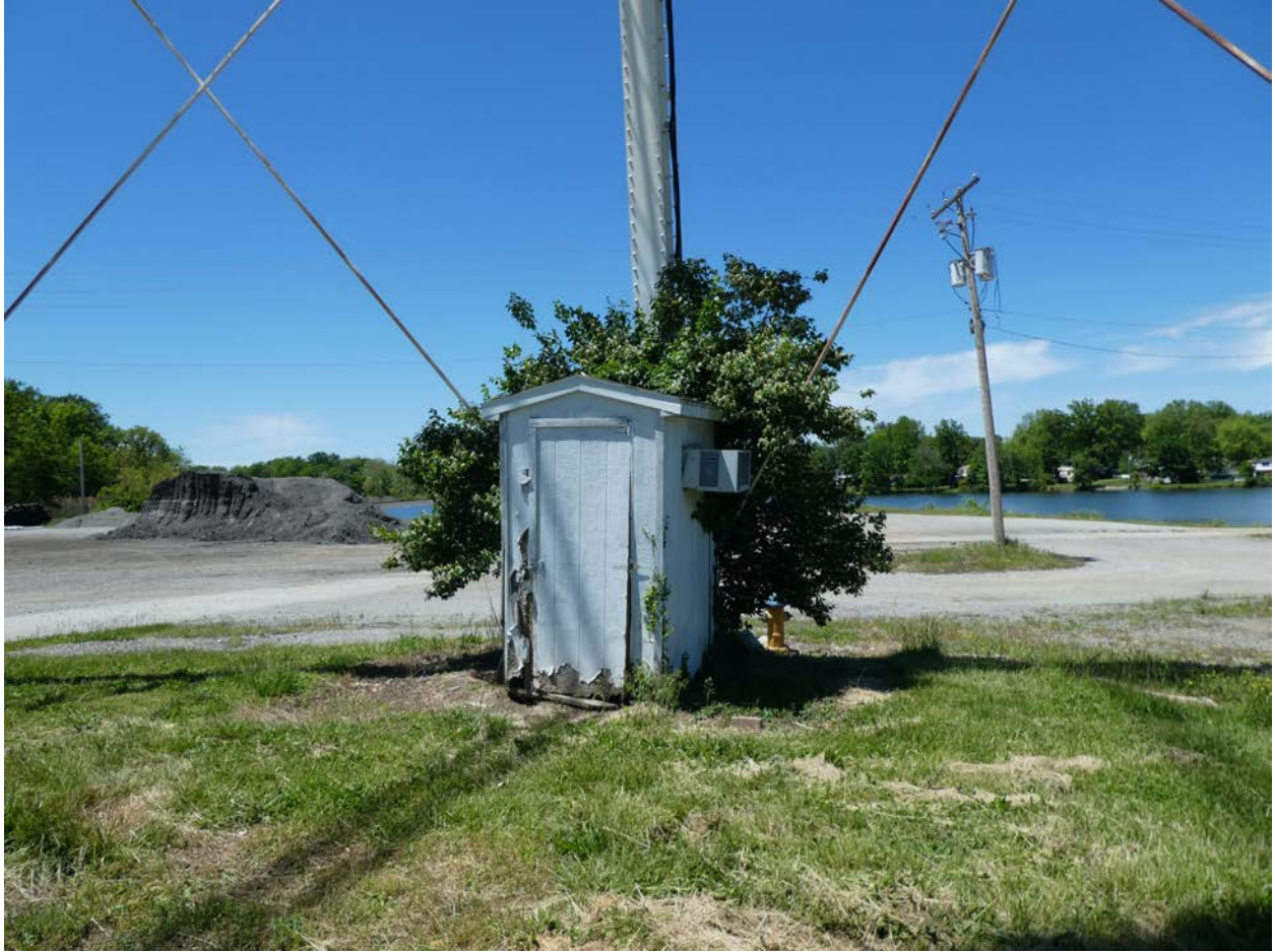
Photo 17 - Shed at base of water tower, facing northwest.
