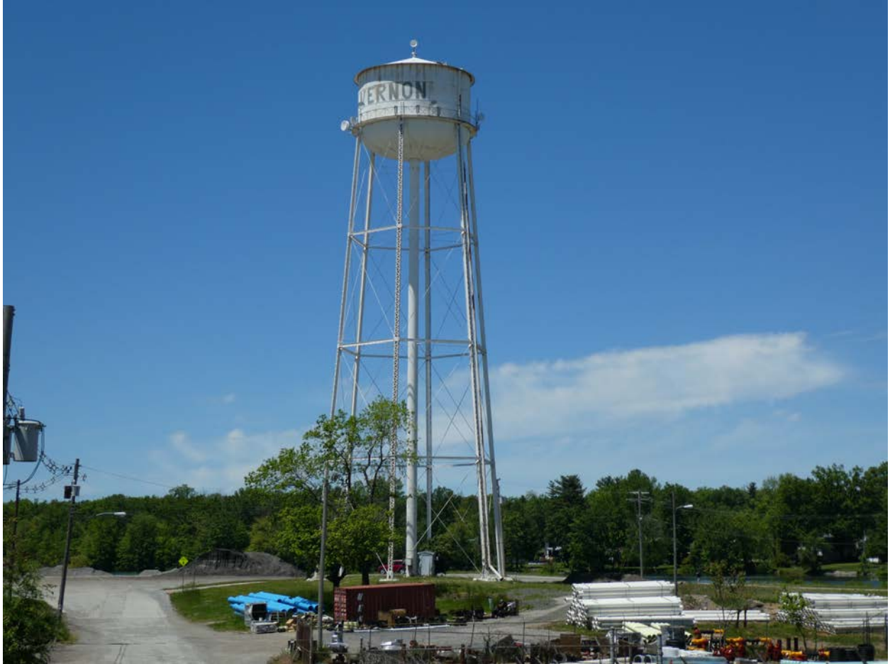
Figure 3. Mt. Vernon L&N Elevated Water Storage Tank contextual view.
