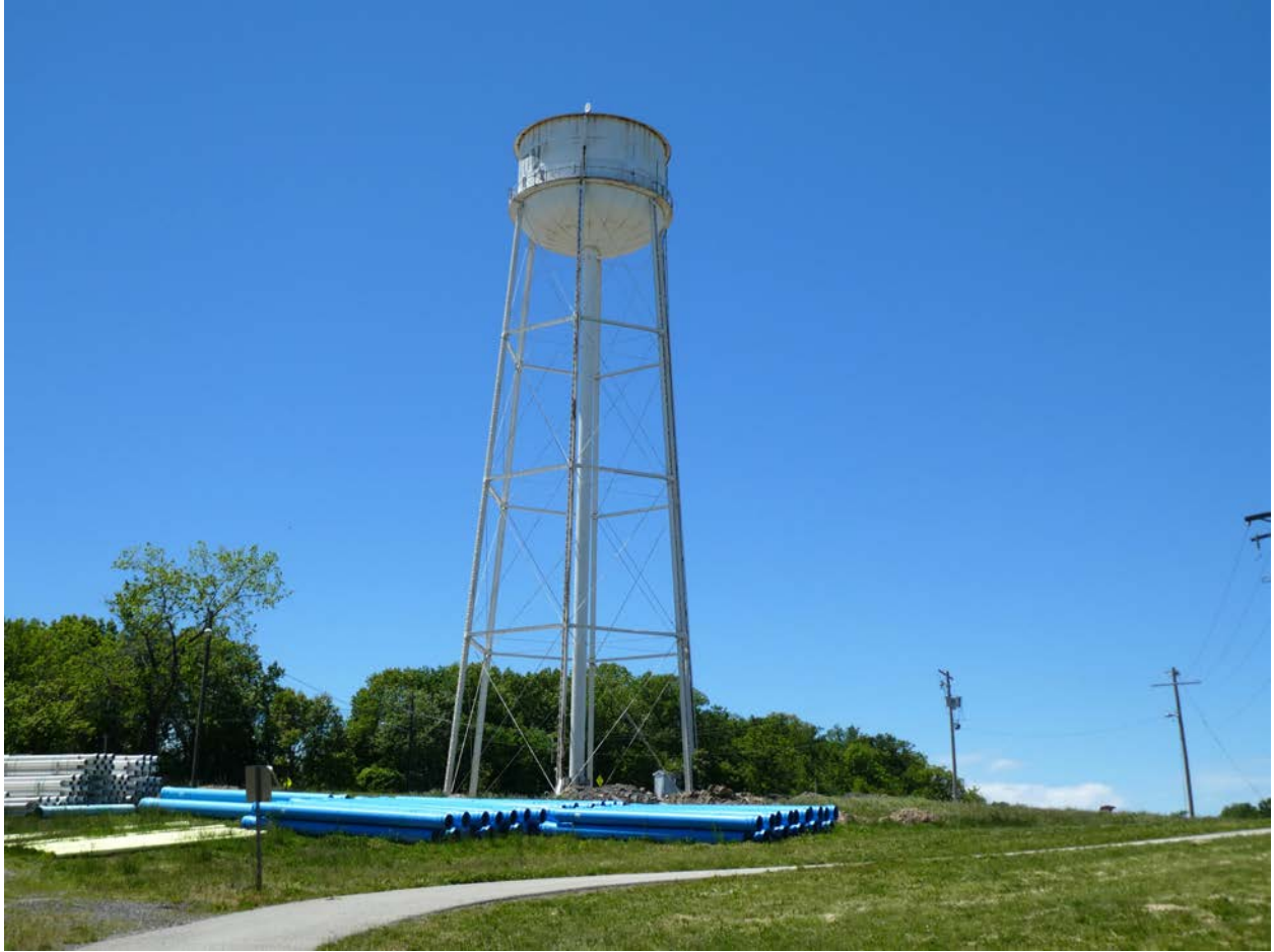
Figure 7. Mt. Vernon L&N Elevated Water Storage Tank, facing west.
