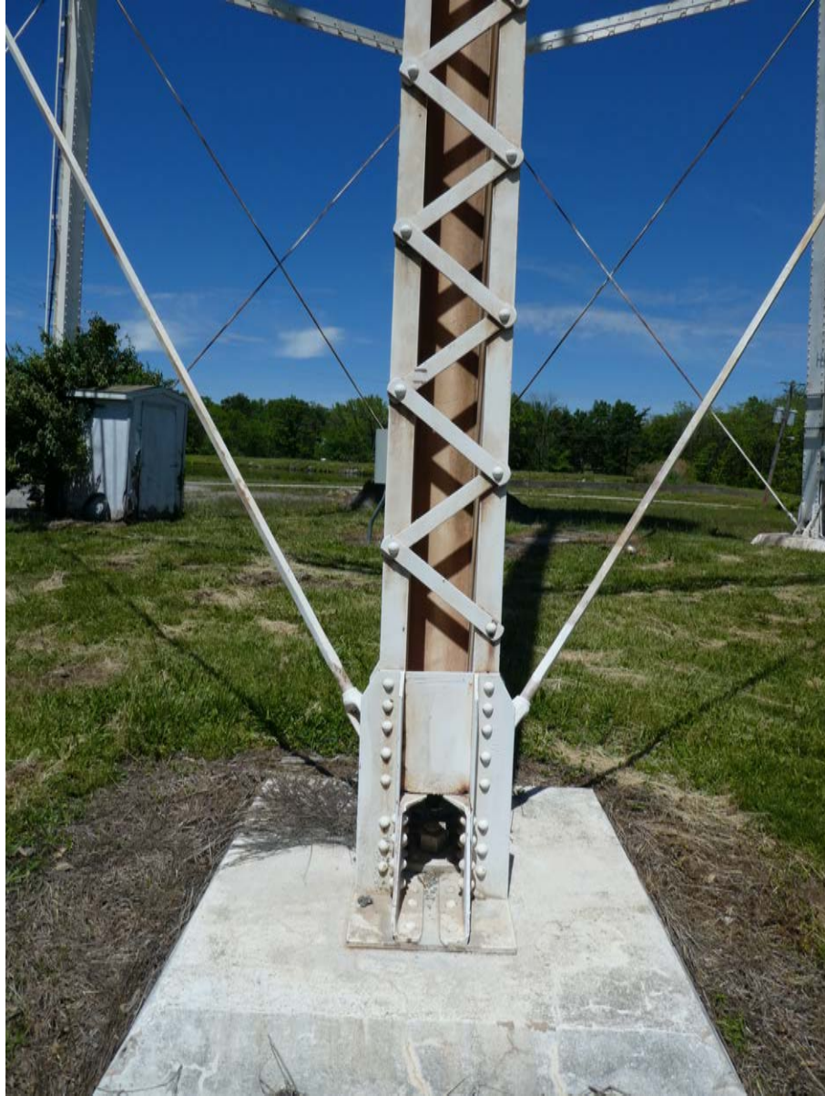
Figure 8. Detail view of tower leg support structure, facing north.
