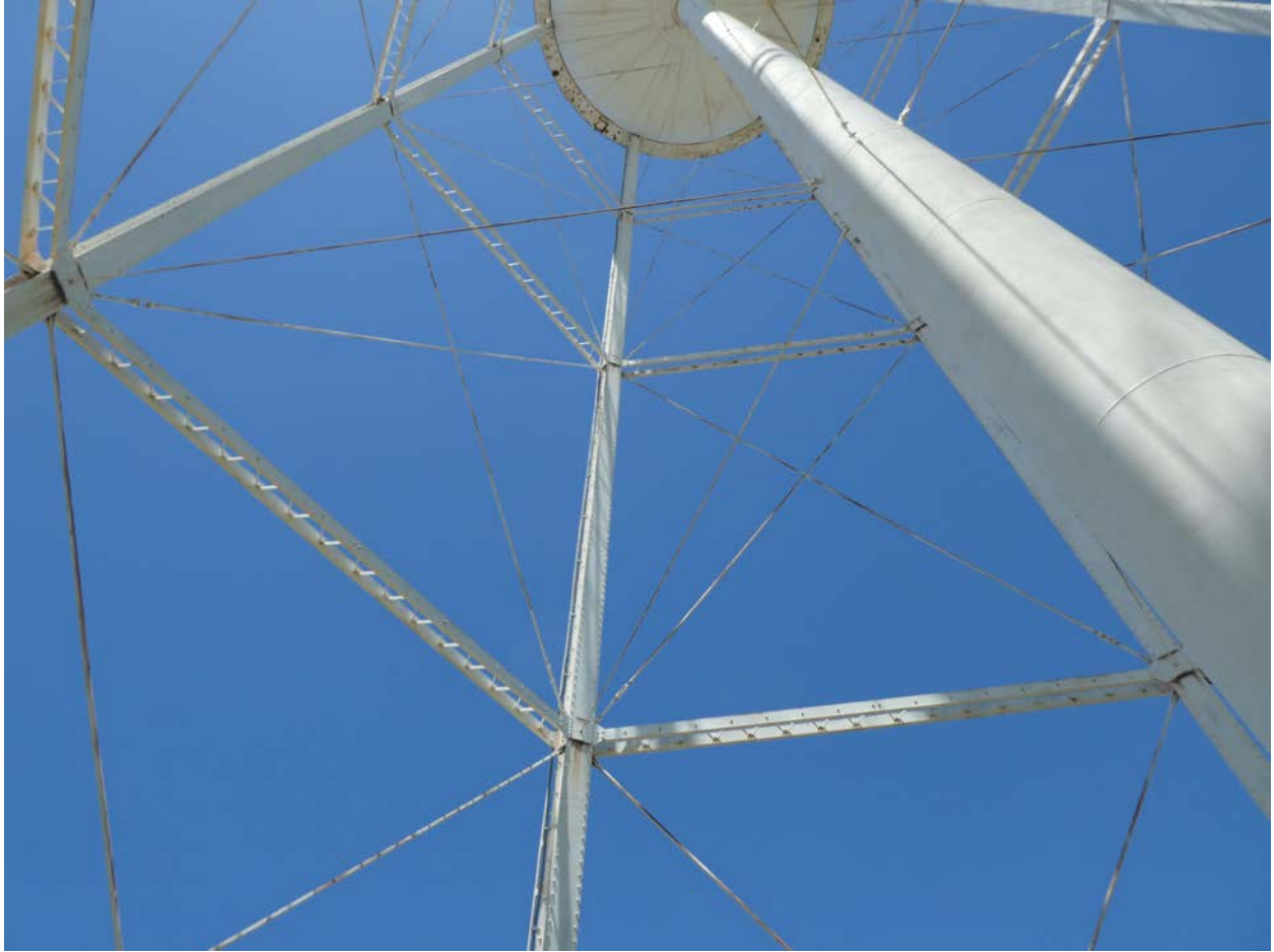
Figure 11. Detail view of tower tension support, facing north.
