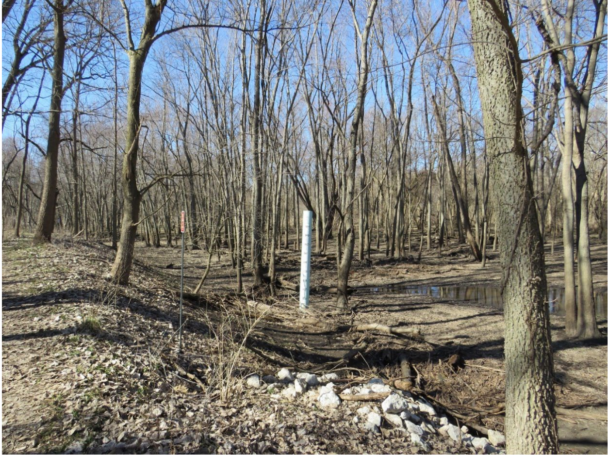
Figure 4-7. BH-RR-01. Bruce Hannon Levee Trail. Culvert and Water Level Gauge. Photograph taken from Tour Stop 4. View to the Northwest. Tetra Tech, 2024.
