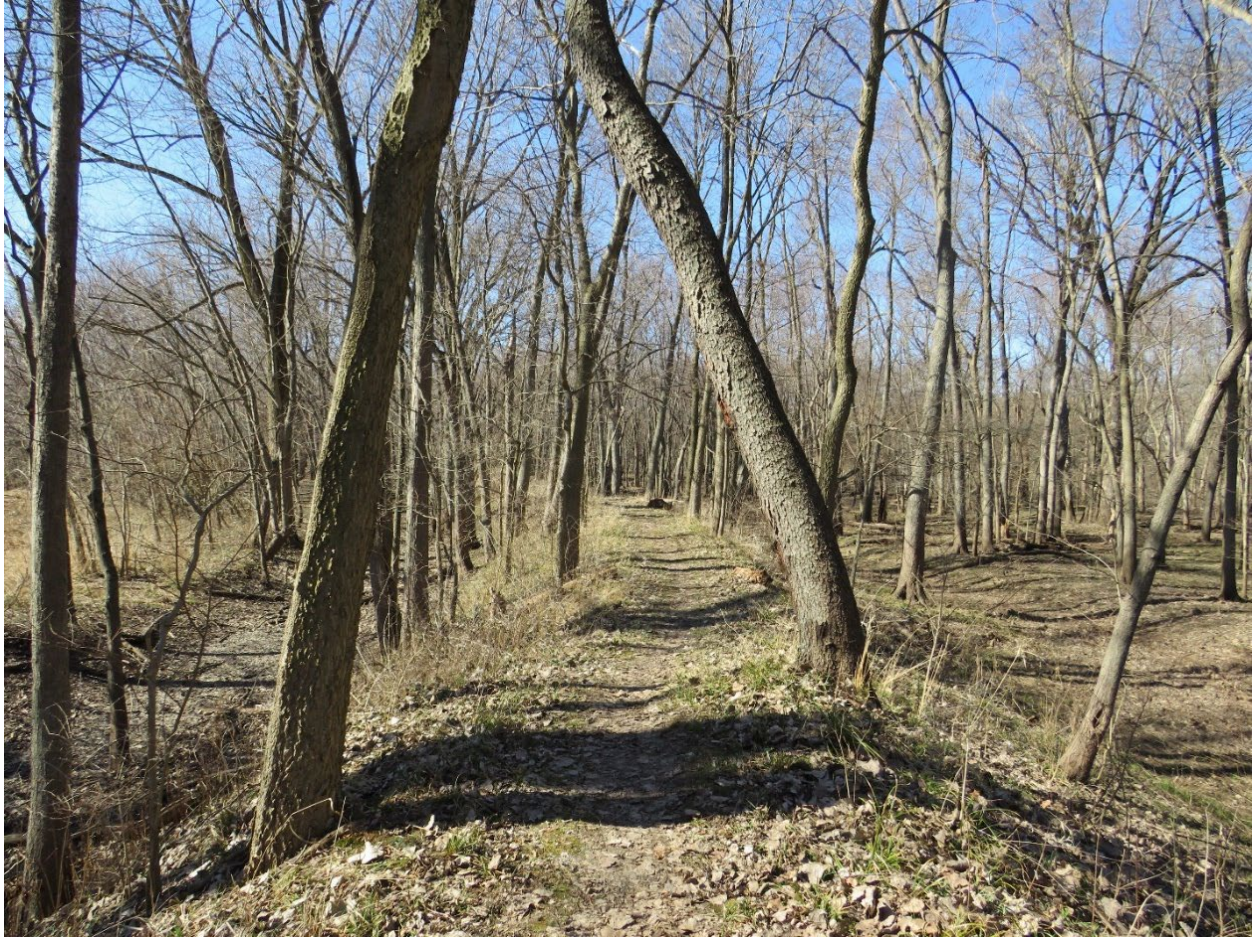
Figure 4-6. Bruce Hannon Levee Trail. Levee Overview. Photograph taken between Tour Stop 3 and Tour Stop 4. View to the Northwest. Tetra Tech, 2024.
