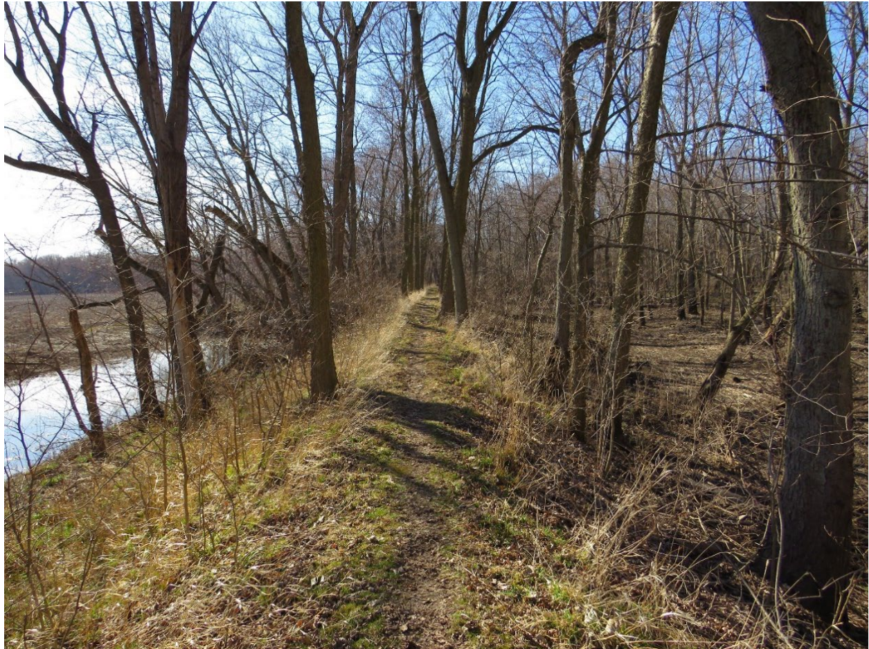
Figure 4-17. Bruce Hannon Levee Trail. Levee Overview, with Floodplain Restoration area at left, and Floodplain Forest at right. Photograph taken between Tour Stop 6 and Tour Stop 7. View to the West. Tetra Tech, 2024.
