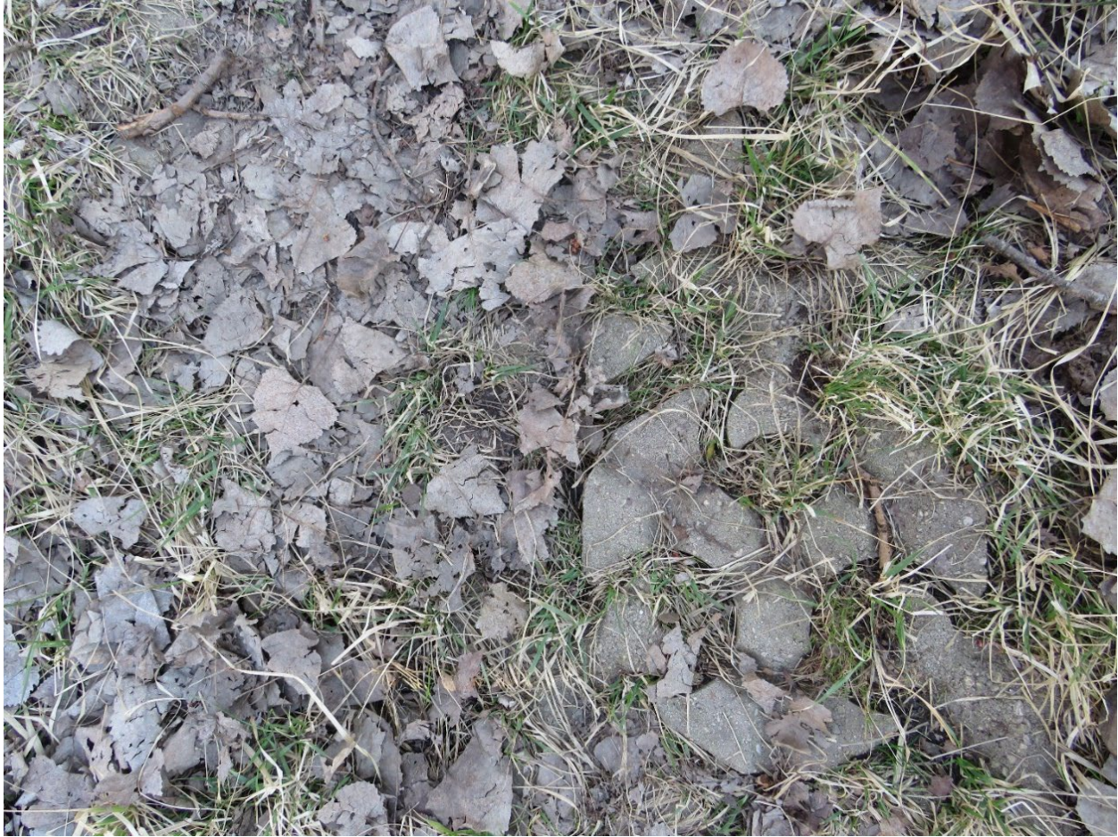
Figure 4-10. BH-RR-02. Bruce Hannon Levee Trail. Detail of Drainage Tiles. Photograph taken between Tour Stop 4 and Tour Stop 5. Tetra Tech, 2024.
