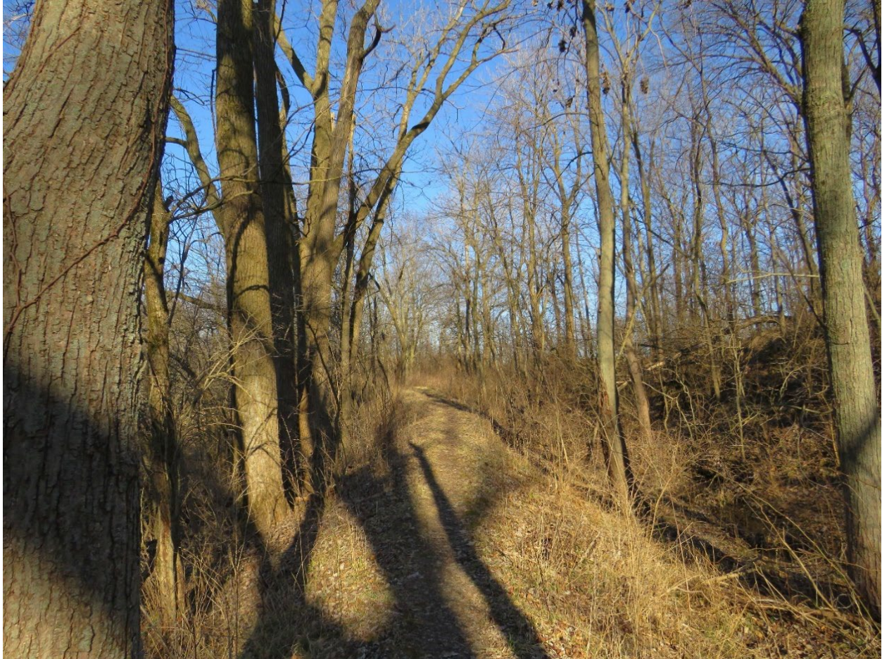
Figure 4-25. Bruce Hannon Levee Trail. Levee Overview. Photograph taken between Tour Stop 11 and Tour Stop 12. View to the Northeast. Tetra Tech, 2024.
