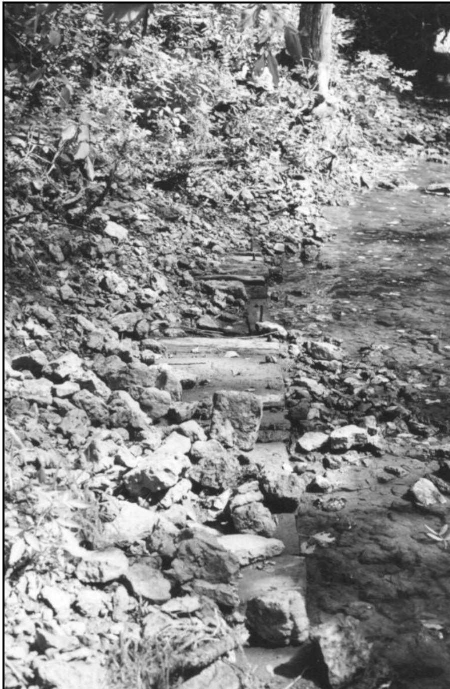
Figure 35. View of the section of framing found exposed along the north bank of the Apple River's south fork in 1999, looking east. The two figures that follow illustrate structural details of the framing (FRR August 1999).
