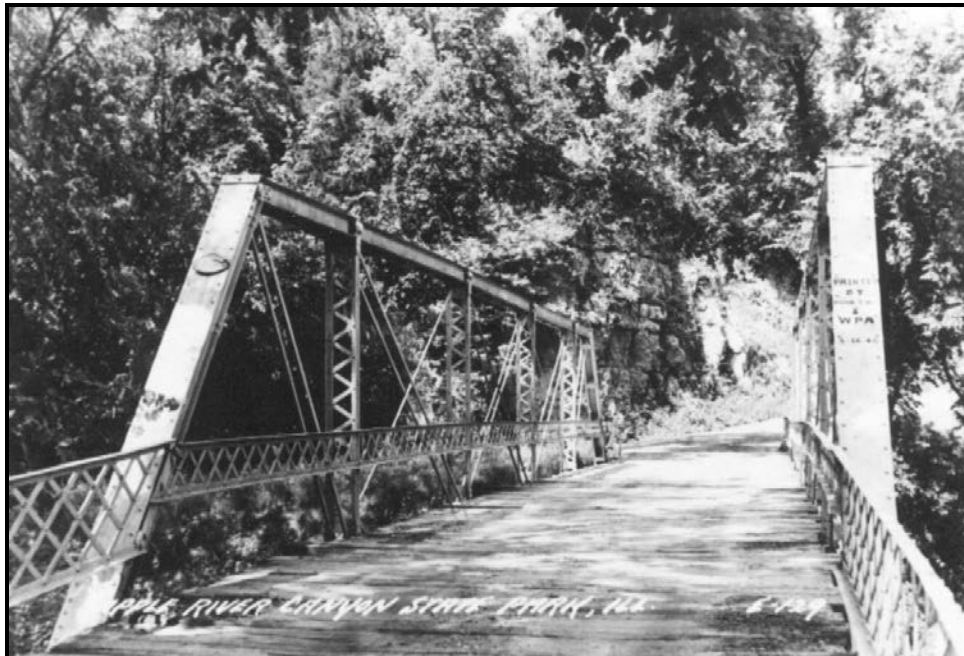
Figure 26. Two historic views of the Pratt Pony Truss bridge that was erected across the South Fork Apple River during the late nineteenth century. The top photograph, which is undated but appears to be the older of the two, was taken from a point downstream from the bridge, looking east. Note the horse-drawn buggy that has stopped on the bridge. The bottom view was taken from the south end of the bridge, looking north. This picture probably dates from the later 1930s or early 1940s (note that the east truss of the bridge is stenciled with a sign saying, “Painted by Rush Twn[?]. & WPA.” The paint line that is visible on the west truss suggests that the bridge either was in the midst of being painted when the photograph was taken, or that the work had not quite been finished (ARCSP photograph collection).
