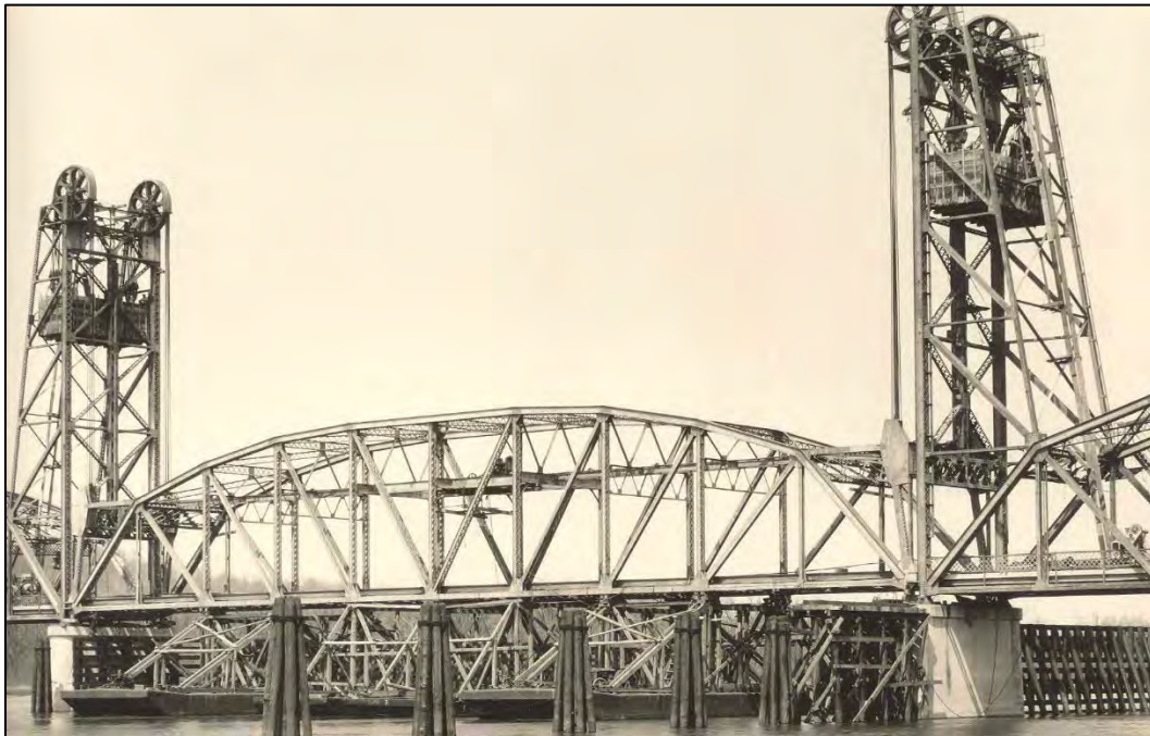
Figure 18: The multi-year project was close to completion when this image was taken. Its caption notes “lift span floated into position” (adapted from the original Bridge Photoset in possession of IDOT and ISAS).
