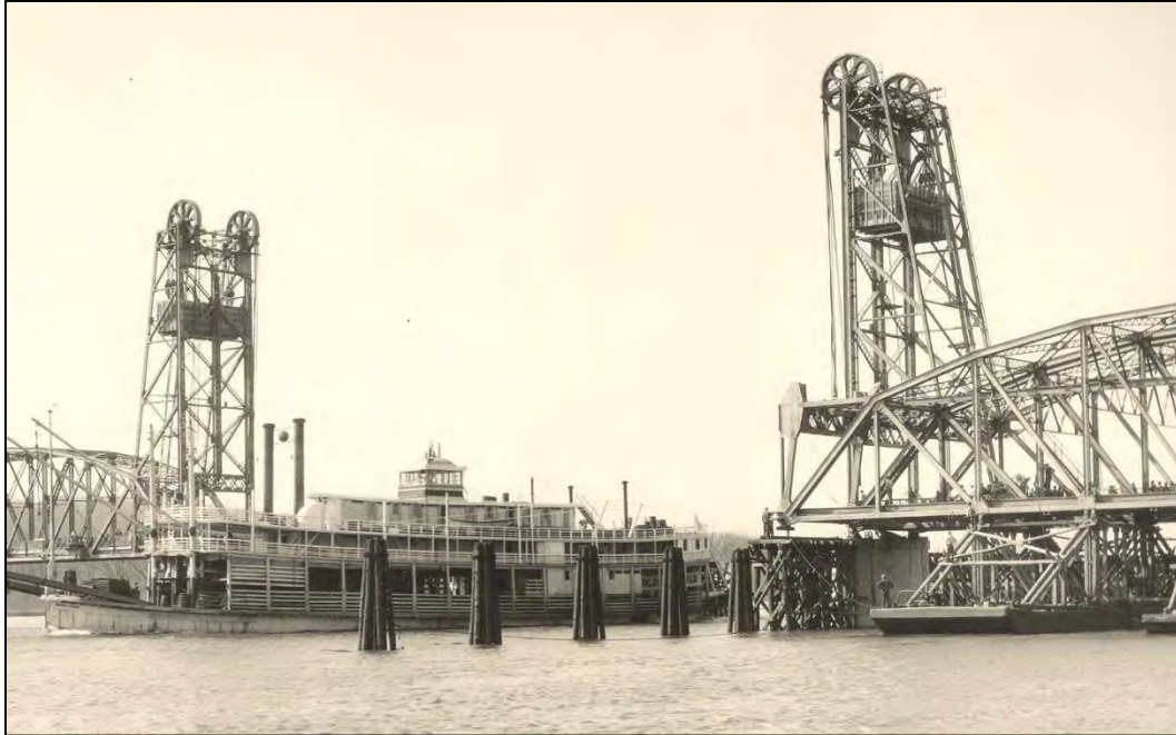
Figure 17: Pictured here, according to the original caption, is “the Golden Eagle going south. Lift span [to the right of the right tower] ready to float into position” (adapted from the original Bridge Photoset in possession of IDOT and ISAS).
