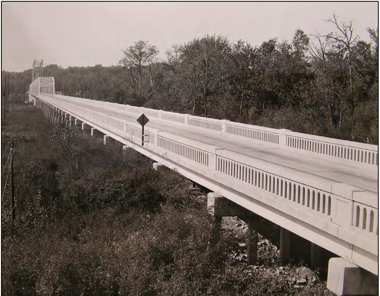
Figure 19: This view is to the north northwest. It illustrates at some unknown point in time the completed structure in general, and the east approach spans in particular. Note that the bridge's original configuration included a Texas Classic Type 411-like, concrete railing with repetitive, arched openings and intermediate blocks over each bent. This railing was subsequently replaced (this image [photo #488608] was viewed at https://bridgehunger.com/il/pike/florence on 15 March 2021).
