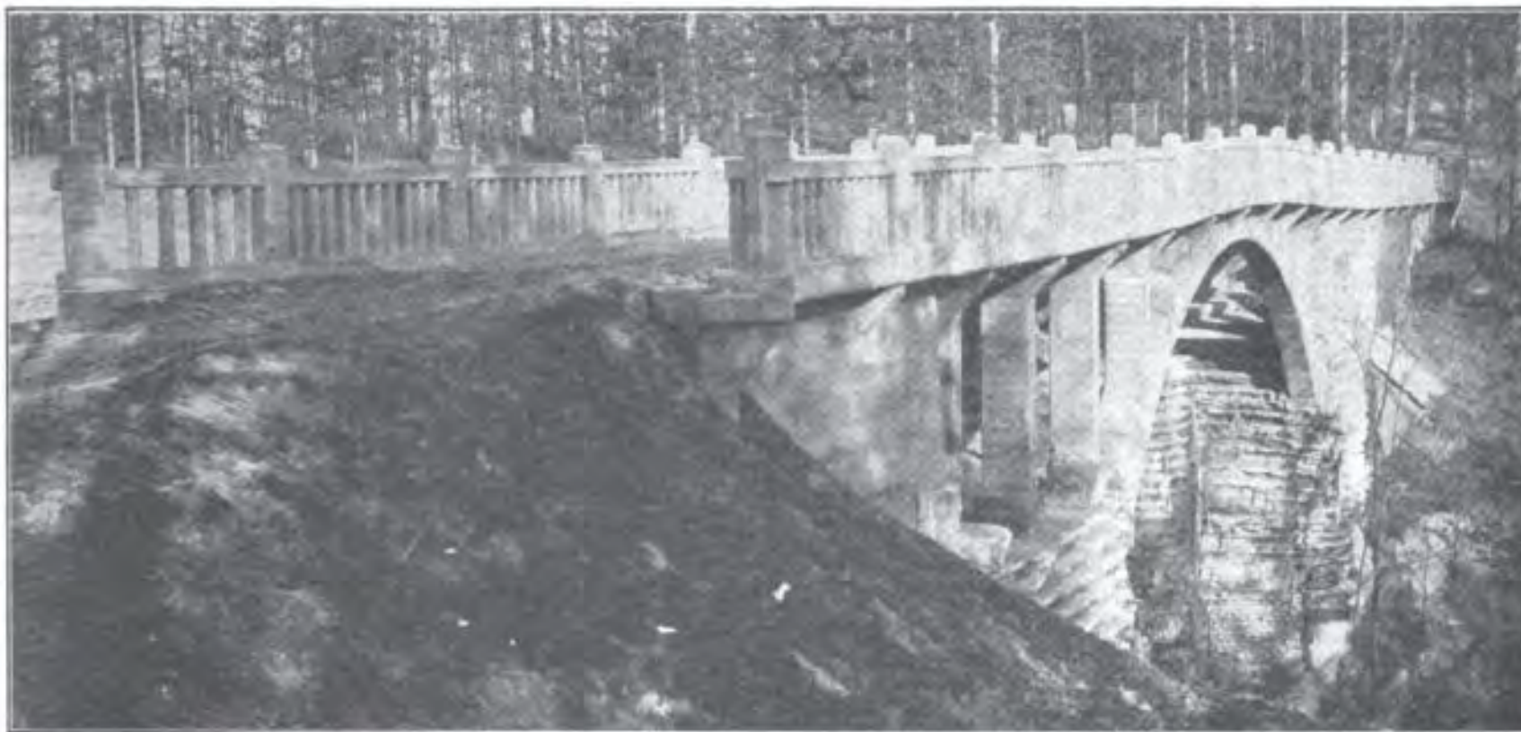
FRONT VIEW OF COMBINED BRIDGE AND DAM, SHOWING IMITATION OF STRATIFIED ROCK IN CONCRETE
