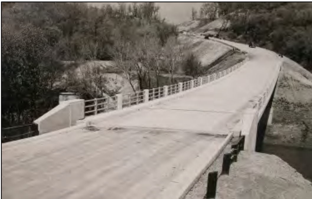
Figure 10: View to North illustrating the original deck and its railing. Viewed at http://bridgehunter.com/il/la-salle/5030381146/ on 05 December 2015.
