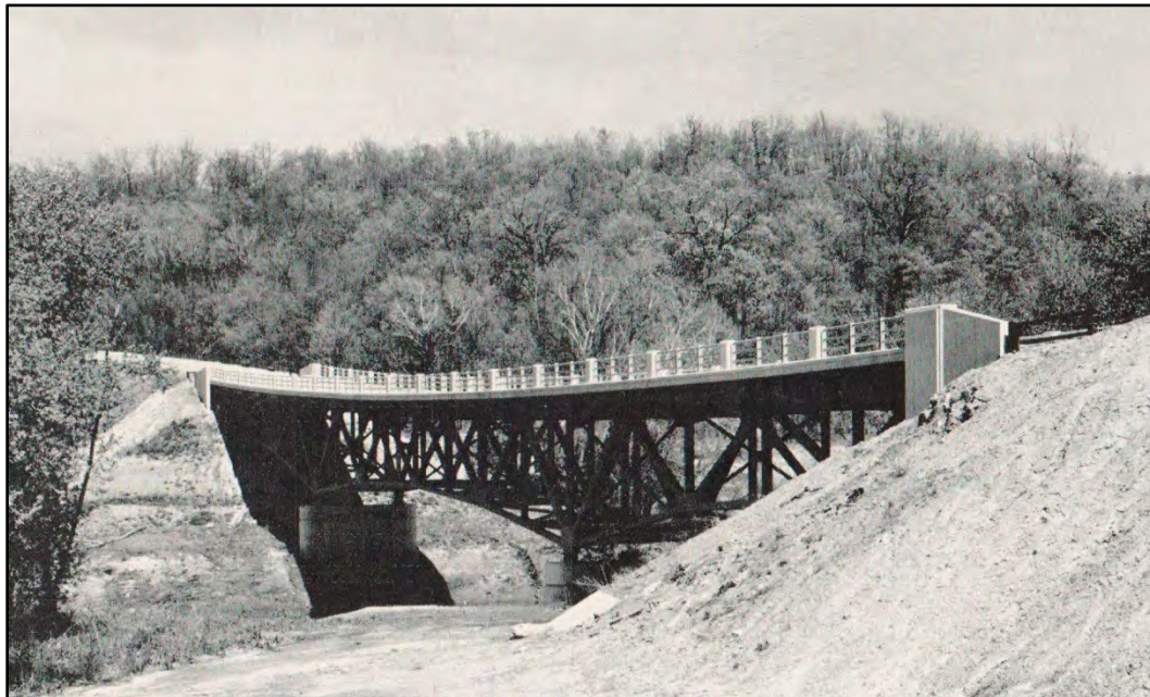
Figure 8: View to the Northeast. This image illustrates the finished bridge. Twenty-Fifth Annual Report of Division of Highways, Department of Public Works and Buildings for the Year 1942 (Springfield, IL: State of Illinois, 1942), 176.
