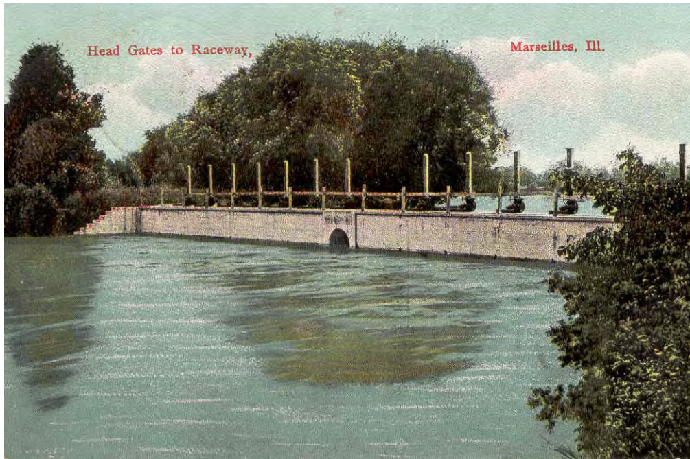
Figure 5. Postcard showing Head Gate at the North Head Race, 1911 From the archives of: Marseilles Land & Water Company
