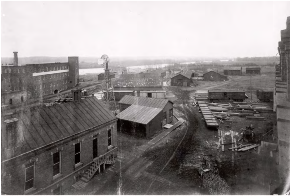
Figure 1. View of Marseilles' manufacturing district, looking southwest toward the Illinois River, ca. 1900. The four-story building at left side of photograph is the former Pitt's Manufacturing Company. The one-story building in the far background, on the river, appears to be the pulp mill and hydroelectric plant that existed by 1898 and was acquired and improved by W.D. Boyce ca.1900.
