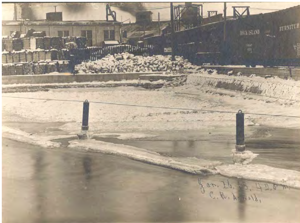
Figure 10. Boyce Paper Mill Site: view looking southeast across forebay of the Marseilles Hydro Plant, 1915 From the archives of: Marseilles Land & Water Company
