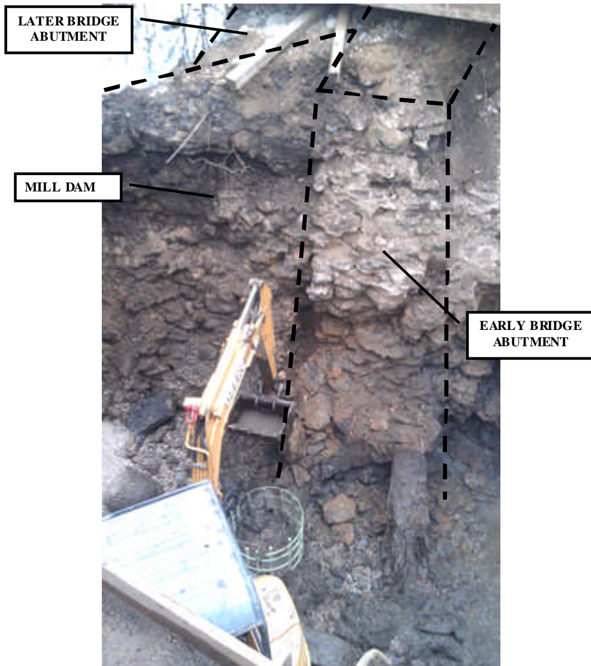
Photograph taken during the excavation of a trench along the rear side of the west end of the Blackberry Creek Dam, showing the junction of the dam and the abutment of the River Road Bridge. This photograph suggests that there may have been two episodes of stone abutments for the bridge: an earlier rubble abutment that the dam was built up against; and a later abutment of ashlar masonry laid up against the pre-existing abutment.
