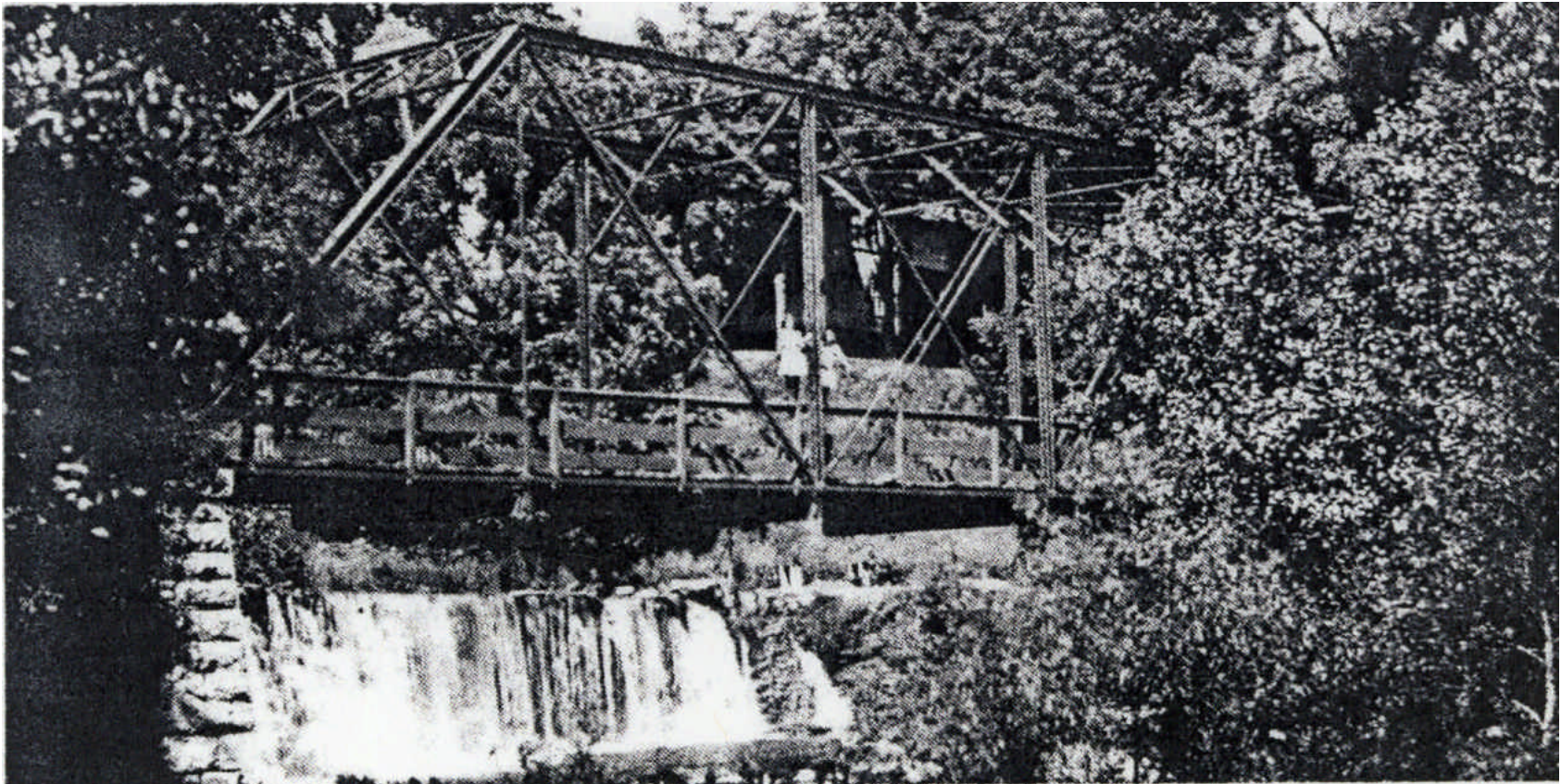
Circa-1900 photograph of the iron-truss bridge over Blackberry Creek on River Street in Bristol. The Blackberry Creek Dam appears in the background, just beyond the bridge. The iron-truss bridge would remain in use until 1959, when it was replaced by a concrete-deck span. The stone bridge abutment shown at left was left undisturbed, however, and it remains in place to the present day. This photograph is part of the Alice Tarbox Dunger Collection and was published in A Bicentennial History of Kendall County (1976).
