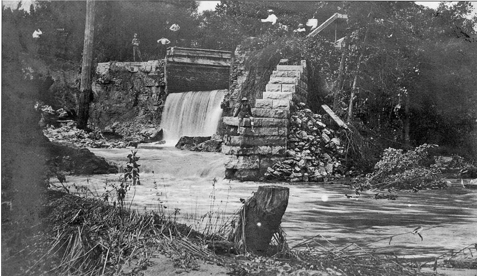
Another view of the Nettle Creek Aqueduct after the break in the canal in the spring of 1910. This image provides a good illustration of the manner in which the abutment wing walls were constructed.
