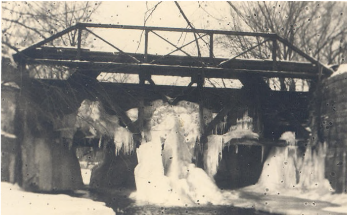
Two other undated photographs of the steel-frame aqueduct over Nettle Creek, possibly taken in the 1920s or early 1930s. Both views show the south side of the aqueduct and illustrate the vehicle bridge here. The downstream side of the bridge deck was carried by the Pratt Pony Truss.
