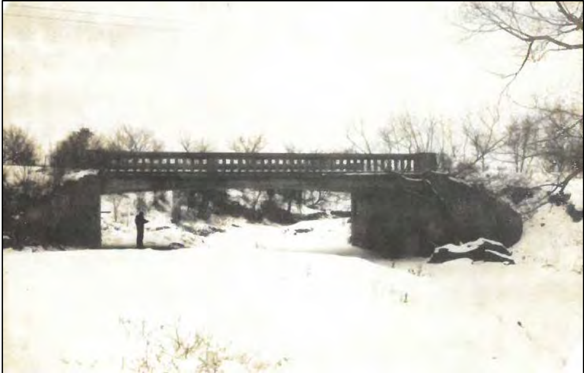
Figure 4: An undated, historic photograph of the bridge in winter. Image provided by Michael A. Maxey, P.E., Fayette County Engineer, to John N. Vogel, Ph.D., Heritage Research, Ltd. (HRL), 12 April 2017 via e-mail, Copy on file at HRL, Menomonee Falls, WI.
