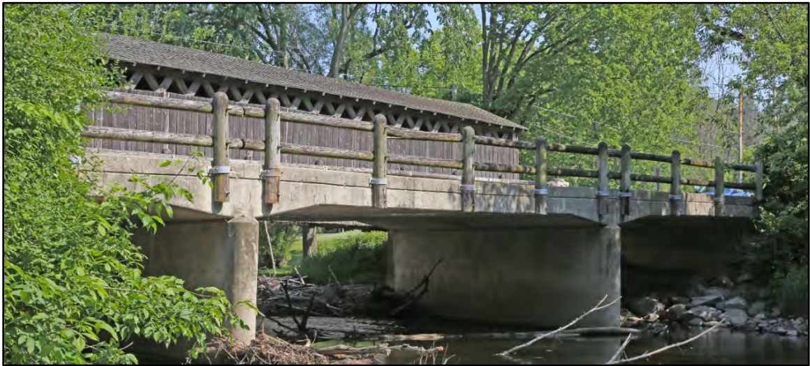
Figure 3: This bridge is located in Ozaukee County, Wisconsin. The haunched slab structure in the foreground replaced the covered bridge behind in 1962. The center span is 43'-10" long. The consistent depth of the slab's greater length is 14". That of the haunch over the piers is 24" and tapers to the 14" depth within 6' 6" of the piers' center.
