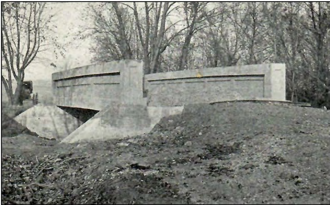
Newly built 1907, reinforced concrete, through girder, Heepke bridge, Madison County, IL.
