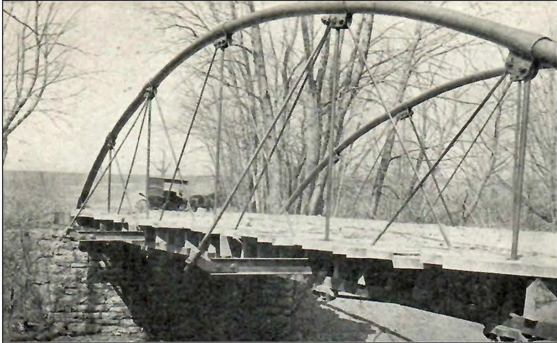
Original Late 19 th century, bowstring truss, Heepke bridge, Madison County, IL.
