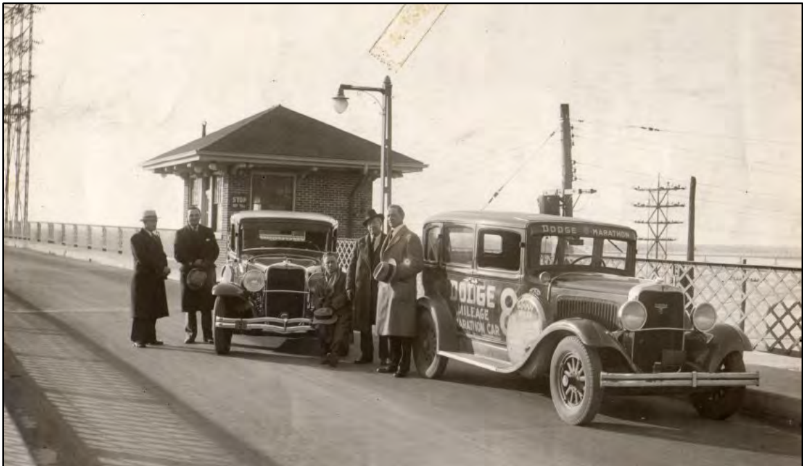
Figure 9: The toll house actually built was located on the north side of the bridge, between Front and Second streets. One reason a more practical, less expensive building was constructed was that it would likely be removed once the bridge no longer charged a toll. The house had a hipped roof, walls of brick, five-light-over-one-light windows and rose three stories from the ground ("Quincy Memorial Bridge and Toll Booth," Object ID P583, Photographs, Historical and Genealogical Research, Historical Society of Quincy & Adams County, Quincy, IL).
