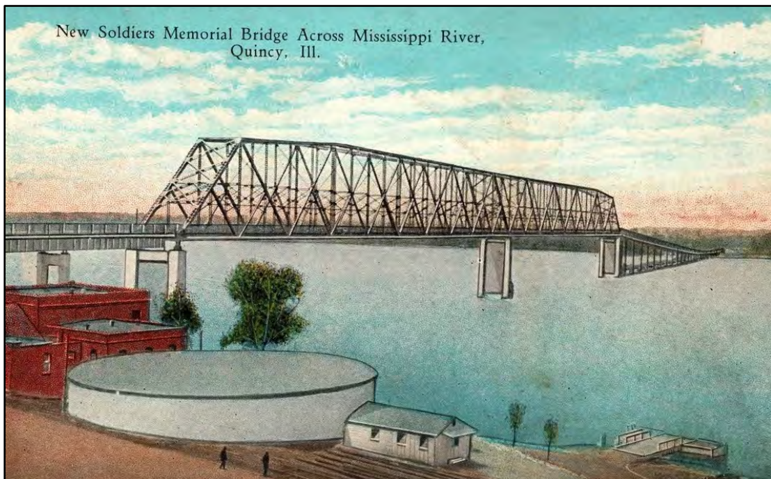
Figure 24: View of Memorial Bridge to the west southwest from the east bank of the river (“New Soldiers Memorial Bridge Across Mississippi River, Quincy, Ill [Chas. E. Wetzel, Quincy, Illinois, C.T. American Art, Colored, Kurt Teich, Chicago, Post Marked on 21 November 1933], Viewed at www.ebay.com on 08 December 2025).
