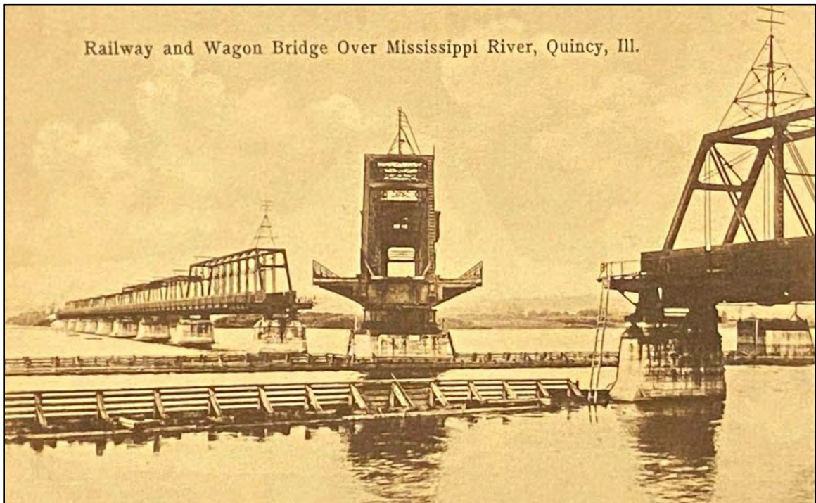
Figure 2: This undated postcard illustrates the CB&Q's bridge at Quincy as well as the two, 1899 vehicular travel lanes that flank it. Those lanes generated tolls between 1919 and 1930 for the railroad valued at over $250,000 ("Dream of Many Years Realized by City when New Memorial Bridge Opens to Traffic Without Ceremony: Old CB&Q Bridge Passed From Activity at Noon Saturday," Quincy (IL) Herald-Whig , 15 June 1930, 11; "Railway and Wagon Bridge over Mississippi River, Quincy, Ill" [Quincy, IL: C.H.P., Importers and Publishers, no date]: postcard, Viewed at www.ebay.com on 07 July 2021).
