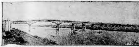
Dear Street Bridge across Illinois River at Peoria, Ill., cost $1,250,000.
